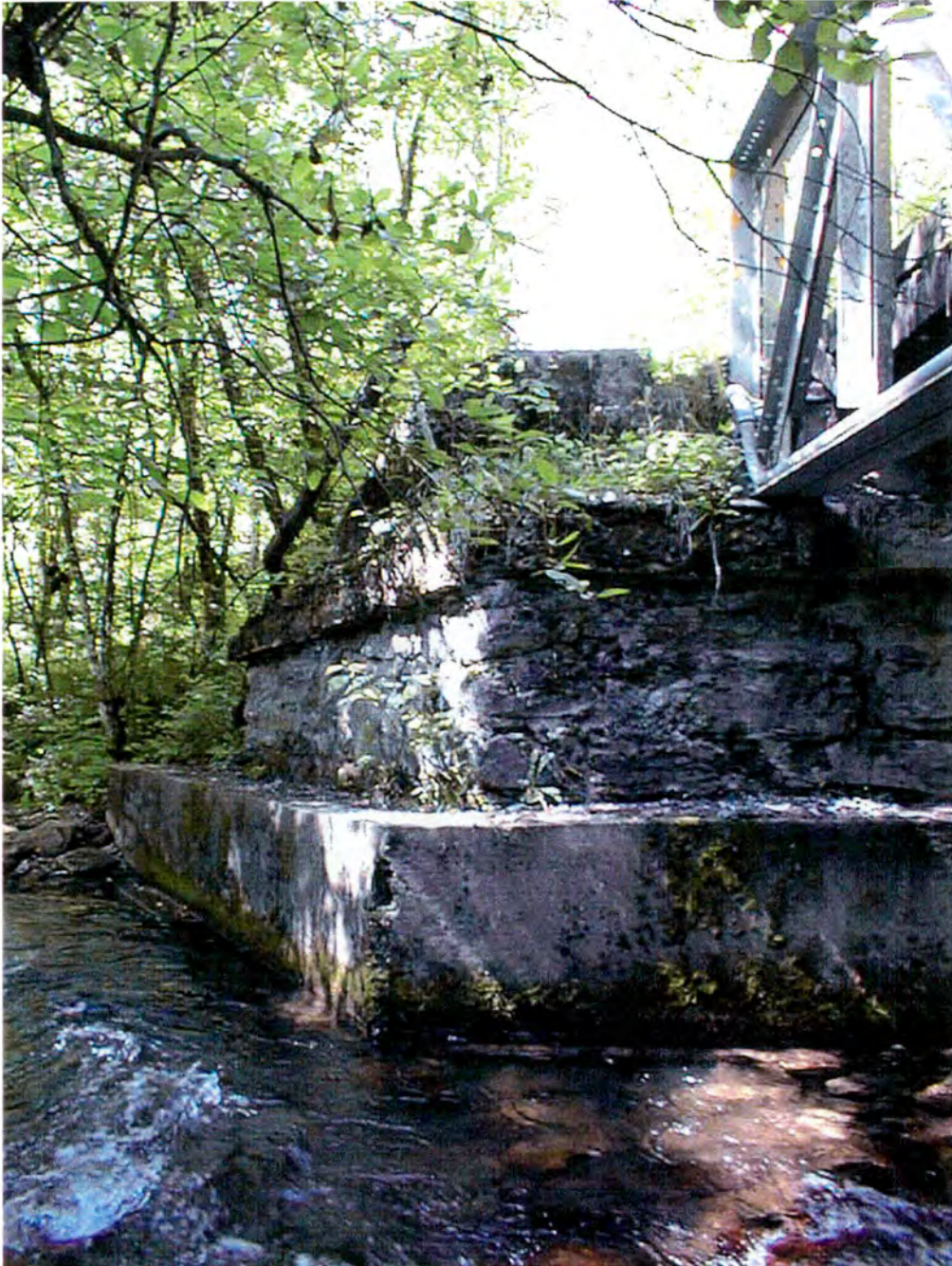
Plate 6: Bridge No. 1 stone abutment showing concrete support wall addition. View SW
