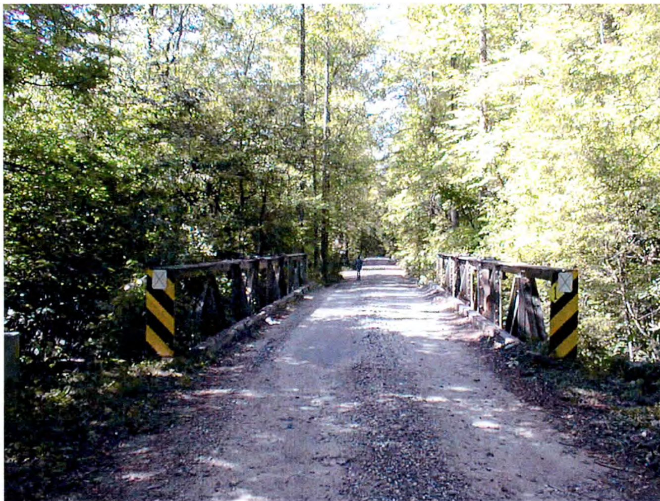
Plate 4: Avery Creek Bridge No. 1. View SW
