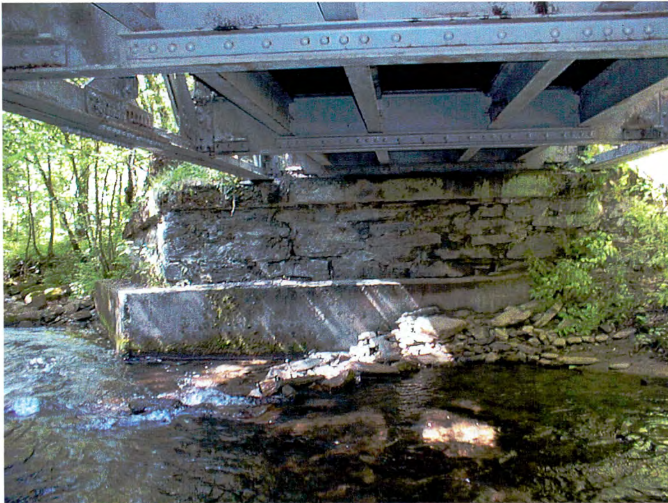
Plate 5: Bridge No. 1 stone abutment. View S
