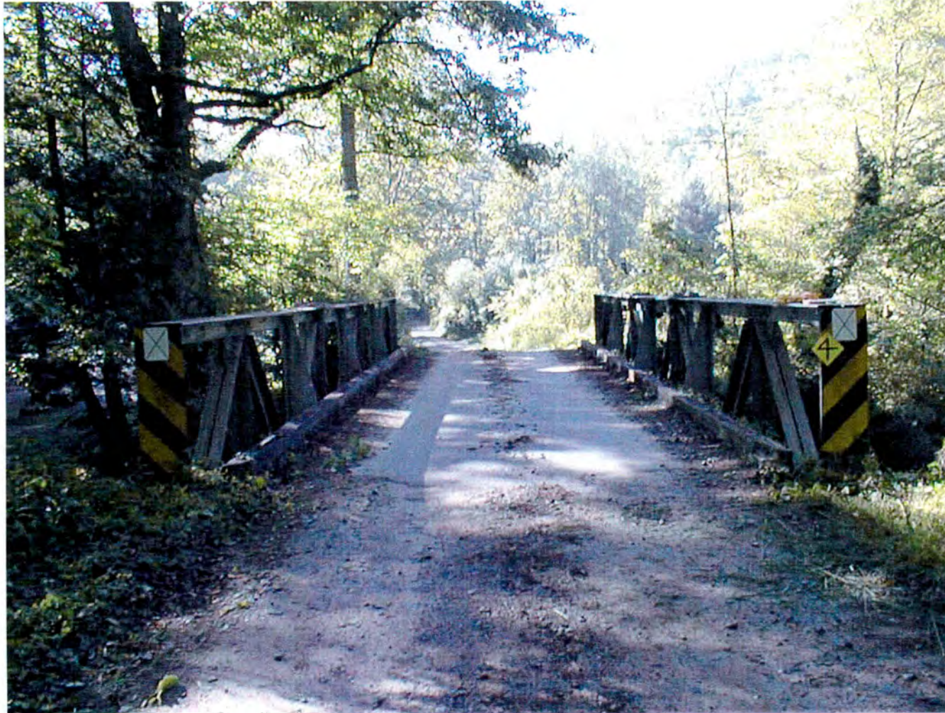
Plate 11: Avery Creek Bridge No. 4. View S.
