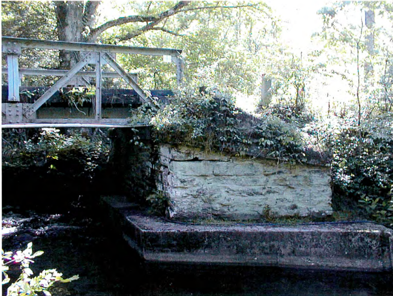
Plate 14: Bridge No. 4, abutment showing concrete support wall. View SW
