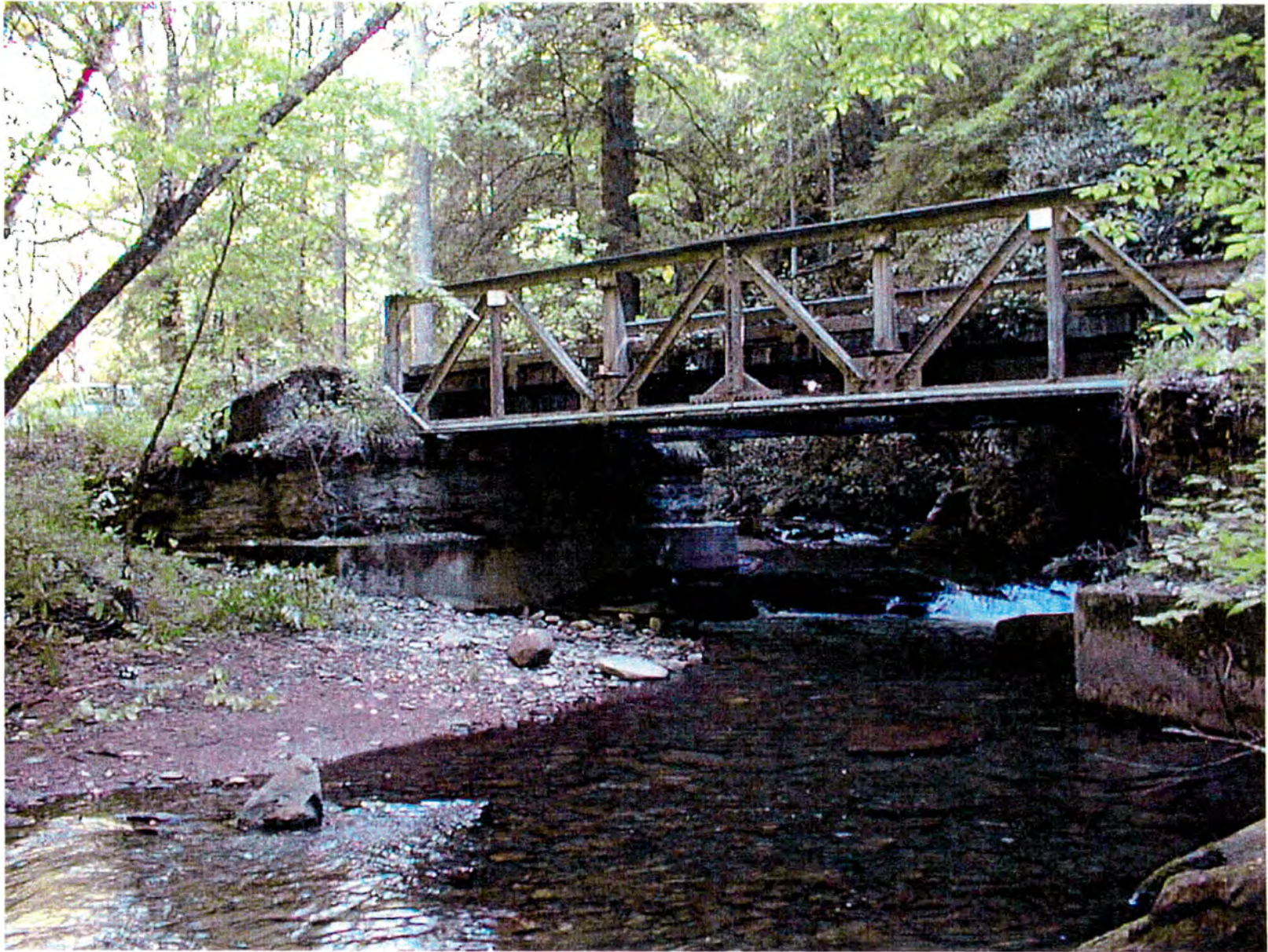
Plate 8: Avery Creek Bridge No. 2. View N.
