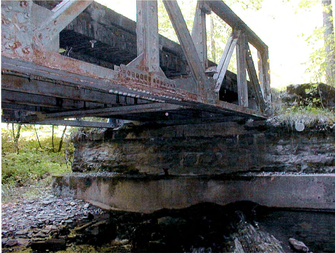
Plate 9: Bridge No. 2, abutment wall. View W.
