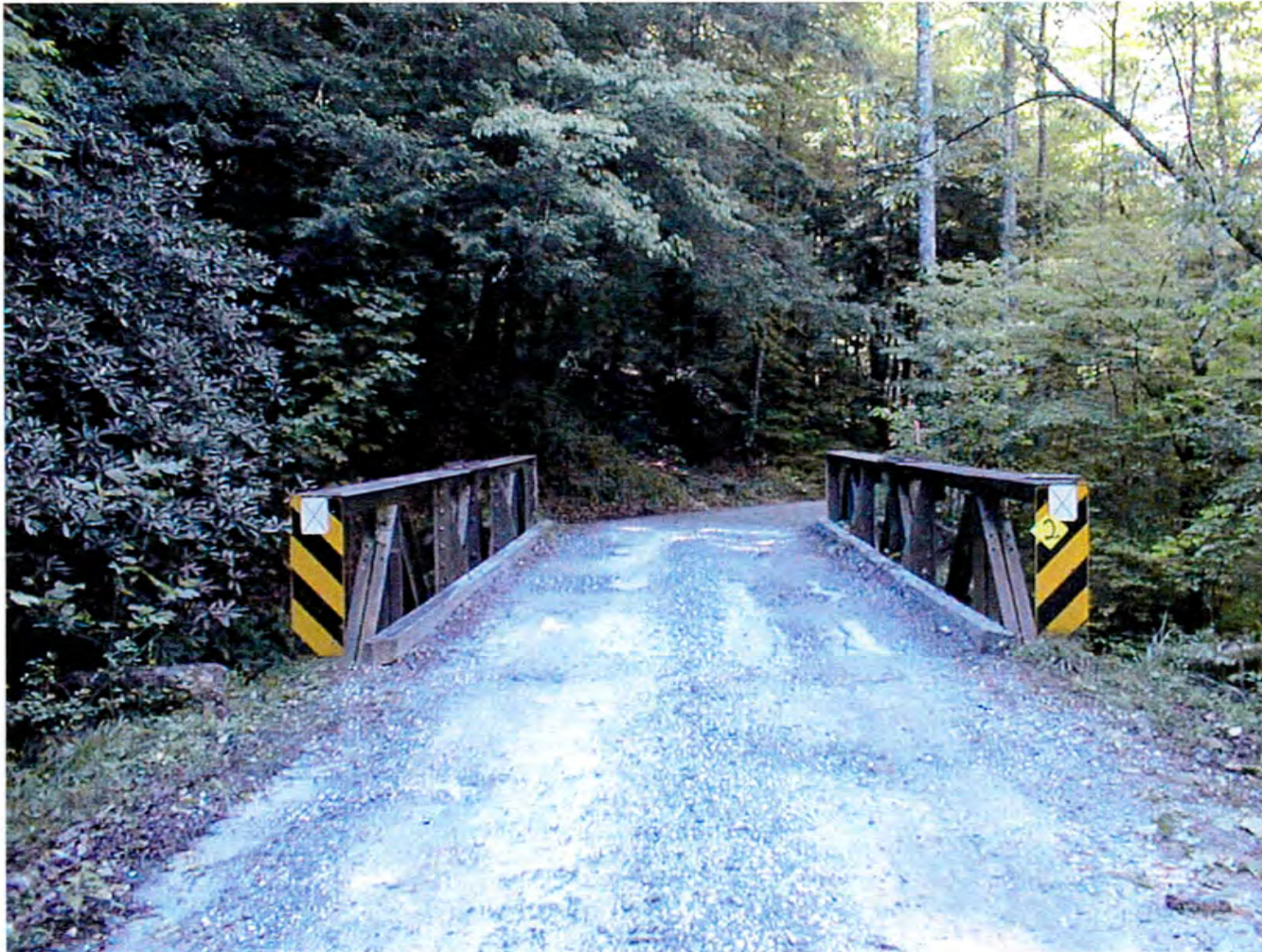
Plate 7: Avery Creek Bridge No. 2. View E.
