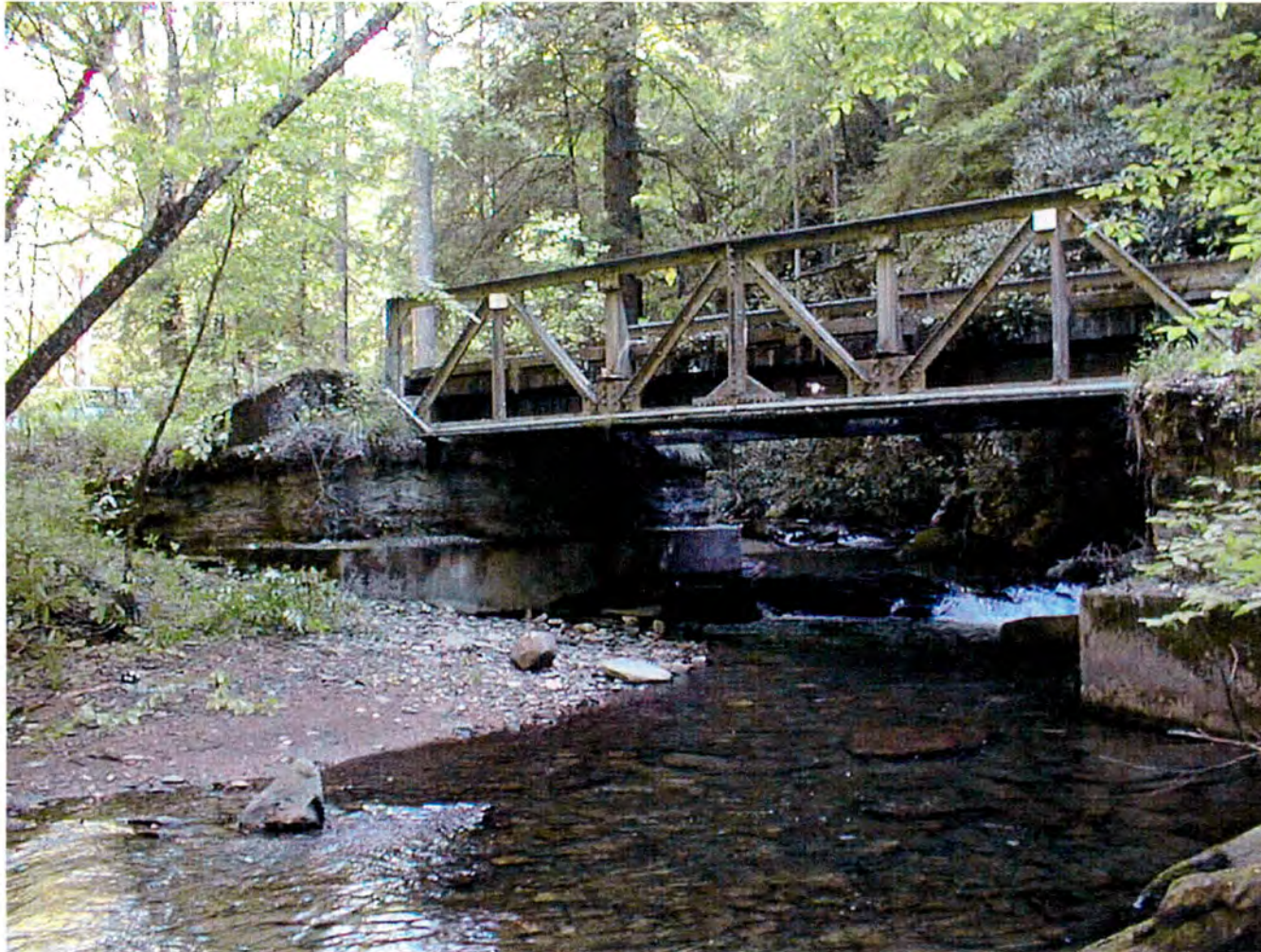
Plate 1: Avery Creek metal truss bridge
