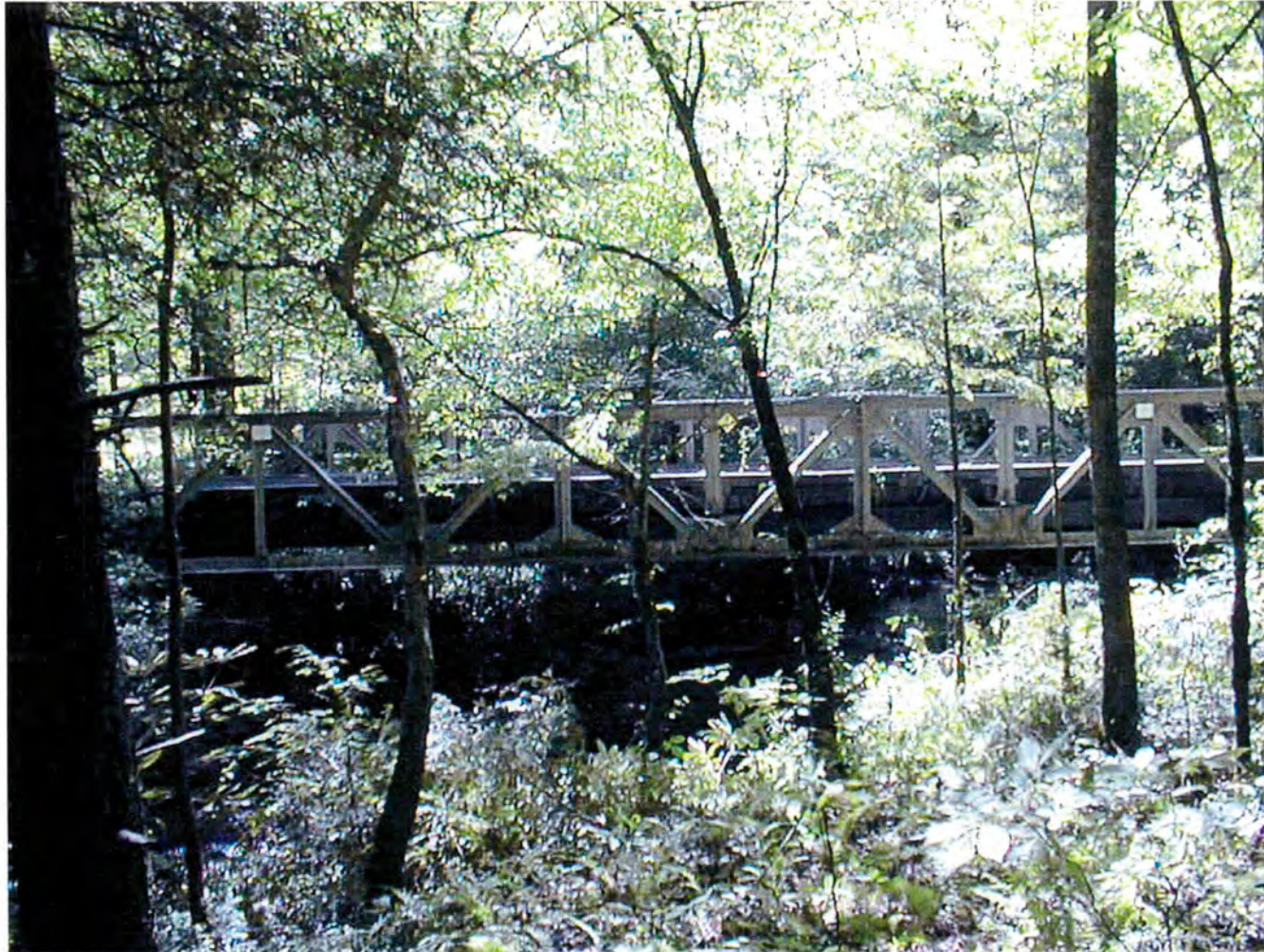
Plate 12: Avery Creek Bridge No. 4. View E.
