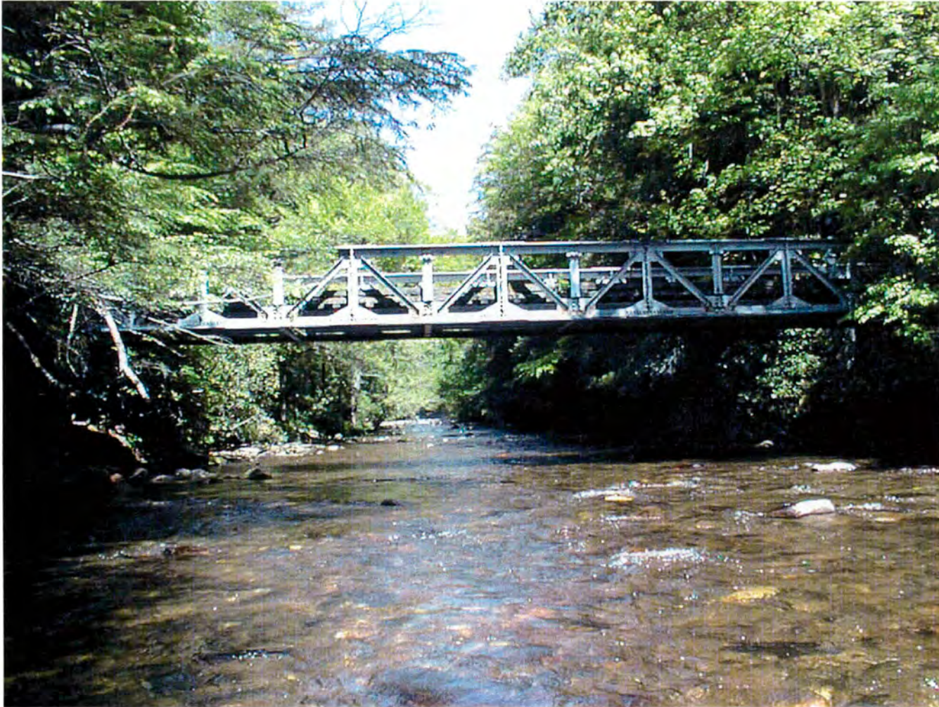
Plate 15: English Chapel Bridge. View NW.
