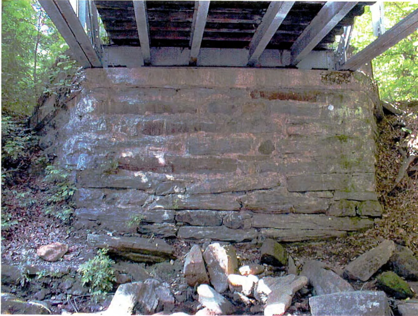
Plate 17: English Chapel Bridge, abutment wall. View E.
