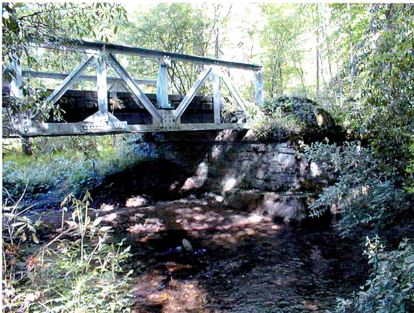
Plate 13: Bridge No. 4, abutment wall. View E.
