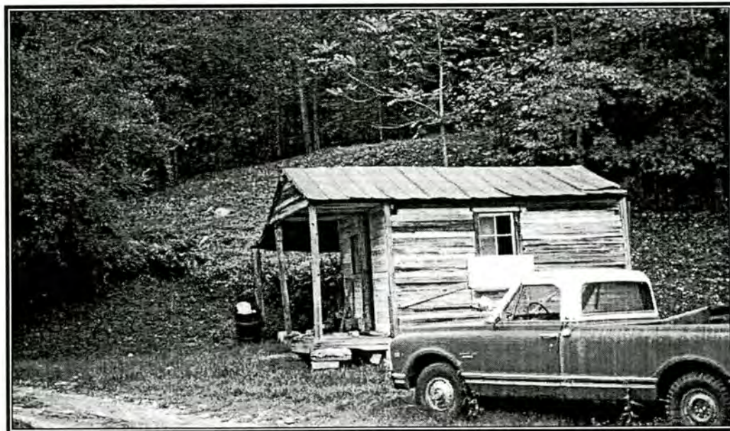
Photograph 4: Outbuilding, Property No. 3
