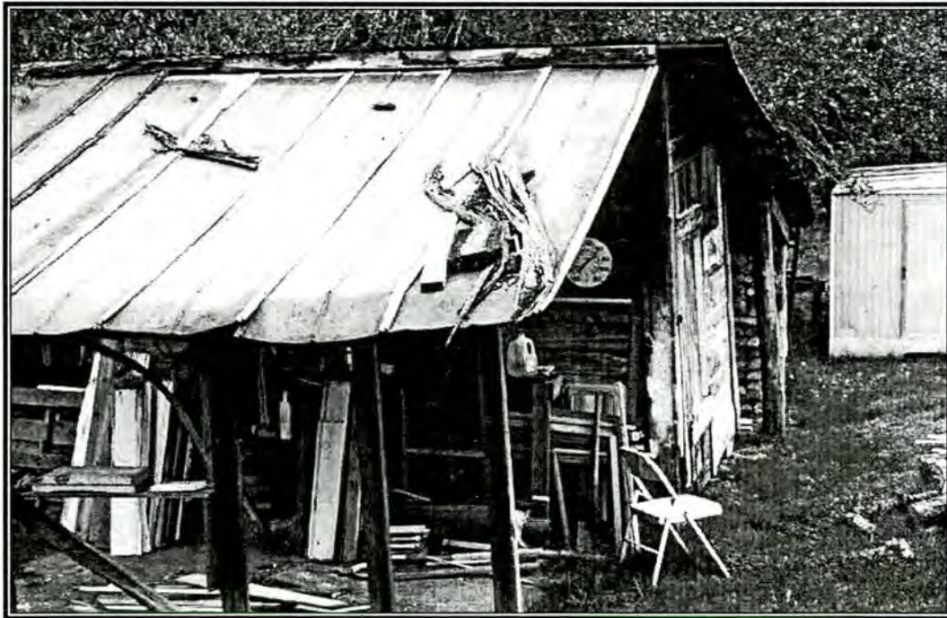
Photograph 6: Shed, Property No. 1
