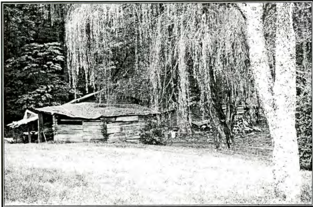
Photograph 3: Barn, Property No. 3
