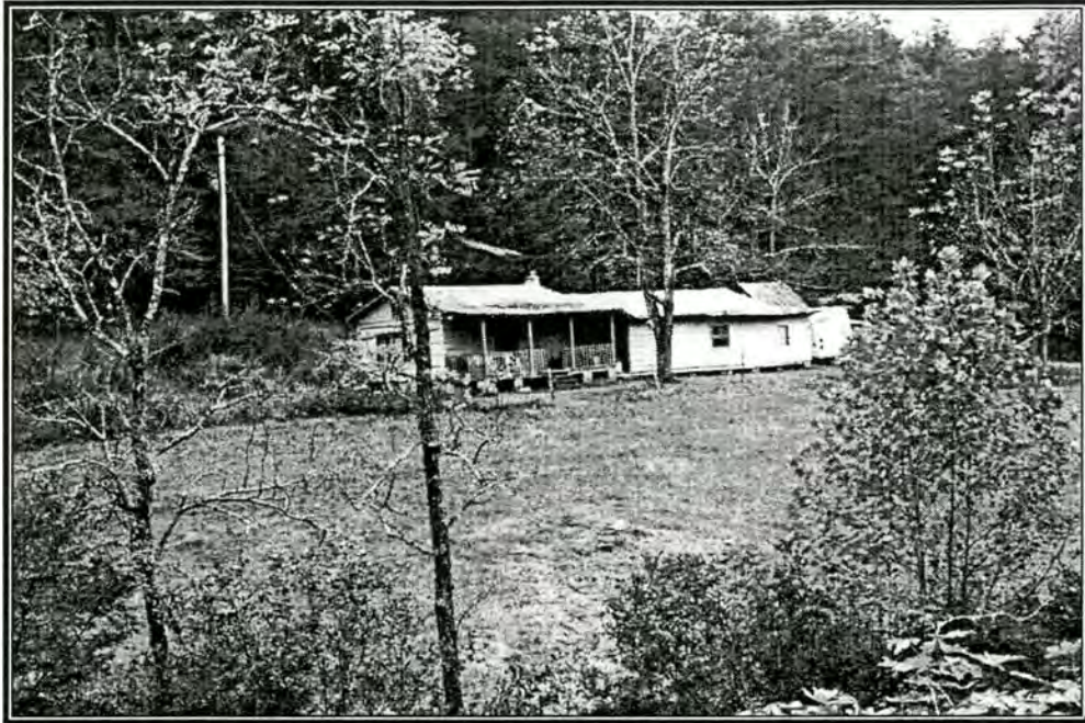
Photograph 1: Reconstructed Log House, Property No. 2
