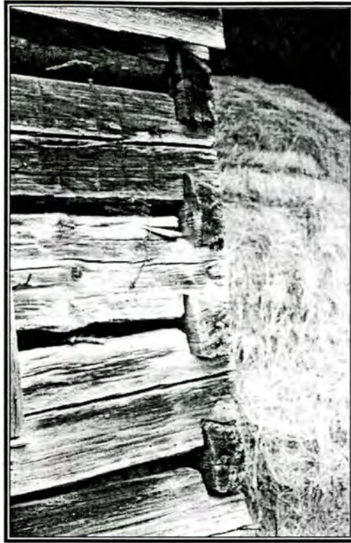
Photograph 9: Detail of Corner Notching, Log House, Sims-Melton Farm
