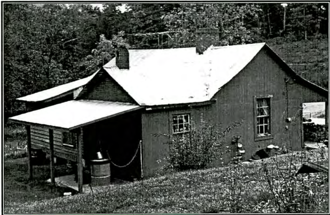
Photograph 2: Rear and Northeast Elevation, Frame House, Property No. 1
