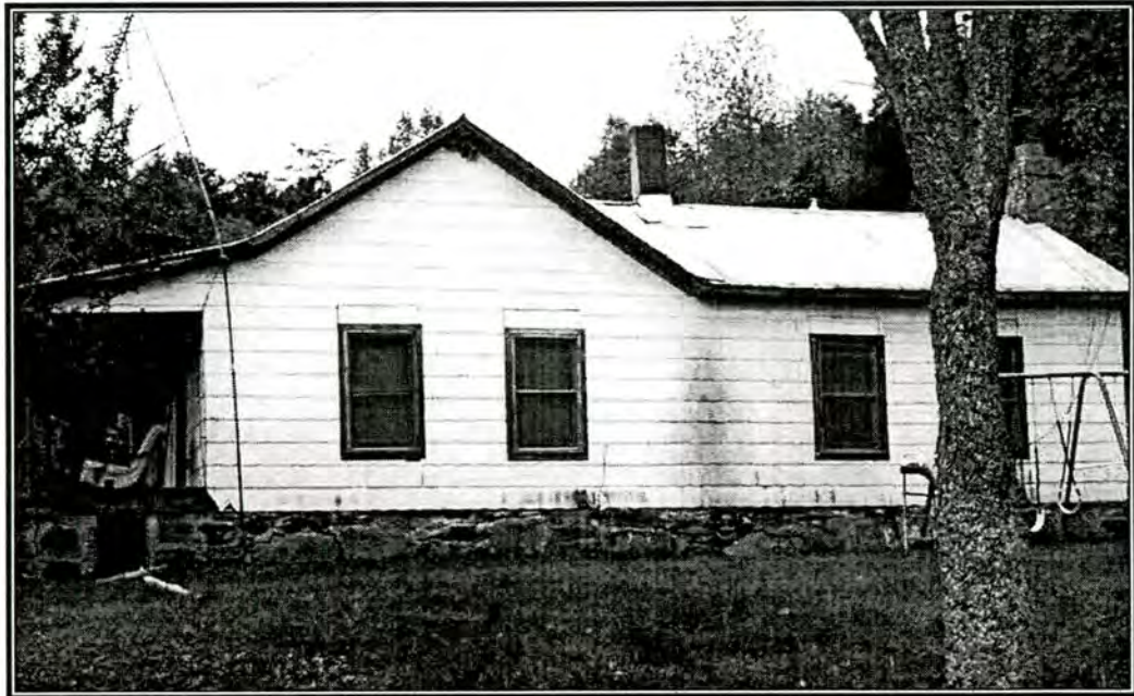
Photograph 2: North Elevation, Frame House, Property No. 3
