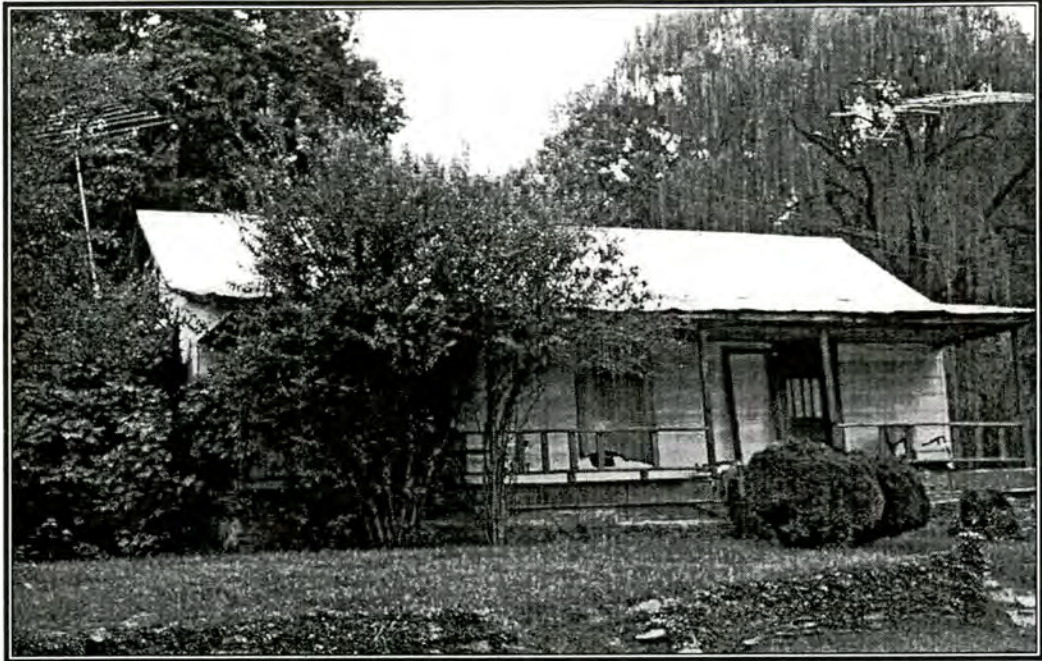
Photograph 1: Façade, Frame House, Property No. 3
