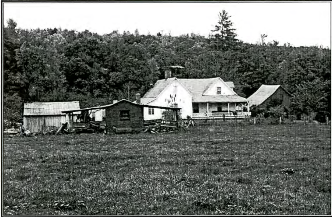
Photograph 3: Frame House, Barn to the right, Kitchen to the left, Sims-Melton Farm
