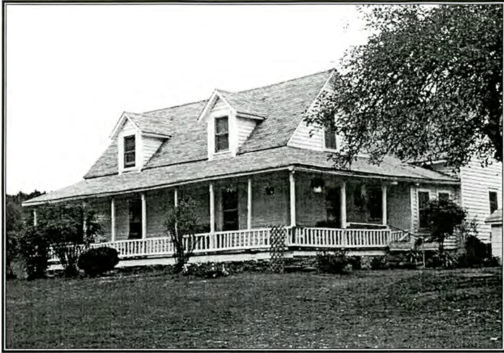
Photograph 1: Façade, Frame House, Sims-Melton Farm
