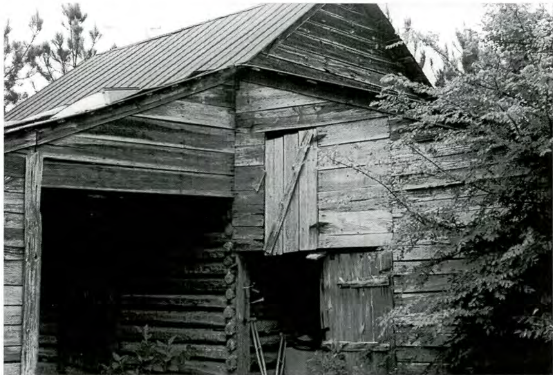
Figure 39: Property #15, William F. Cole Farm, log barn with shed additions
