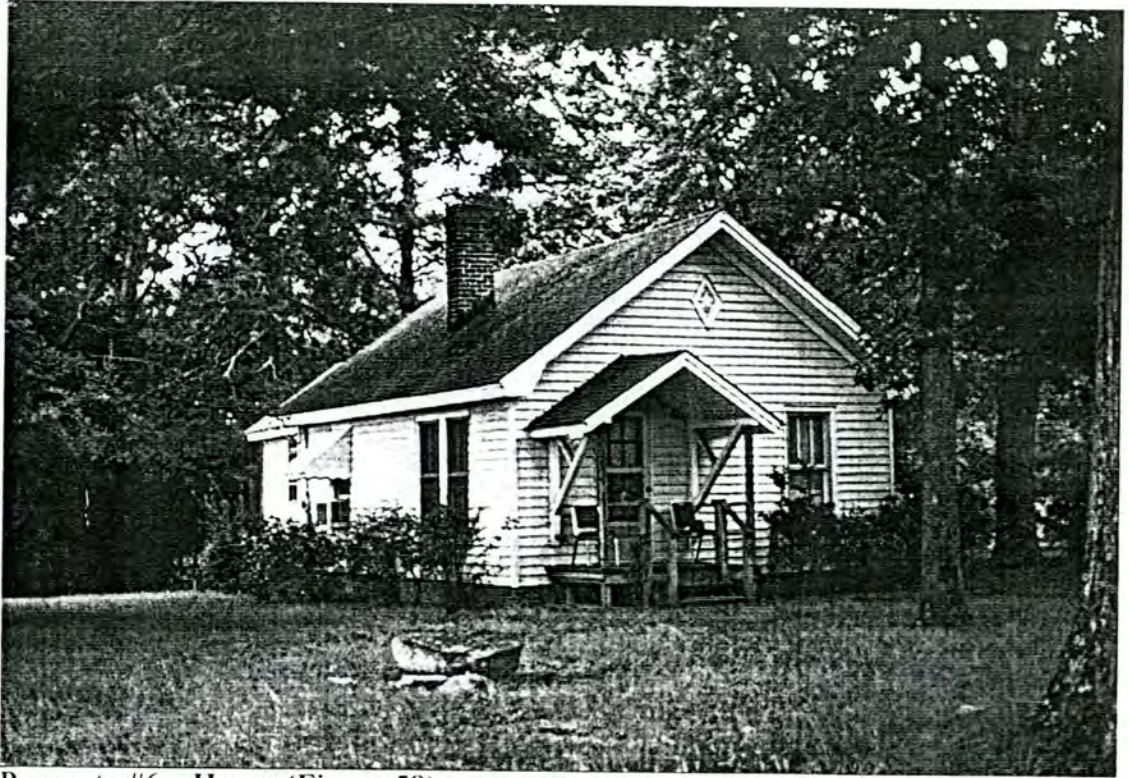
Property #6—House (Figure 58)
