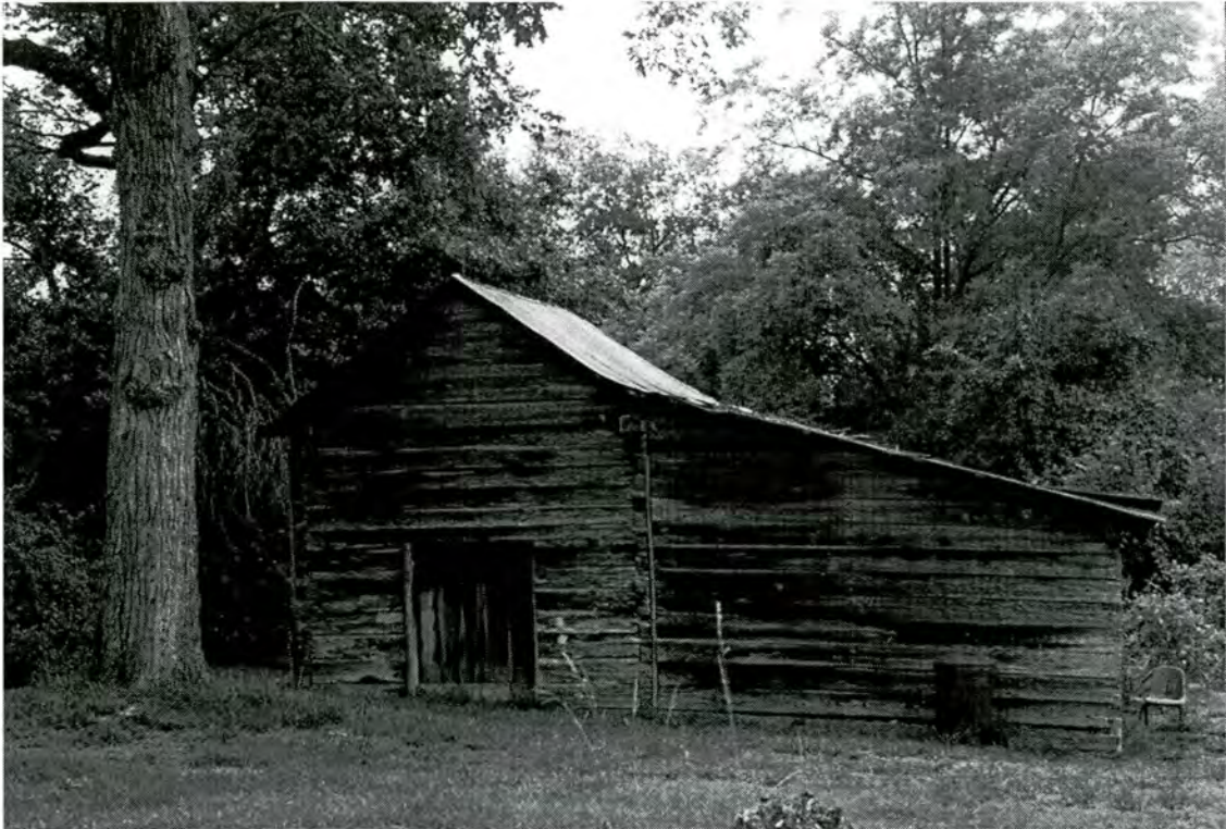
Figure 36: Property #15, William F. Cole Farm, plank outbuilding with shed addition
