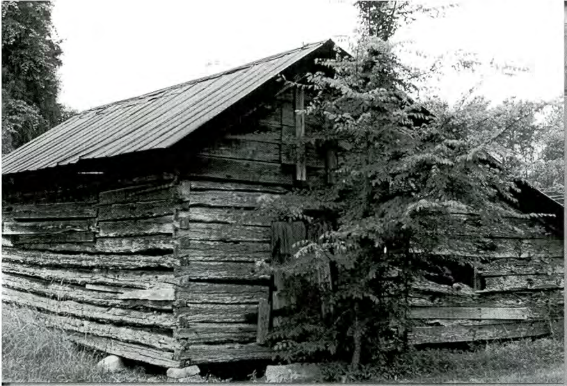
Figure 38: Property #15, William F. Cole Farm, plank outbuilding with shed addition
