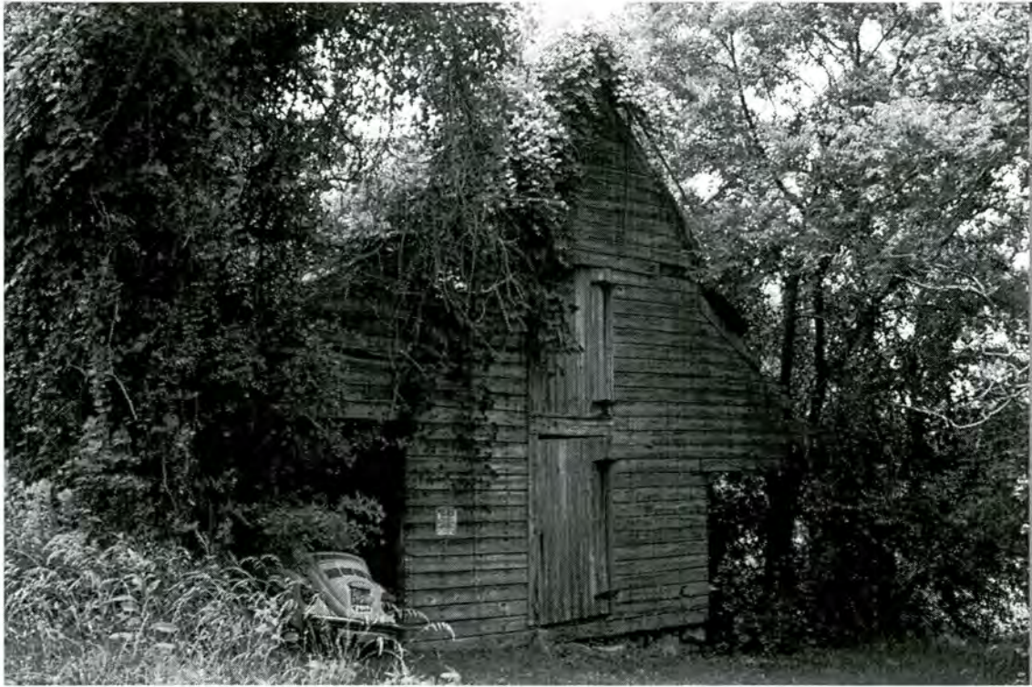
Figure 50: Property #16, Cole Farm, barn
