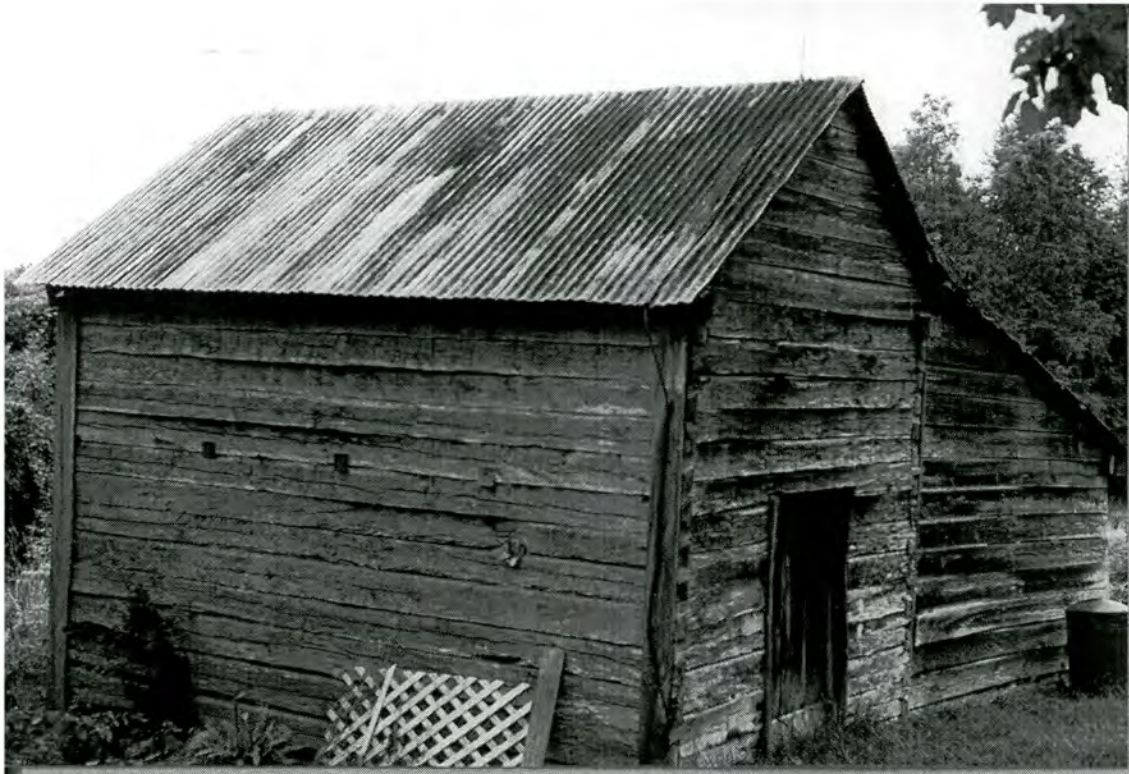
Figure 37: Property #15, William F. Cole Farm, plank outbuilding with shed addition
