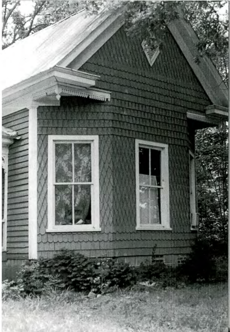
Figure 45: Property #16, Cole Farm, dwelling, front elevation, detail
