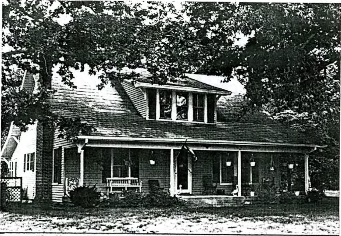
Property #9—House (Figure 59 )
