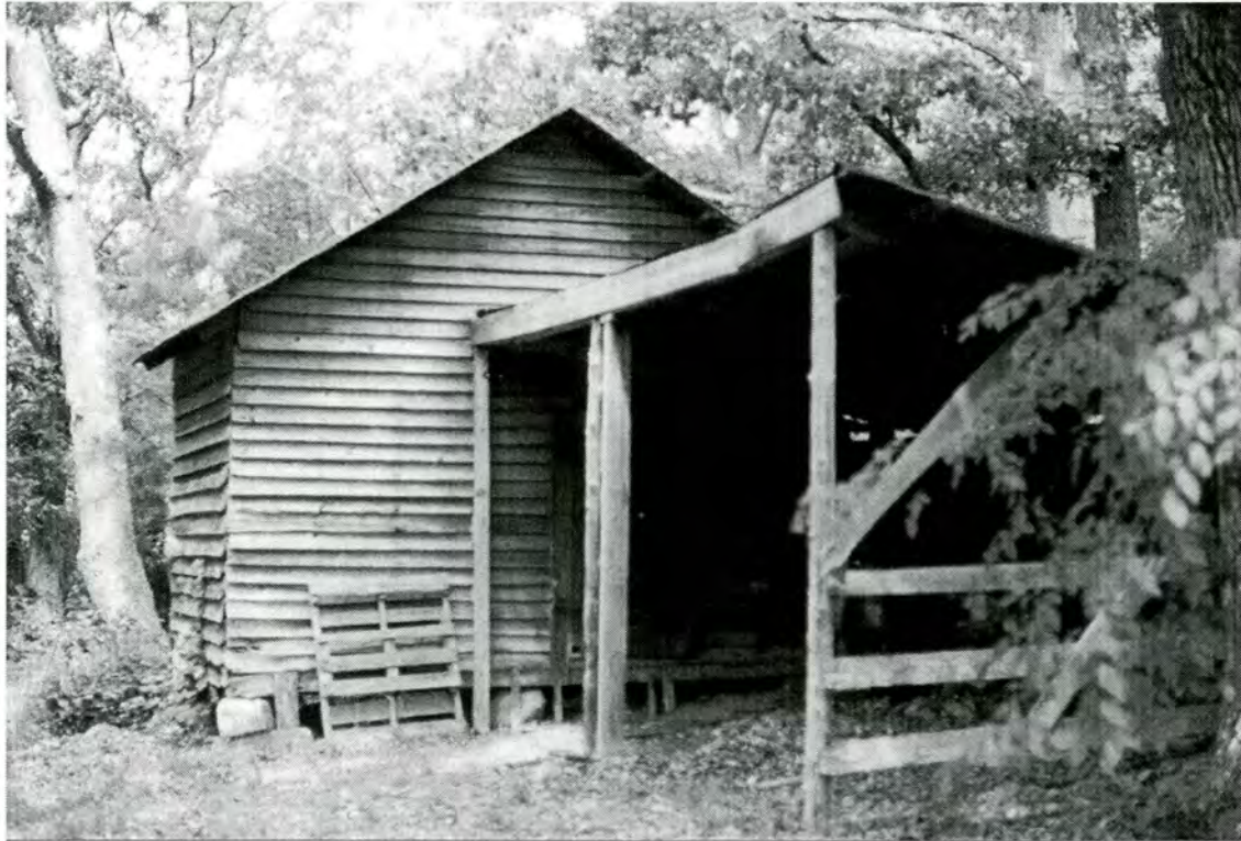
Figure 52: Property #16, Cole Farm, outbuilding with shed addition
