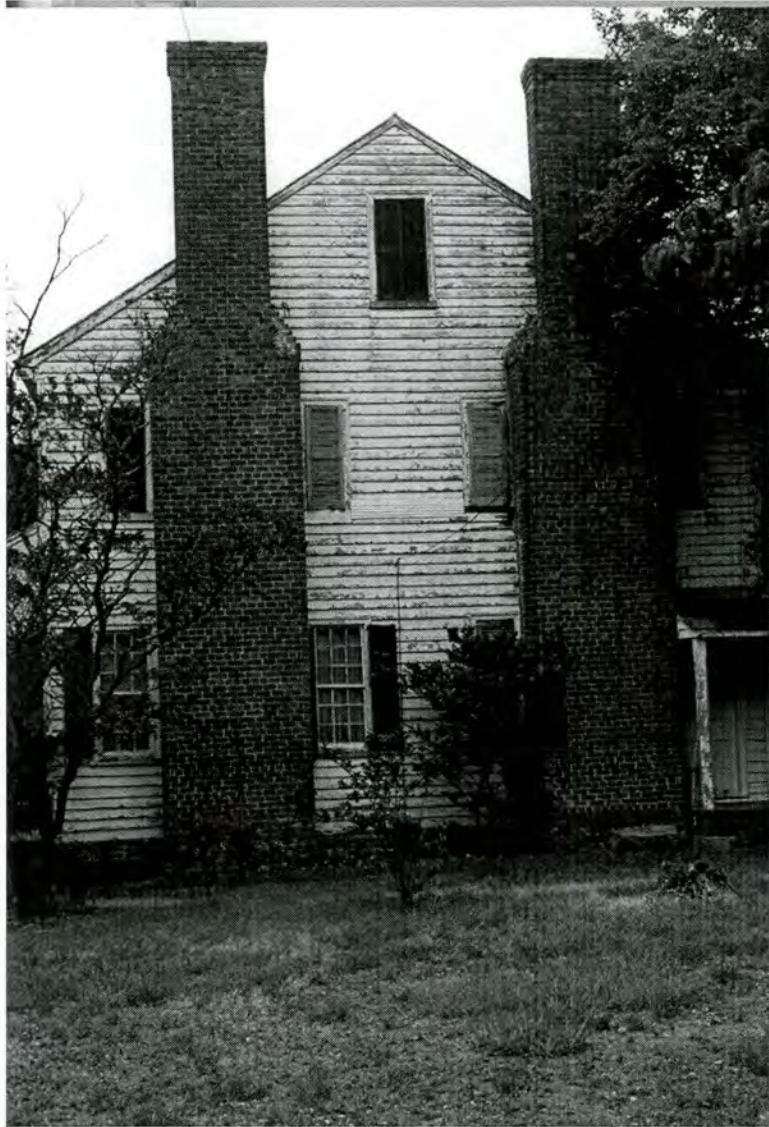
Figure 10: Property #7, Smith-Cole Farm, Smith-Cole House, north elevation
