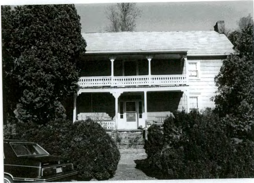
3. South front facade
