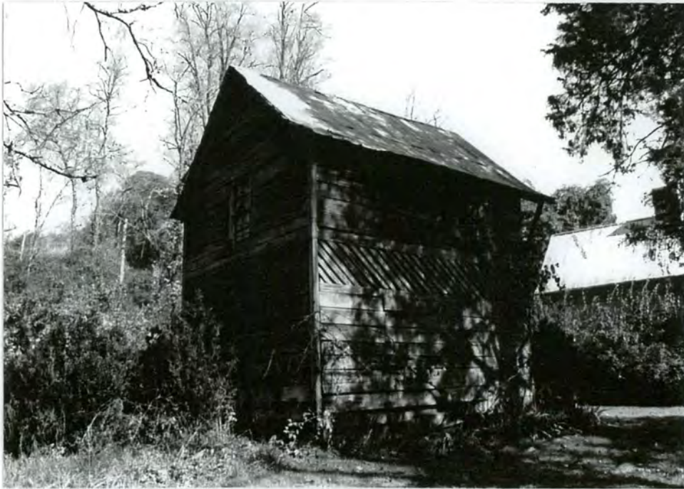
17. Rear and side facades of frame smokehouse
