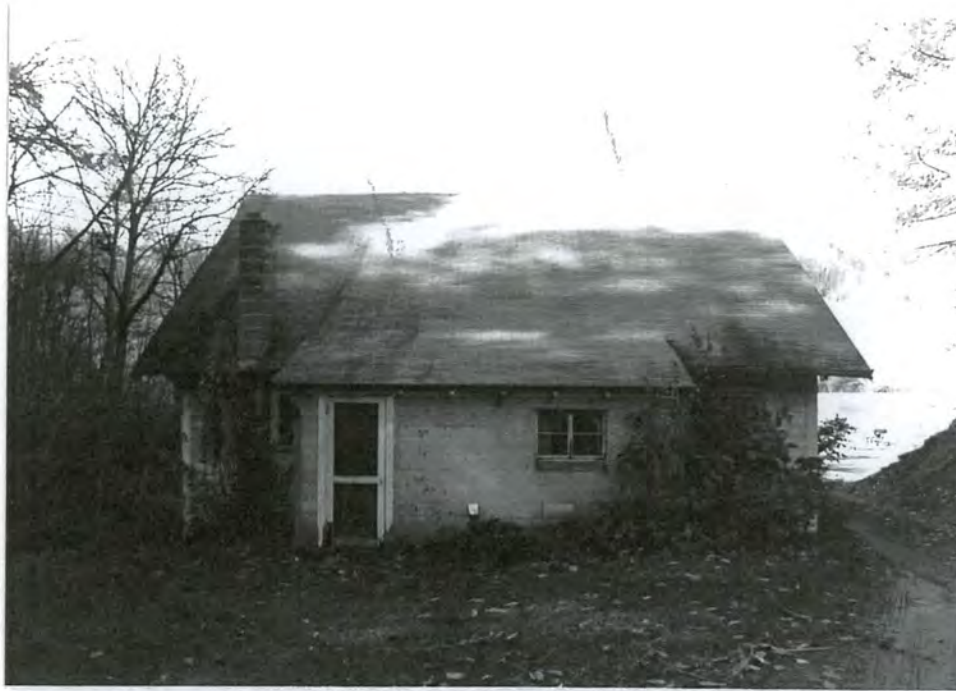
10. Southeast rear facade with concrete block shed addition
