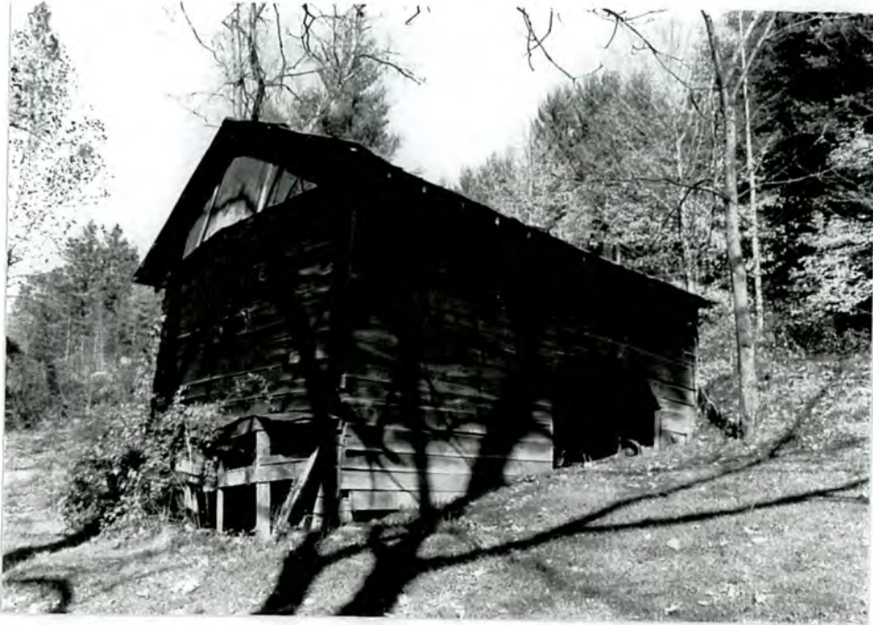
15. Frame equipment storage building
