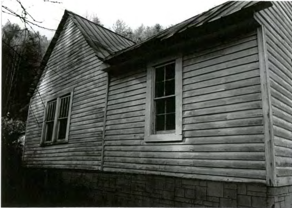
14. East facade of main section and front-gabled wing
