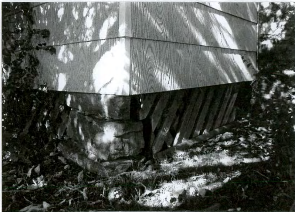
7. Detail of stone-pier foundation
