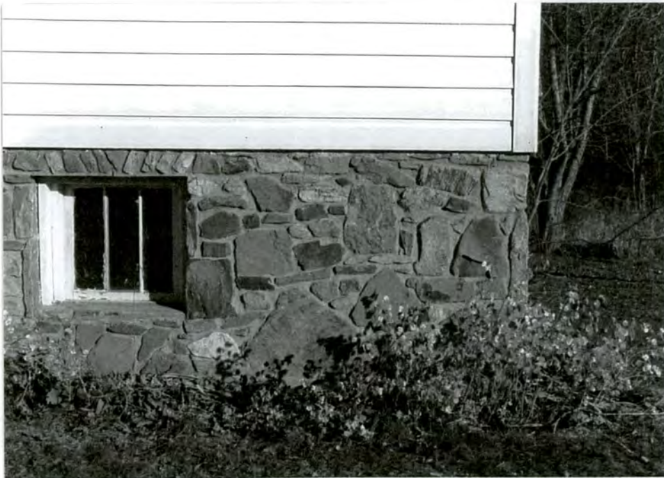
6. Detail of stone foundation
