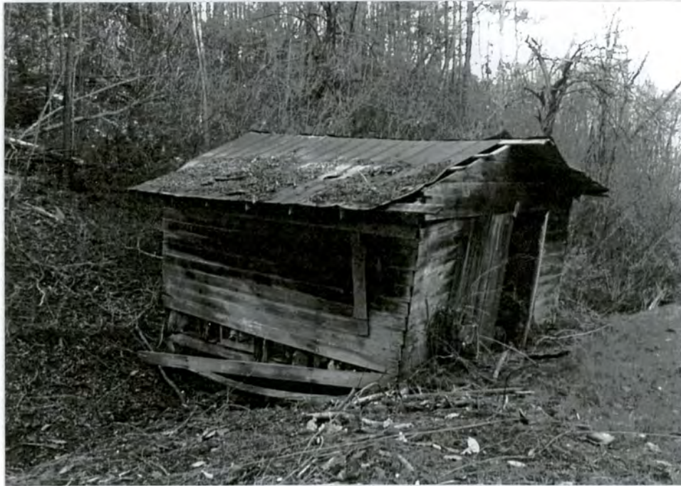
11. Small frame outbuilding spanning the creek bed
