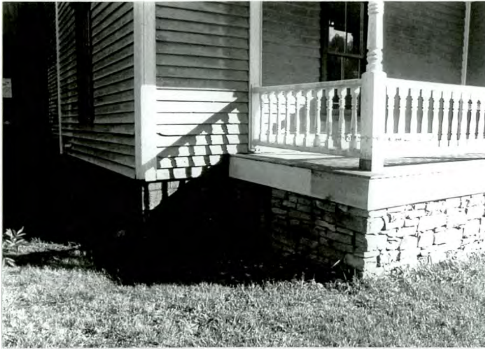
9. Detail of stone and concrete block foundation
