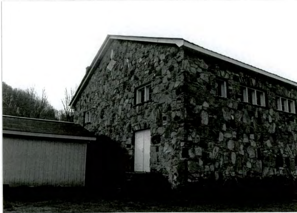
18. East rear facade of gymnasium
