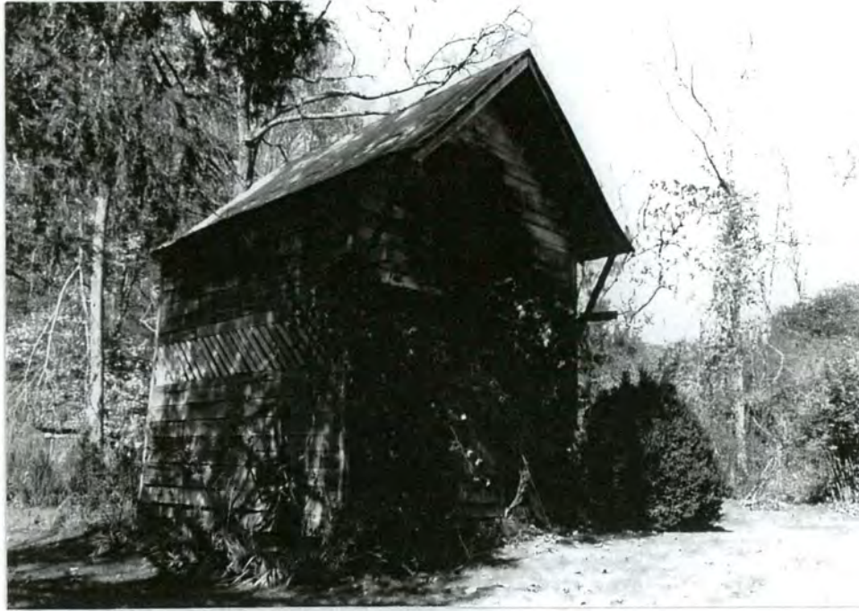
16. Front facade of frame smokehouse
