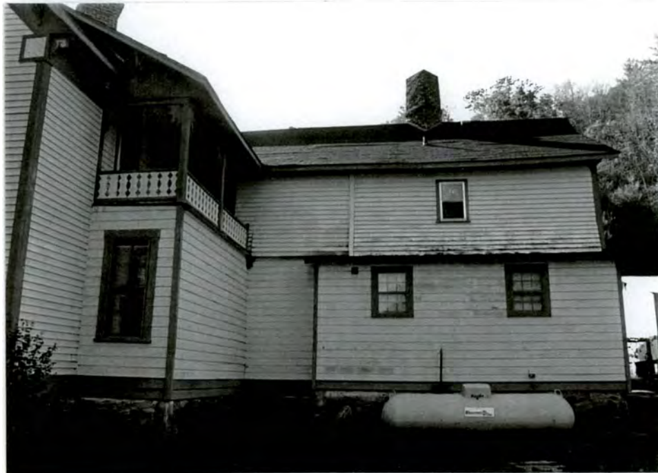
15. East side facade of rear wing and rear porch with enclosures
