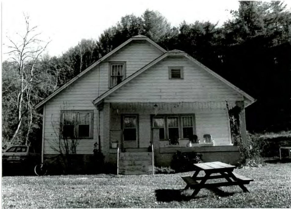
5. Northwest front facade
