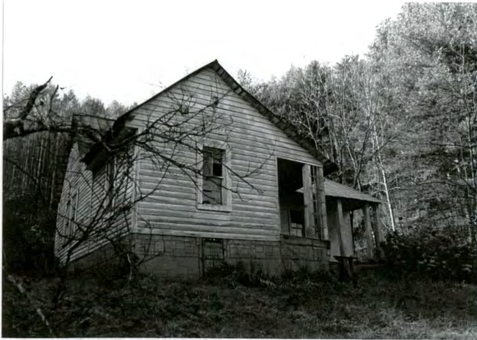
3. North front and east side facades
