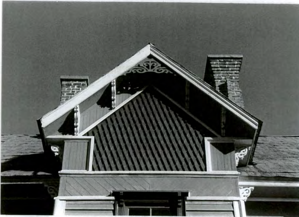
8. Detail of second-floor gable on projecting entrance bay
