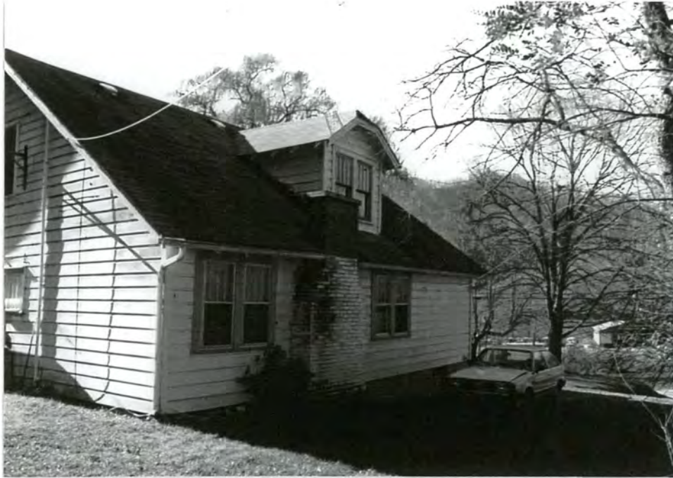
9. Northeast side facade
