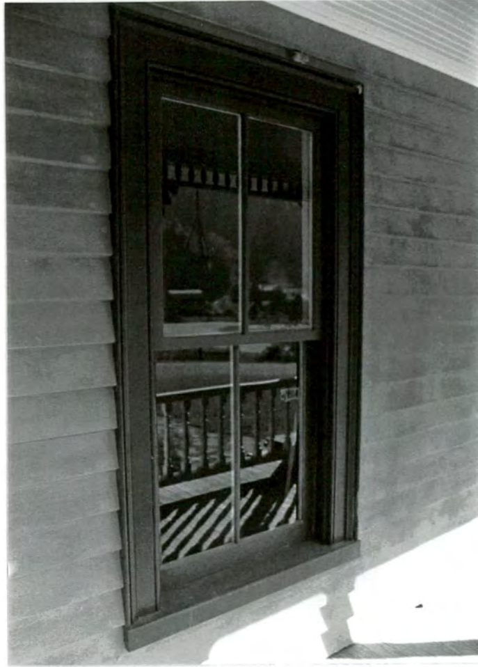
11. Detail of front facade window
