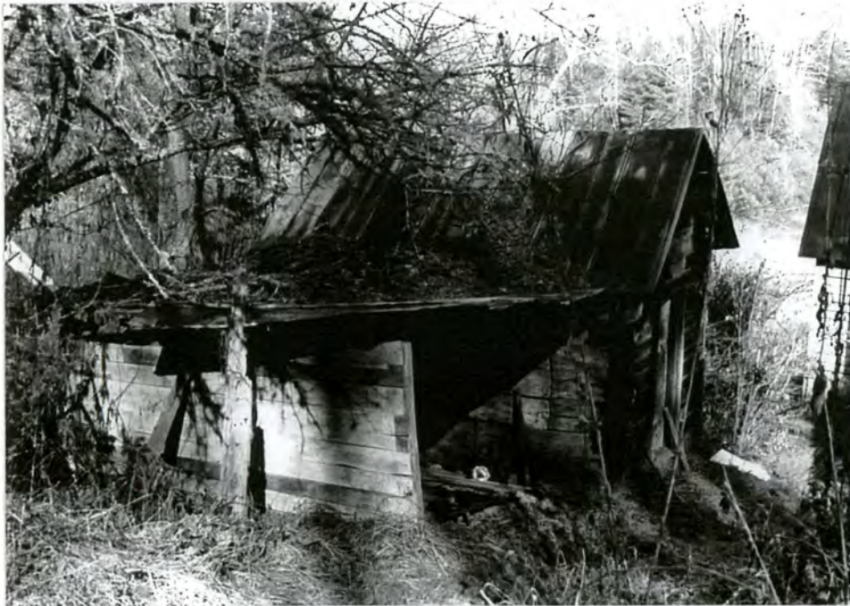
15. Frame storage building behind house
