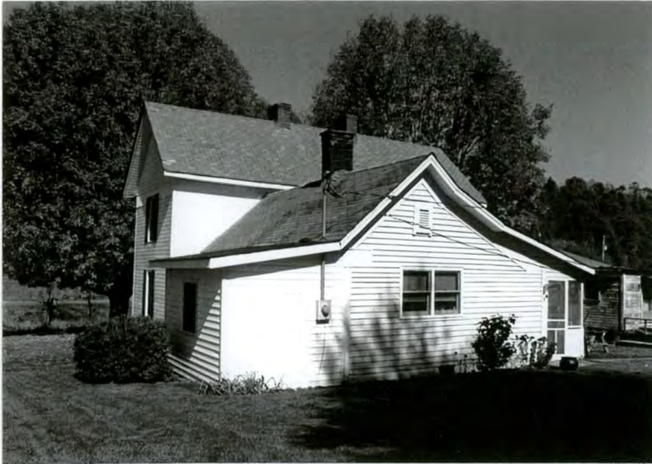
8. West side and south rear facades showing rear wing and addition
