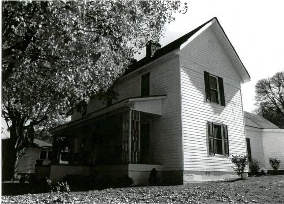
3. North front and west side facades
