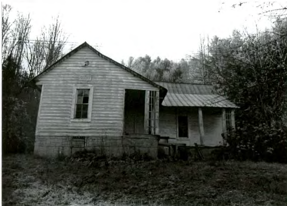
4. North front facade showing main section and front-gabled wing
