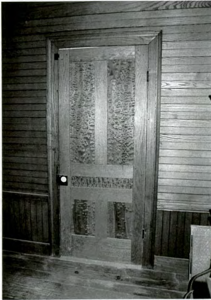
19. Detail of interior door showing use of various woods
