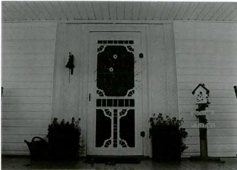
4. Detail of main entrance on front porch; note artificial siding
