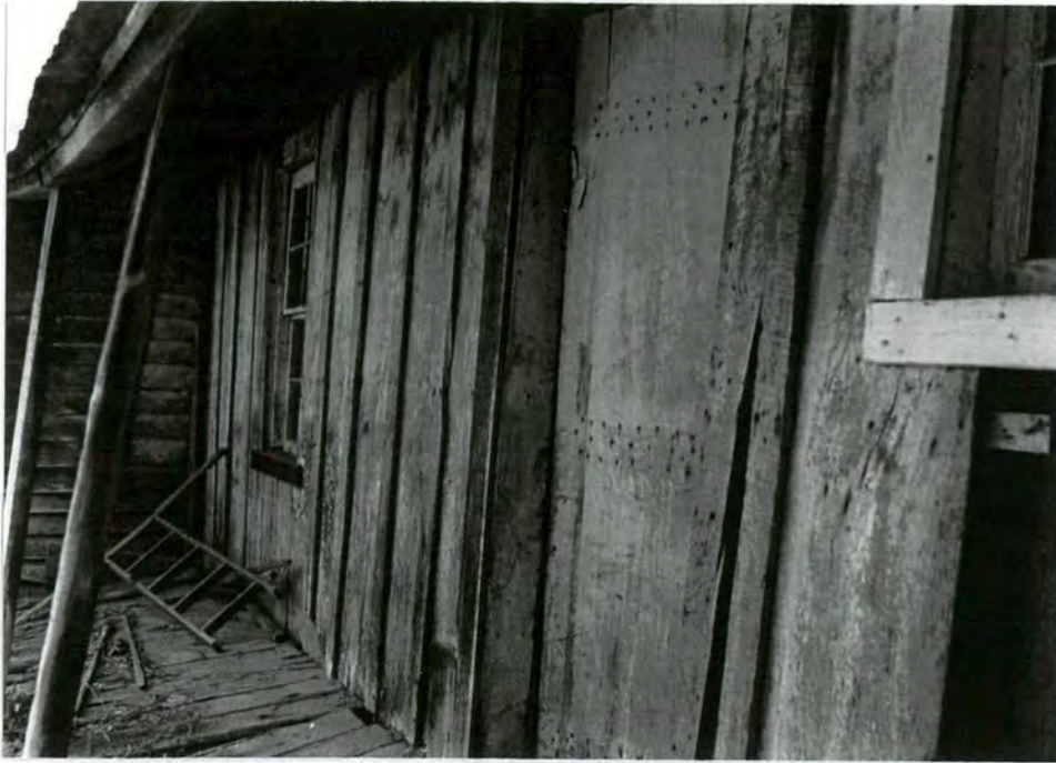
11. Detail of west facade of rear wing
