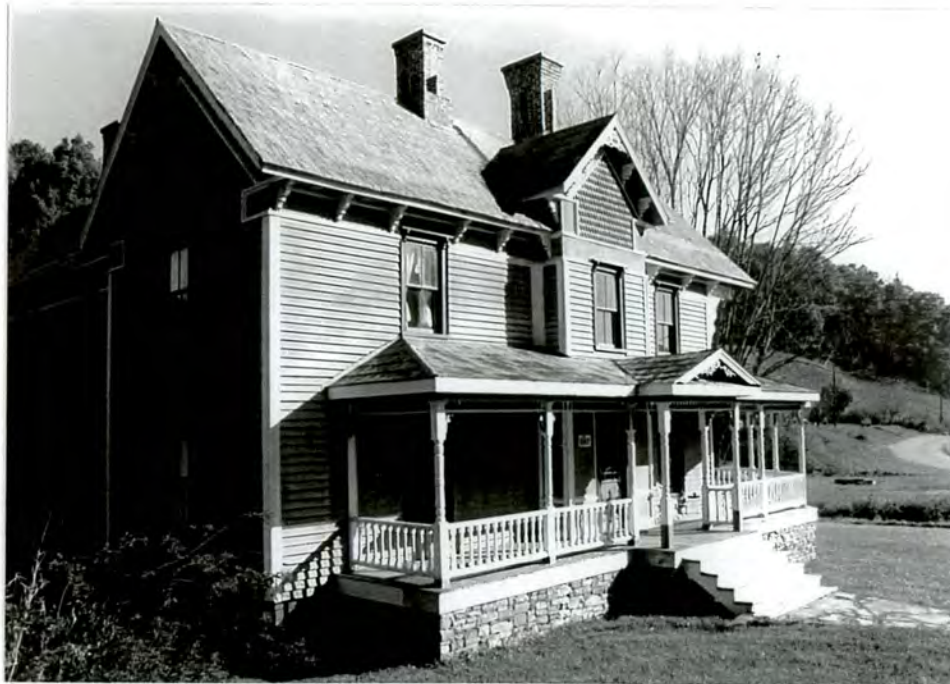
6. South front and west side facades
