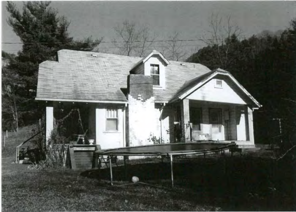
7. Southwest side facade
