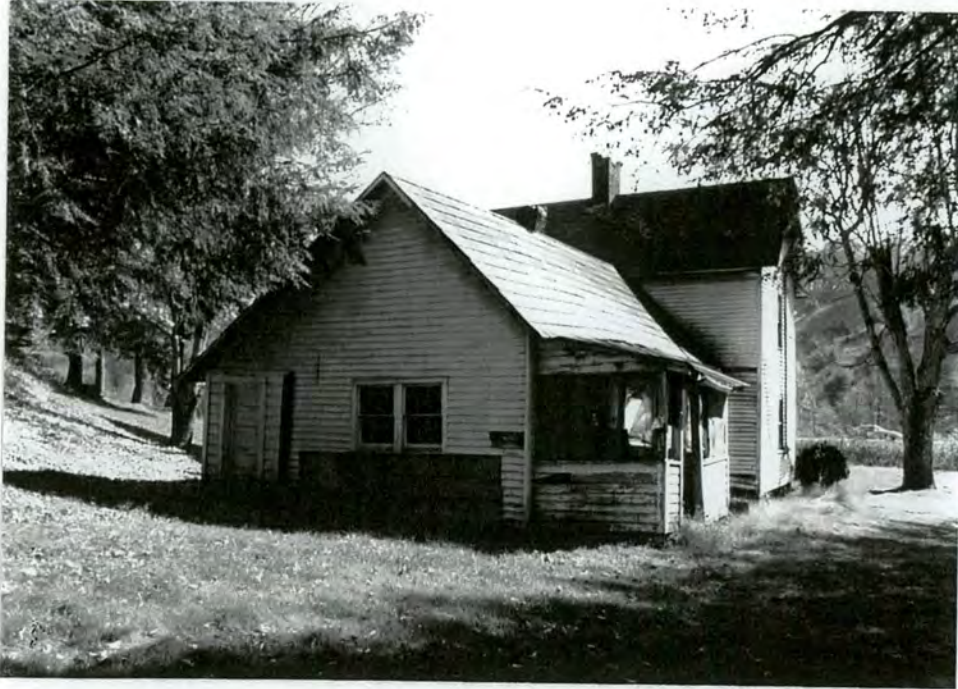
10. North end facade of rear wing
