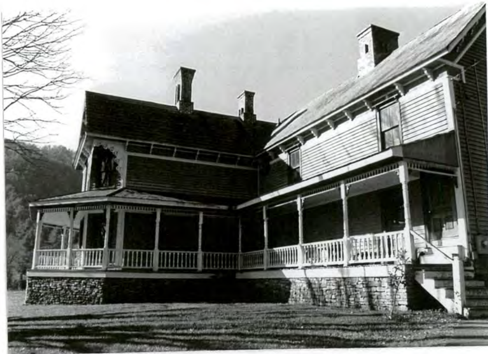
12. East side facade showing rear wing
