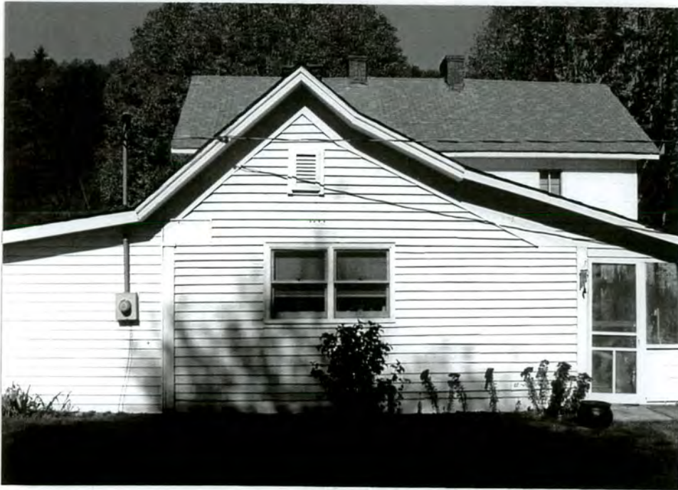
9. South end facade of rear wing with original weatherboard siding visible
