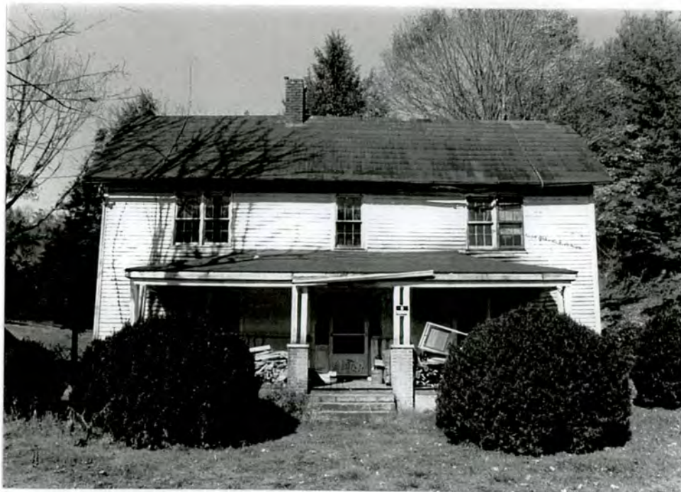
2. South front facade
