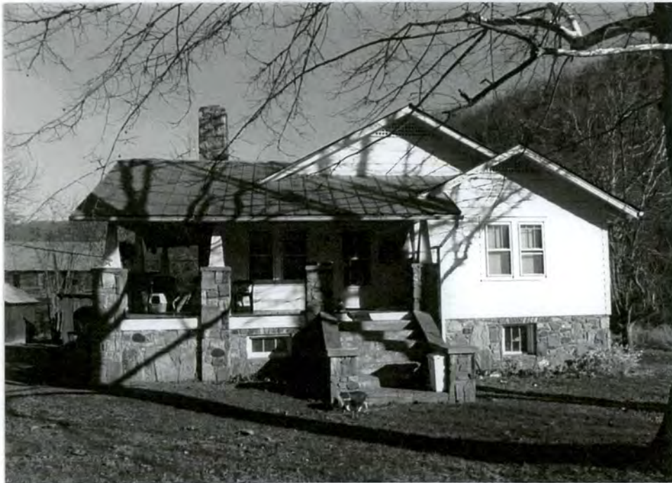
4. Northwest front facade
