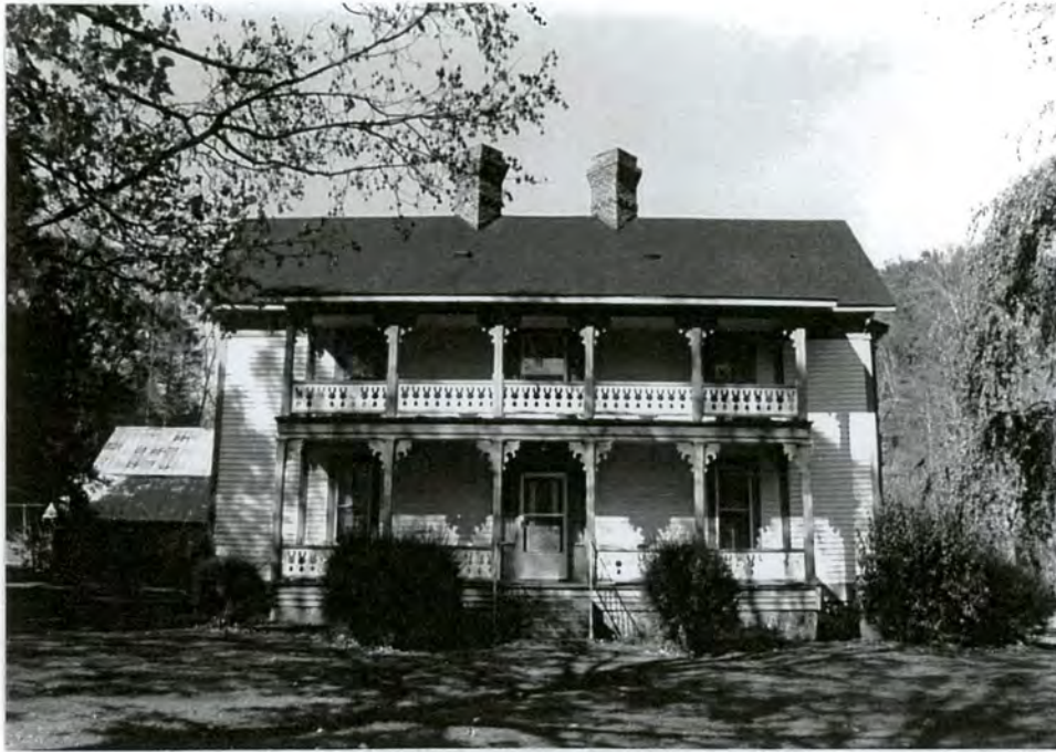
3. South front facade
