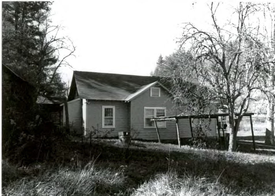
8. Northeast side facade
