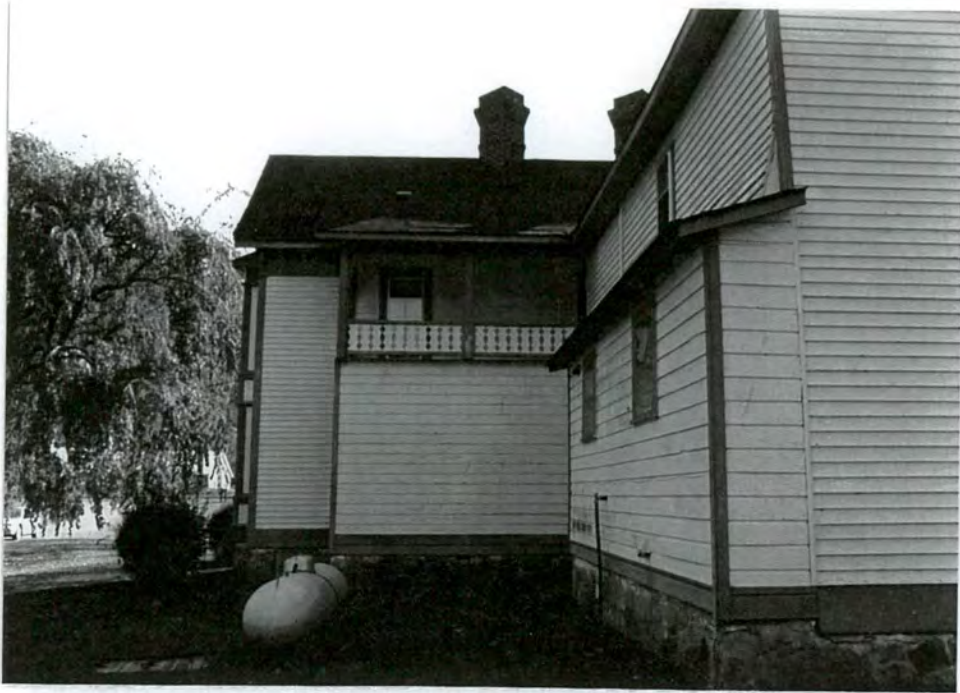
16. L-shaped rear porch with enclosures
