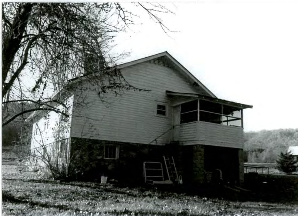
10. Southeast rear facade
