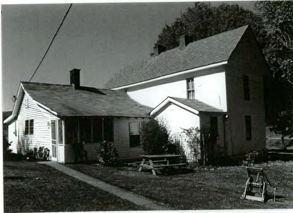
10. South rear and east side facades showing additions
