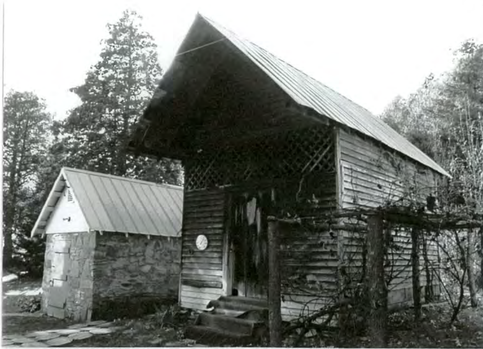
20. Front facade of frame smokehouse
