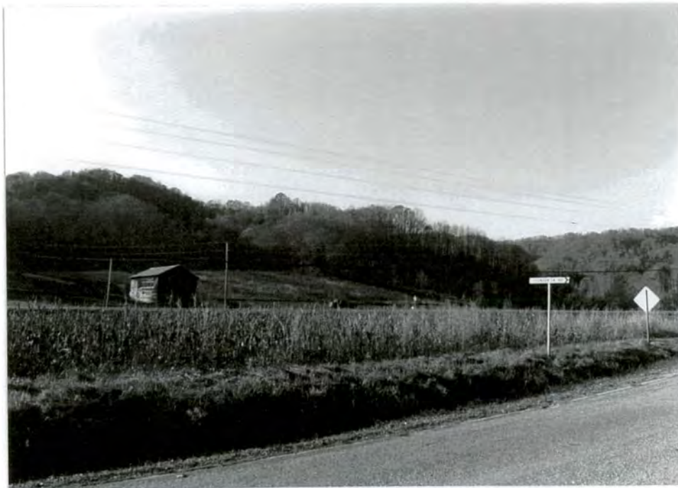
2. View from old highway 19 at Ponder Creek Road toward US 19
