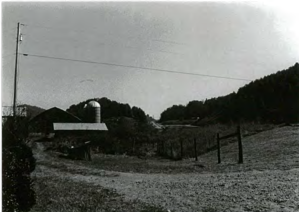
25. View of farm complex from front of house with US 19E (right)
