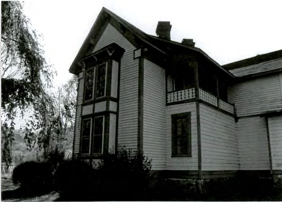
14. East side facade and rear porch
