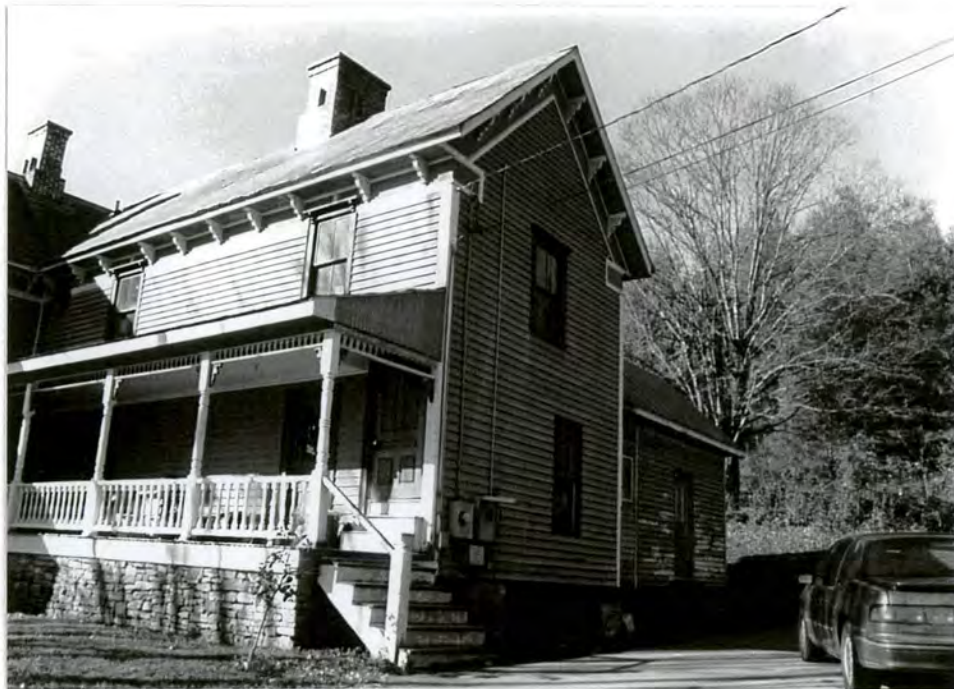
13. North end facade of rear wing
