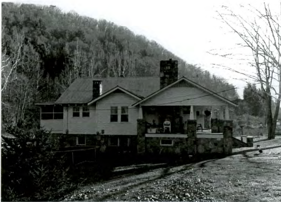
9. Northeast side facade
