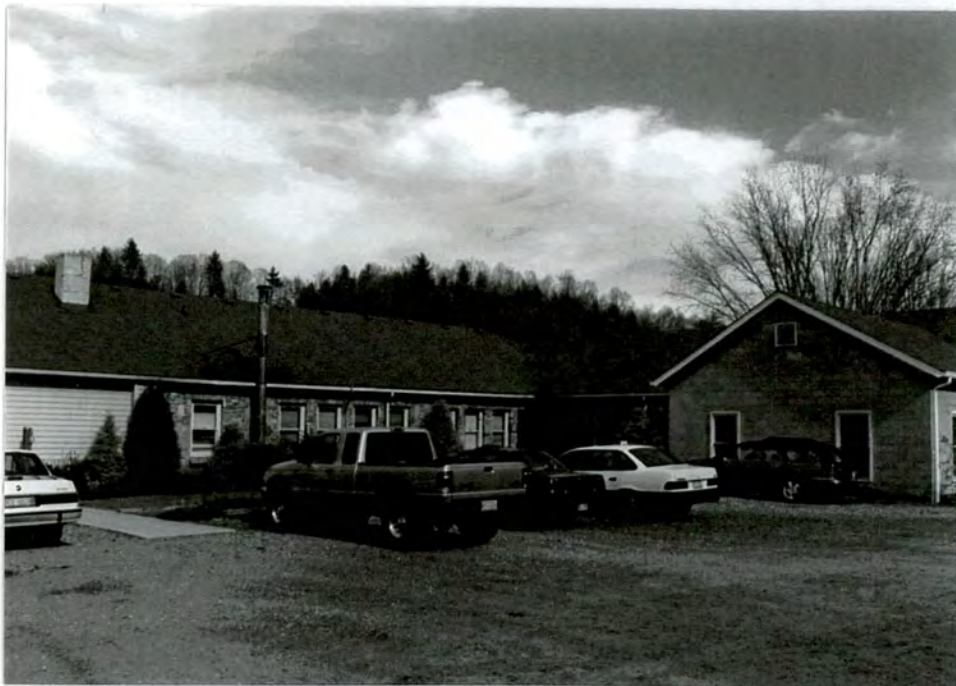
10. South rear facade and east wing
