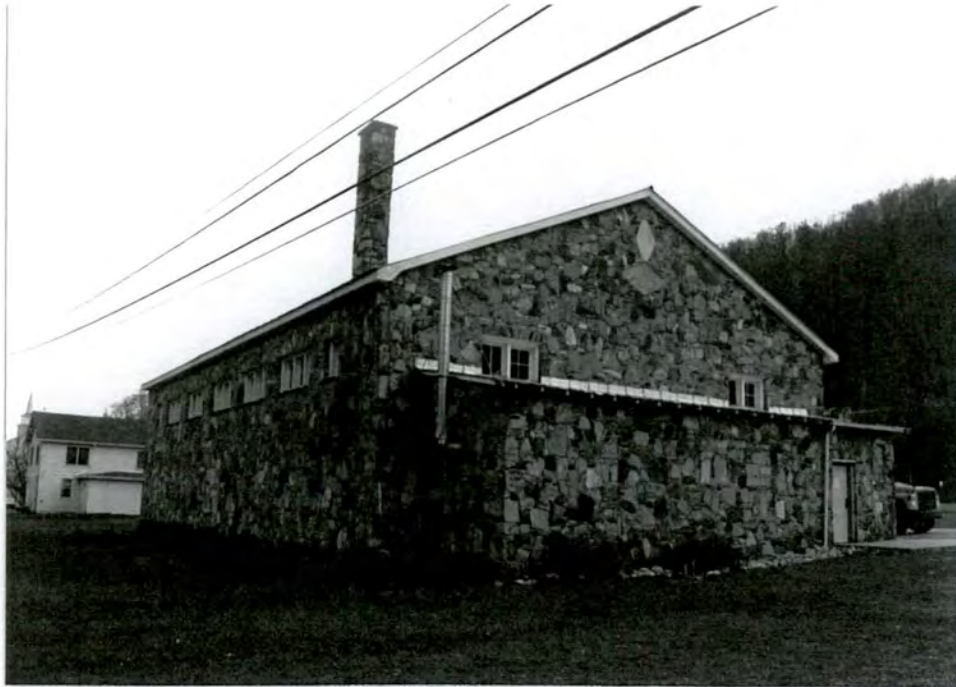
17. West front and north side facades of gymnasium
