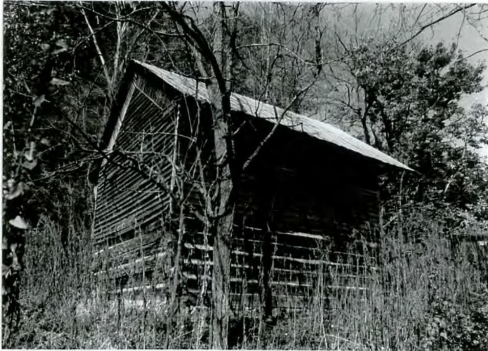
20. Rear and side facades of log/frame apple/potato storage house
