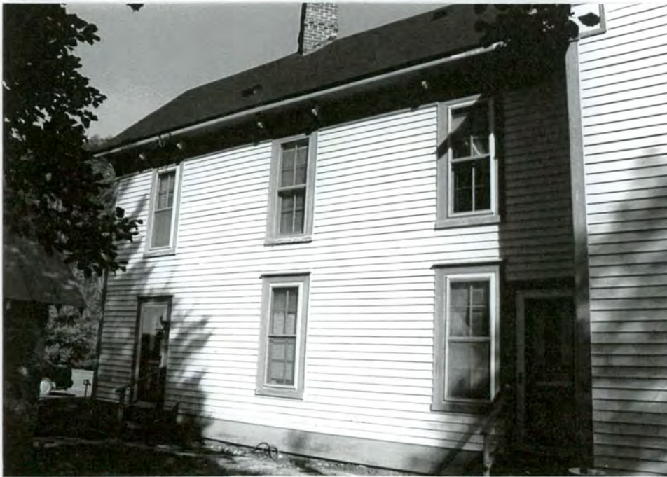
13. West side facade of rear wing
