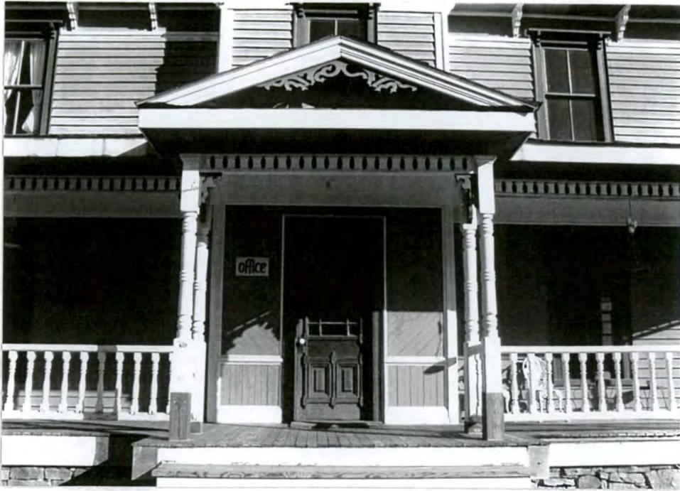
7. Detail of first-floor front porch and projecting entrance bay
