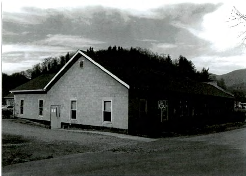
9. Classroom addition on rear of east wing
