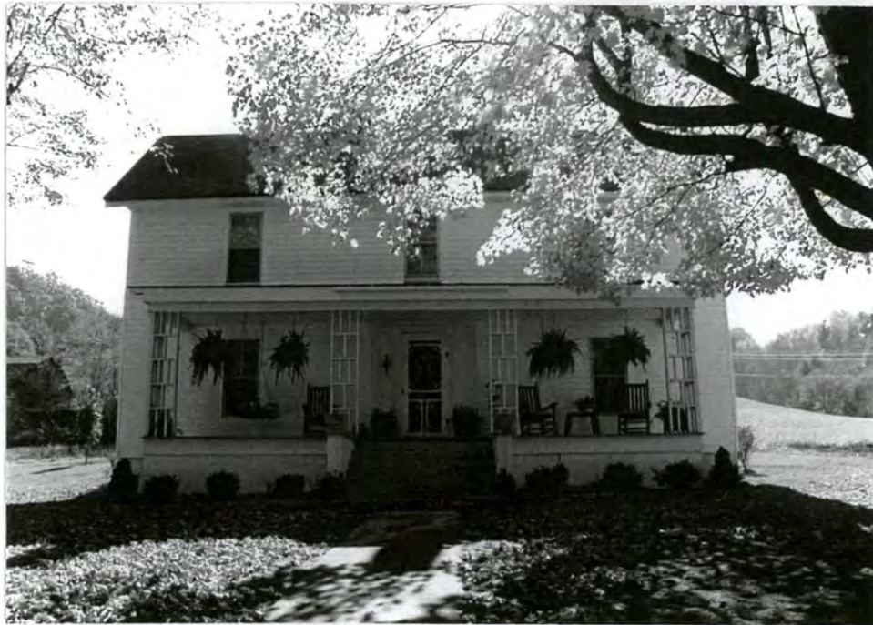
2. North front facade
