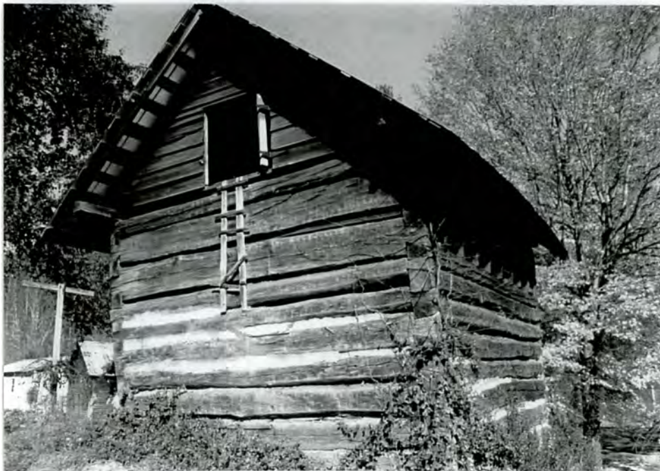
23. Rear facade of log apple/fruit storage house
