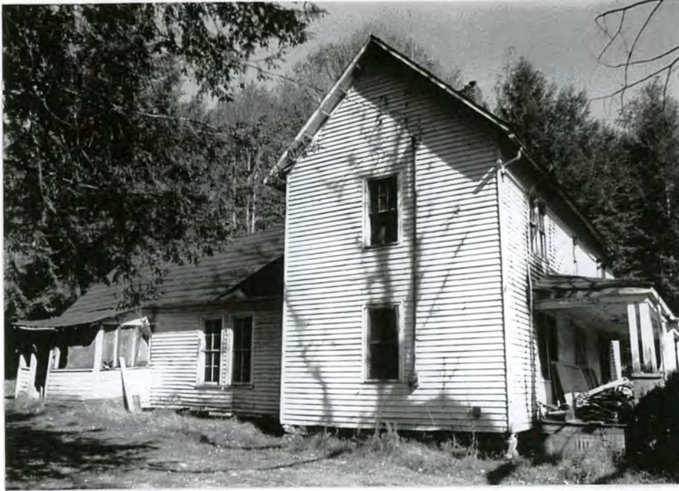
3. West side facade and rear wing
