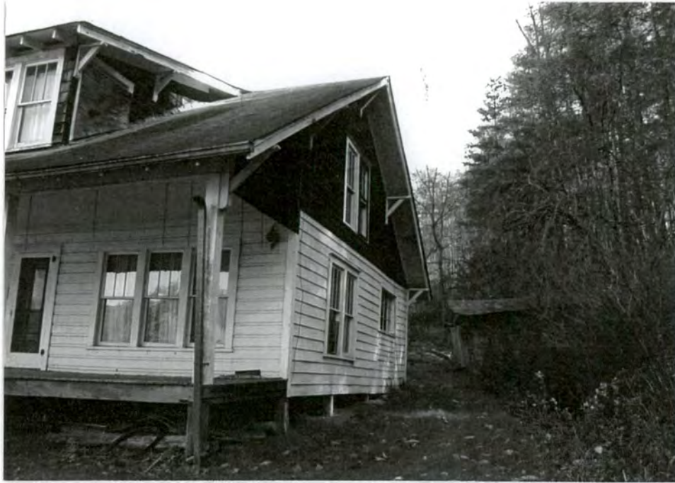
7. Southwest side facade adjacent to creek
