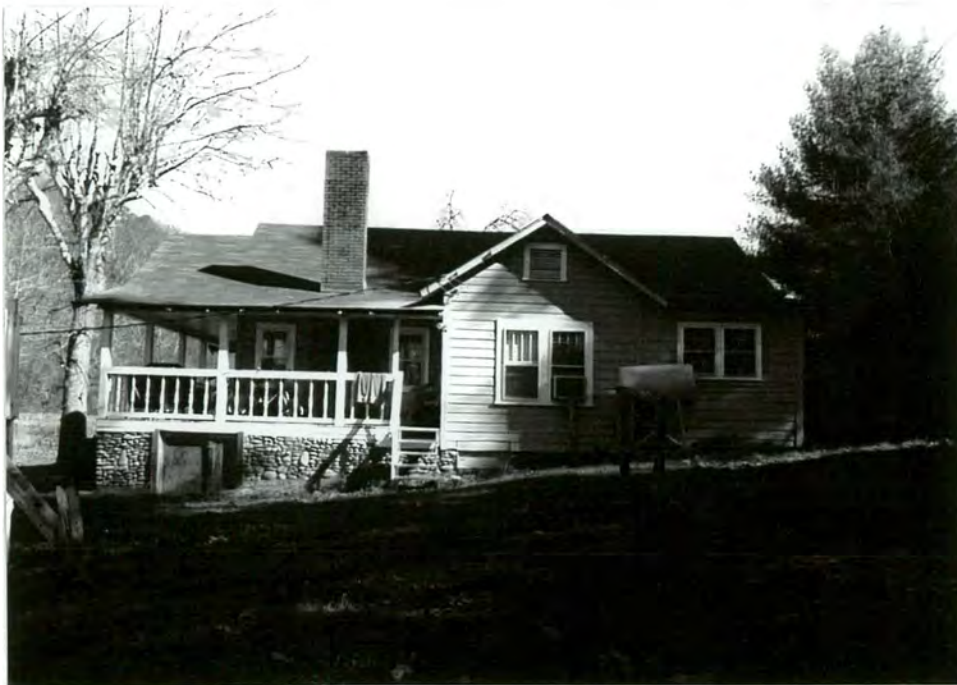
6. Southwest side facade
