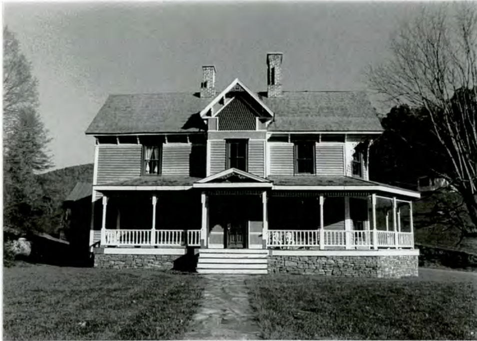
5. South front facade
