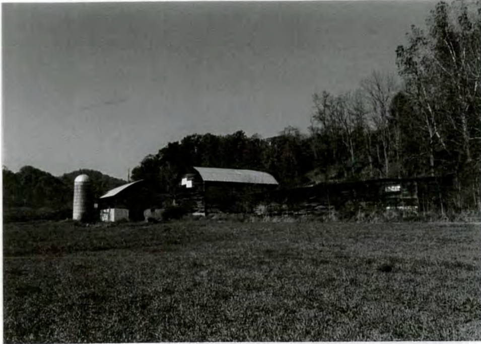
34. View across cultivated field looking west toward farm complex
