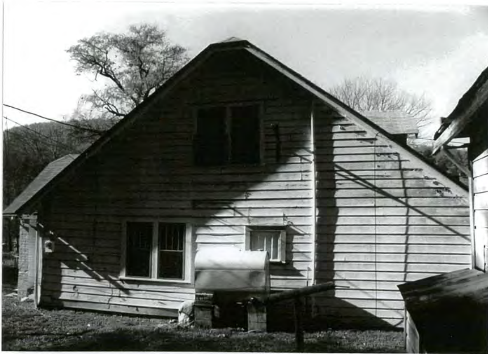
10. Southeast rear facade
