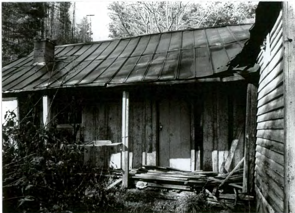
12. Detail of east facade of rear wing
