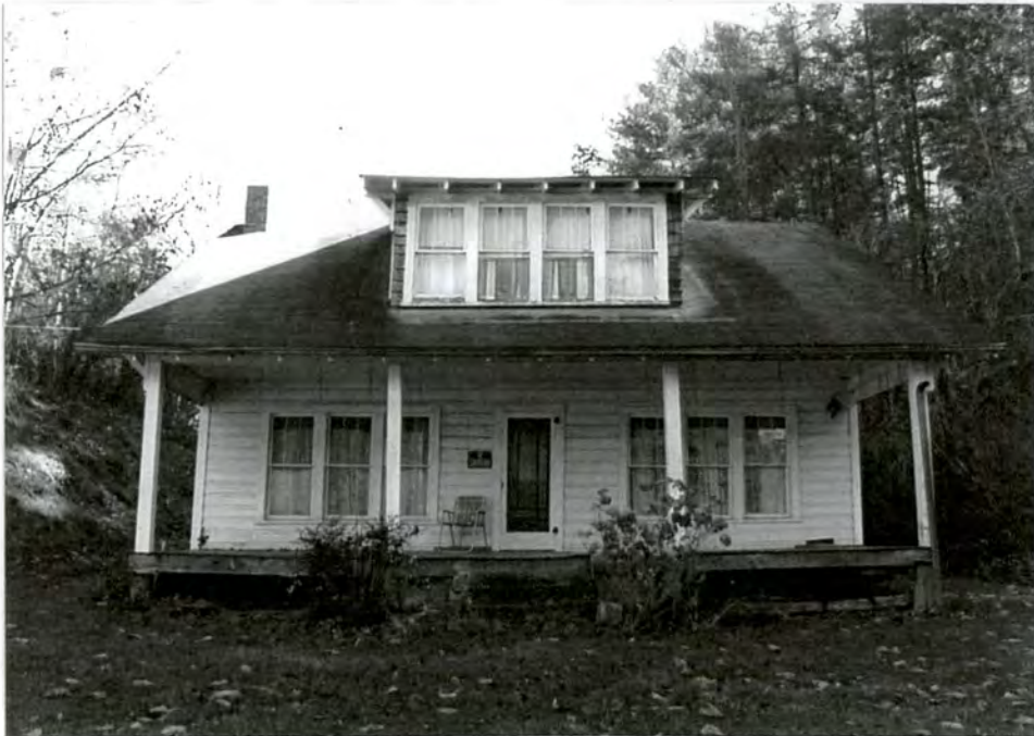
4. Northwest front facade
