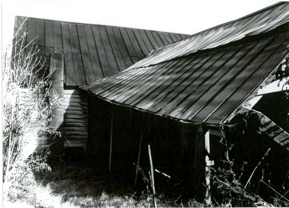
7. West side facade of rear wing
