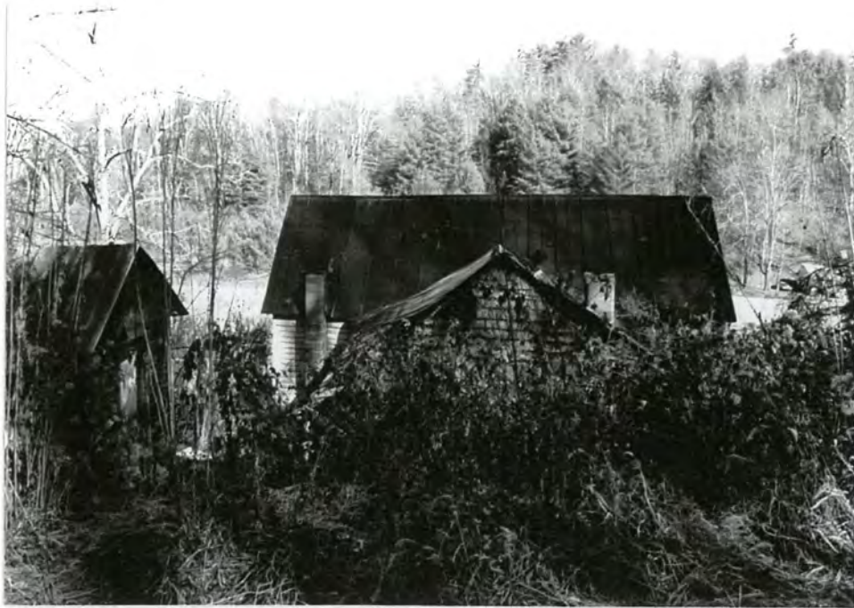
9. South rear facade showing rear of main section and rear wing
