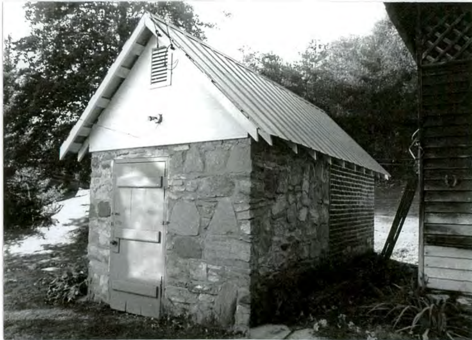
21. Front facade of stone/brick springhouse
