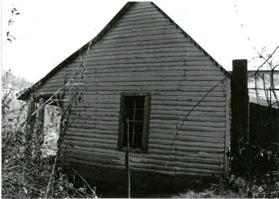
6. West side facade of main section
