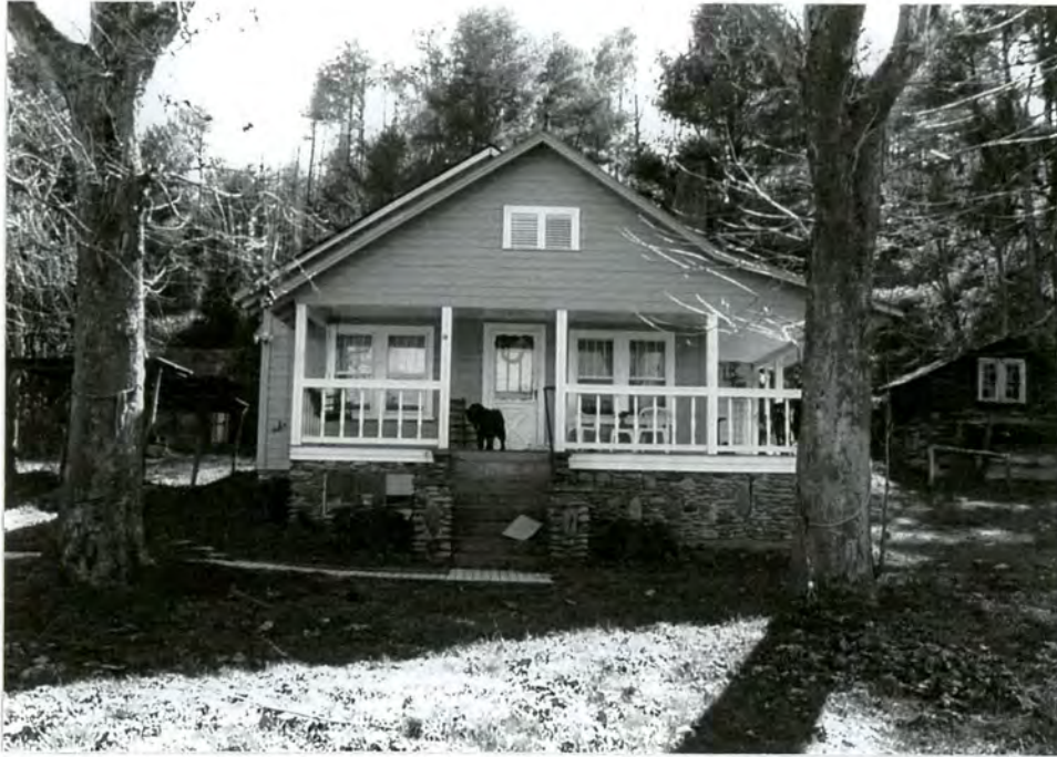
3. Northwest front facade
