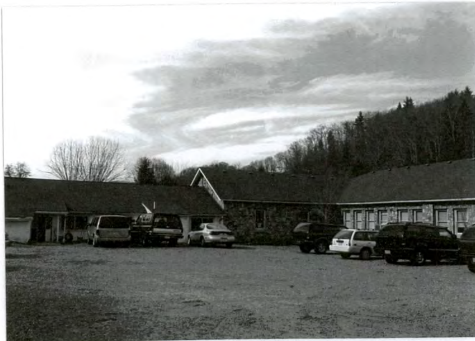
12. South rear facade and west wing with 1950s cafeteria addition
