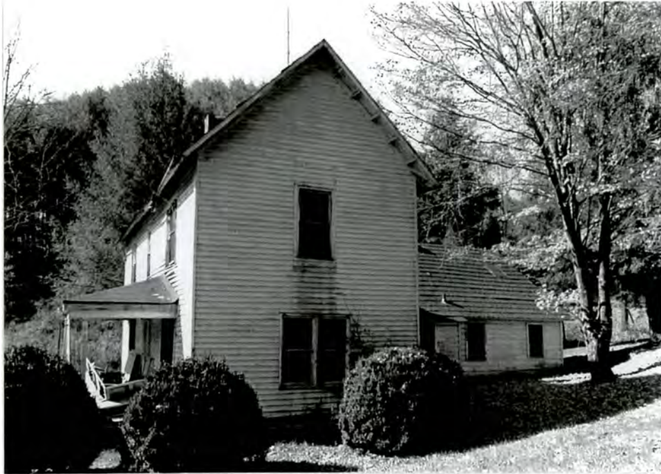
8. East side facade
