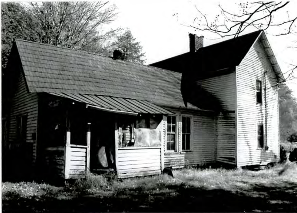
9. West side facade of rear wing
