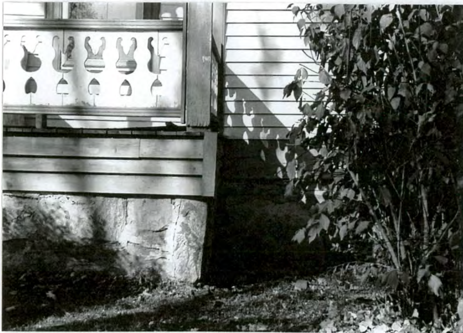
8. Detail of solid stone foundation
