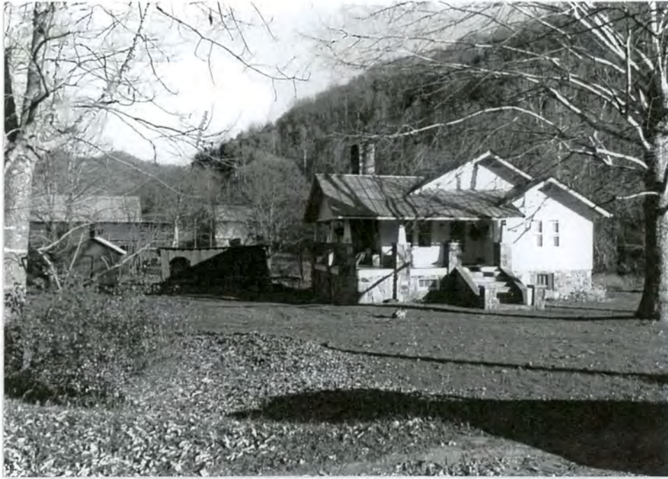
3. Buckner House in its setting
