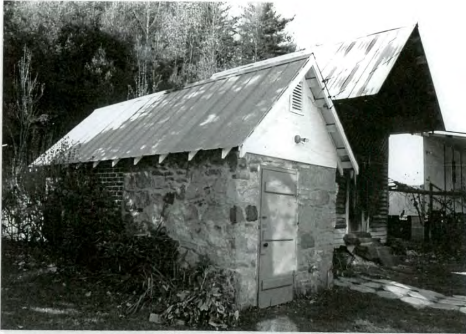
18. Front facade of stone/brick springhouse
