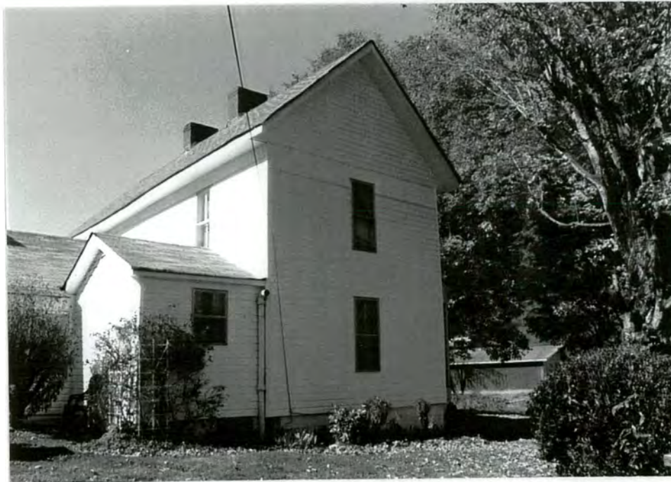
11. East side facade
