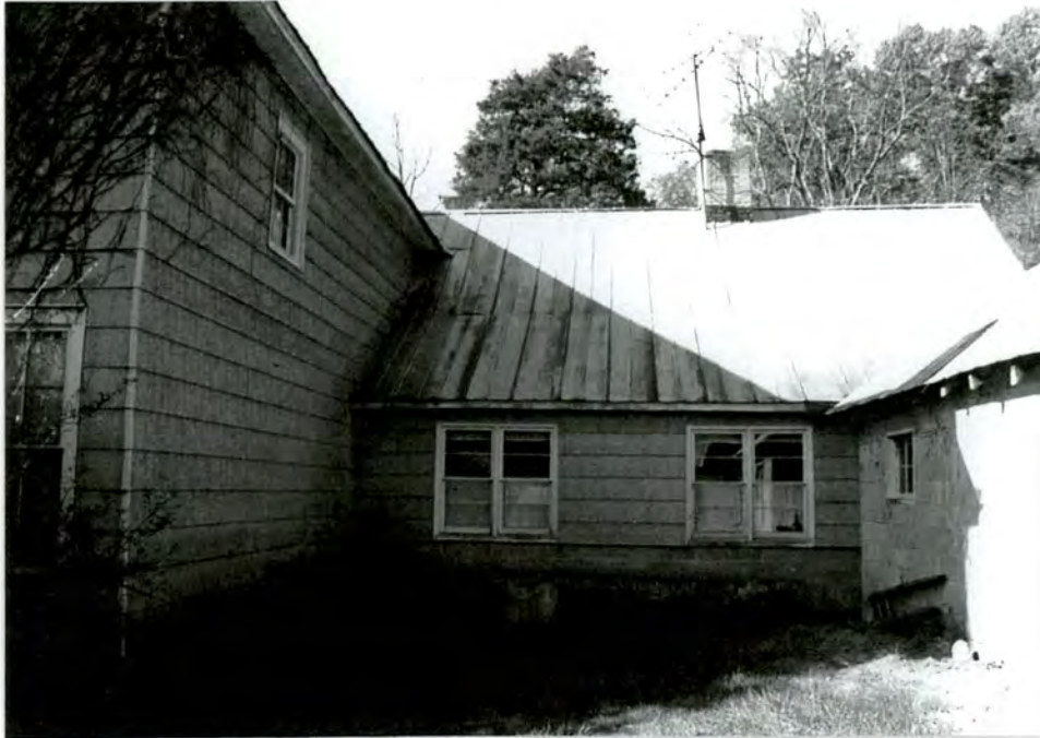
14. East side facade of rear wing
