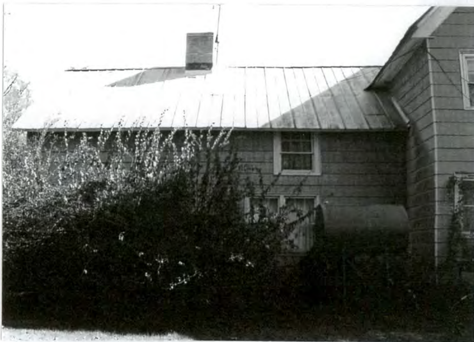
9. West side facade of rear wing
