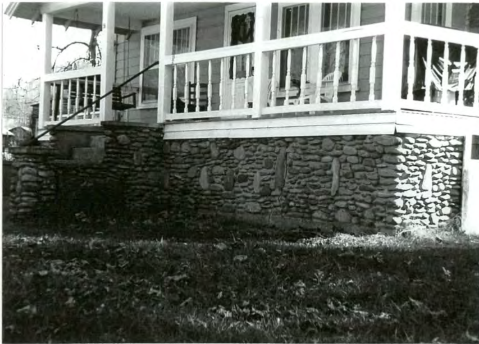
5. Detail of stone foundation
