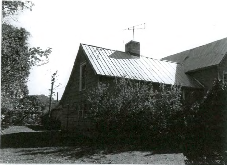
12. West side and north end facade of rear wing
