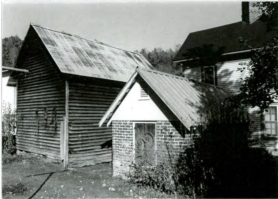
19. Rear facades of stone/brick springhouse and frame smokehouse
