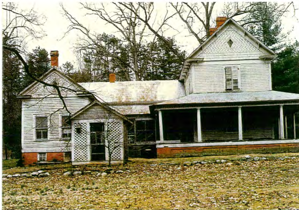
Figure 32: Henry Webster Farm (CH 598), south elevation with well house in foreground
