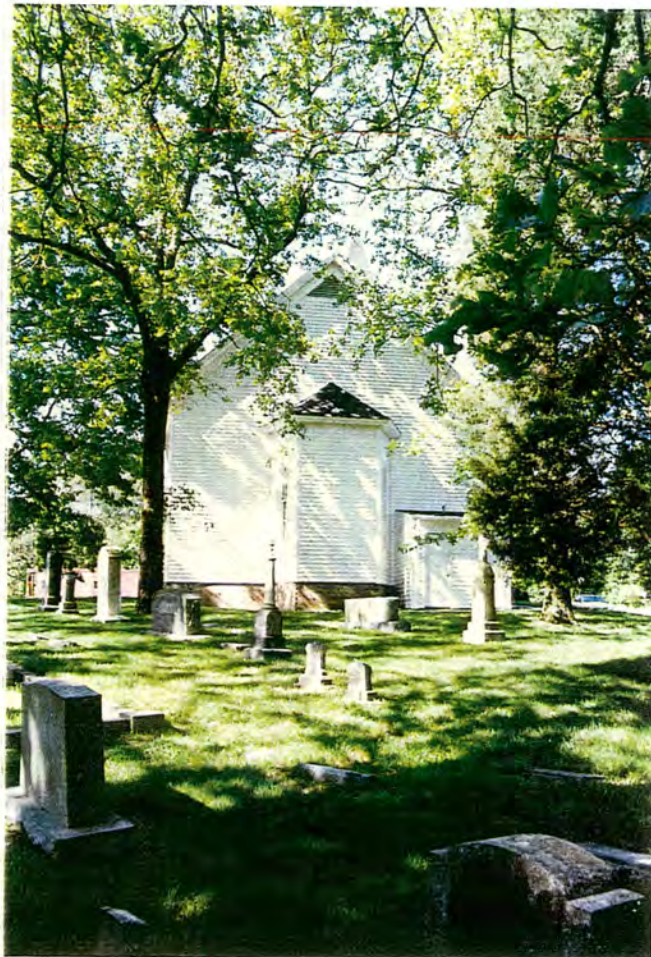
Figure 23: Gulf Historic District (CH 785), Property 8, Gulf Presbyterian Church (CH 764), south elevation
