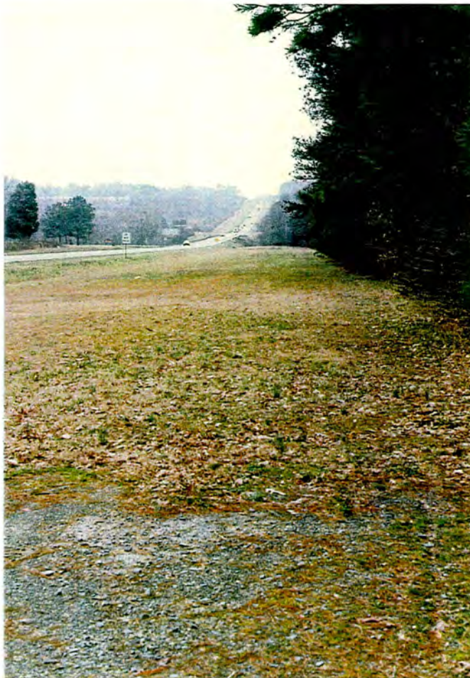
Figure 41: Henry Webster Farm (CH 598), view south, maintained right-of-way
