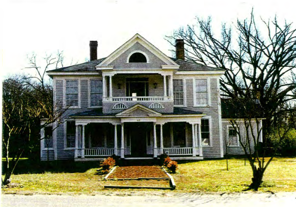
Figure 12: Gulf Historic District (CH 785), Property 3, J. M. Haughton-McIver House, facade
