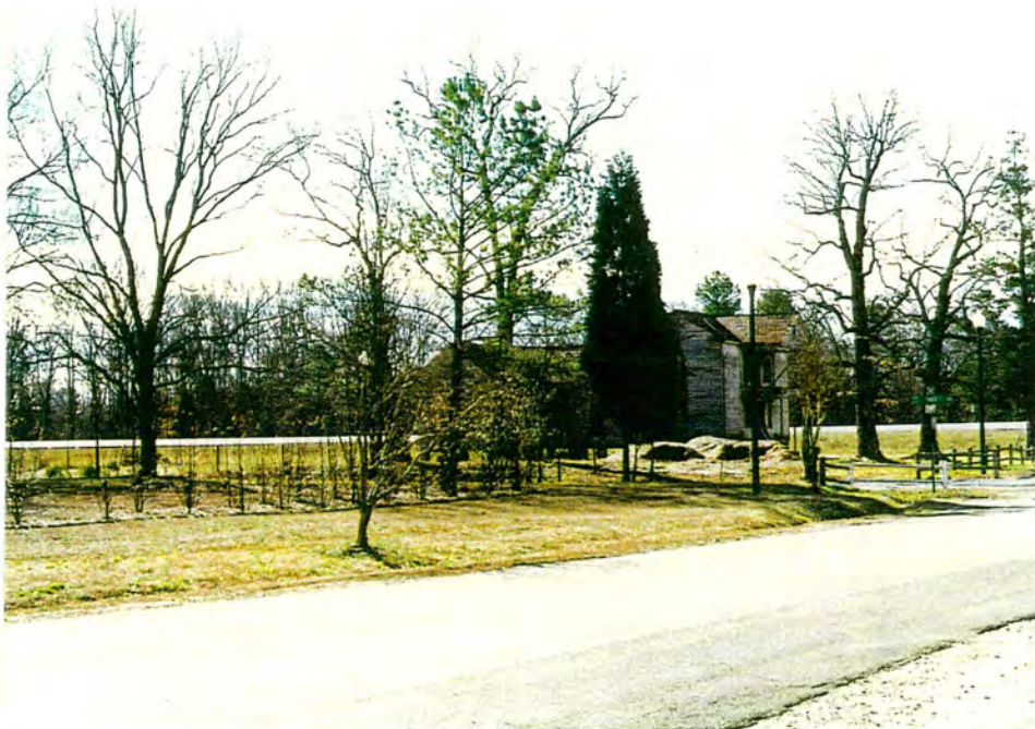
Figure 11: Gulf Historic District (CH 785), Property 2, south elevation, oblique angle
