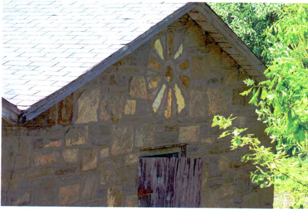
Photograph 11: Decorative detail in gable end of stone addition.
