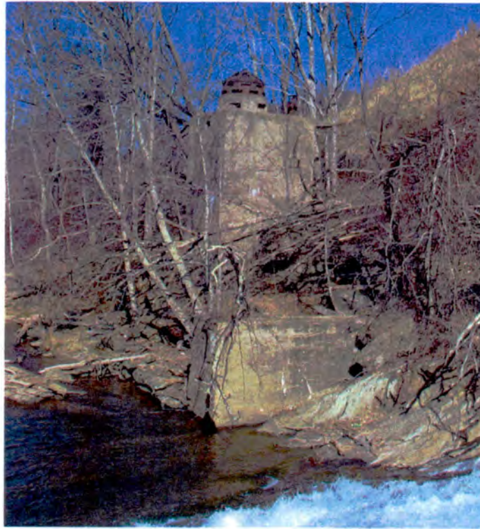
Photograph 44: View of generator from vicinity of gazebo.
