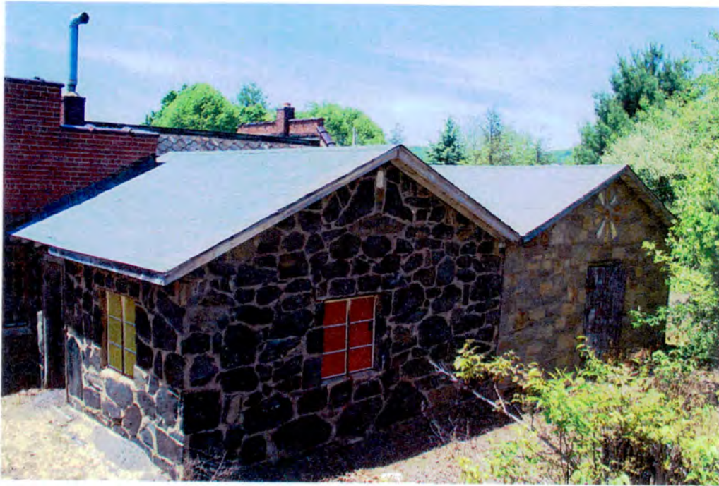
Photograph 9: Stone additions on the east side of the Main Prison Block.
