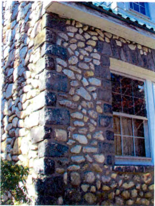
Photograph 32: Detail of stonework.
