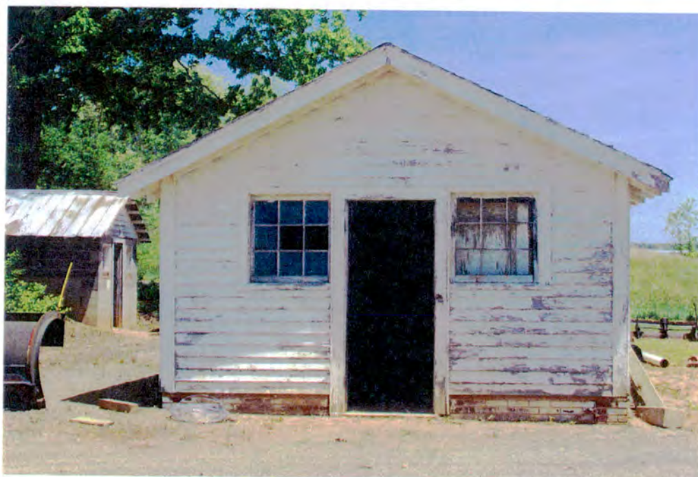
Photograph 20: Laundry and Wash House – west elevation.
