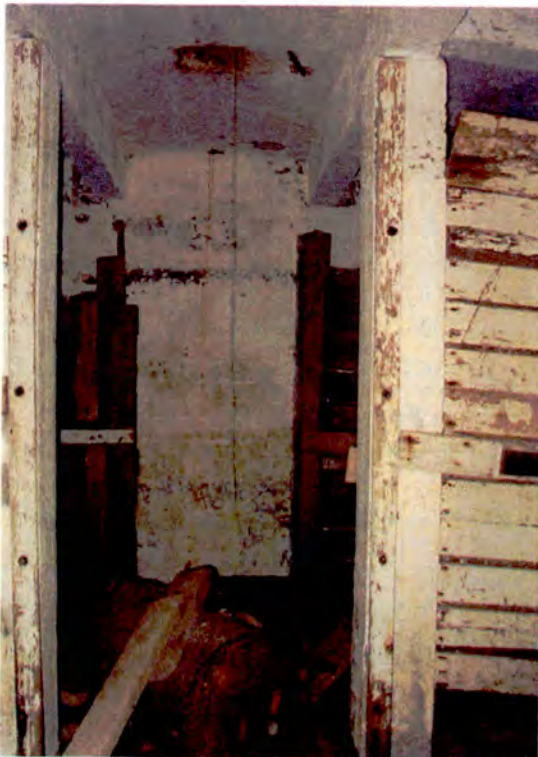
Photograph 28: Interior of Root Cellar.
