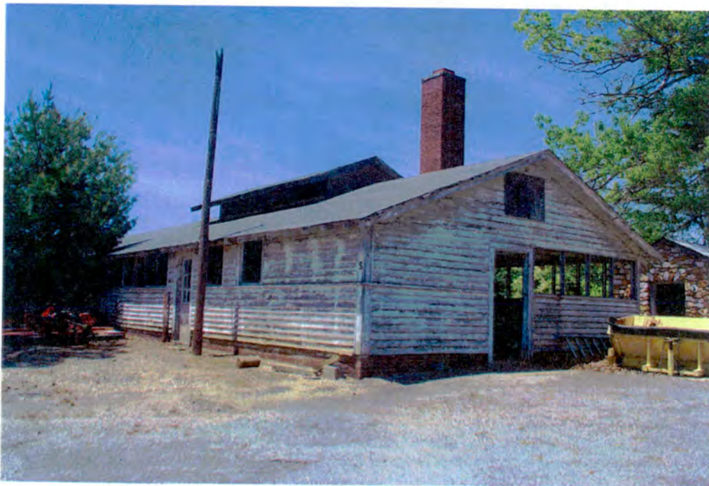
Photograph 14: View of monitor over kitchen area on east end of the Kitchen and Mess Hall.
