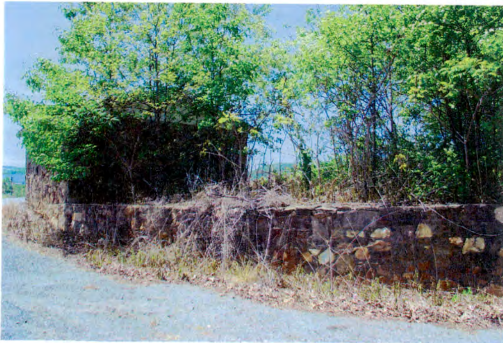
Photograph 26: Stone retaining wall between Shed #11 and Root Cellar.
