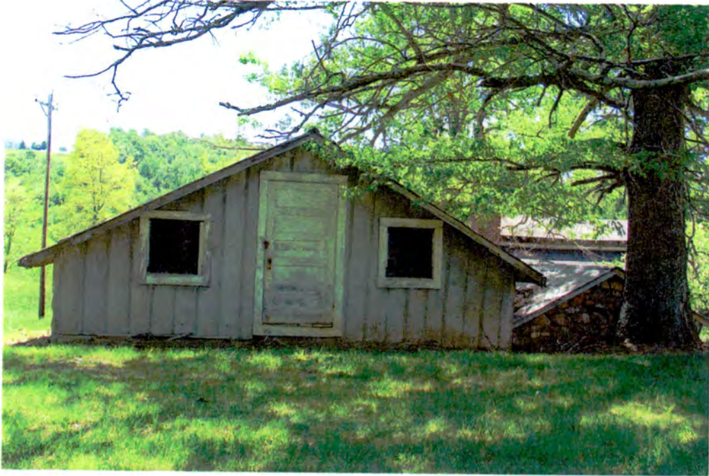
Photograph 17: Upper story on north elevation of Shed #4. Smokehouse roof on right.
