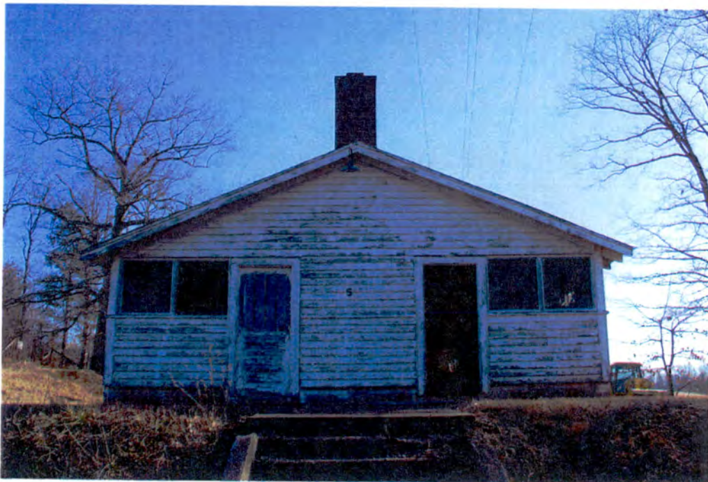
Photograph 12: Kitchen and Mess Hall – west elevation.
