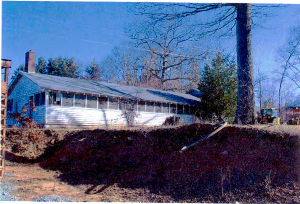
Photograph 13: Kitchen and Mess Hall – south elevation.
