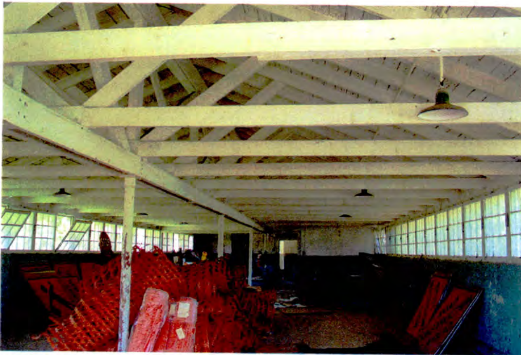
Photograph 15: Interior view of the mess hall.
