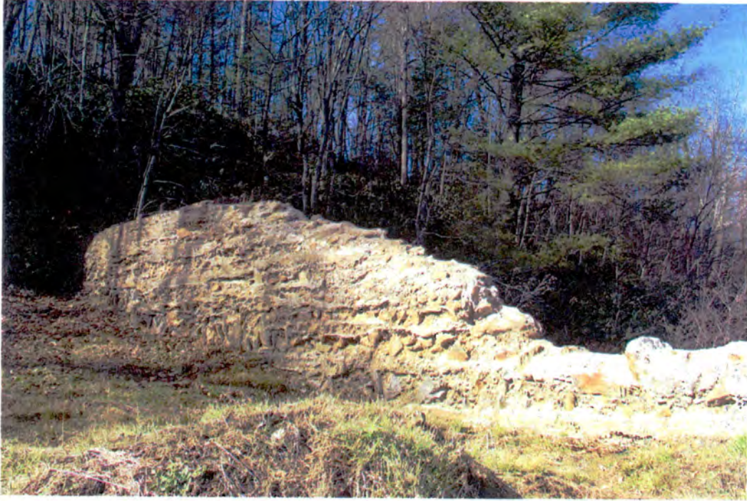
Photograph 42: Remaining portion of dam wall.
