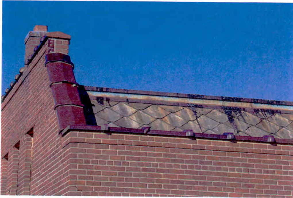
Photograph 7: Coping along roof parapet of Main Prison Block.
