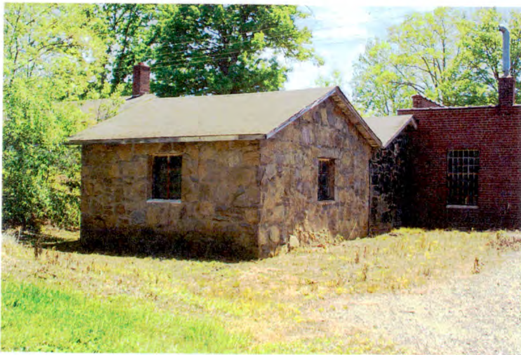
Photograph 10: North and west elevations of stone additions.
