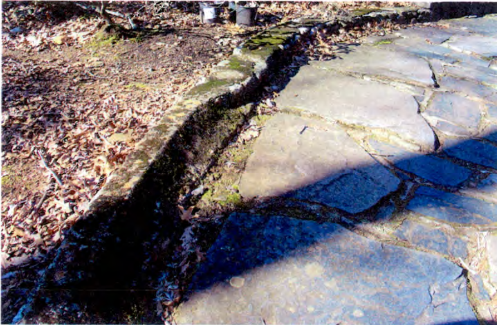
Photograph 37: Detail of granite curbing and flagstone driveway.
