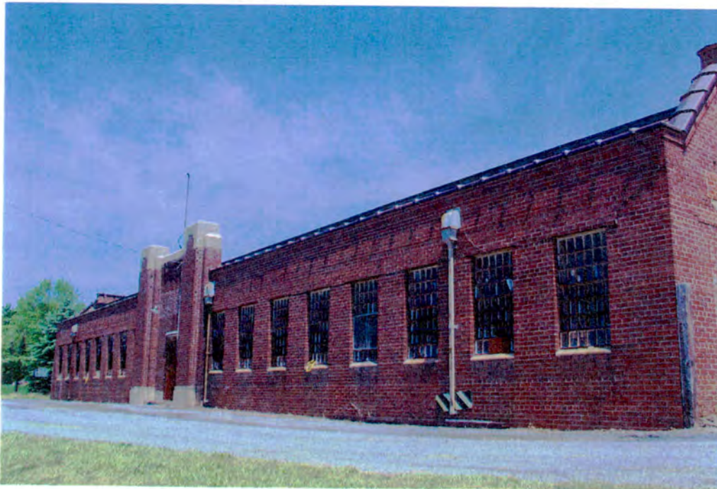
Photograph 4: West facade of the Main Prison Block.
