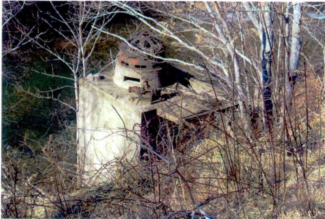
Photograph 45: View of the generator from the hill above the Little River.
