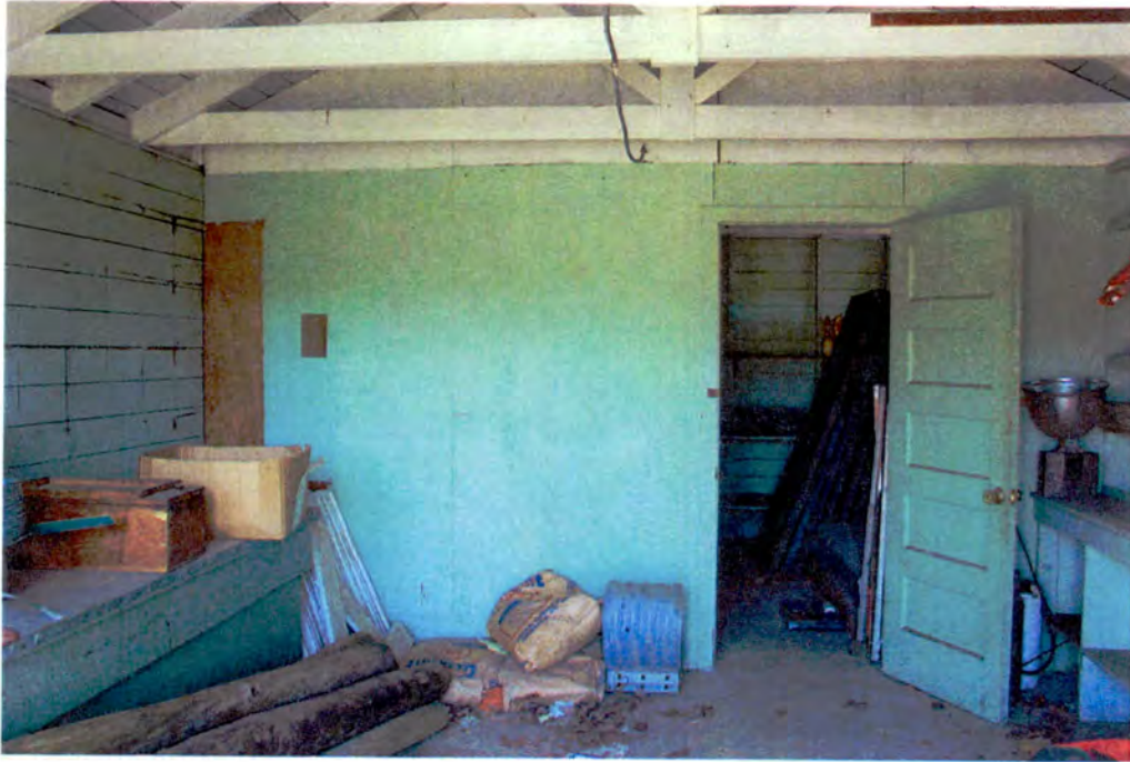
Photograph 21: Interior view of Laundry and Wash House.
