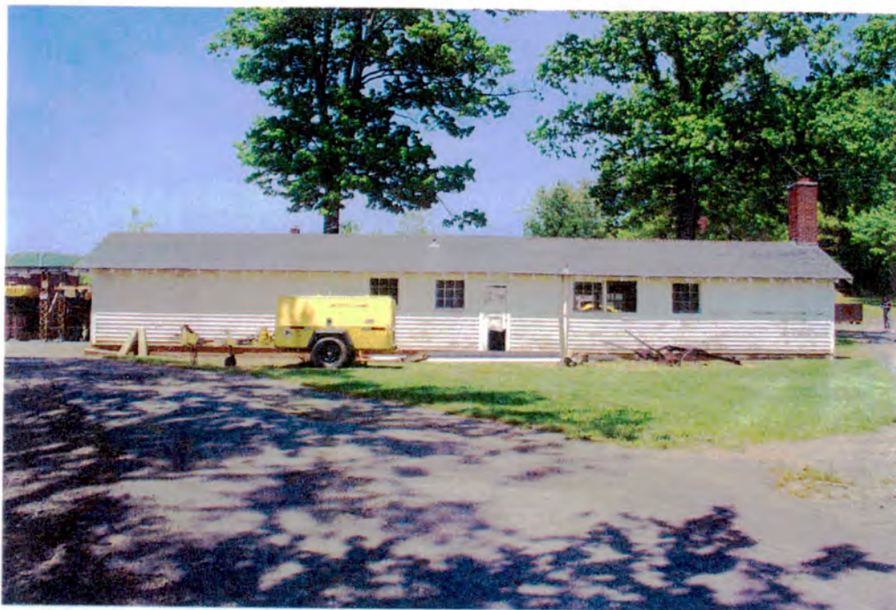
Photograph 19: Laundry and Wash House – south elevation.
