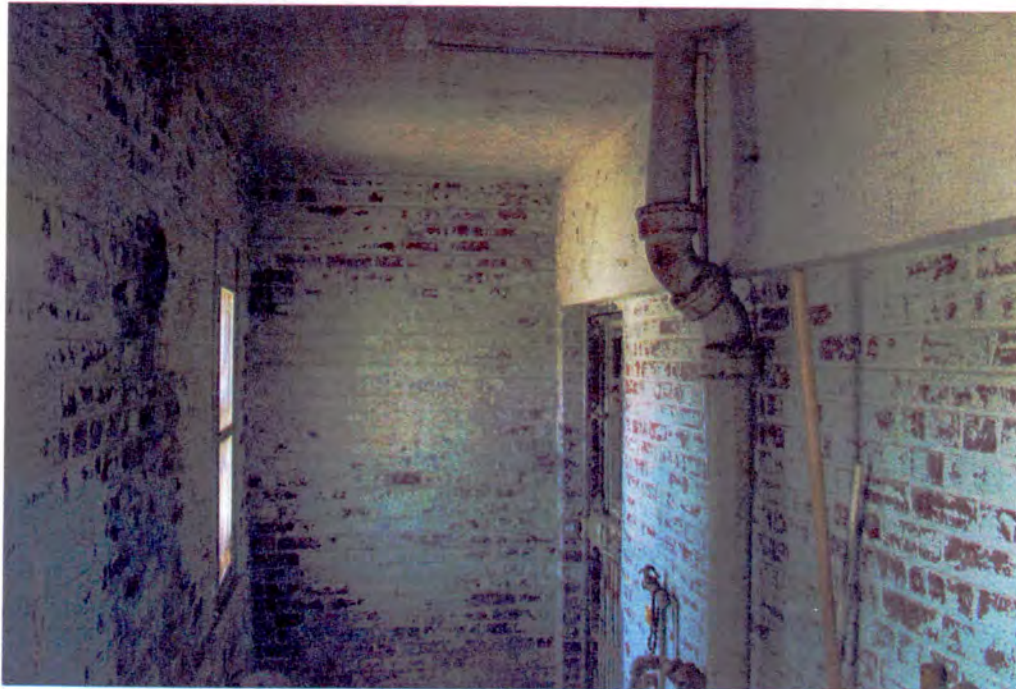
Photograph 24: Interior view of Solitary Confinement.
