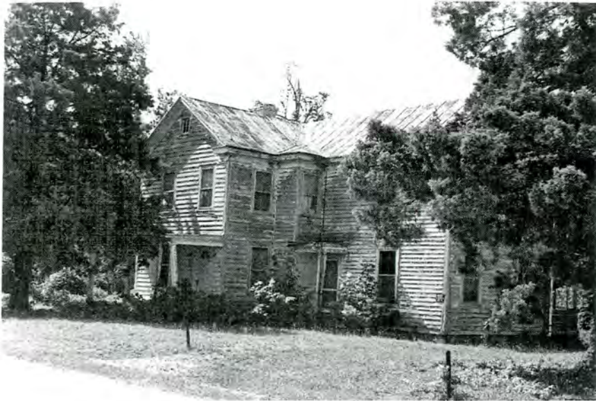
Plate 16. Pollocksville Historic District (No. 11), Stationmaster's House, Looking Southeast.
