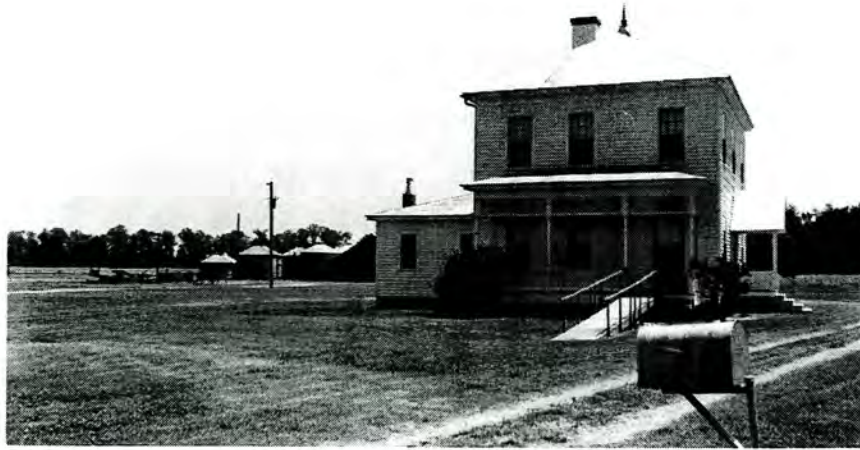
Plate 19. J. Nathan Foscue Farm (No. 12), House, Outbuildings, and Fields, Looking Northeast.
