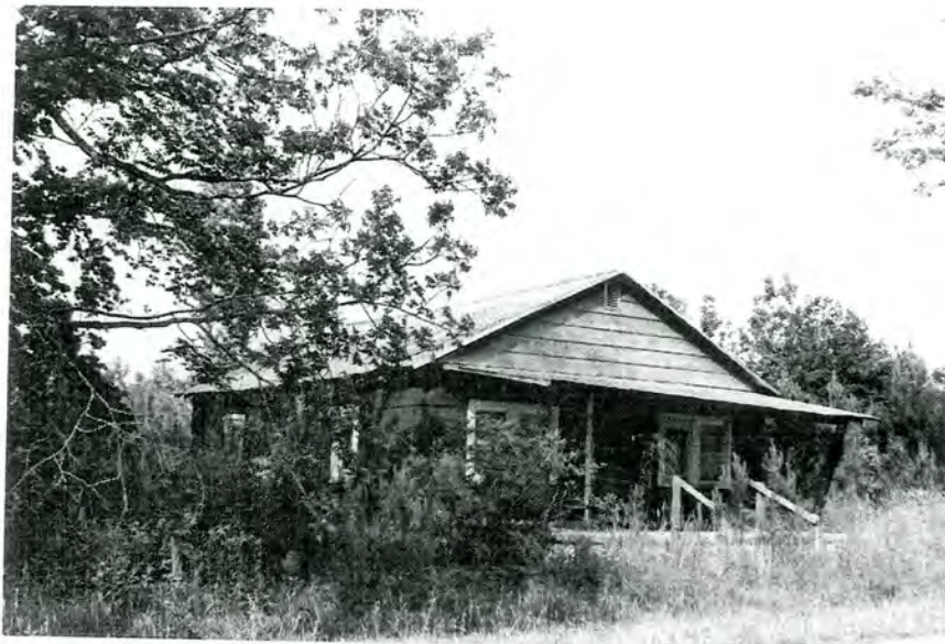
Plate 2. House (No. 2), Looking Northeast.
