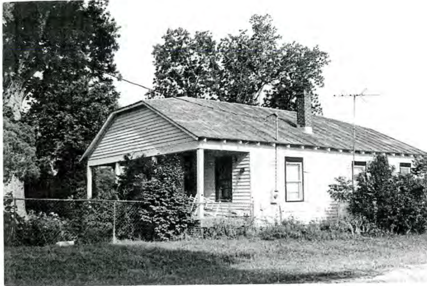
Plate 5. House (No. 4), Looking Southeast.
