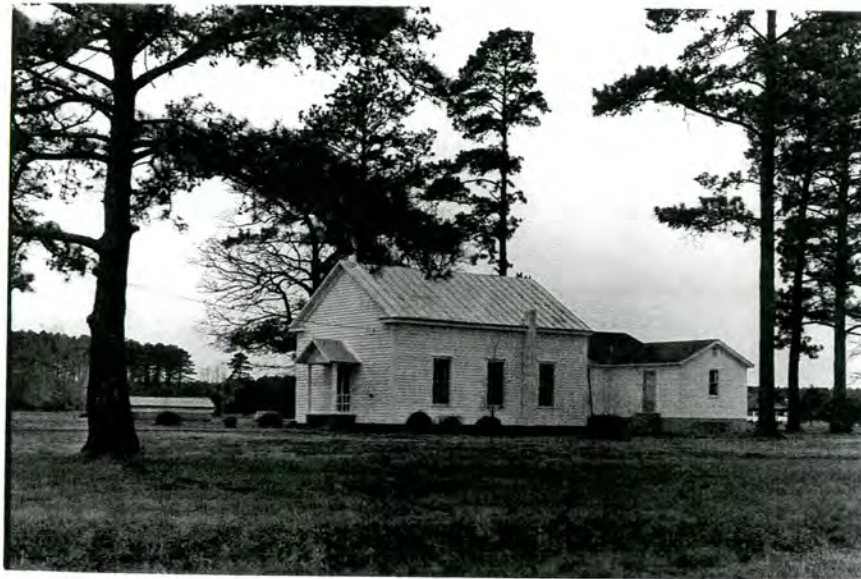
Plate 92. Lee's Chapel United Methodist Church, East and North Elevations, Looking Southwest.
