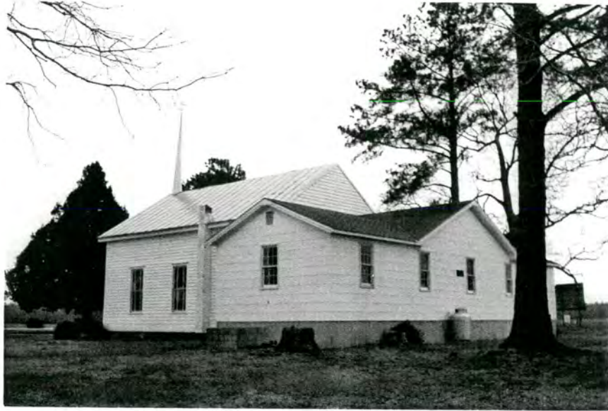
Plate 93. Lee's Chapel United Methodist Church, Rear Addition, Looking Southeast.
