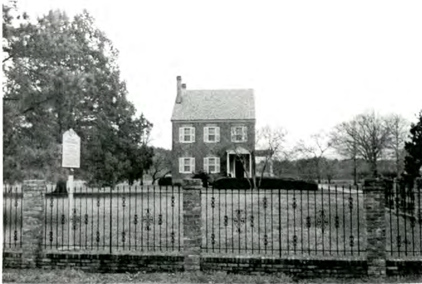
Plate 1. Foscue Plantation House, Facade.
