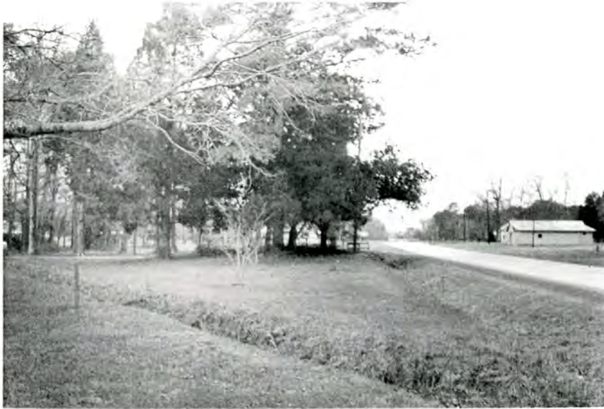
Plate 5. Foscue Plantation House, U.S. 17 Right-of-Way, Looking South.
