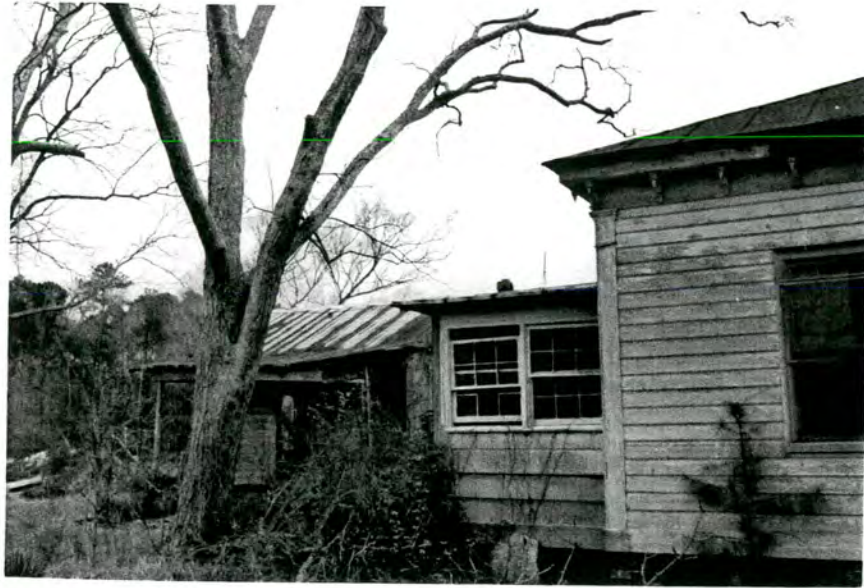
Plate 39. Amos L. Simmons, Jr. House, Rear Ell, South Elevation.
