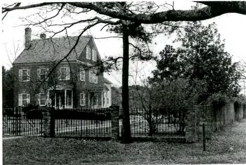
Plate 2. Foscue Plantation House, Facade and South Elevation.
