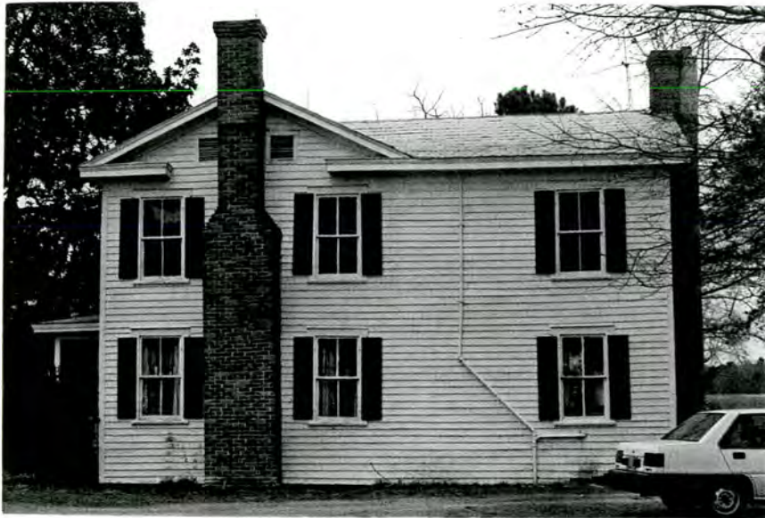
Plate 79. Nelson Deppe House, South Elevation, Looking North.
