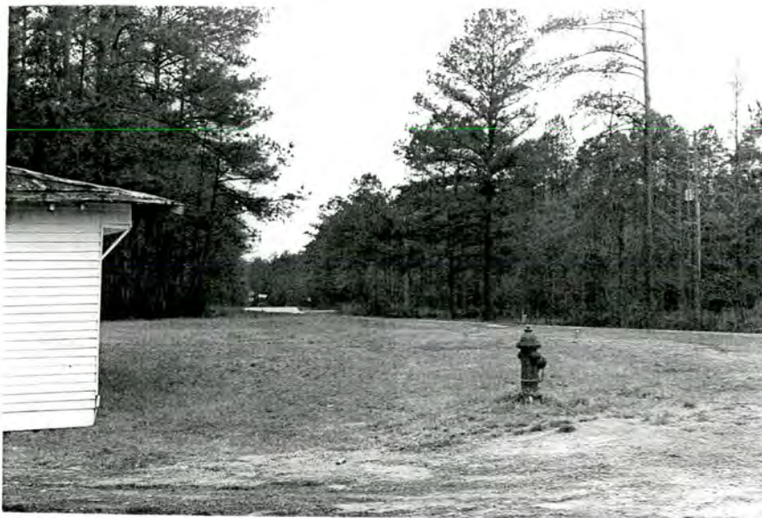
Plate 29. Gas Station/Store, S.R. 1002 Right-of-Way, Looking Southwest.
