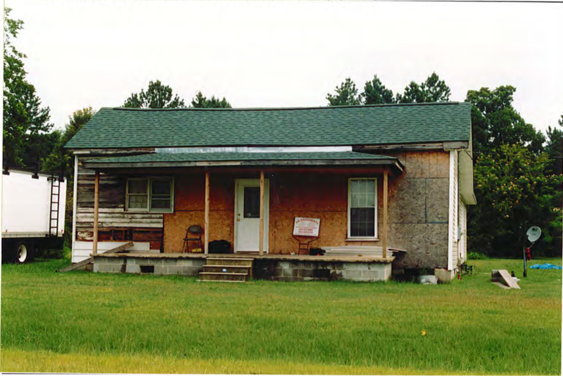
Figure 63. House on Parcel 026694
