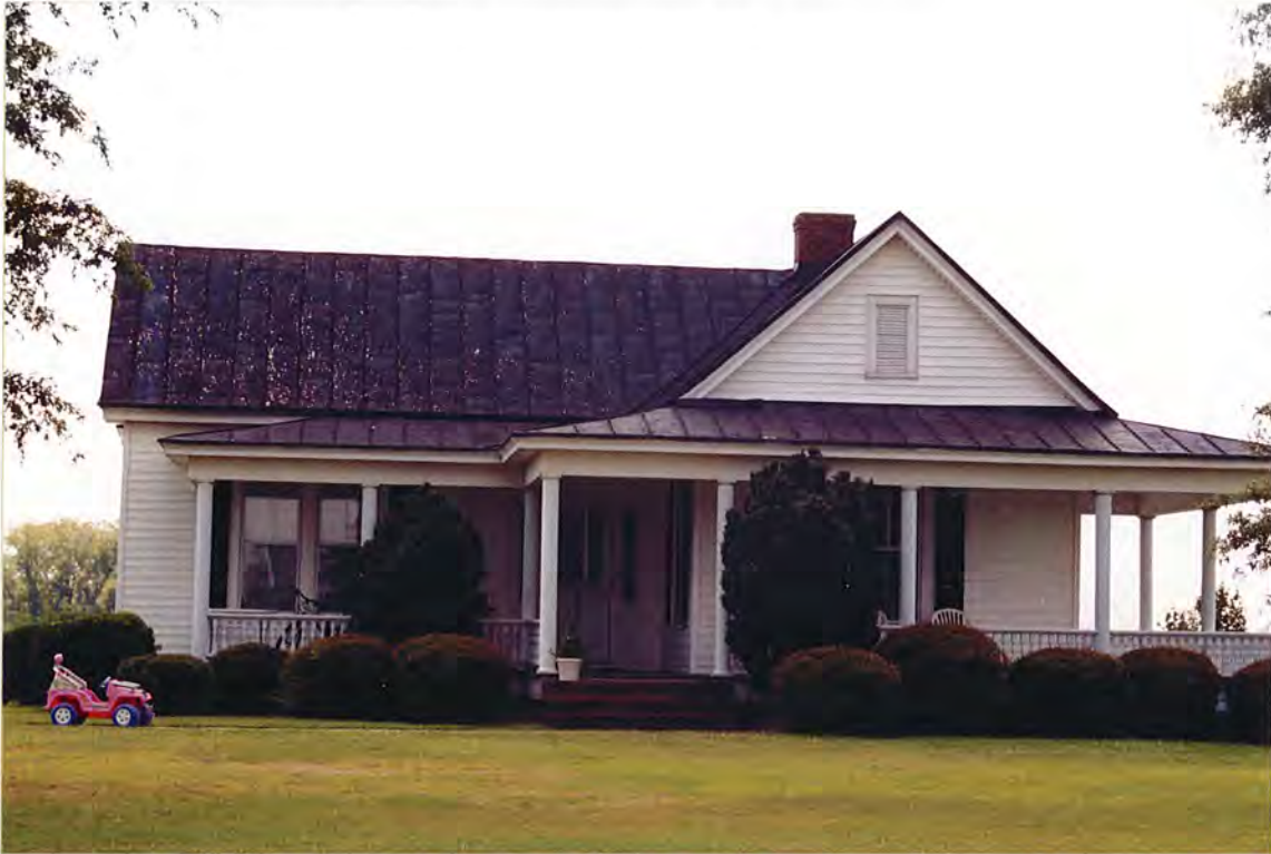
Figure 28. Queen Anne house, view from Frog Level Road (Inventory #1)
