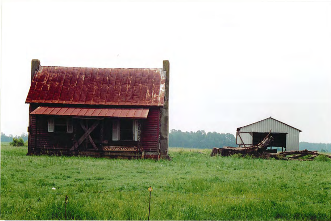
Figure 72. Spier Worthington House with garage behind (#2, #2a.)
