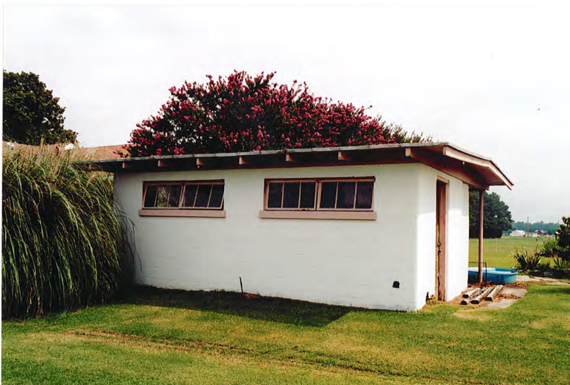
Figure 74. Concrete-block storage building (#3a)
