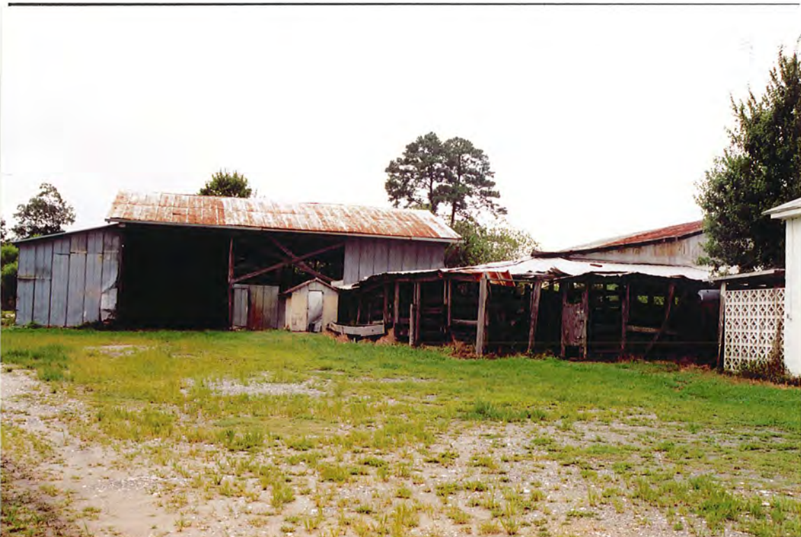
Figure 122. Garage/Corral barn (#16u)
