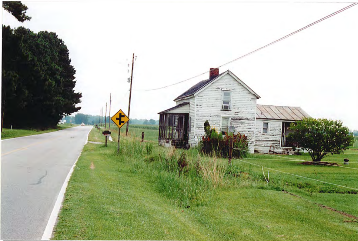
Figure 70. Tenant House, 4043 NC 903 (Inventory #1)
