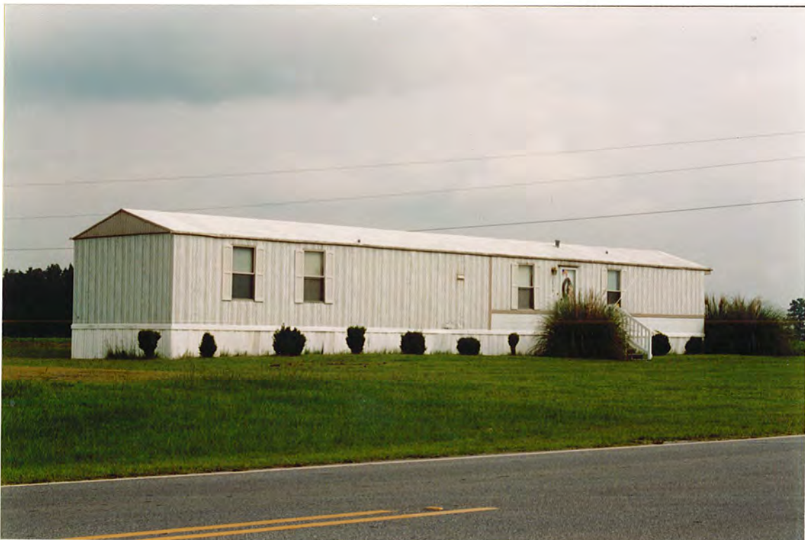
Figure 39. Mobile home, on parcel at corner of NC 903 and Abbott Farm Road
