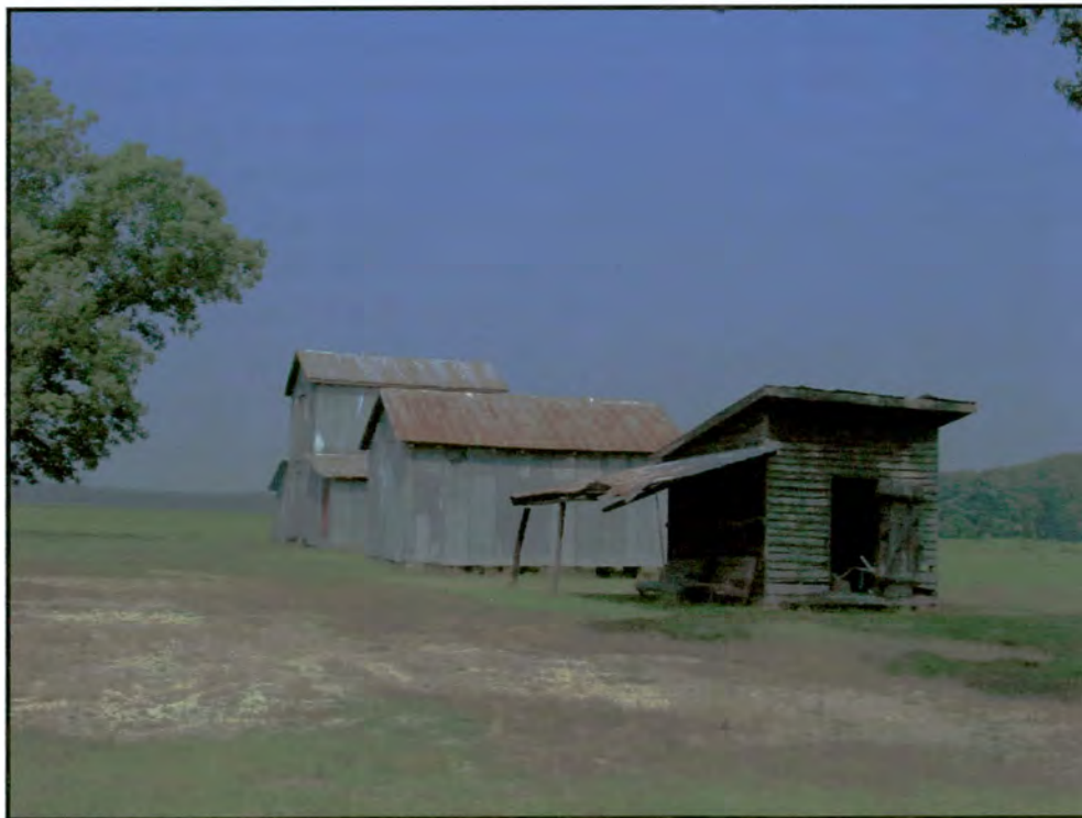
Figure 6. Outbuildings beside hip-roofed house
