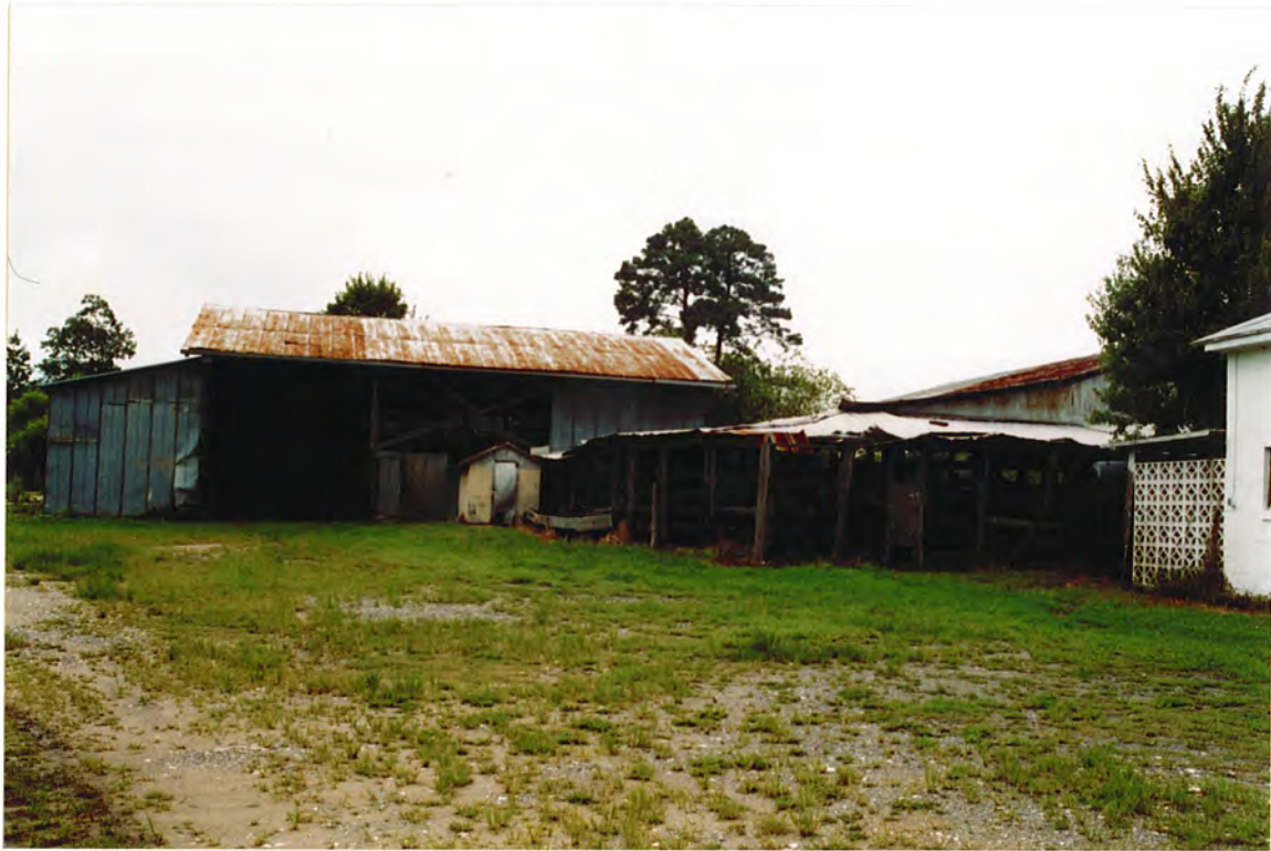
Figure 49. Garage and corral
