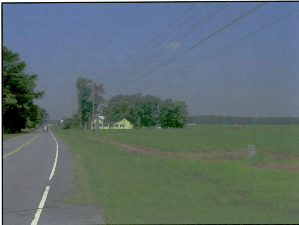
Figure 25. House and Packhouse, N side NC 102, near W end of district
