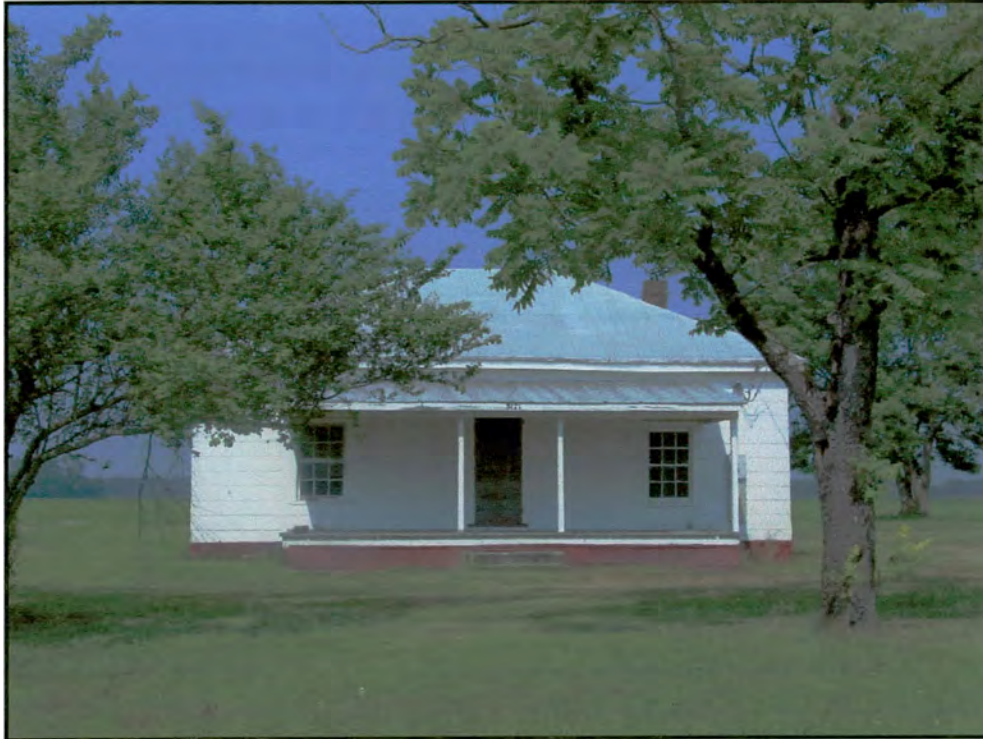
Figure 5. Hip-roofed house E of W arm of Lemon Road (loop road)
