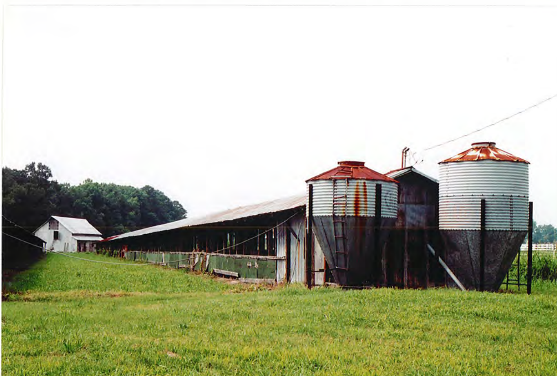
Figure 75. Poultry houses (#3c-e) and mule barn (#3h)
