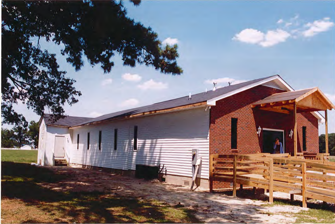
Figure 56. Zion Hill Church, showing renovations
