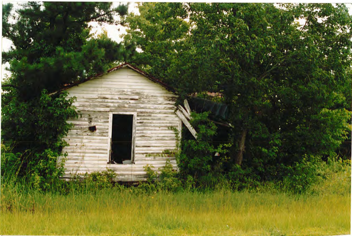
Figure 62. Building on Parcel 020398
