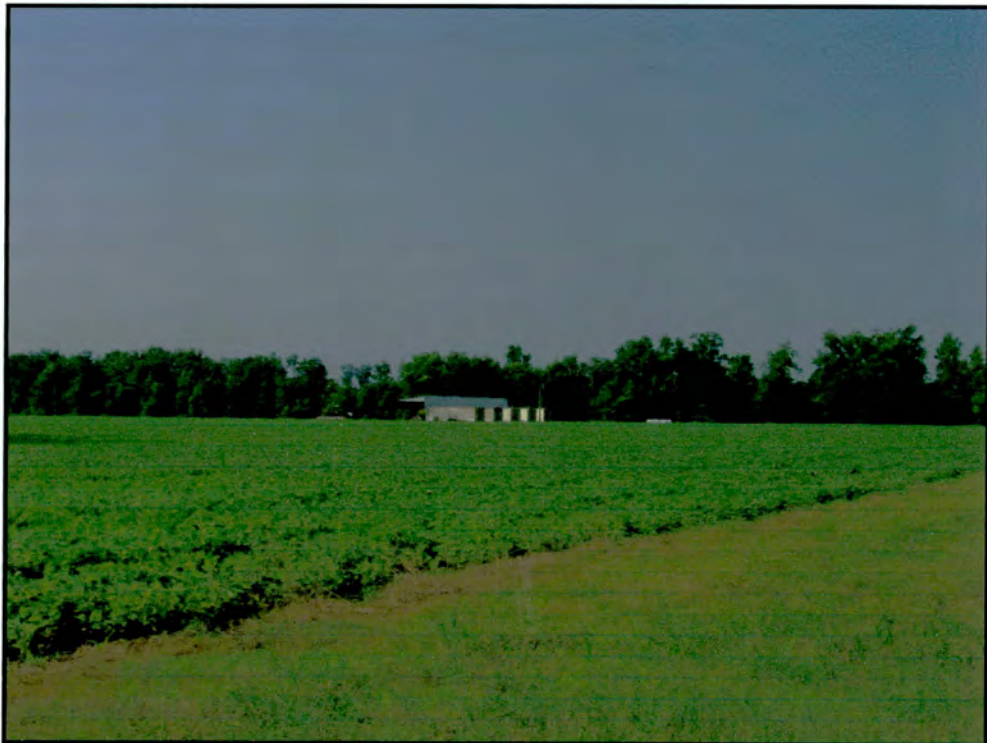
Figure 12. Bulk barns joined with shed roof, behind barn on S side of NC 121 W of loop road
