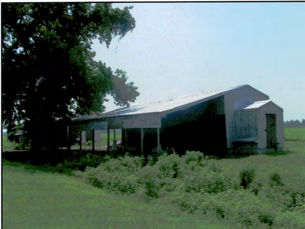
Figure 21. Equipment Sheds, S of NC 102, just E of County Home
