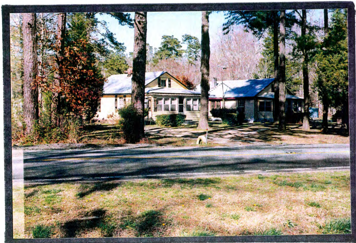
Property #12 Southwest elevation
