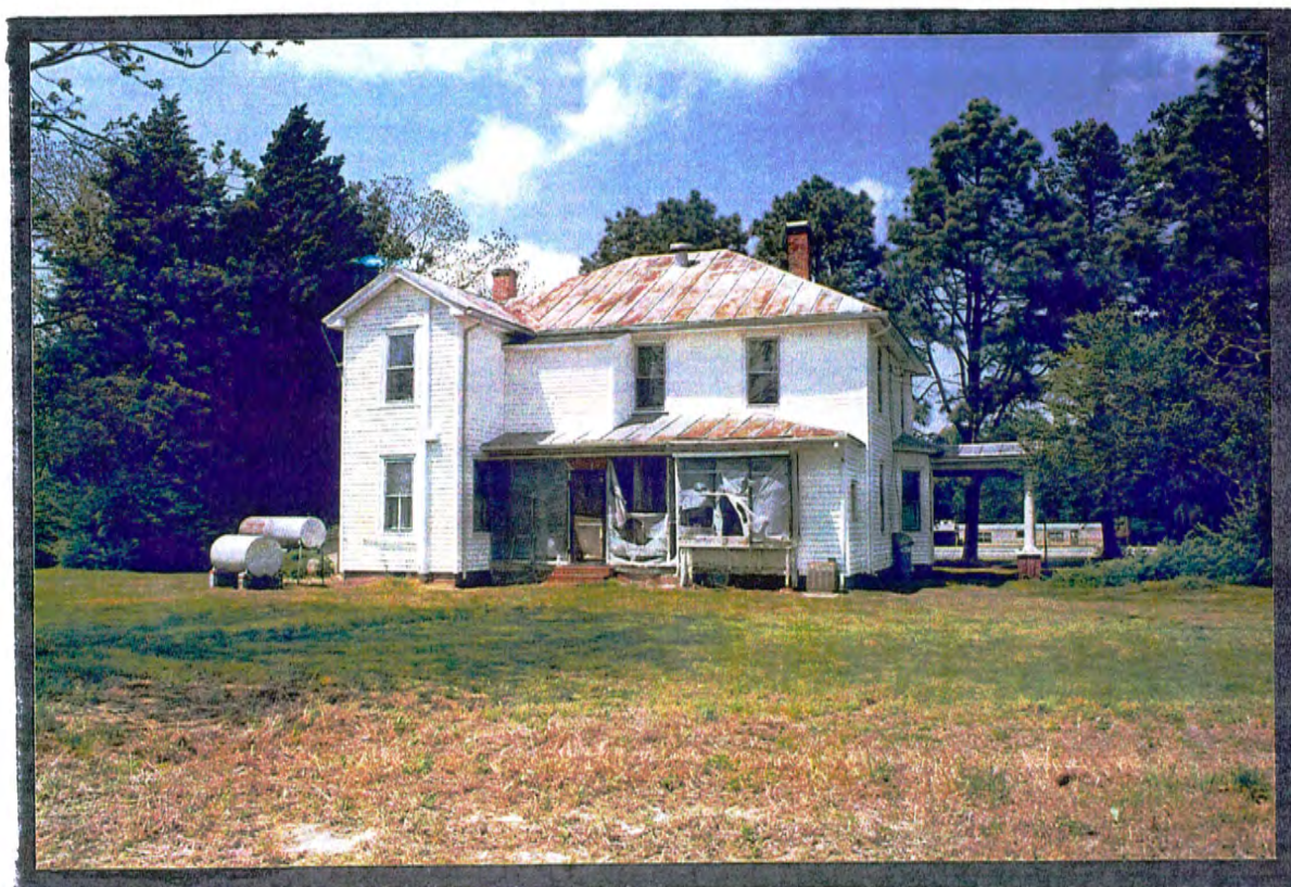
Property #6 Tarkenten House South elevation
