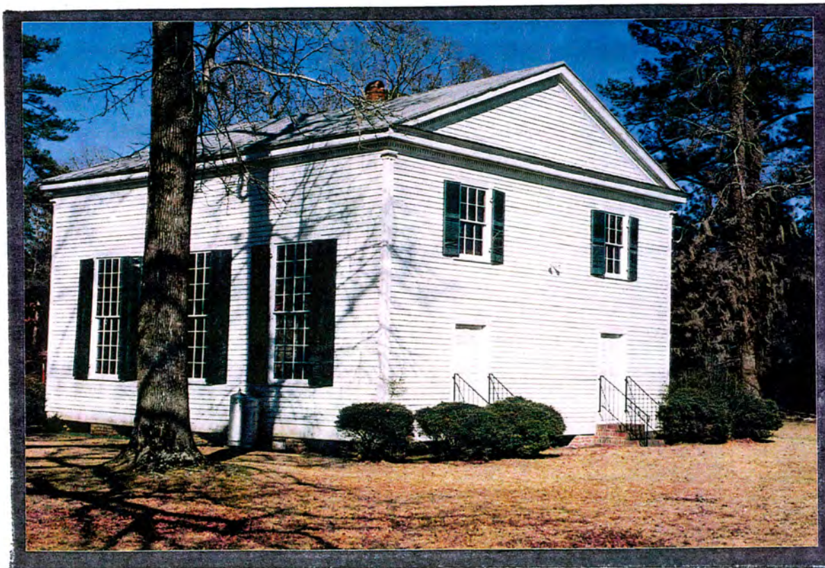
Property #11 Rehoboth Methodist Church (NR) Southwest elevation
