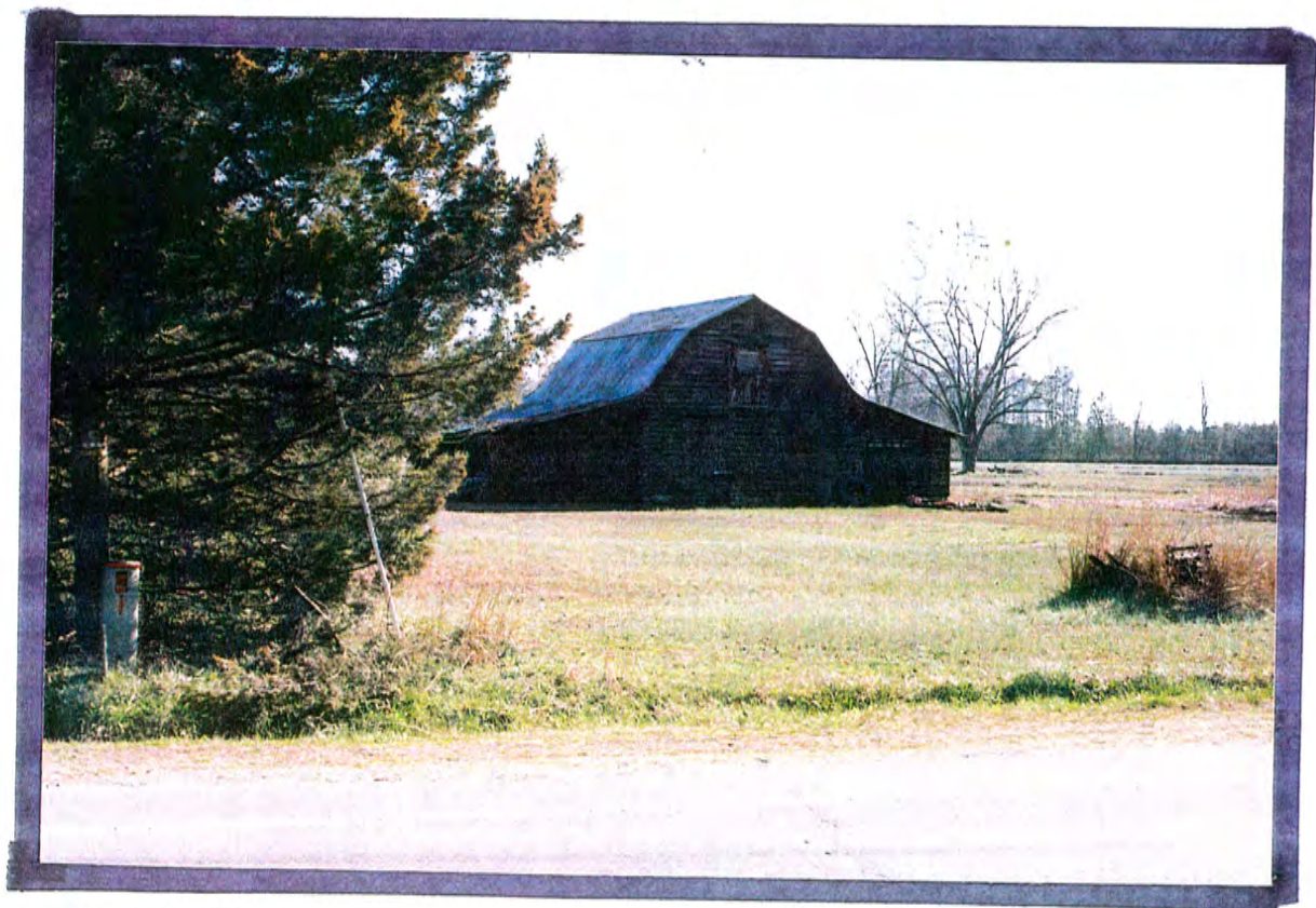
Property #8 North elevation of barn
