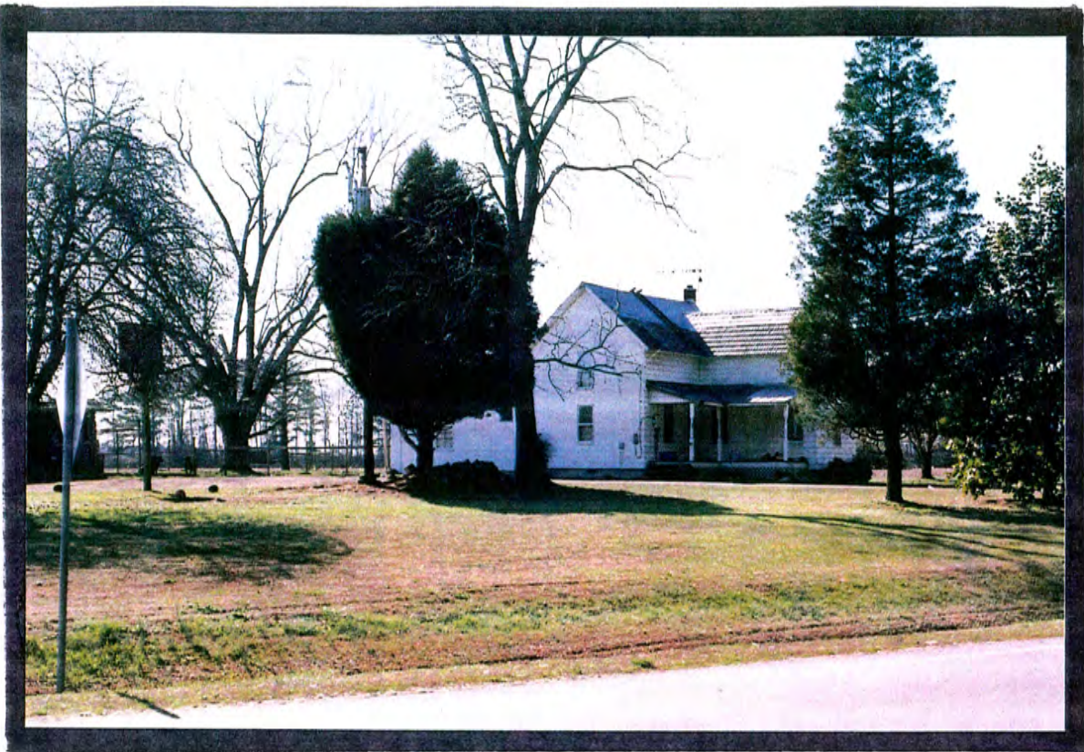
Property #3 East elevation of house
