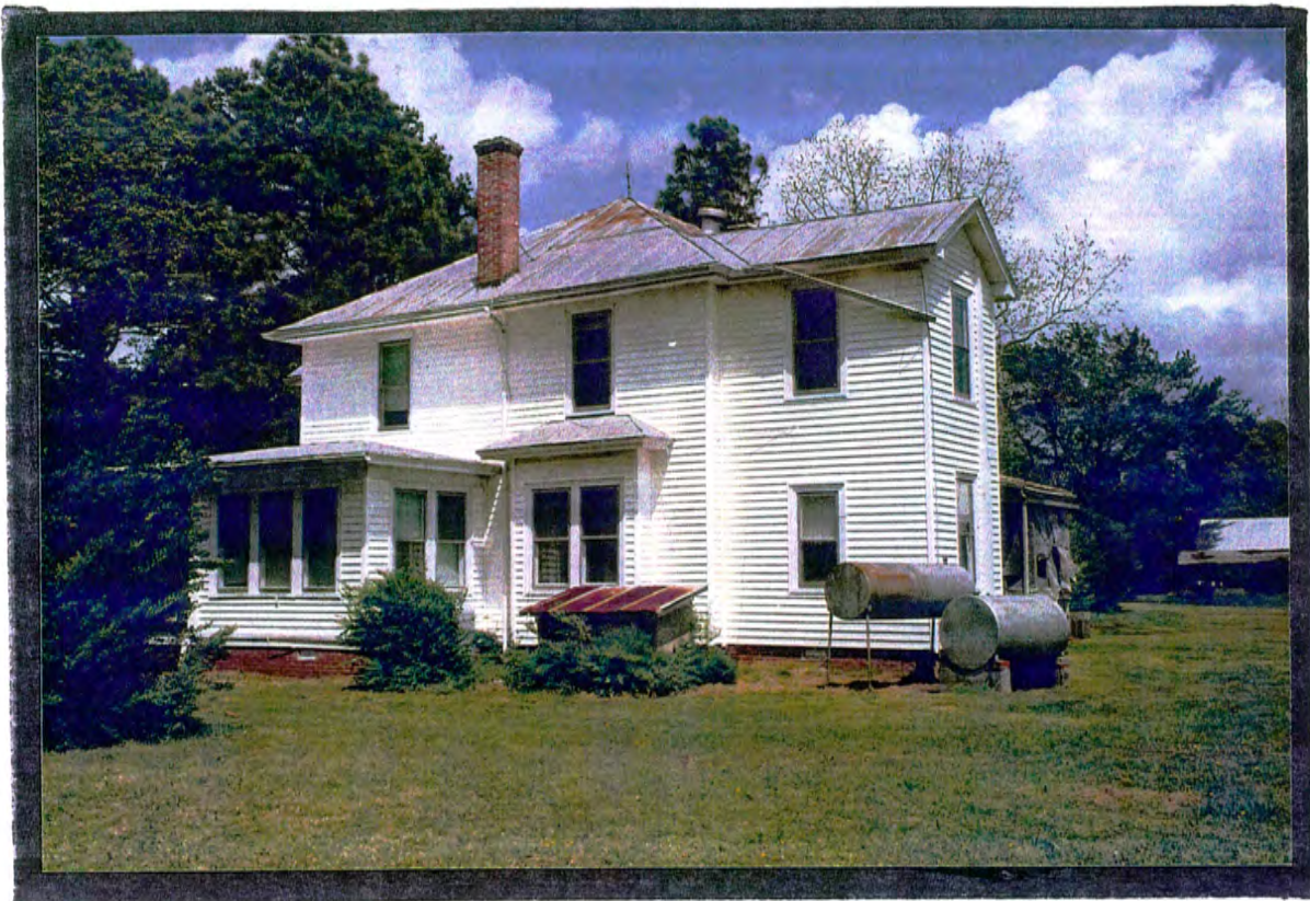
Property #6 Tarkenten House West elevation
