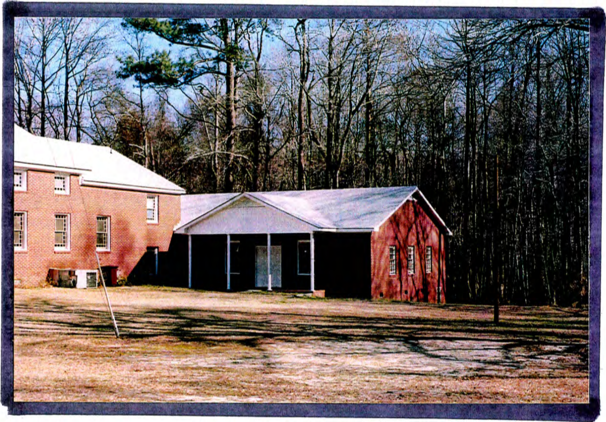
Property #5 Oak Grove Baptist Church Southwest elevation showing addition
