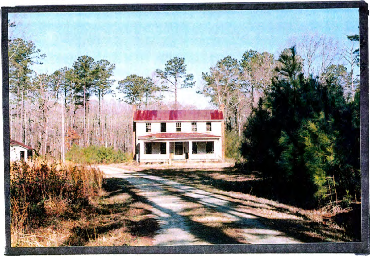
Property #10 Southeast elevation (close-up)
