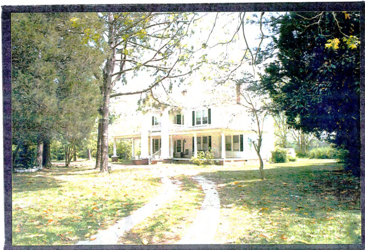
Property #6 Tarkenten House Northwest elevation
