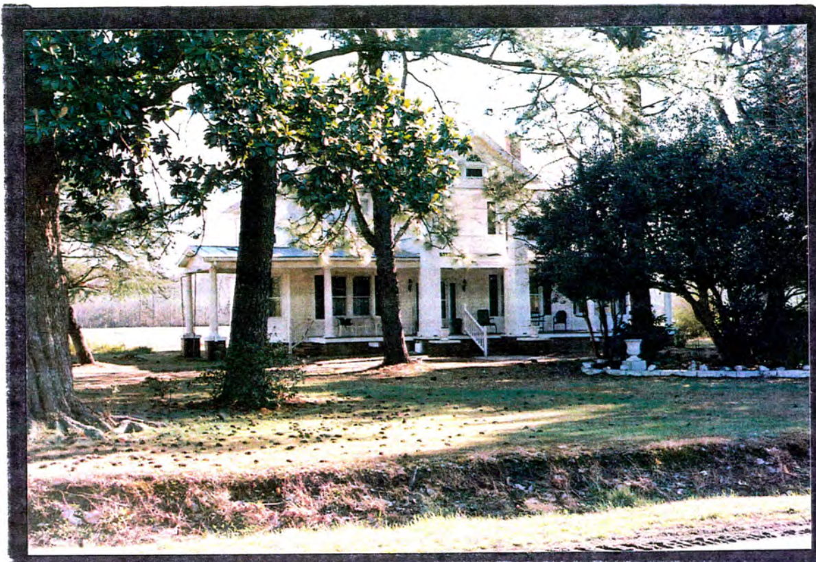
Property #6 Tarkenten House North elevation
