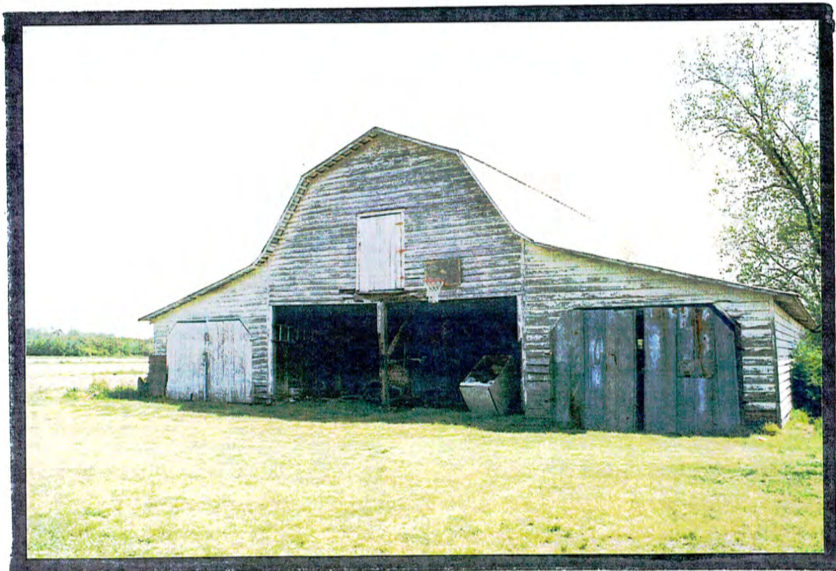
Property #6 Tarkenten House North elevation of barn
