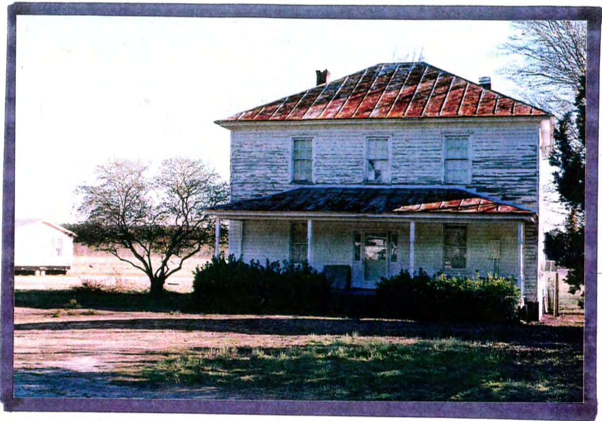
Property #8 North elevation of house
