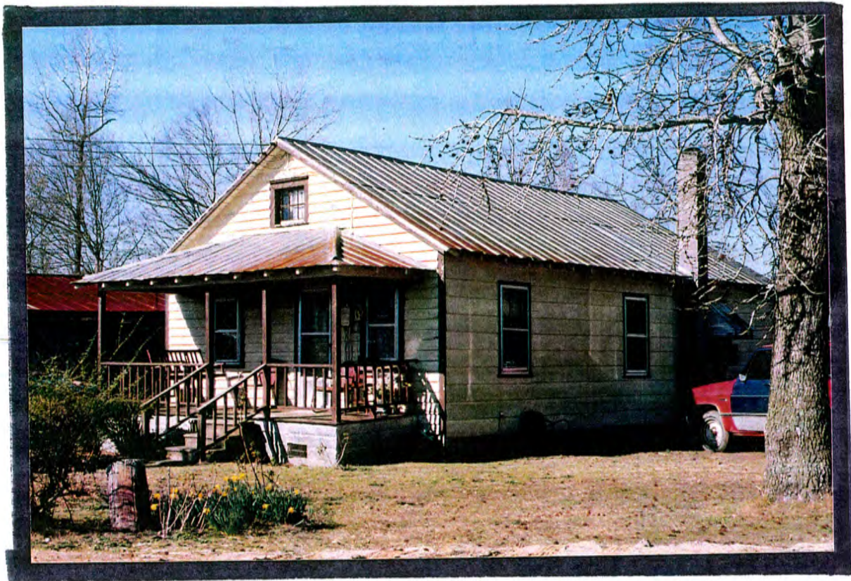
Property #4 Southeast elevation
