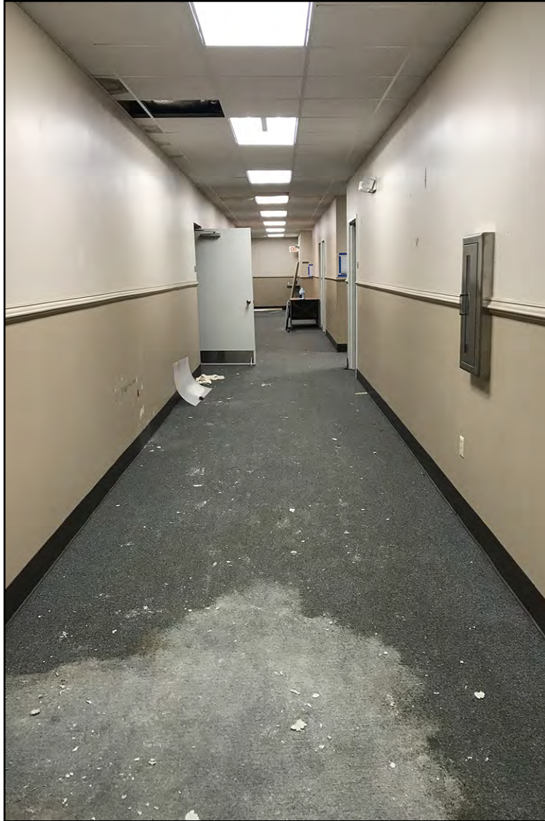
PLATE 27: Interior Hallway, Building 116 (NH2664), Looking East, New Hanover County, North Carolina
