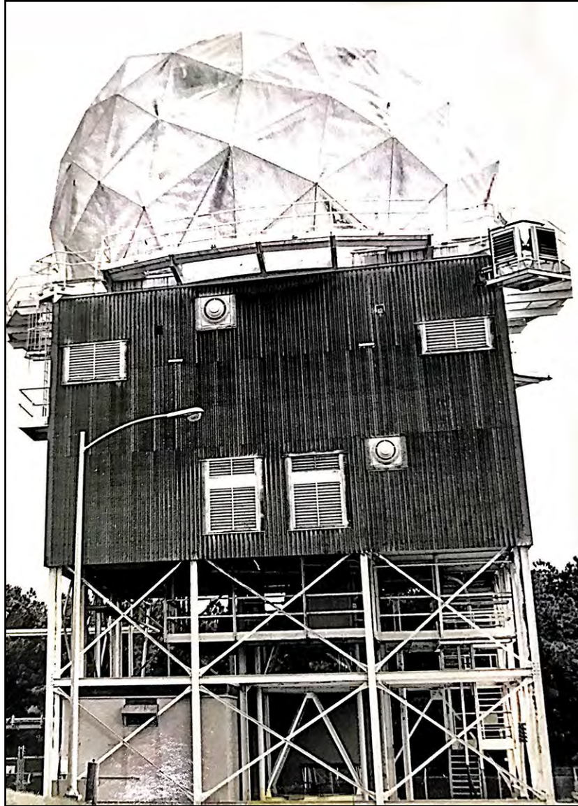
PLATE 2: Newly Constructed Radome Tower, Fort Fisher Air Force Radar Station, 1967 (North Carolina Military History Museum)
