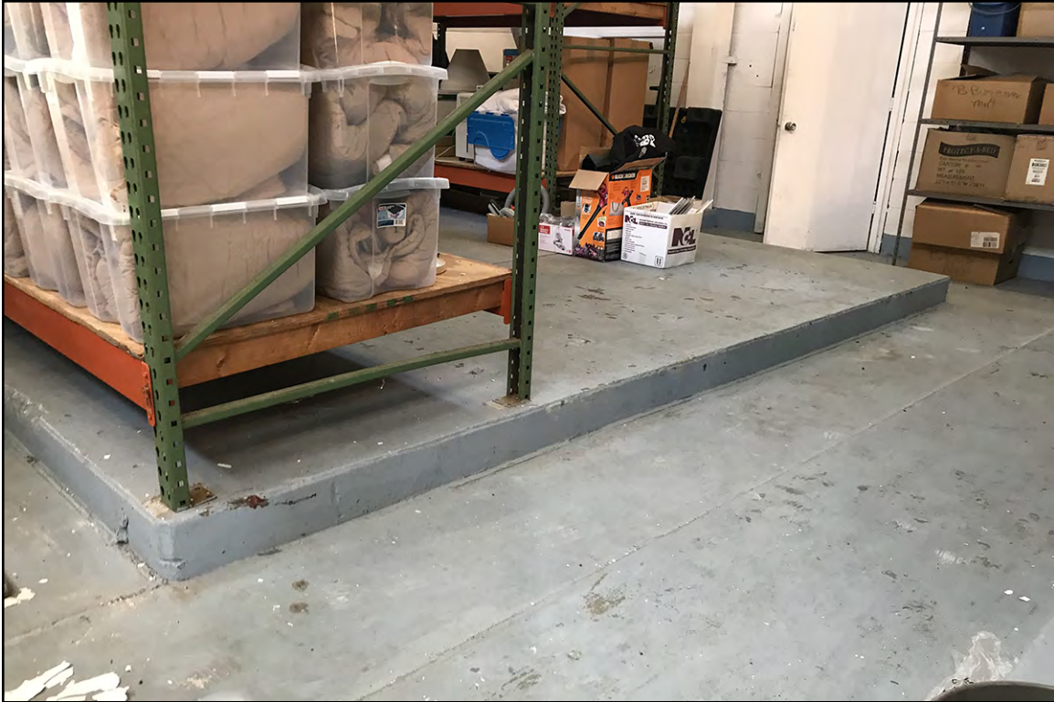
PLATE 36: Detail of Raised Concrete Platforms for Holding Generators in the Power Plant, Building 117, New Hanover County, North Carolina, Looking Northwest
