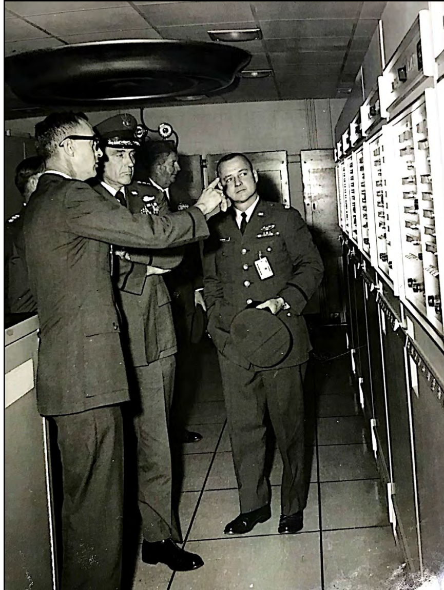
PLATE 31: Interior of Control/Command Room of Building 116, 1969 (North Carolina Military History Museum)
