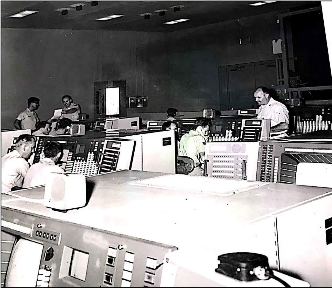
PLATE 5: Interior of Primary Operations/Control Room of BUIC Facility (Building 116), ca. 1969 (North Carolina Military History Museum)
