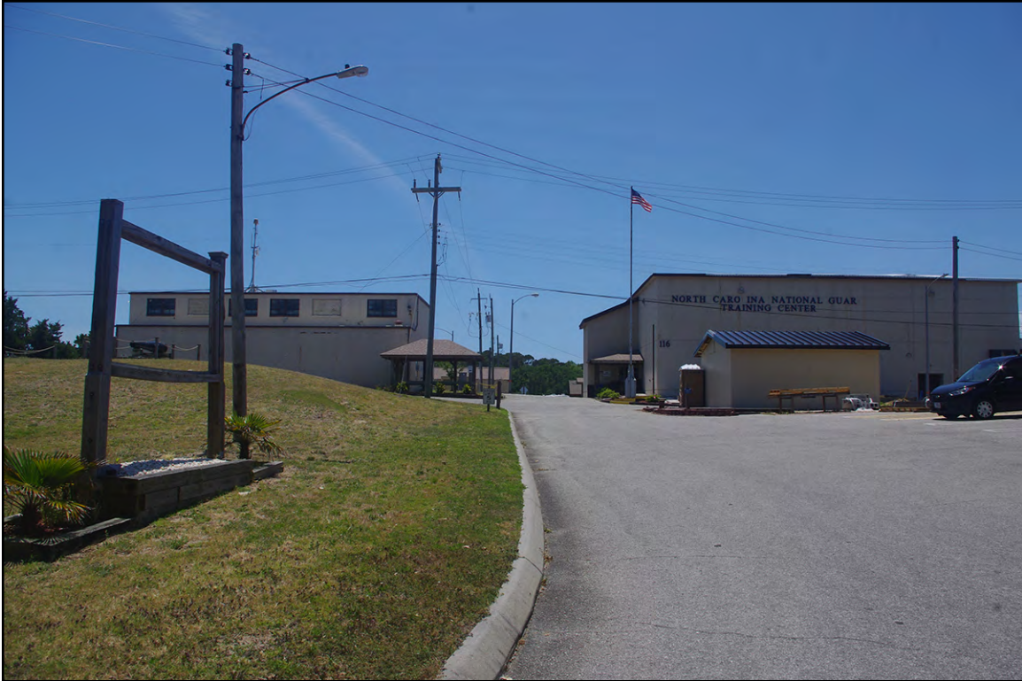
PLATE 17: Building 116 (NH2664), North Elevation, Looking South from Parking Lot of Entrance to Buildings 116 and 117, New Hanover County, North Carolina
