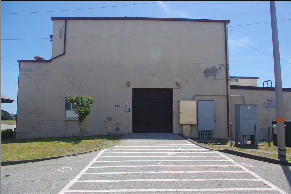
PLATE 34: West Elevation, Building 117, New Hanover County, North Carolina, Looking East
