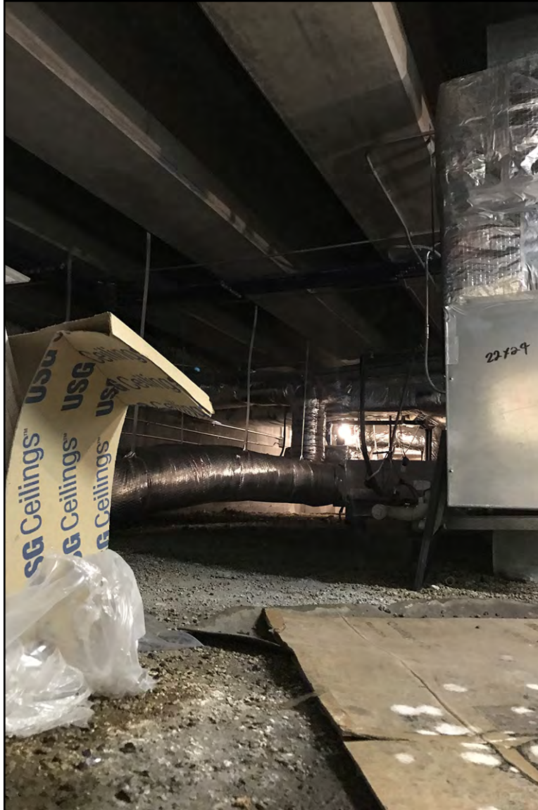
PLATE 30: Detail of Concrete Framing Structure in Attic, Building 116 (NH2664), New Hanover County, North Carolina
