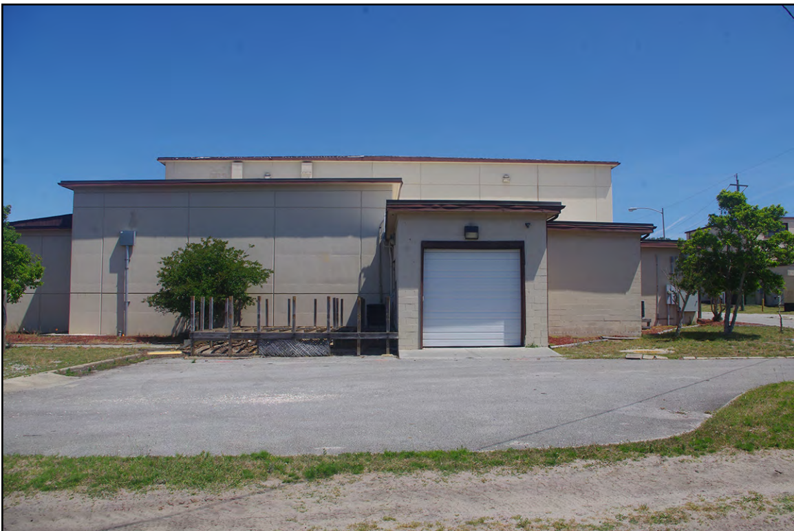
PLATE 23: Building 116 (NH2664), South Elevation, New Hanover County, North Carolina, Looking North
