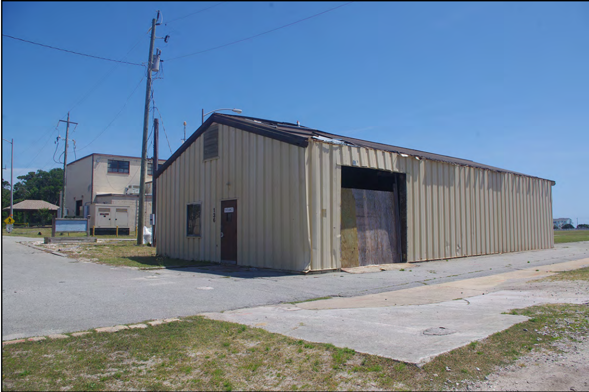
PLATE 40: Building 136, New Hanover County, North Carolina, Looking Northeast
