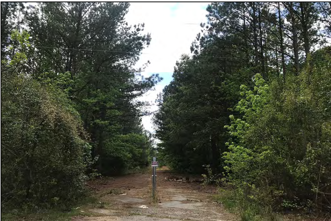
PLATE 13: Main Access Road (Airbase Road) with Former Buildings and Facilities Blocked, at (former) Roanoke Rapids Air Force Radar Station (HX315), Halifax County, North Carolina
