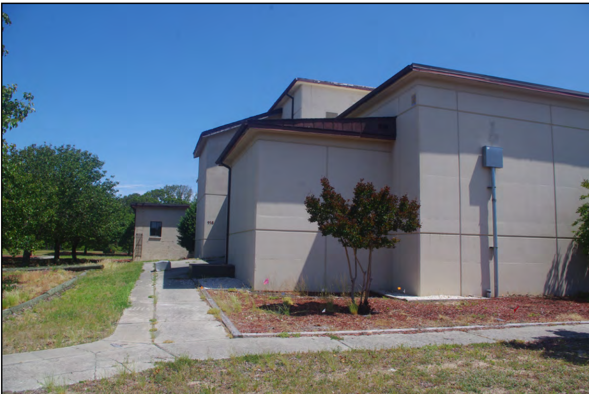
PLATE 25: Oblique View of West Elevation, Building 116 (NH2664), New Hanover County, North Carolina, Looking Northeast
