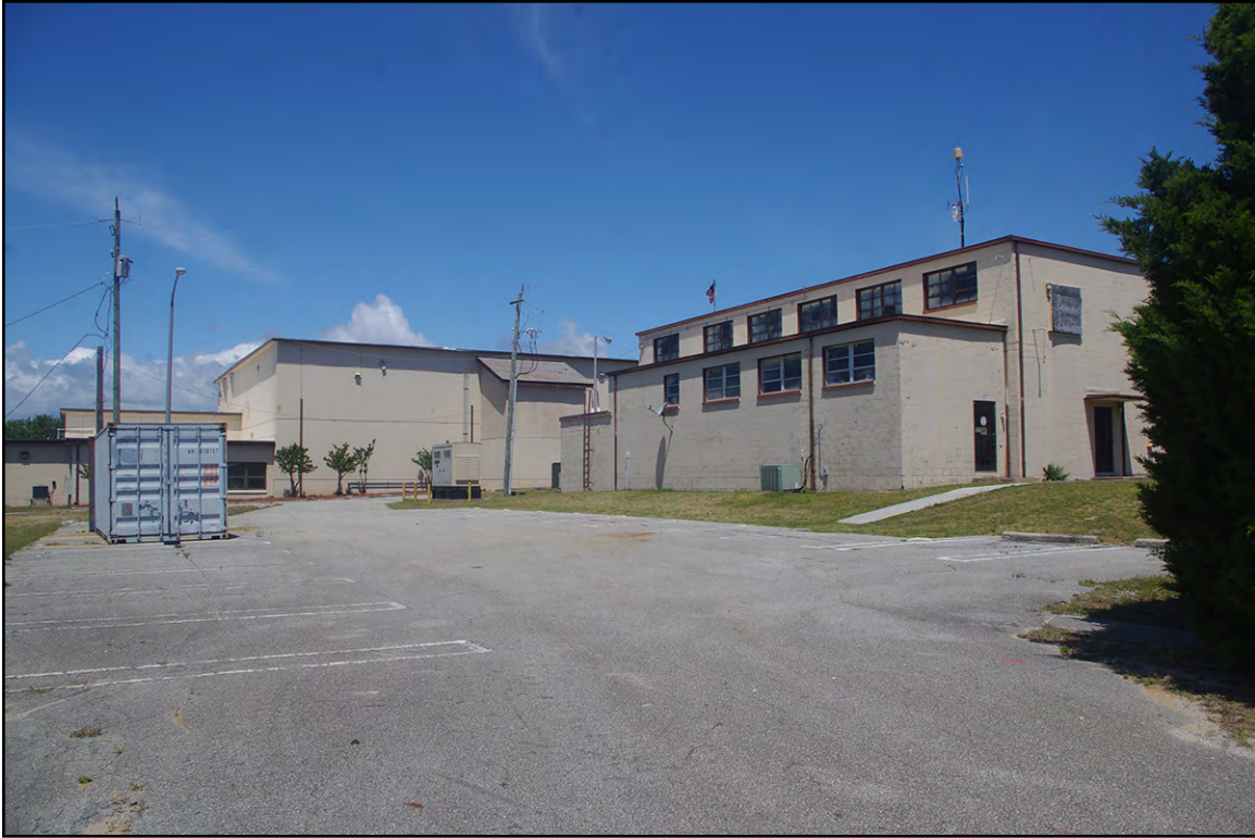
PLATE 32: Oblique View of South Elevation, Building 117, New Hanover County, North Carolina, Looking Northwest
