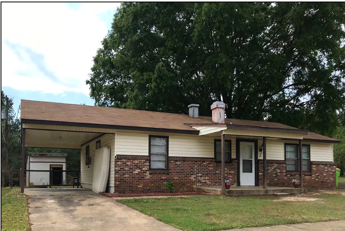
PLATE 15: Typical One-story House Constructed for Family Housing at (former) Roanoke Rapids Air Force Radar Station (HX315), Halifax County, North Carolina, Looking North
