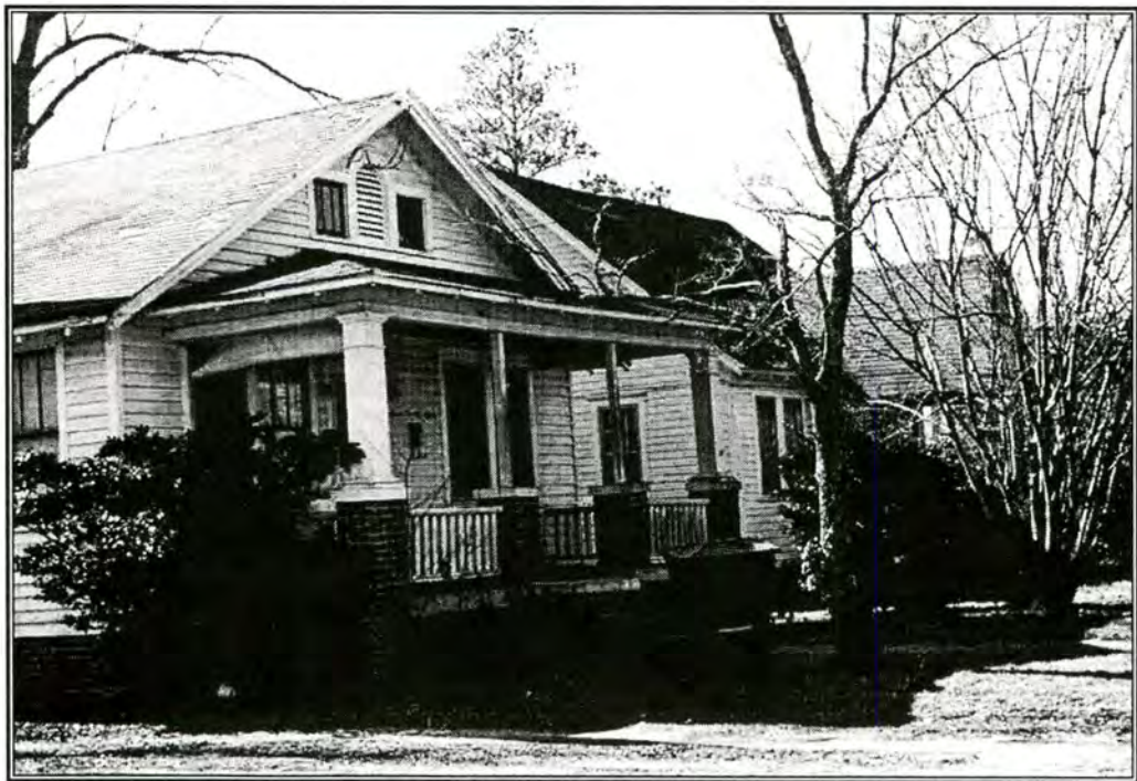
Photograph 7: Elizabeth City Iron Works-Aydlett Division Historic District, Morgan Street, looking southeast
