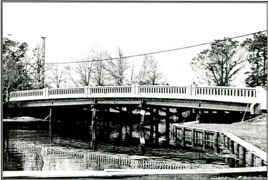
Photograph 3: Bridge No. 28, view looking northwest
