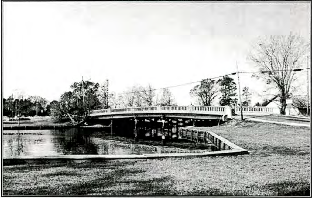
Photograph 2: Bridge No. 28, looking northwest
