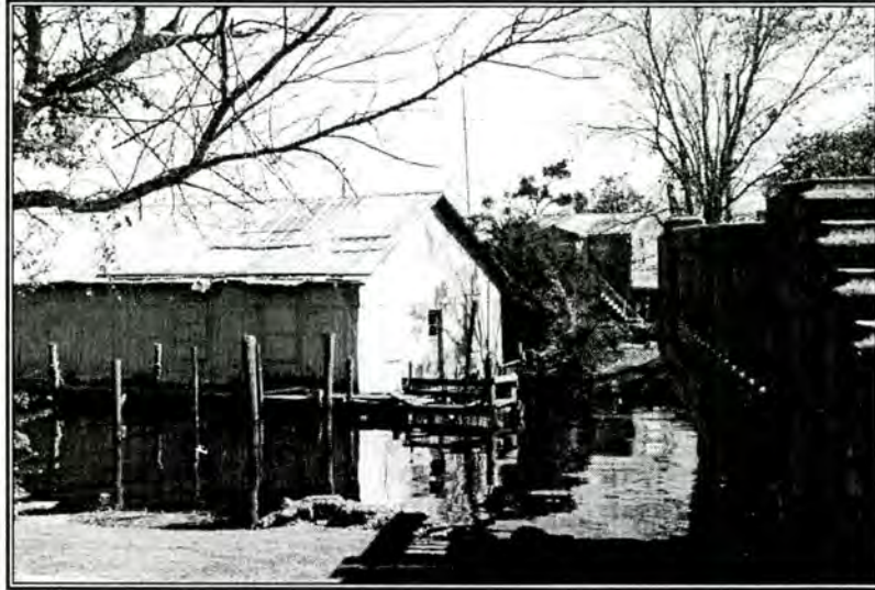
Photograph 6: Bridge No. 28, showing relationship between bridge and the Elizabeth City Iron Works-Aydlett Division Proposed Historic District
