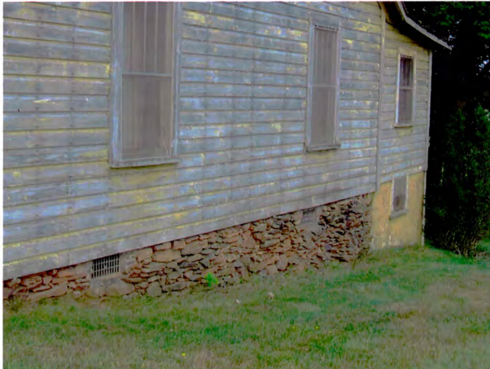
Figure 4B. Parsons House. West (rear) and south elevations (above), detail of dry-laid stone foundation, north elevation (below).
