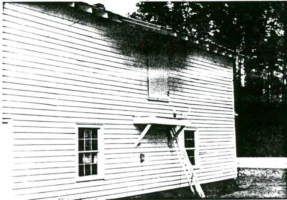
Plate 38. Griffen's Hatchery, showing added packhouse door & shed roof
