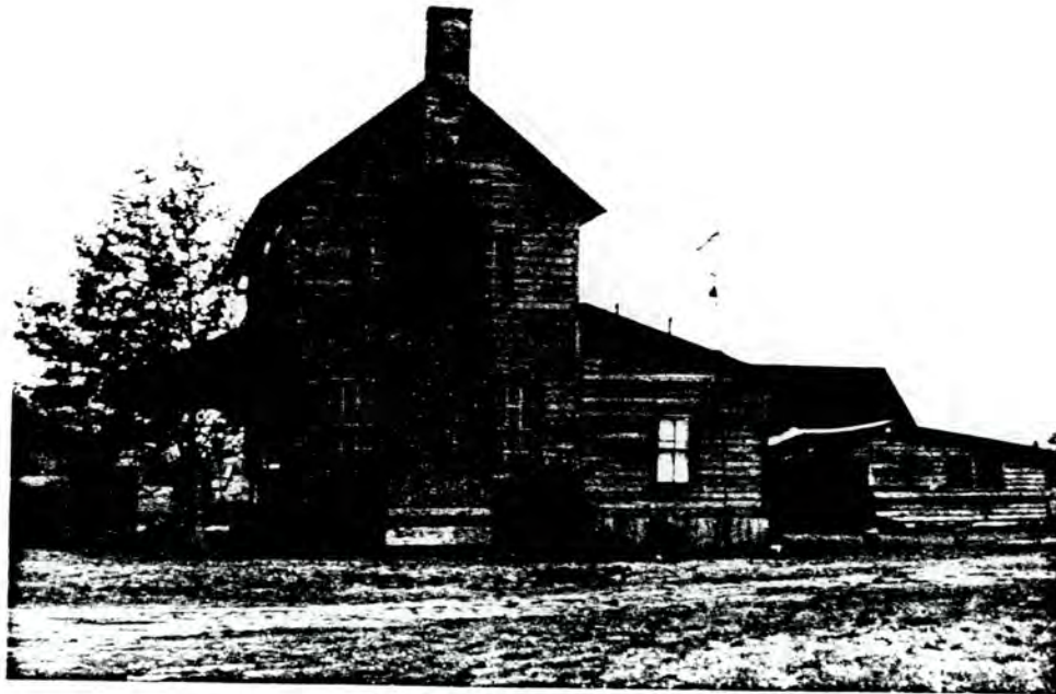
Plate 17. Woolard-Perry House, North Elevation
