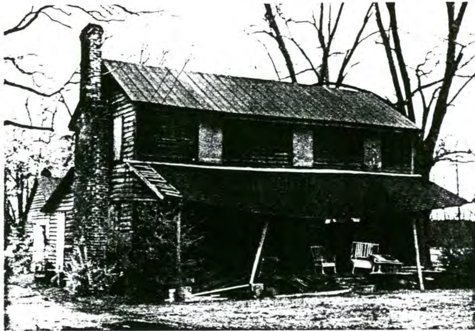
Plate 18. Hadley House, East Elevation
