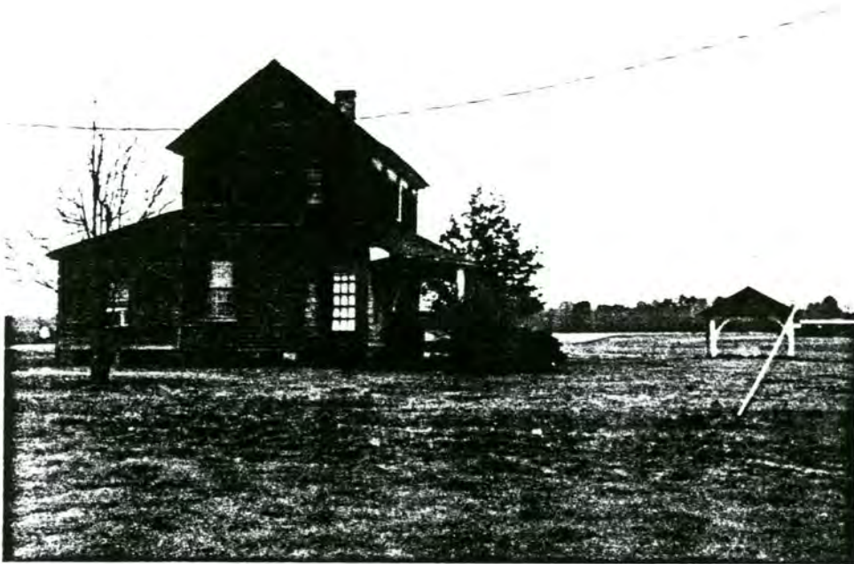
Plate 13. Woolard-Perry House, view north showing well house. March, 2000
