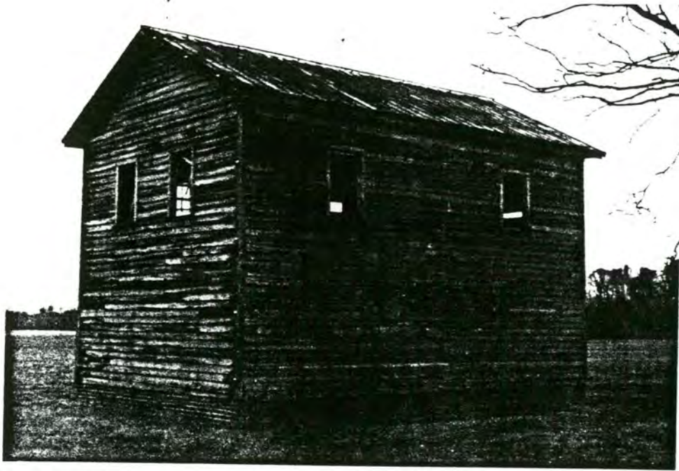
Plate 7. Smithwick-Green House, Packhouse, North and West Elevations, looking southeast, March 2000
