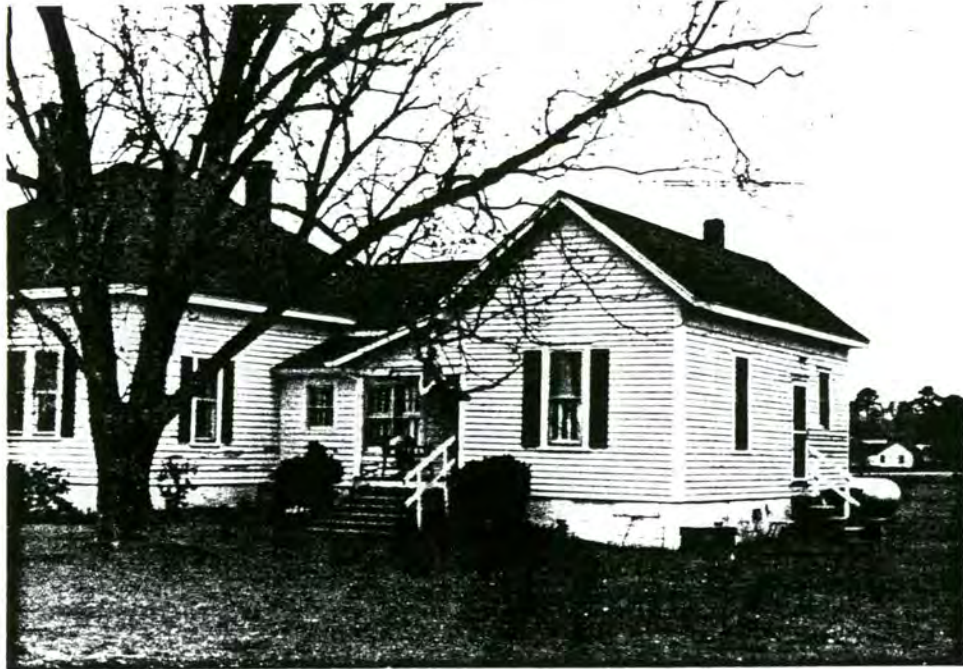
Plate 27. Ward House, East Elevation
