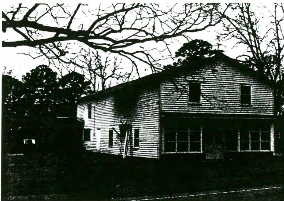
Plate 35. Griffen's Hatchery, South Elevation
