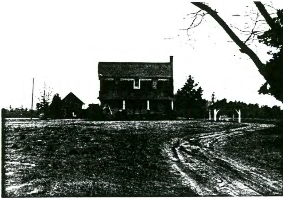
Plate 9. Woolard-Perry House, East Elevation, March 2000
