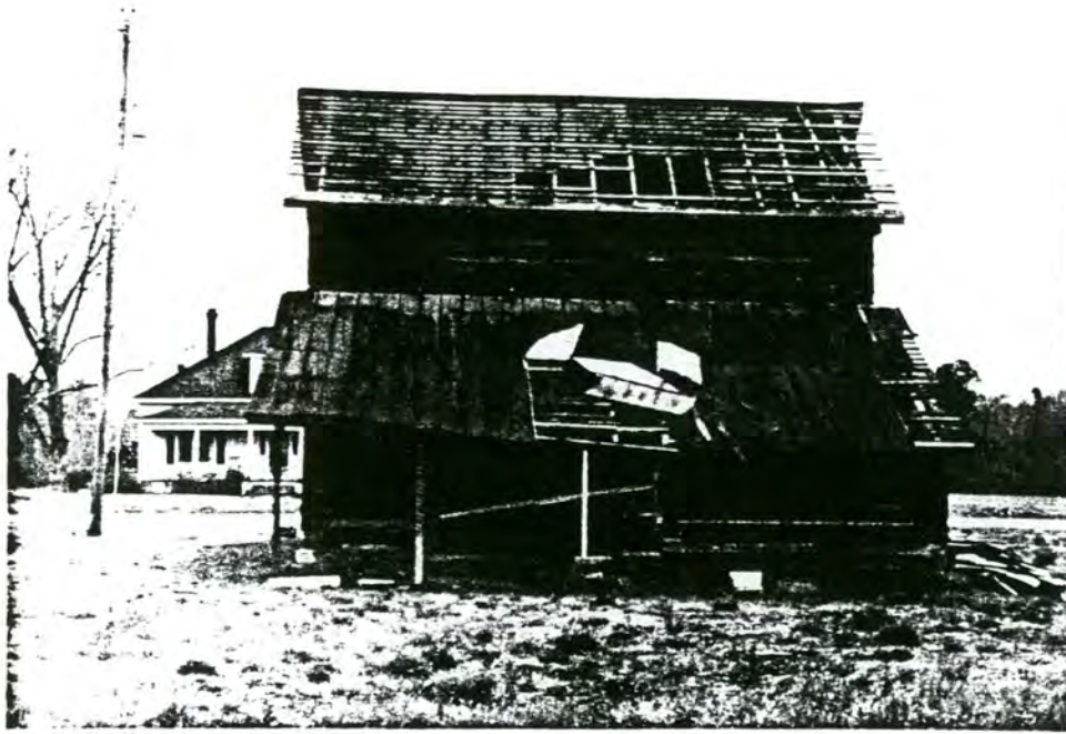
Plate 29. Ward Farm, Packhouse # 1, West Elevation
