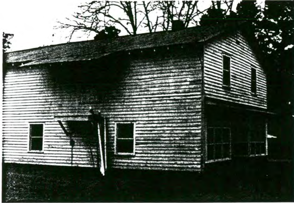
Plate 37. Griffen's Hatchery, showing added packhouse door & shed roof
