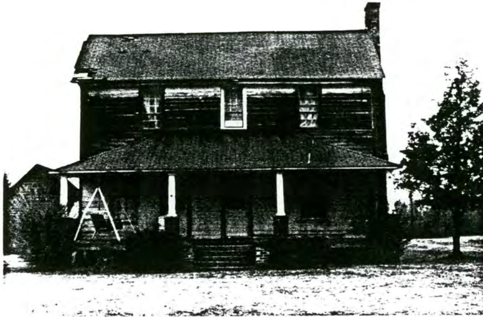
Plate 11. Woolard-Perry House, East Elevation, March 2000
