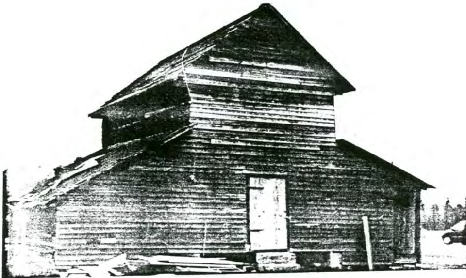
Plate 30. Ward Farm, Packhouse # 1, South Elevation
