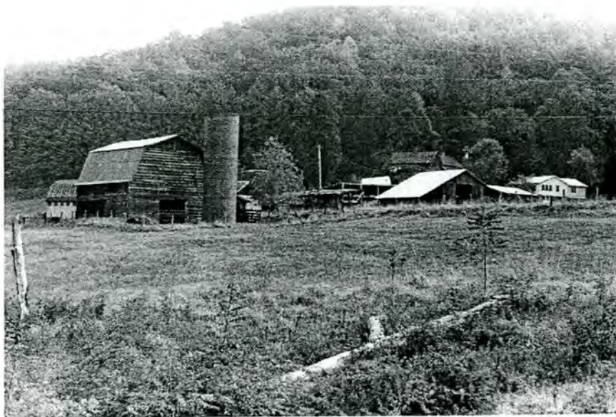
Plate 6. Slagle Farm, Farm Complex, Looking North from Bridge No. 16.
