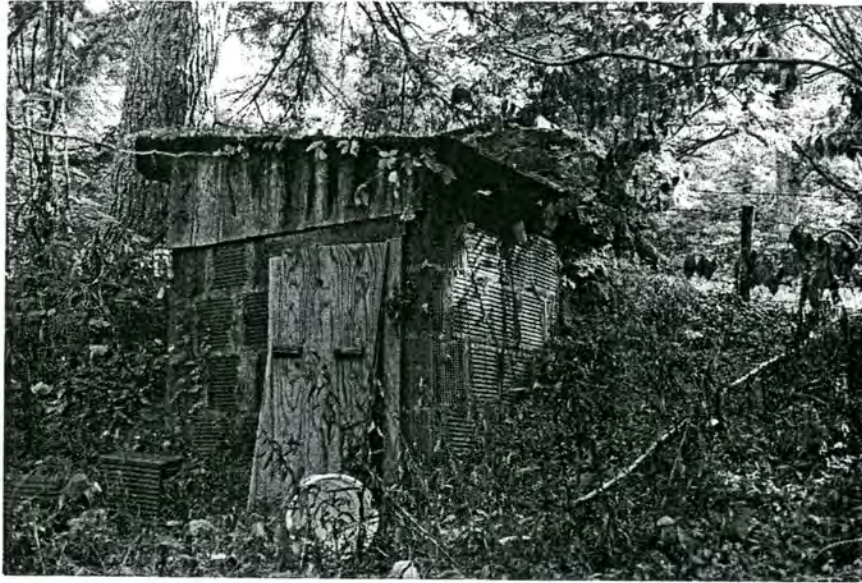
Plate 13. Slagle Farm, Canning House.
