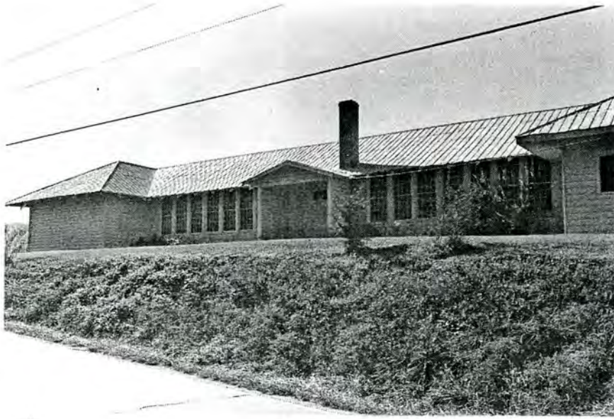
Plate 3. Stoney Fork School, Front Facade, Looking West.
