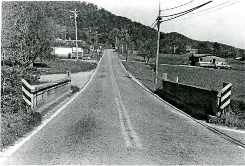
Plate 24. Bridge No. 181, Looking North.
