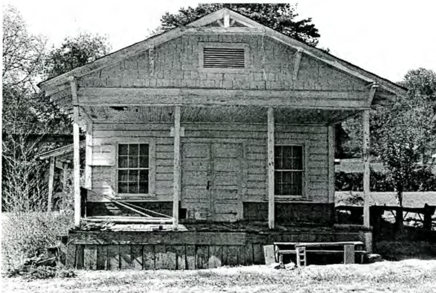
Plate 15. Davis Store, Front Facade, Looking West.
