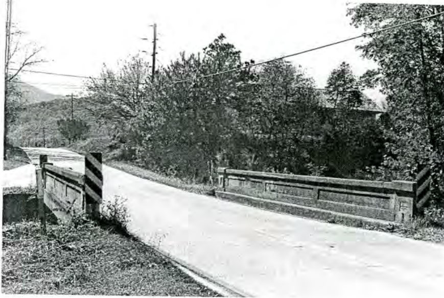
Plate 26. Bridge No. 181, Looking South.
