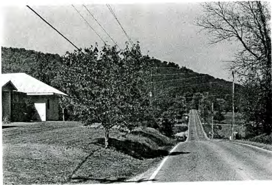
Plate 2. Stoney Fork School and Setting, Looking North towards Bridge No. 181.
