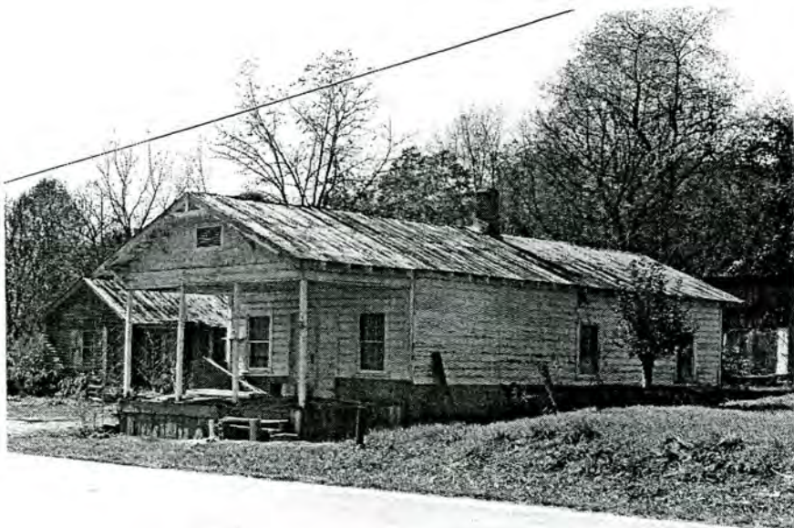
Plate 13. Davis Store and Feed Mill, Looking Southwest.
