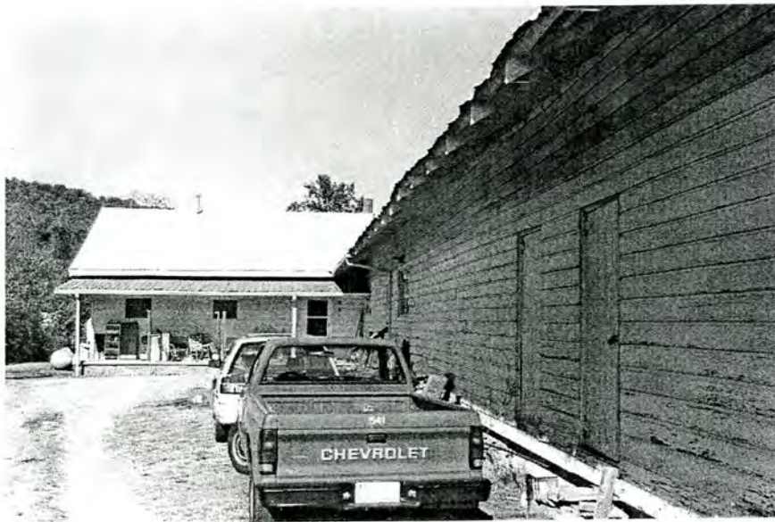
Plate 6. Stoney Fork School, Rear Elevation and Rear Wing, Looking North.
