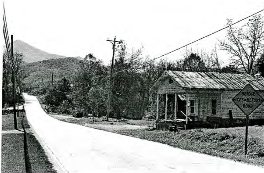
Plate 23. Davis Store and Feed Mill, Looking South.
