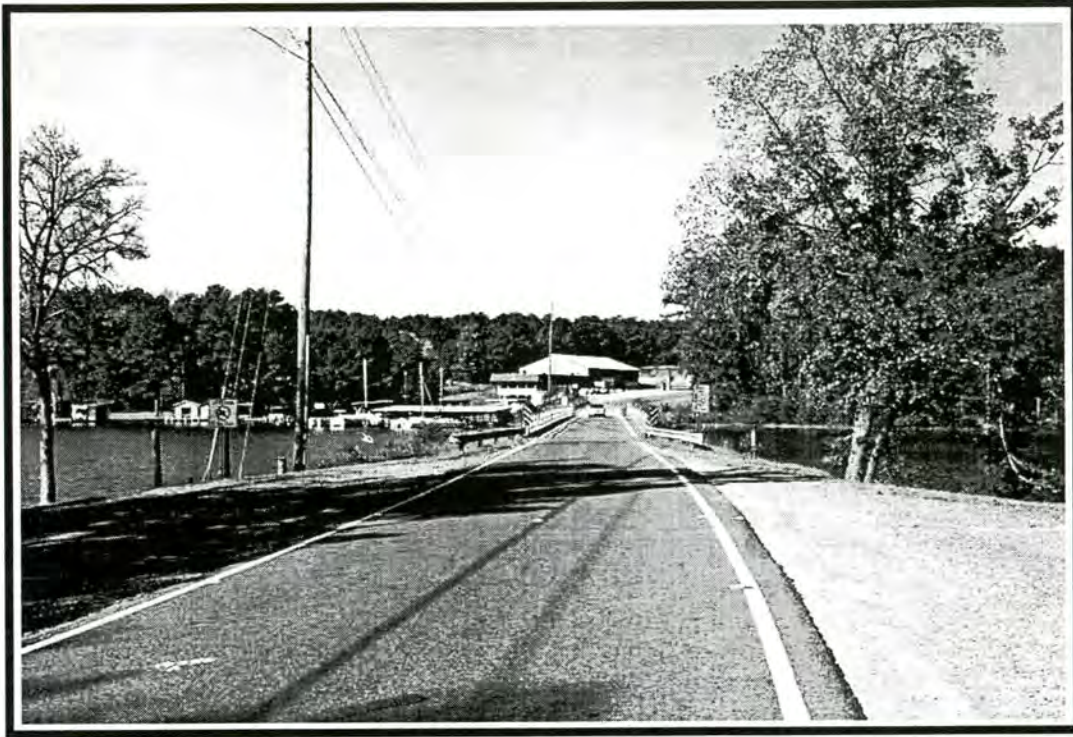
Figure 4 – View of Bridge No. 26 from SR 1110, looking west
