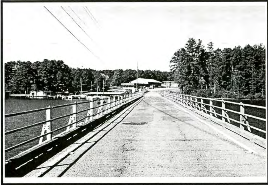
Figure 6 – View of Bridge No. 26, roadway and bridge railing
