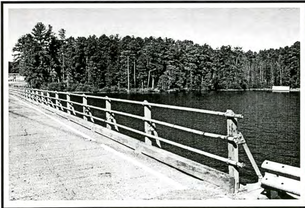
Figure 7 – View of Bridge No. 26, bridge railing
