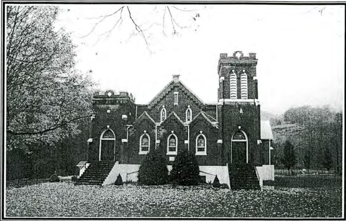
Figure 3 - Henson United Methodist Church
