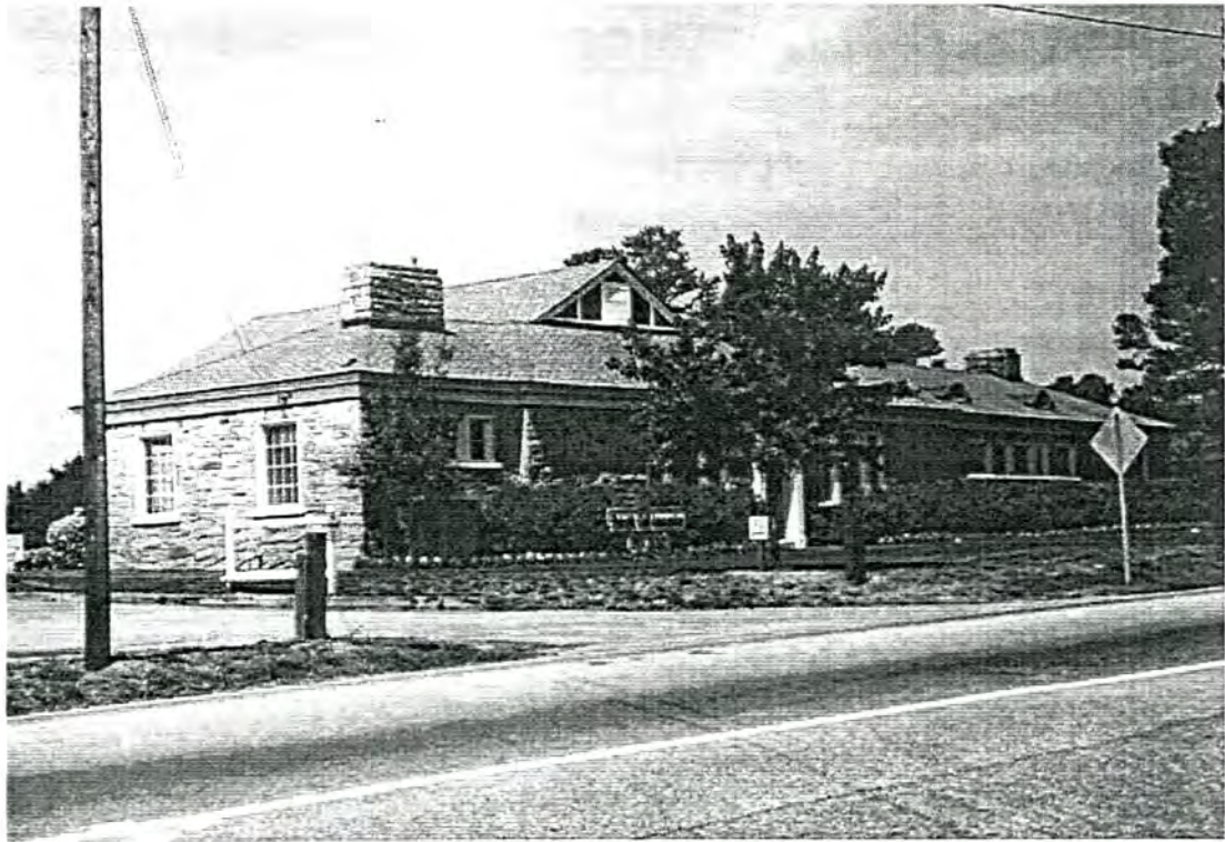
Raleigh Golf Association Clubhouse, view facing southwest
