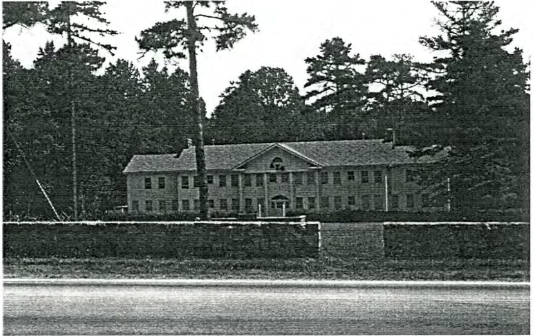
View of Carolina Pines Hotel, facing north
