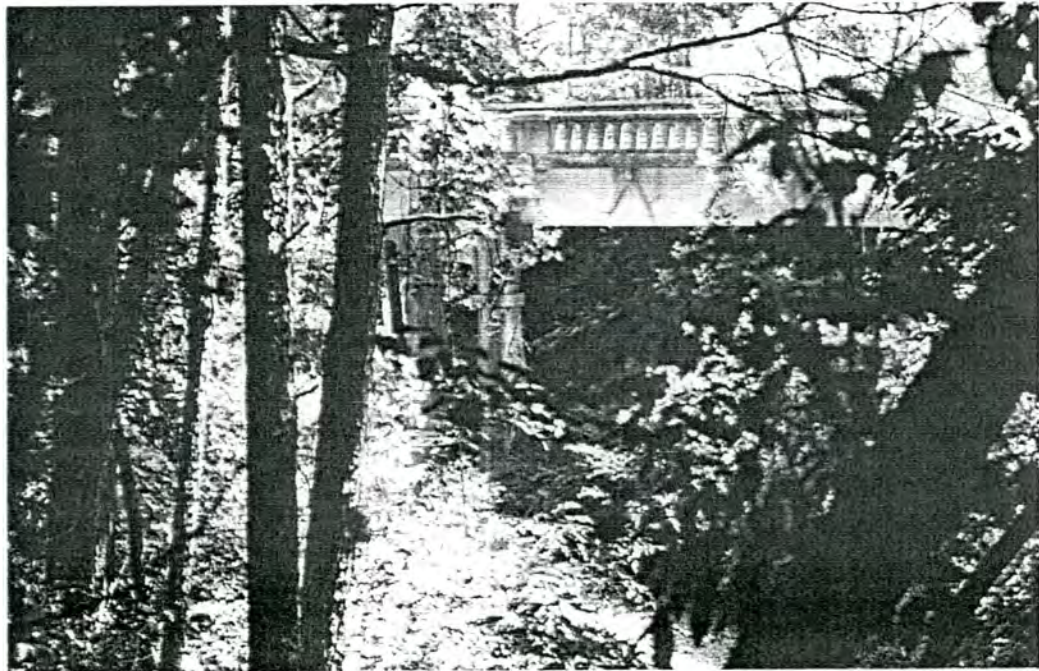
Bridge No. 269, detail, view facing northeast
