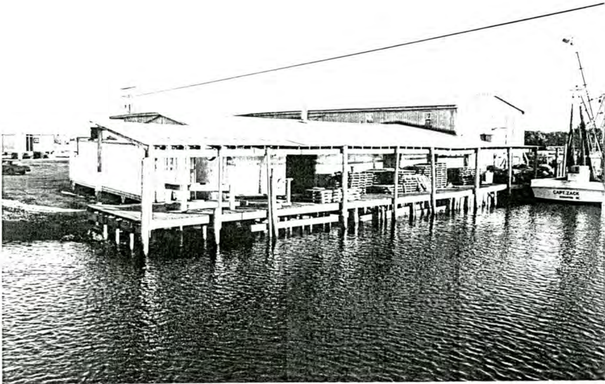
Plate 2: West side elevation of Rose Bay Oyster Company from Hyde County Bridge No. 32
