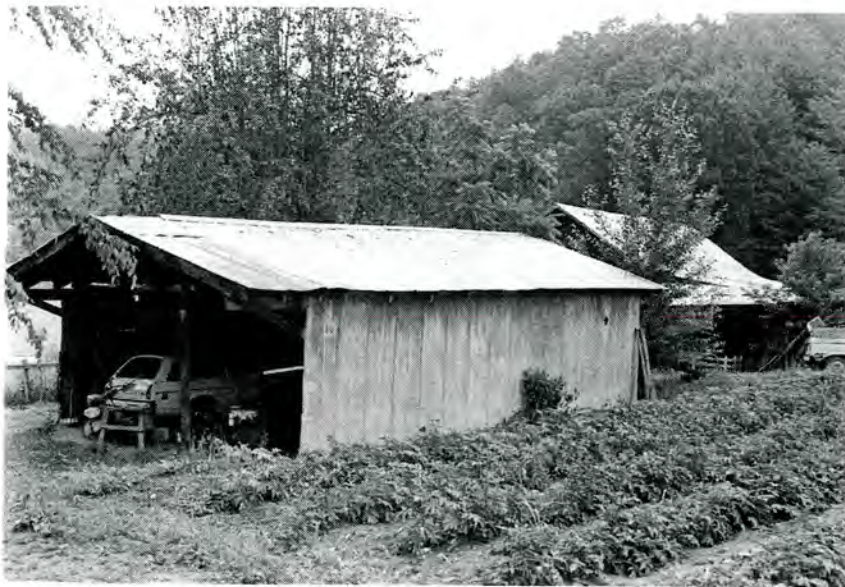
Plate 10. Peek Farm, Garage, South and East Elevations.
