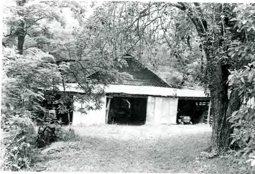
Plate 9. Peek Farm, Barn Entrance and South Elevation.
