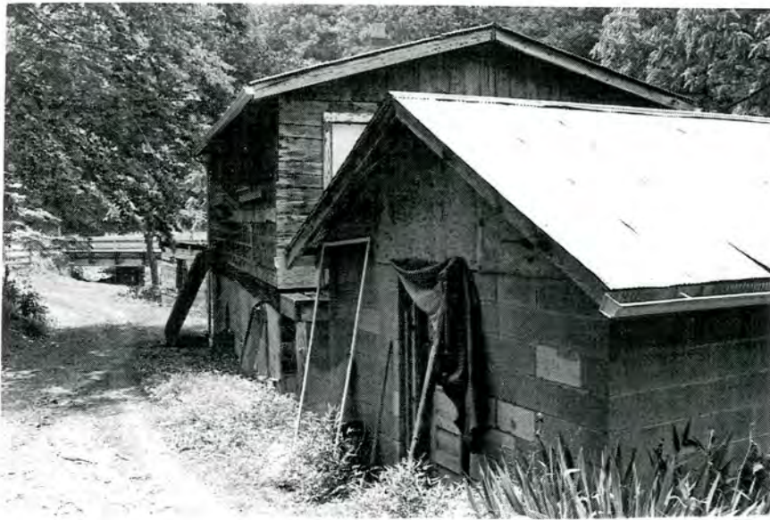
Plate 15. Peek Farm, Storage Buildings, Looking South.
