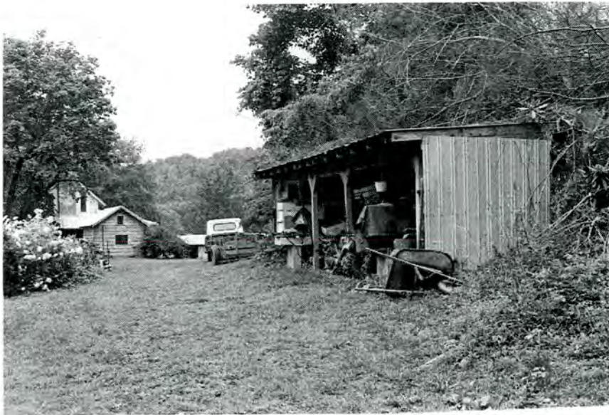
Plate 12. Peek Farm, Equipment Shed (Springhouse in Background), Looking Northeast.
