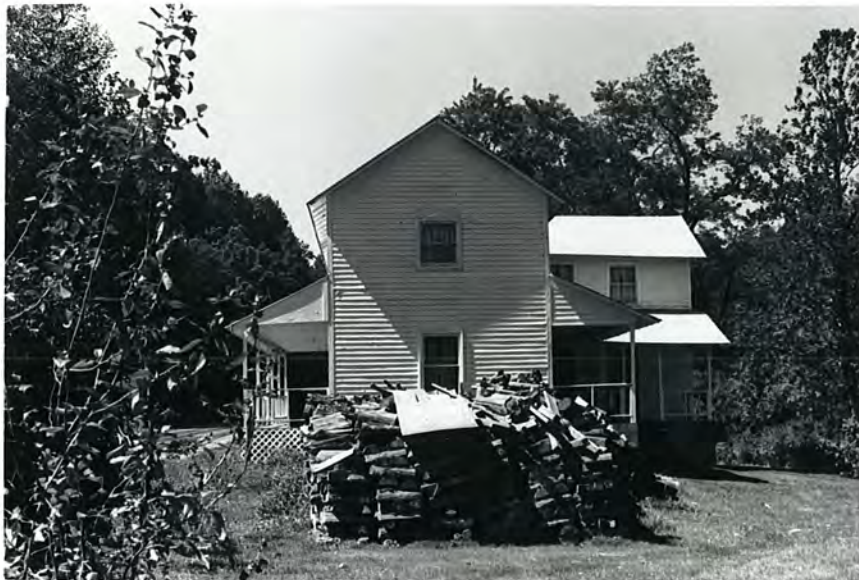
Plate 10. House (No. 4), East Elevation and Rear Ell, Looking West.
