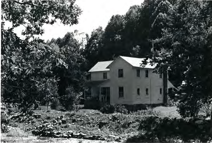
Plate 11. House (No. 4), West Elevation and Rear Ell, Looking Southeast from across the Elk River.
