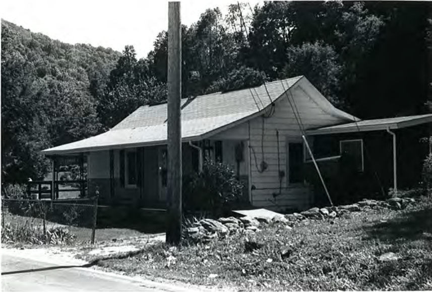
Plate 5. House (No. 3), Looking Southeast from S.R. 1321.
