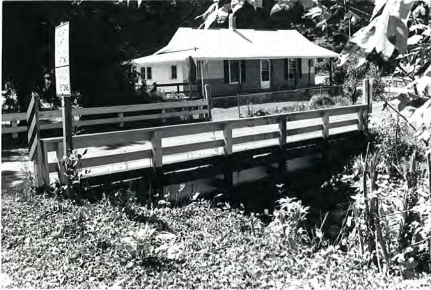
Plate 1. Bridge No. 28, Looking Southwest (House No. 3 in Background).
