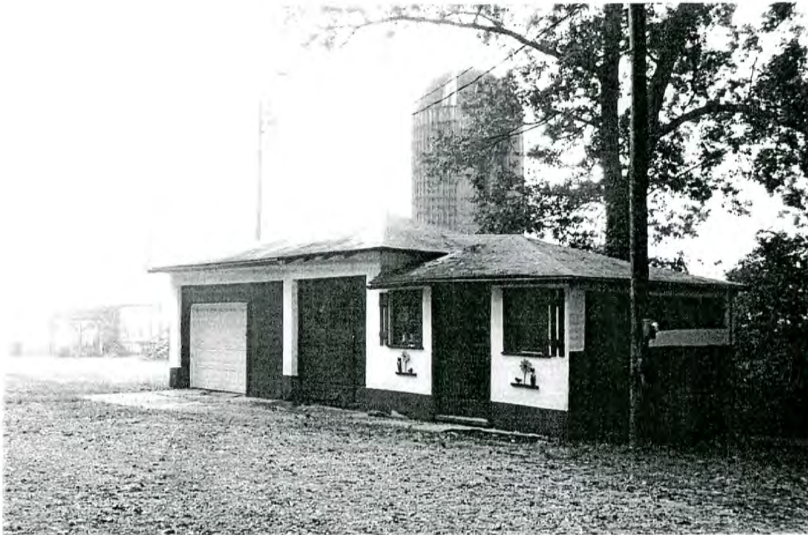
Plate 32: Merchant- Goodson House—garage, northeast front and northwest side elevations
