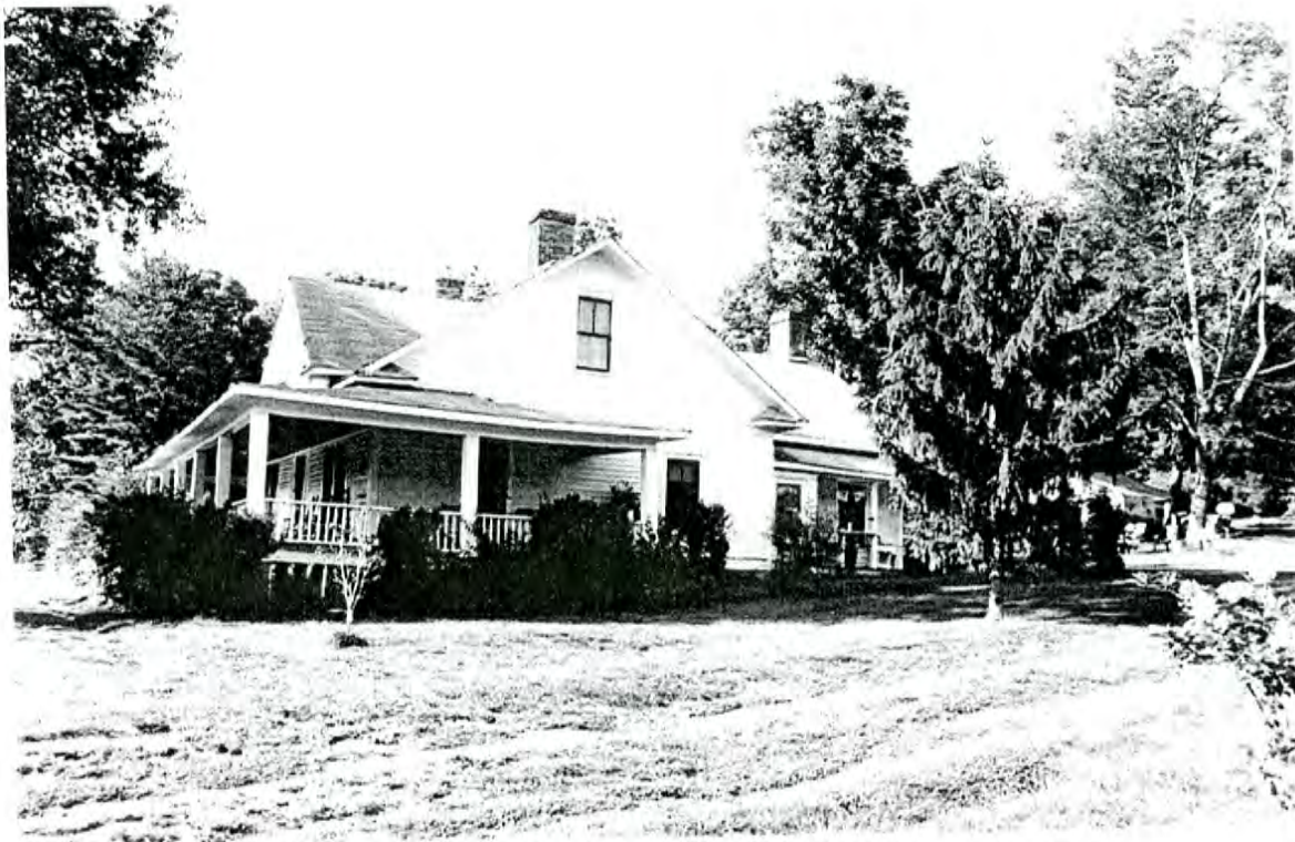
Plate 74: Jamison House—house, southeast side and southwest front elevations
