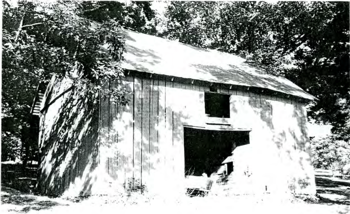
Plate 79: Jamison House-barn, looking west
