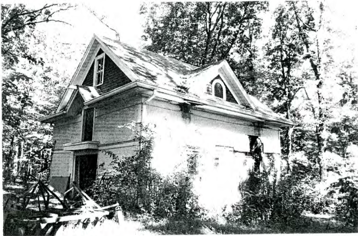
Plate 21: T. Jackson Henderson Estate—barn, south and west elevations
