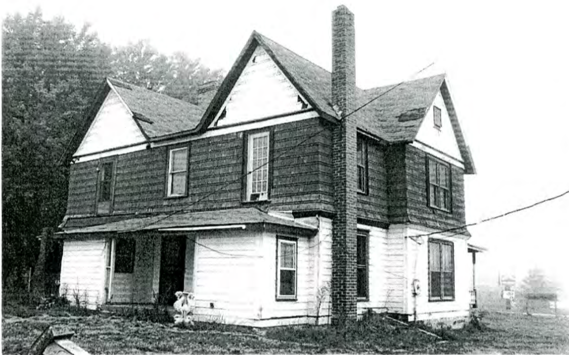
Plate 40: Dr. Solomon E. Greenwood House— southeast side and southwest rear elevations
