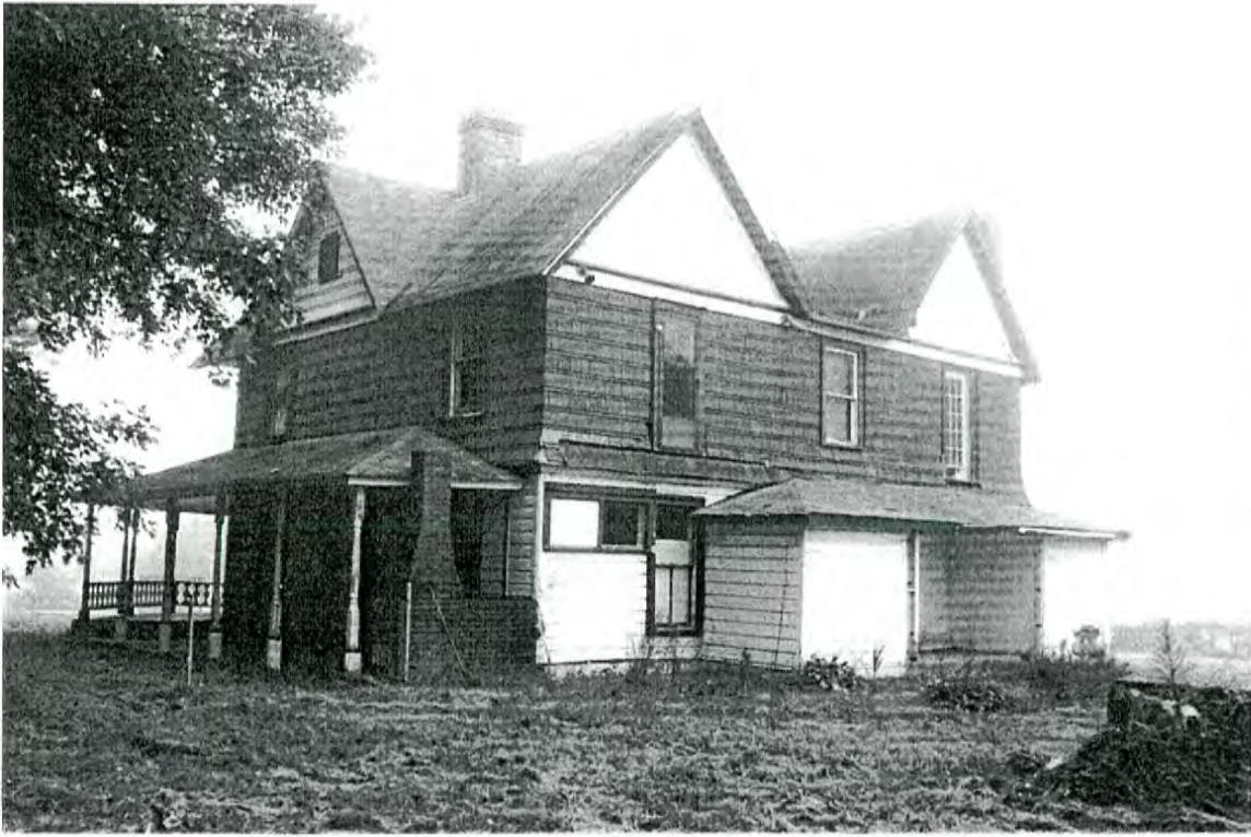
Plate 41: Dr. Solomon E. Greenwood House— southwest rear and northwest side elevations
