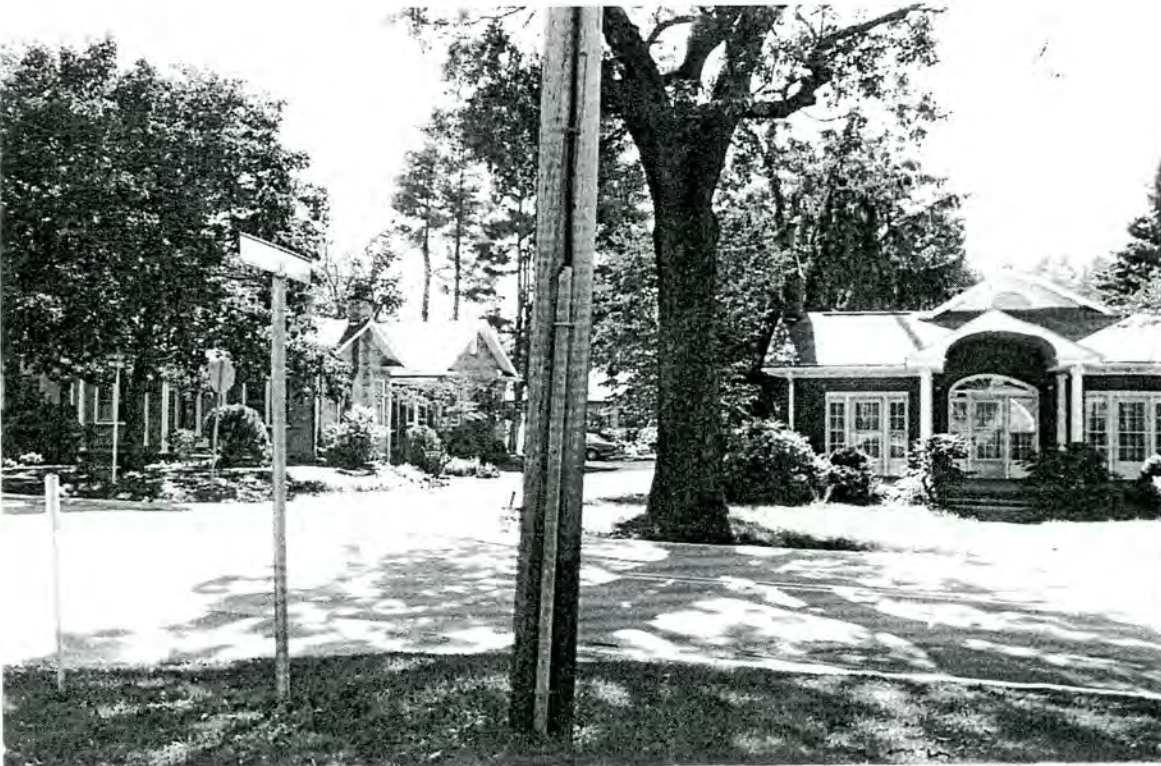
Plate 48: Druid Hills Historic District (Extension)— 1721, at left, and 1731, at right, Haywood Road, looking south
