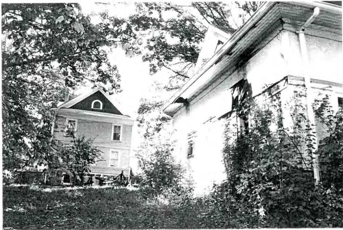
Plate 20: T. Jackson Henderson Estate— carriage house at left, east elevation; barn at right, south elevation
