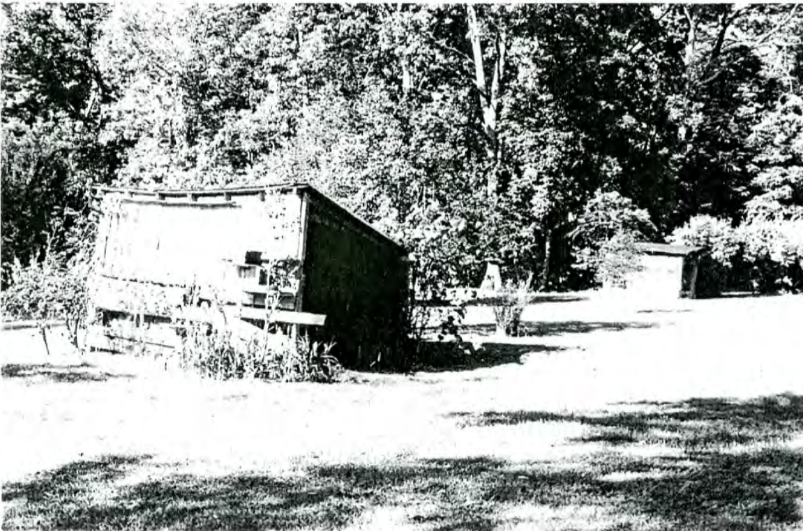
Plate 78: Jamison House— looking north toward chicken house, at left foreground, and tool house, at right rear
