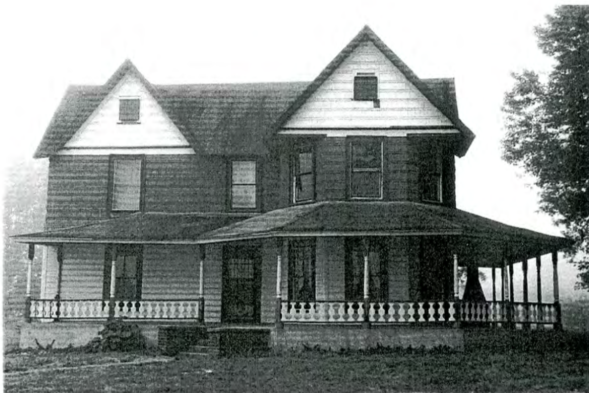
Plate 38: Dr. Solomon E. Greenwood House— northeast front elevation
