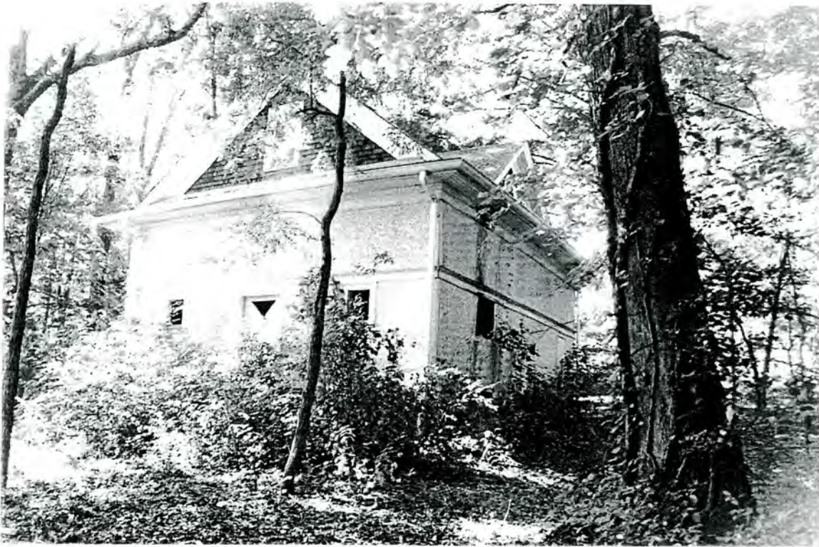
Plate 22: T. Jackson Henderson Estate—barn, north and east elevations
