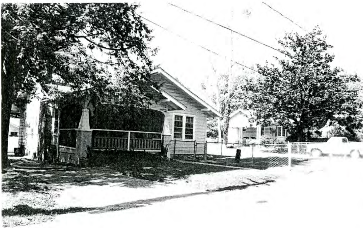
Plate 66: Druid Hills Historic District (Extension)— 1525, at left, and 1527, at right, Ridgewood Boulevard, looking northwest
