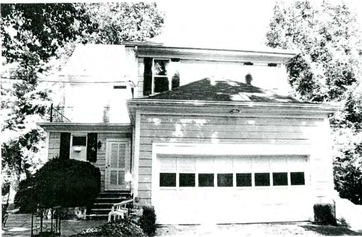
Plate 4: Dr. William Scheppegrell Estate—main house, south rear elevation
