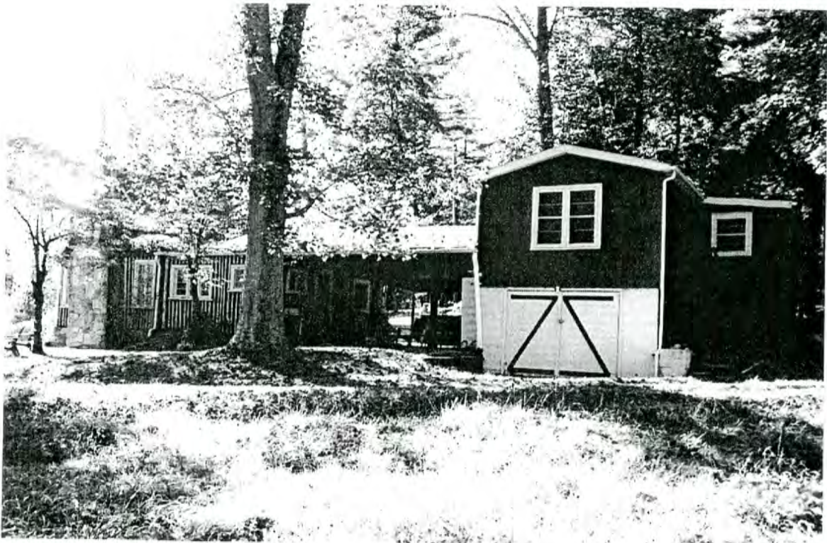
Plate 71: Pearce House— southeast side and northeast rear elevations
