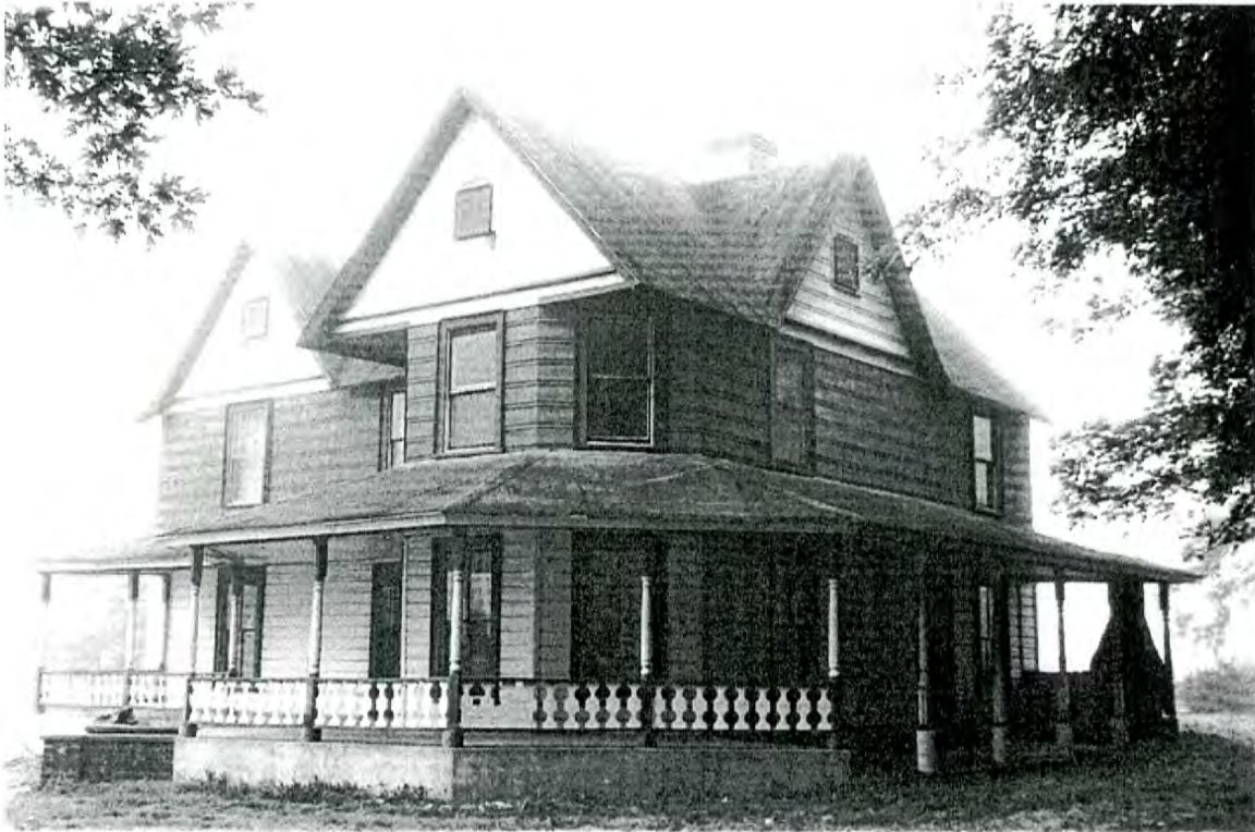
Plate 42: Dr. Solomon E. Greenwood House— northwest side and northeast front elevations
