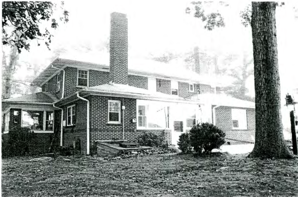
Plate 26: Merchant- Goodson House—main house, southwest rear and northwest side elevations
