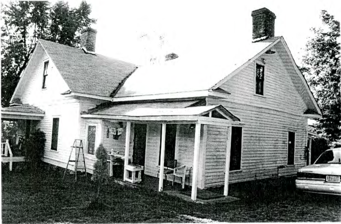
Plate 75: Jamison House—house, northeast rear and southeast side elevations
