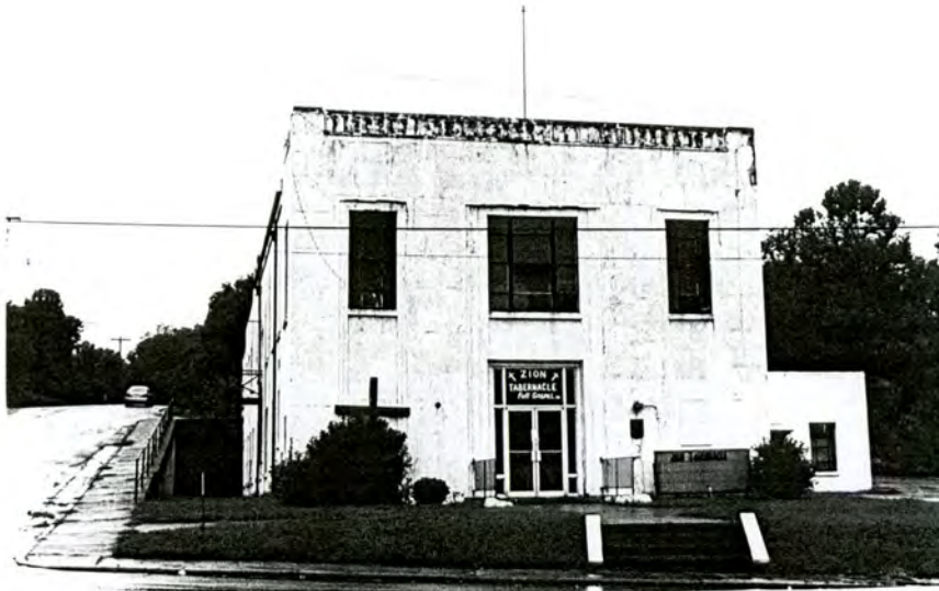
Plate 9. (Former) Leaksville Township Municipal Building (No. 2), Looking Southwest from Boone Road.
