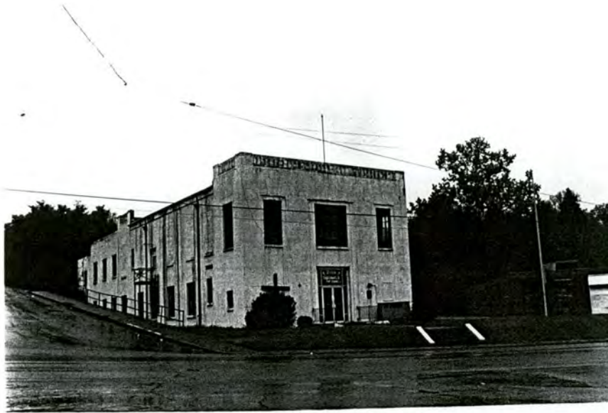
Plate 8. (Former) Leaksville Township Municipal Building (No. 2), Looking West from Boone Road.
