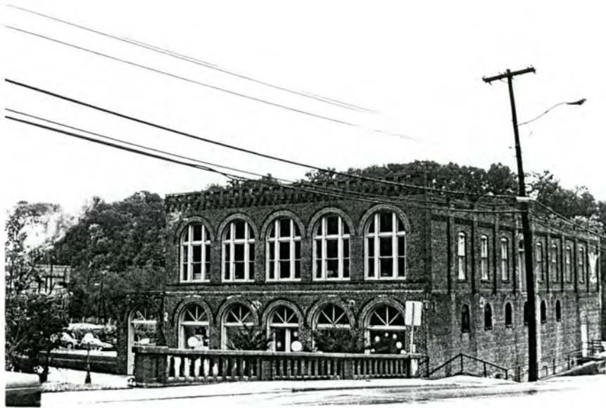
Plate 3. Spray Industrial Historic District, Spray Mercantile Building, Looking Northeast across Church Street.
