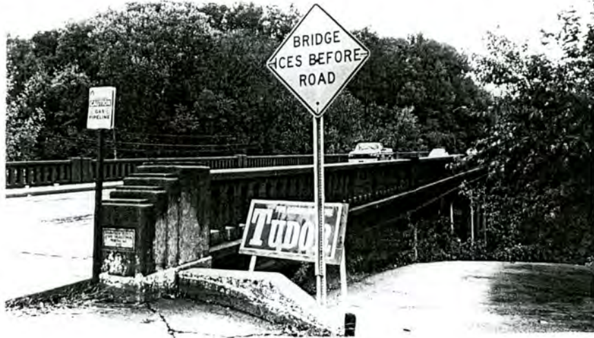
Plate 10. Bridge No. 75, Looking East from Boone Road.
