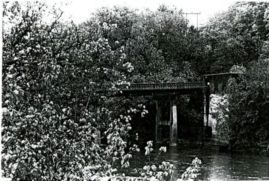
Plate 11. Bridge No. 75 and Pump House (No. 8), Looking Northeast across the Smith River.
