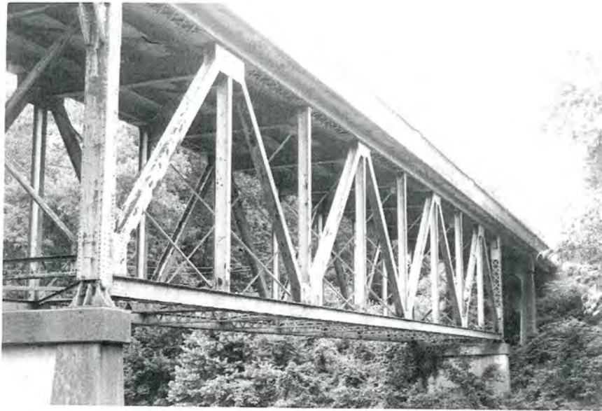
Plate 17. Bridge No. 434, Warren Truss, Looking Northeast.
