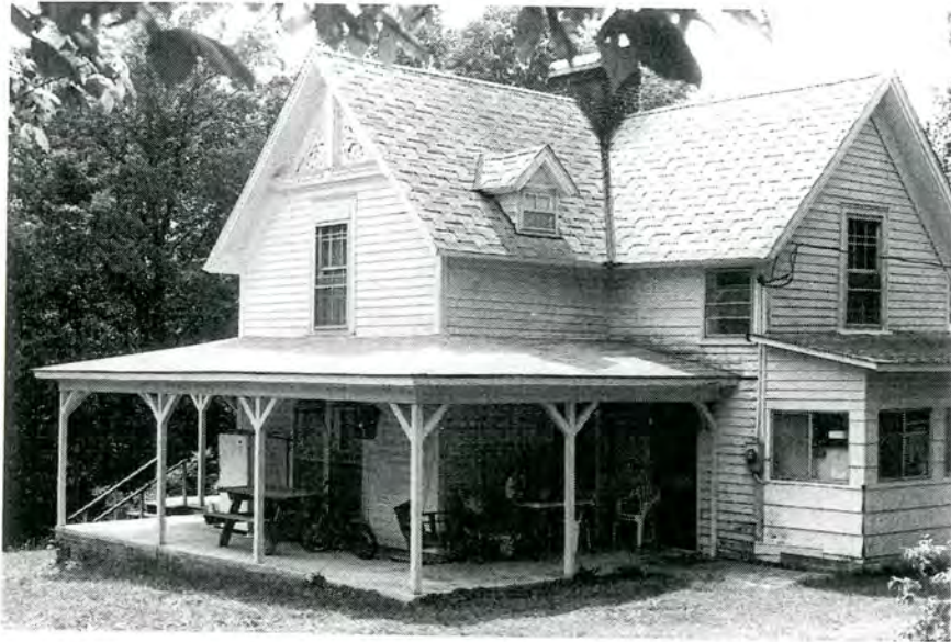
Plate 5. Mill Supervisor's House No. 1, South Elevation, Looking Northwest.
