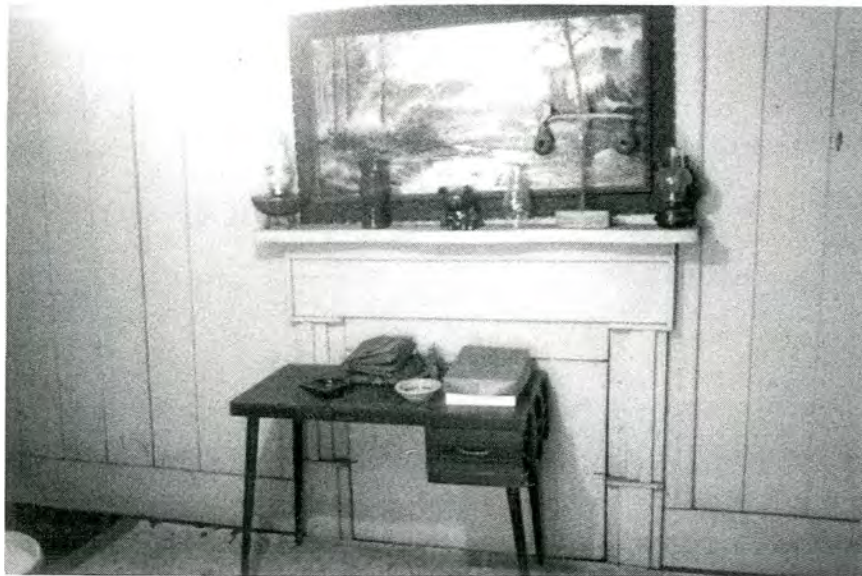
Plate 10. Mill Supervisor's House No. 1, Bedroom Mantel.
