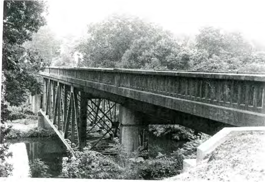
Plate 19. Bridge No. 434, Looking East.
