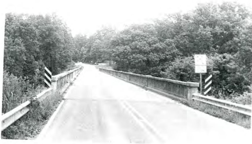
Plate 15. Bridge No. 434, Looking East.
