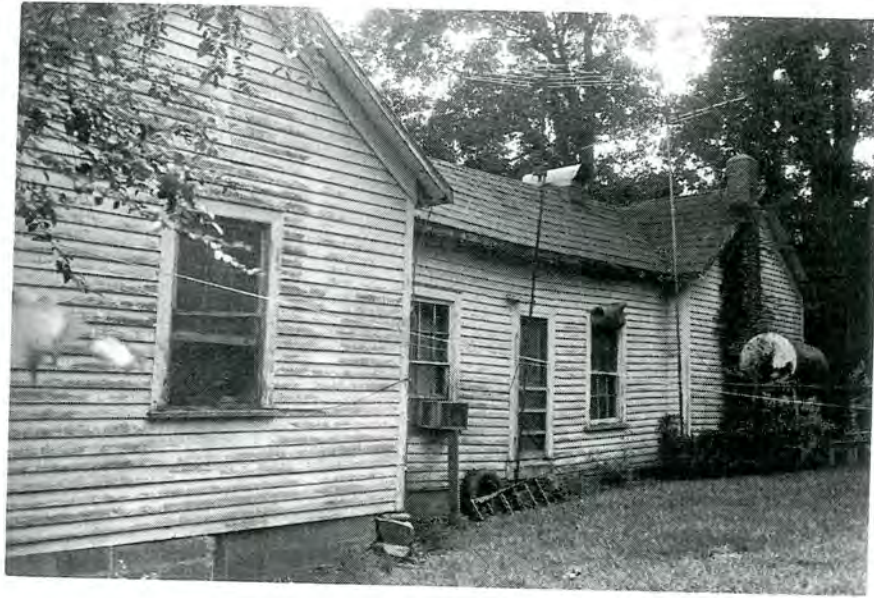
Plate 13. Mill Supervisor's House No. 2, North Elevation, Looking Southwest.
