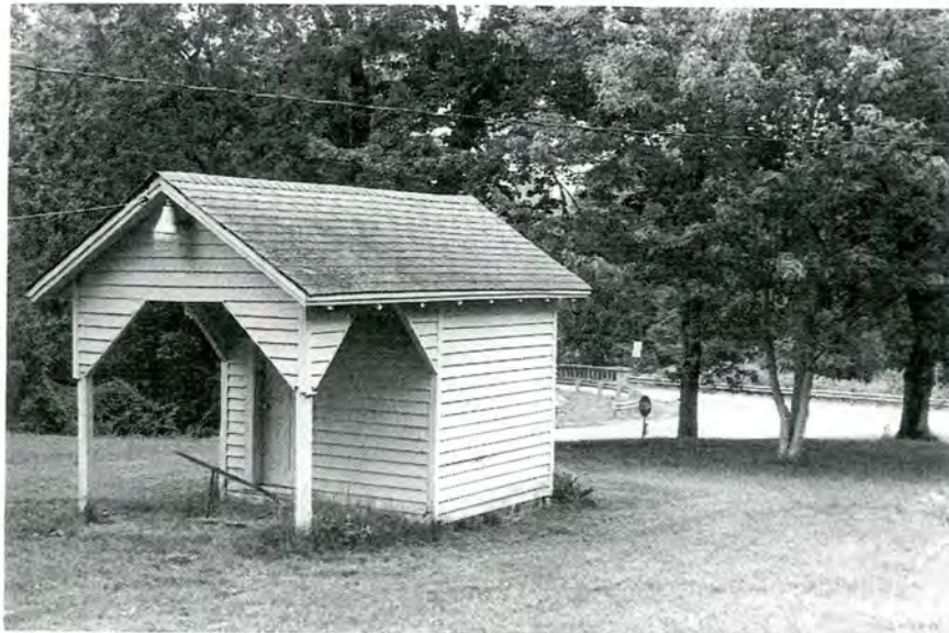
Plate 6. Mill Supervisor's House No. 1, Well House, Looking Northwest.
