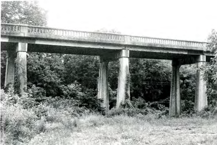
Plate 20. Bridge No. 434, Concrete Post-and-Lintel Supports, Looking North.
