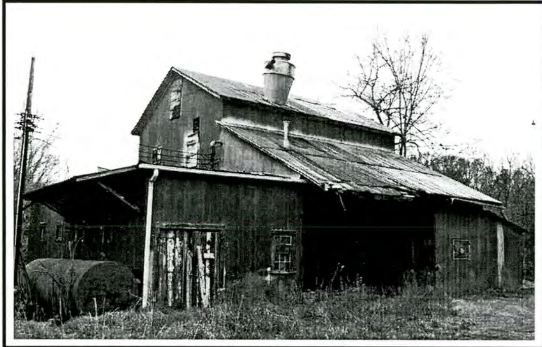
Figure 7 - Hub Mill, SE elevation
