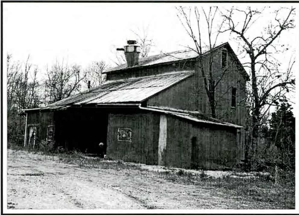
Figure 5 - Hub Mill, NE elevation
