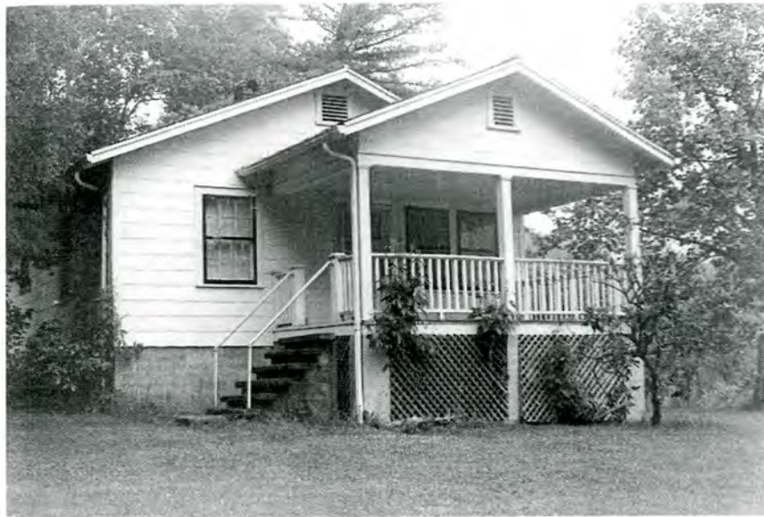
Plate 8. Thorpe Dam Complex, Cottage, Looking East.
