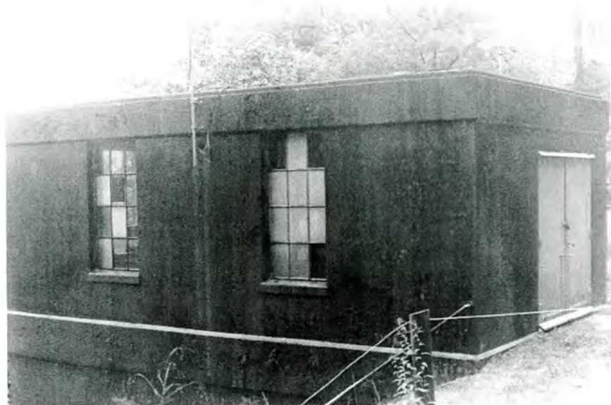
Plate 5. Thorpe Dam Complex, Gate Building No. 1, Looking Southwest.
