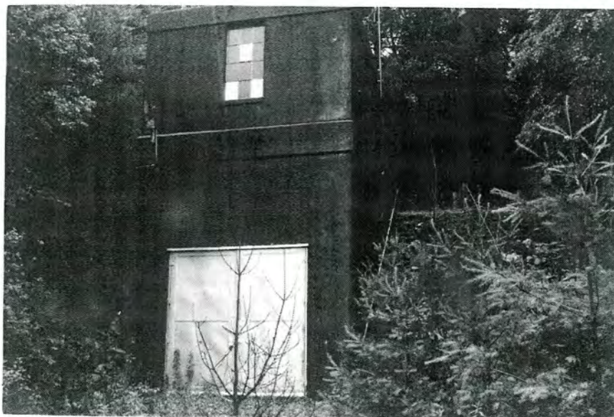
Plate 6. Thorpe Dam Complex, Gate Building No. 1, Looking North.
