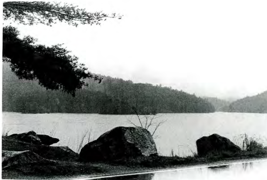
Plate 12. Thorpe Dam Complex, Thorpe Lake, Looking South.
