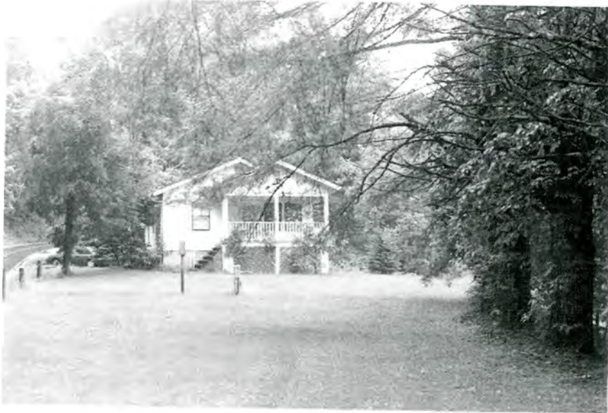
Plate 7. Thorpe Dam Complex, Cottage, Looking East.
