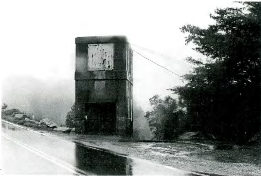
Plate 10. Thorpe Dam Complex, Gate Building No. 2, Looking North.
