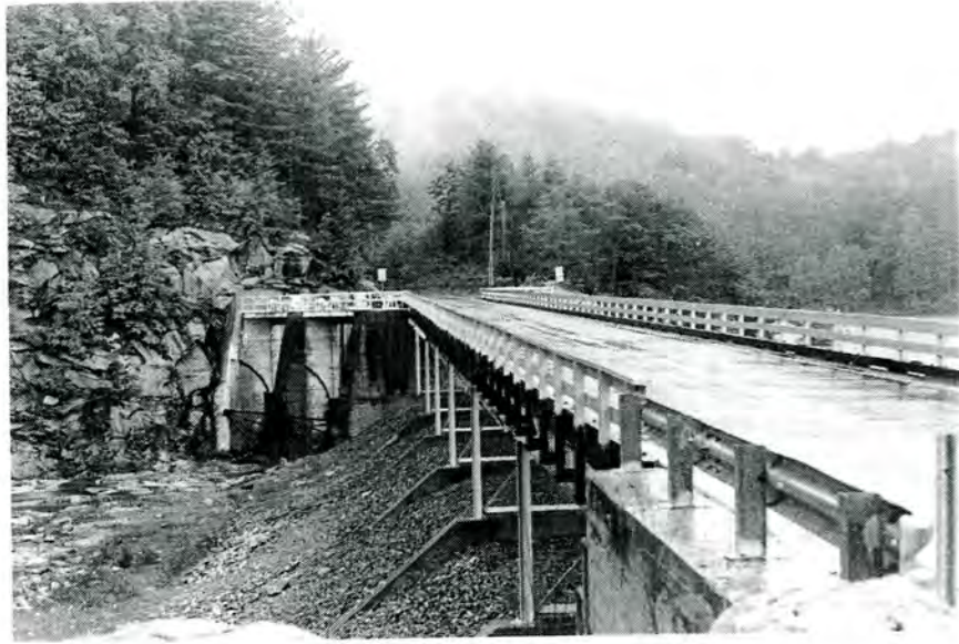
Plate 1. Thorpe Dam Complex, Bridge No. 193 and Dam, Looking East.
