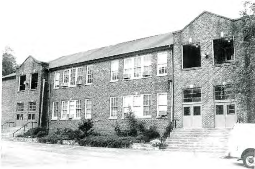
Plate 15. (Former) Marshall High School, Front Facade.
