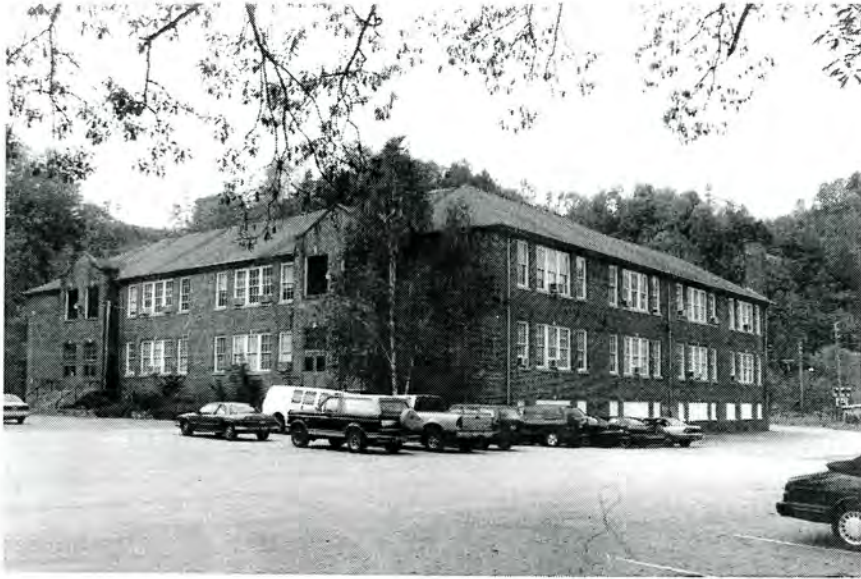
Plate 13. (Former) Marshall High School on Blennerhassett Island, Looking West.
