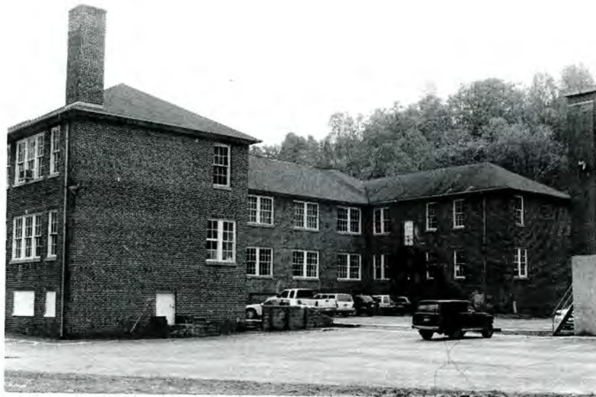
Plate 16. (Former) Marshall High School, Rear Elevation.
