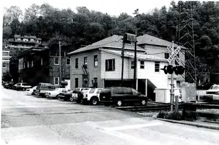
Plate 4. Marshall Commercial Historic District, Looking Northeast towards the Sheriff's Department/Jail.
