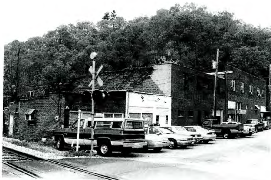
Plate 6. Marshall Commercial Historic District, Looking Northwest along Bridge Street, West Side.
