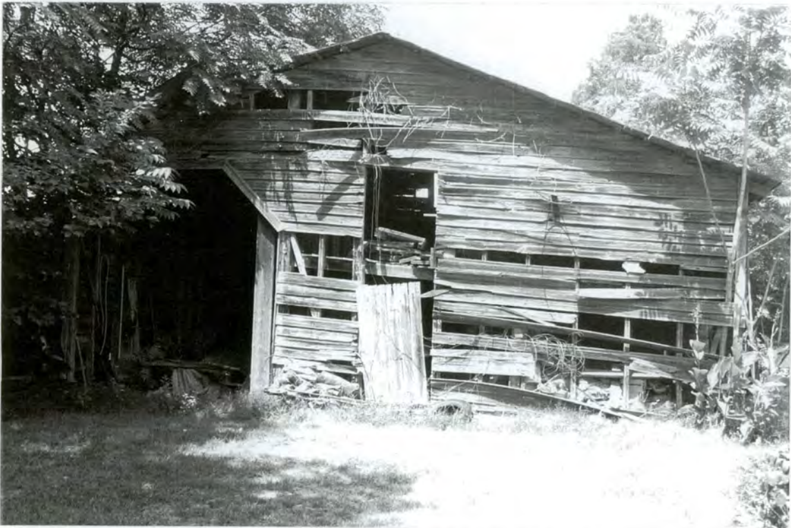
Plate 17 House and Outbuildings (#1) - South front elevation of barn
