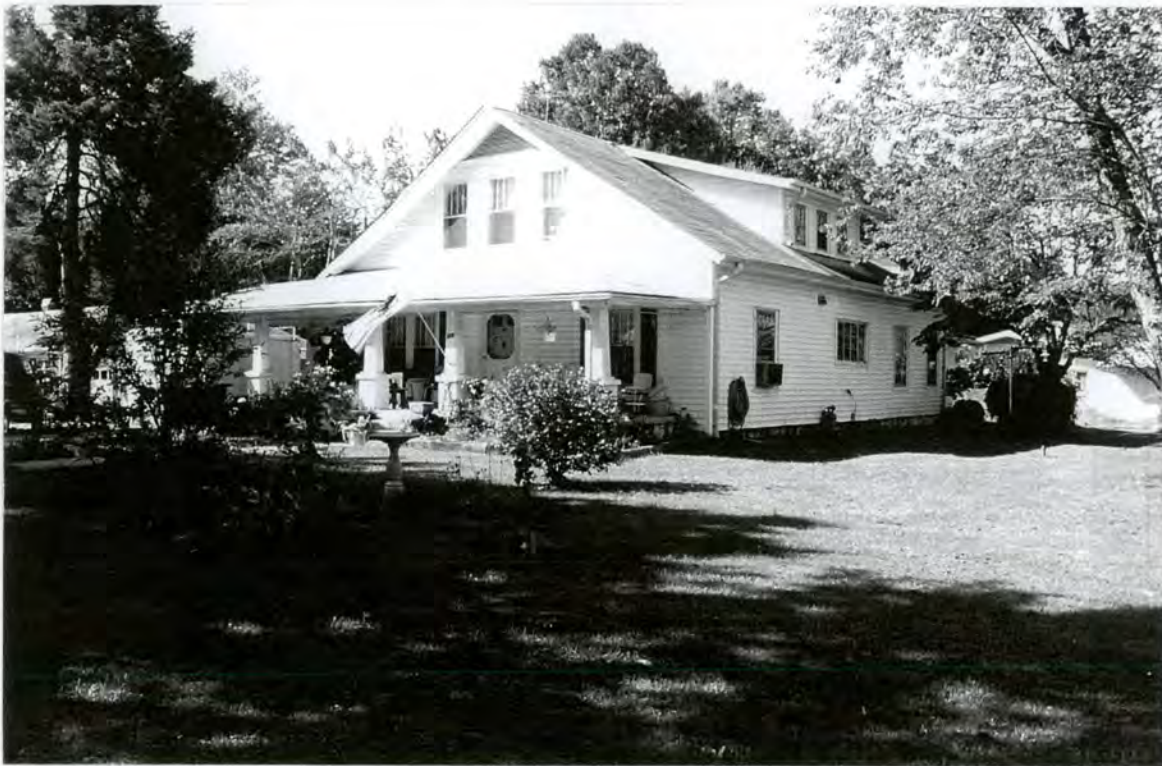
Plate 35 Bungalow (#18) - East front and north side elevations
