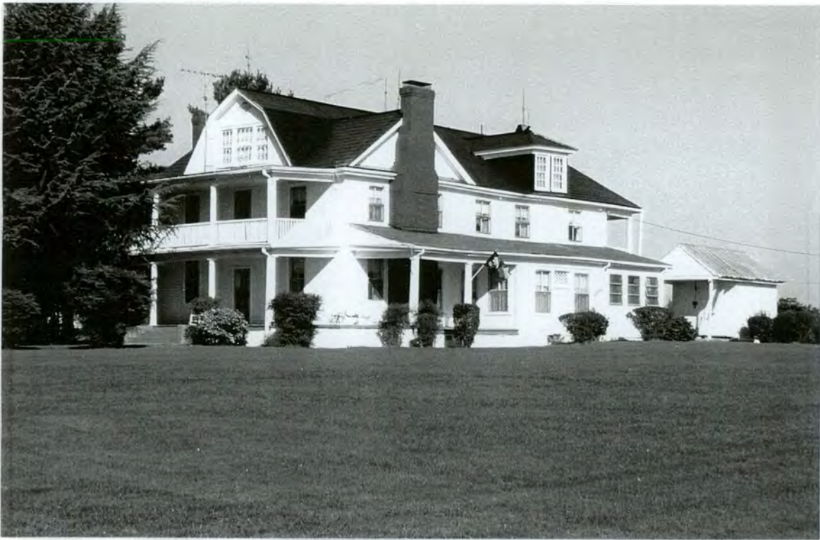
Plate 4 Campbell-Gray Farm (#8) - South and west elevations of house
