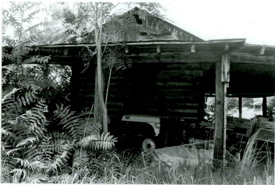
Plate 18 House and Outbuildings (#1) - West elevation of tobacco barn
