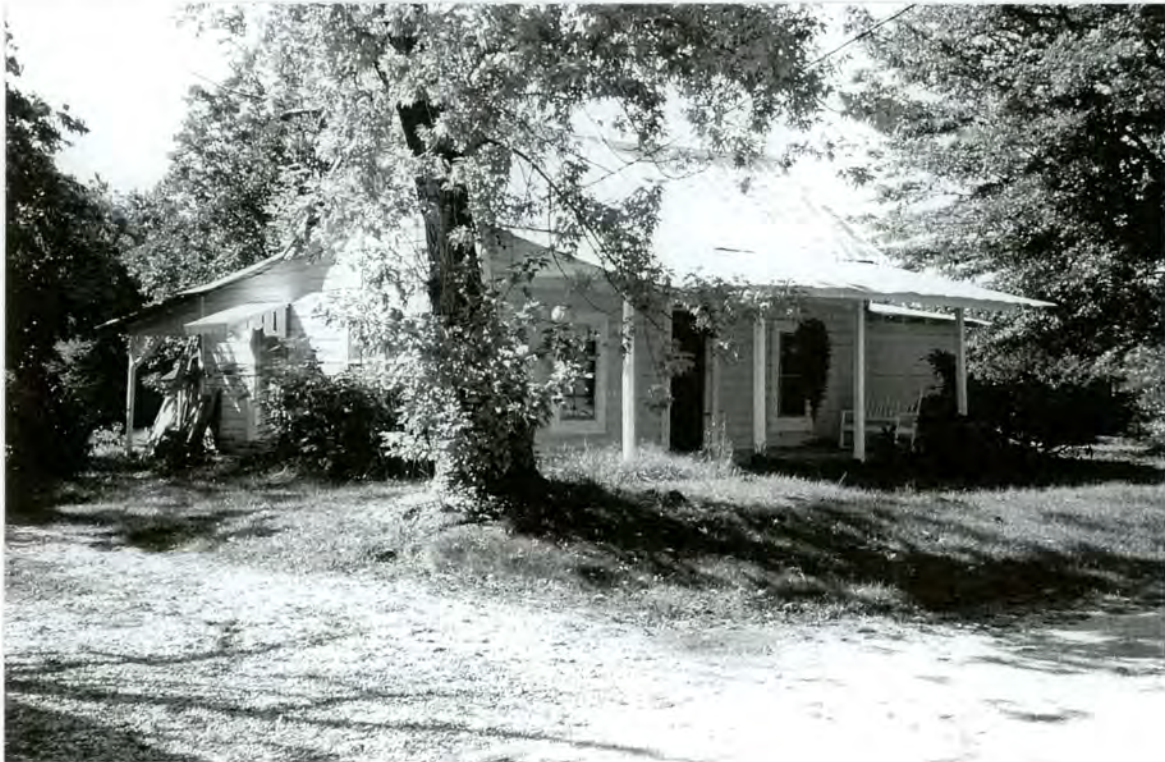
Plate 24 House (#5) - North front and east side elevations
