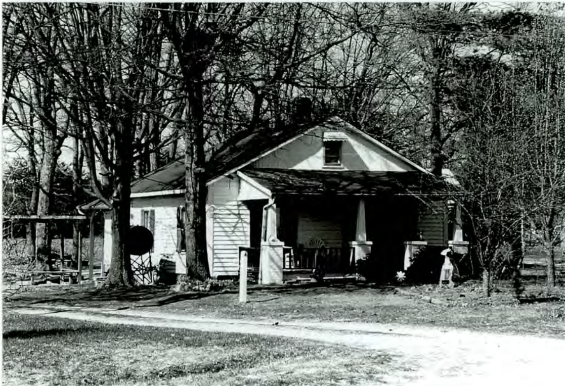
Plate 61 House (#43) - East front and south side elevations
