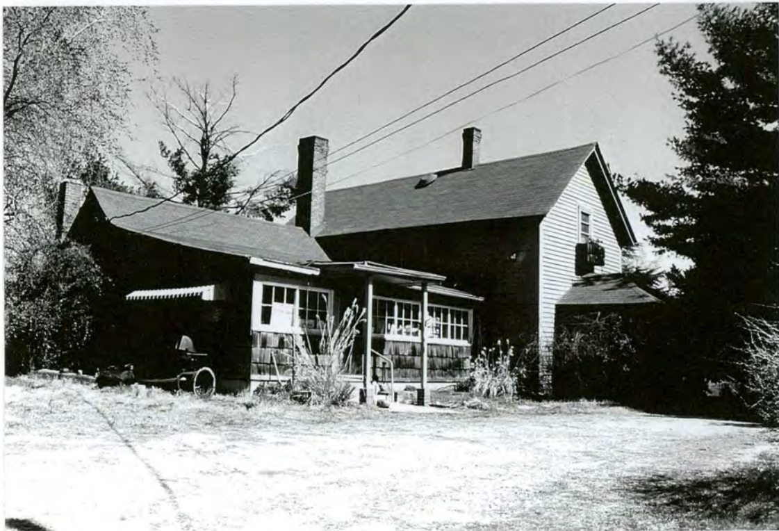
Plate 66 House (#48) - South side and west rear elevations
