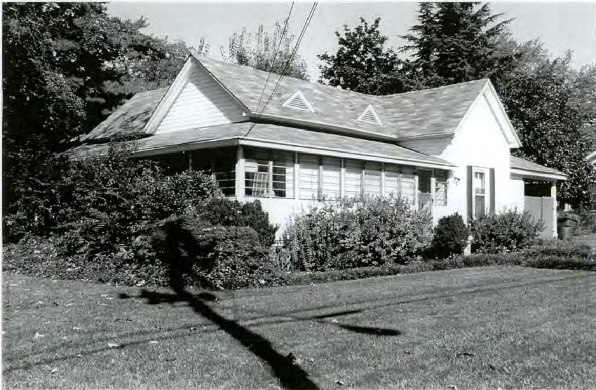
Plate 38 House (#20) - East front and south side elevations
