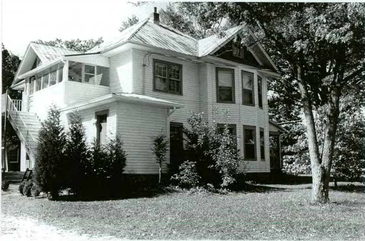
Plate 44 House (#25) - North side and east rear elevations
