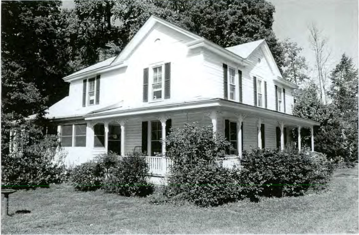
Plate 12 Dr. McCracken House (#30) - East front and south side elevations of house
