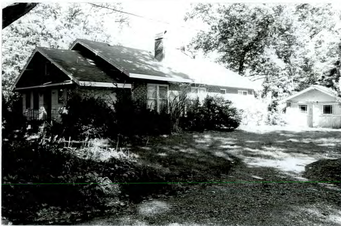
Plate 40 Bungalow (#22) - South front and east side elevations; garage to right
