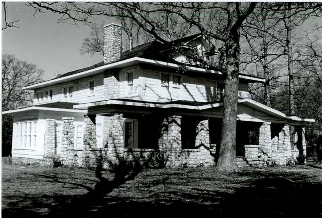
Plate 6 Roy Edgerton House (#42) - East front and south side elevations
