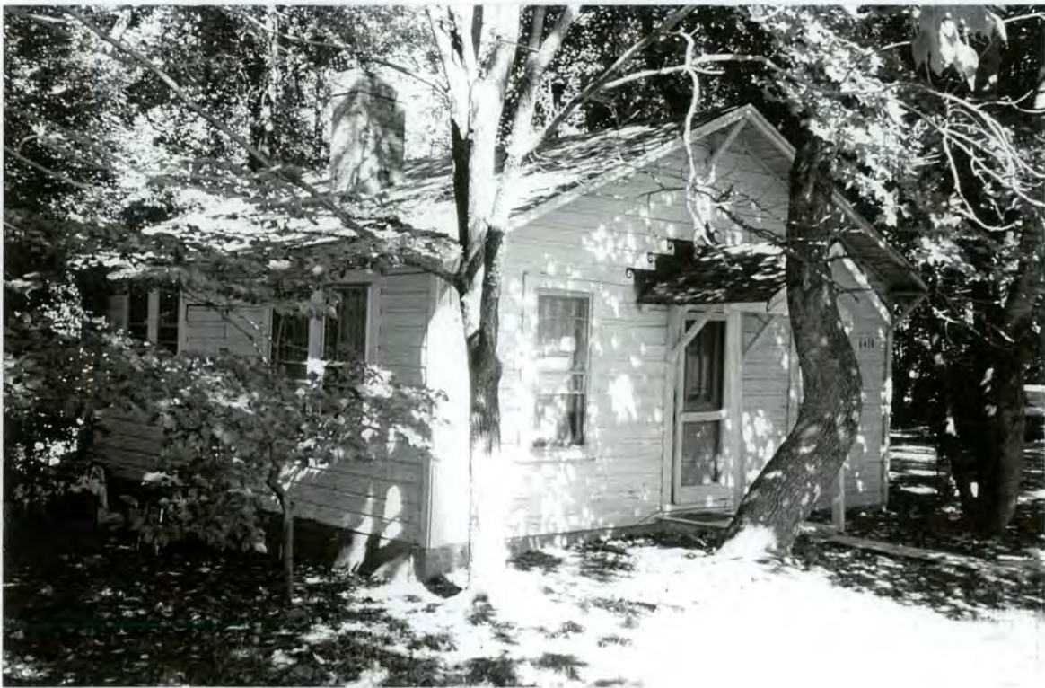
Plate 34 House (#13) - South front and west side elevations
