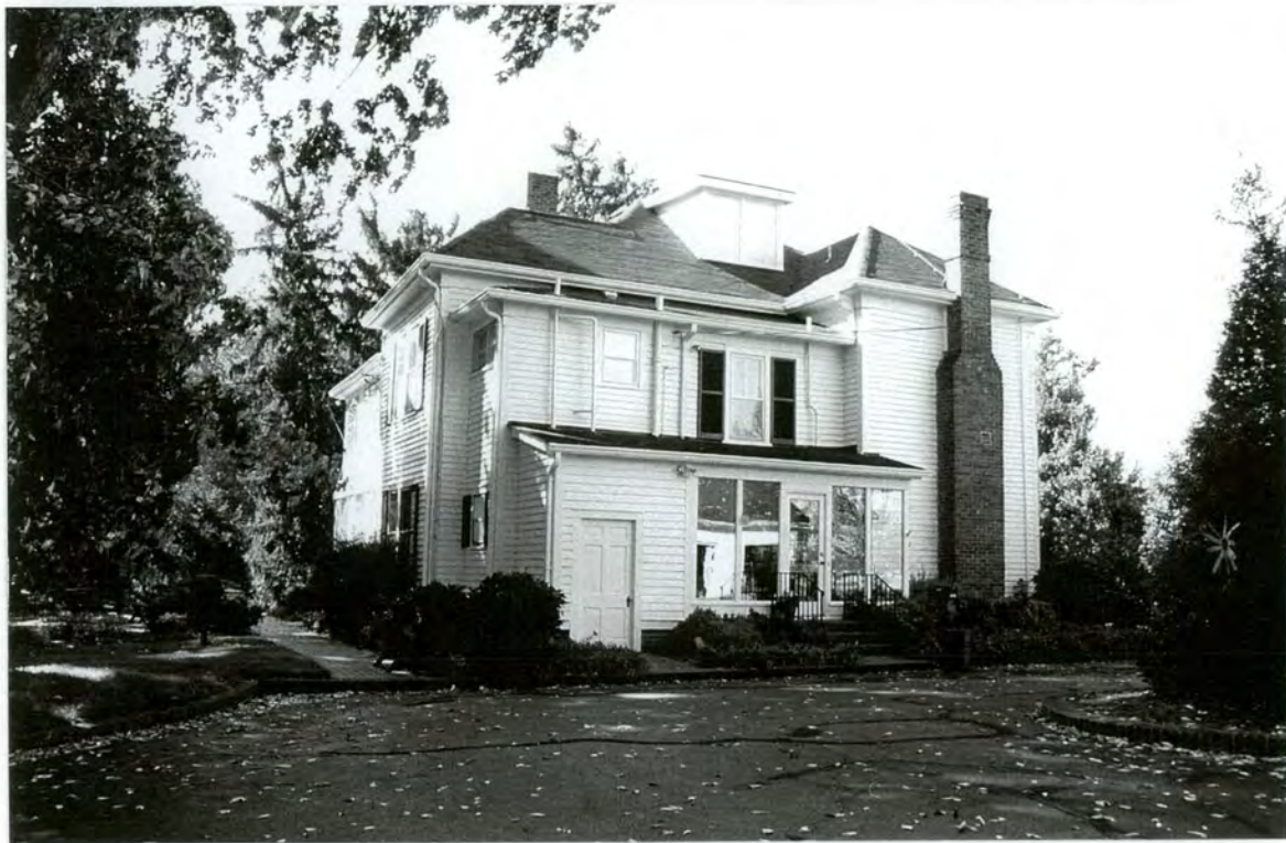
Plate 10 Coble Farm (#15) - North rear and east side elevations of house
