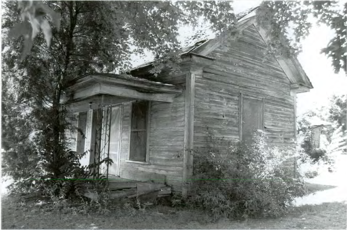
Plate 16 House and Outbuildings (#1) - South front and east side elevations of house
