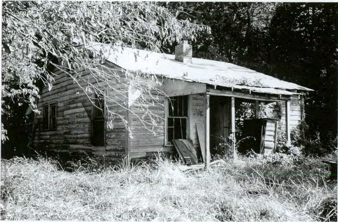
Plate 26 House and Outbuildings (#7) - South front and west side elevations of house
