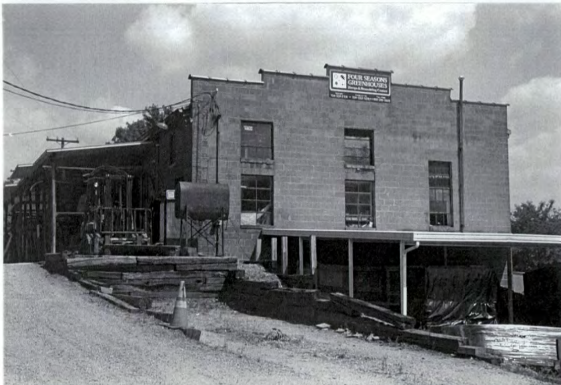
Plate 30: Catawba Transit Company Garage – northeast and southwest elevations
