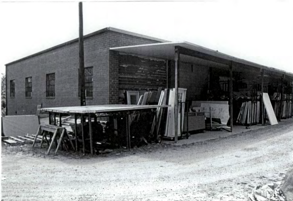
Plate 32: Catawba Transit Company Garage – southwest and northwest elevations
