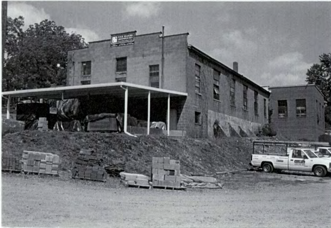
Plate 29: Catawba Transit Company Garage – southeast and northeast elevations
