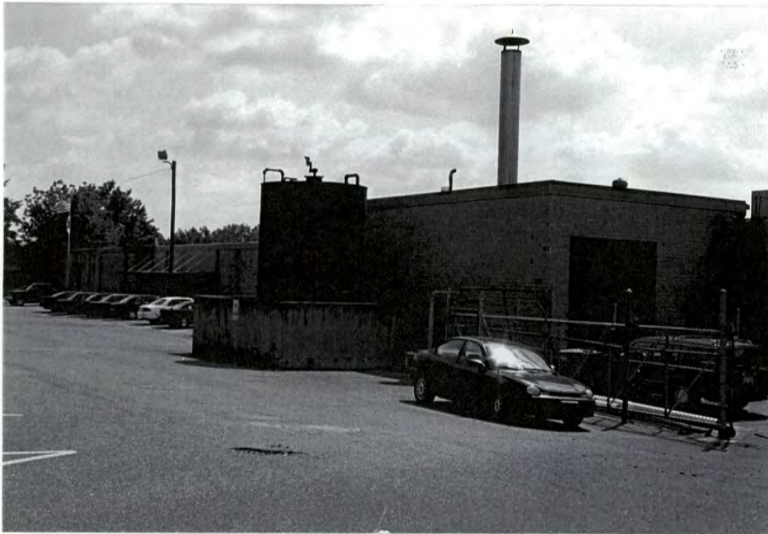
Plate 27: Whisnant Hosiery Mill – southwest rear and northwest side elevations of modern block
