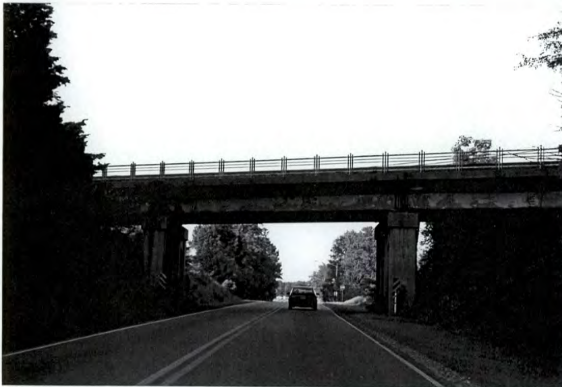
Plate 18: Railroad bridge over US 70, Conover, looking east (outside of APE)
