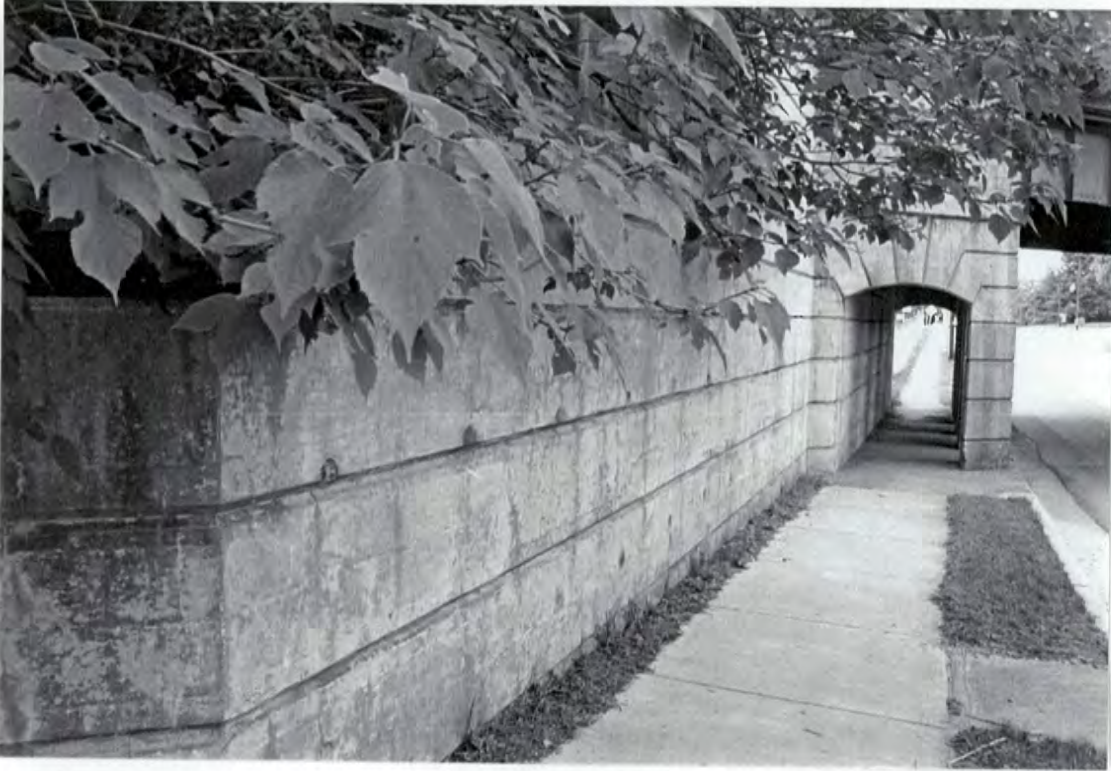
Plate 15: Highland Avenue Southern Railway Bridge – southwest retaining wall looking north
