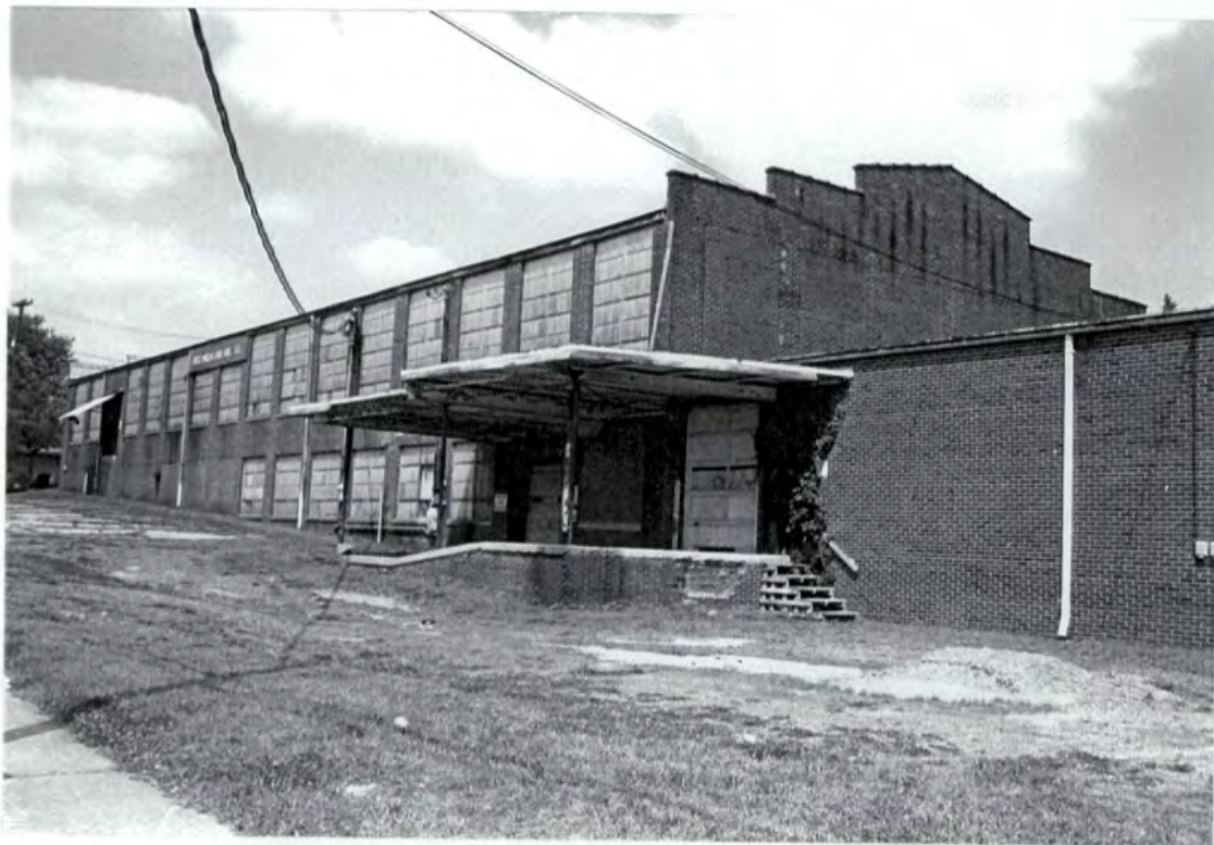
Plate 4: Hollar Hosiery Mills Building - south side and east rear elevation of ca. 1930 block; late 1960s hyphen at right
