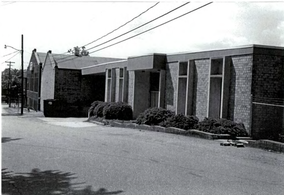
Plate 28: Whisnant Hosiery Mill – northeast front elevation of modern block at right, 1920s block at left center, and 1930s block at far left
