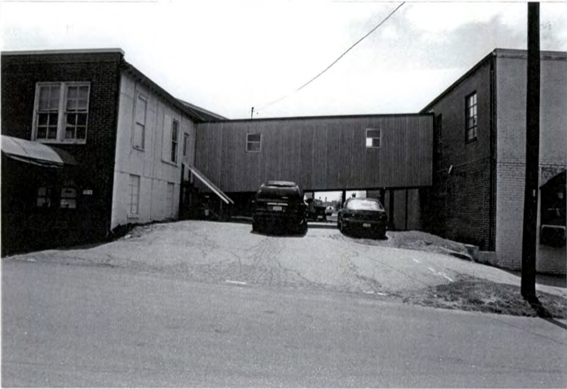
Plate 38: Hickory Hosiery Mill – enclosed walkway connector looking southeast
