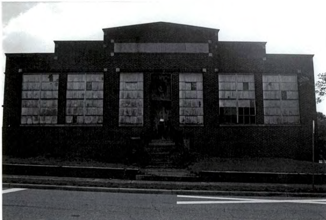
Plate 2: Hollar Hosiery Mills Building – west front elevation of ca. 1930 block
