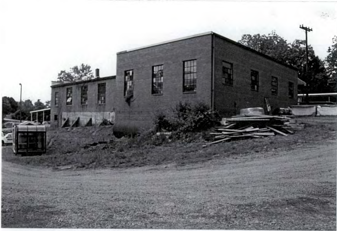
Plate 33: Catawba Transit Company Garage – northwest and northeast elevations
