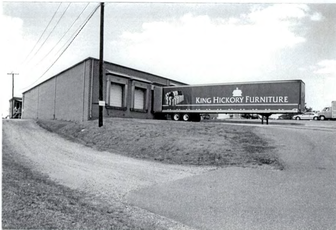
Plate 41: Hickory Hosiery Mill – shipping facility and loading docks looking south
