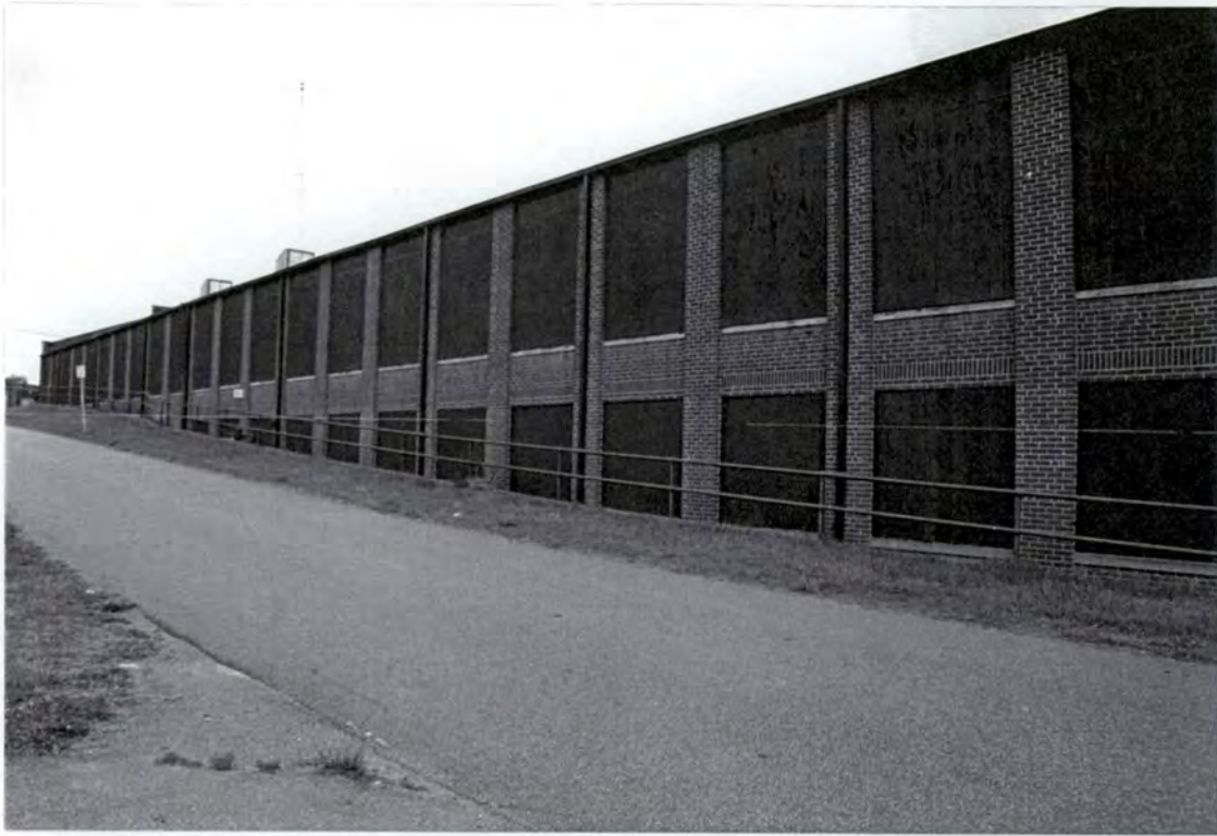
Plate 25: Whisnant Hosiery Mill – south elevation of 1930s block
