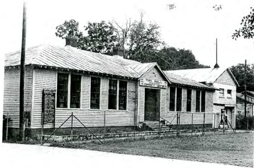
Plate 2. Princeville Historic District, Princeville Town Hall/School, Looking Southwest.
