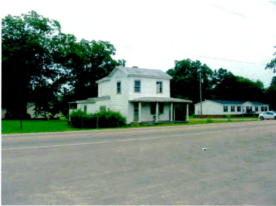
Plate 20. Bridgers House, 225 Main Street, Facade and Side (North) Elevation, Looking Southeast.
