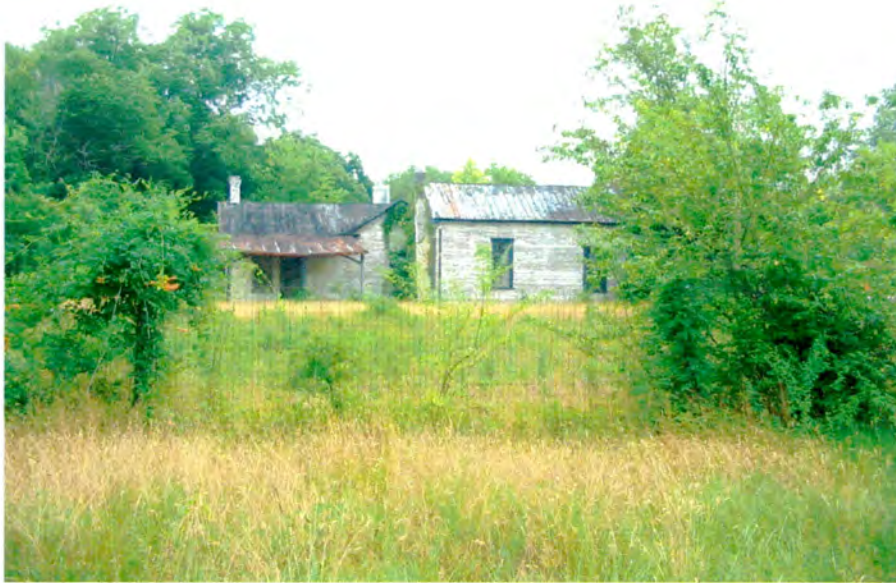
Plate 12. Abraham Wooten House, Side (West) Elevation, Looking East from Mutual Boulevard.
