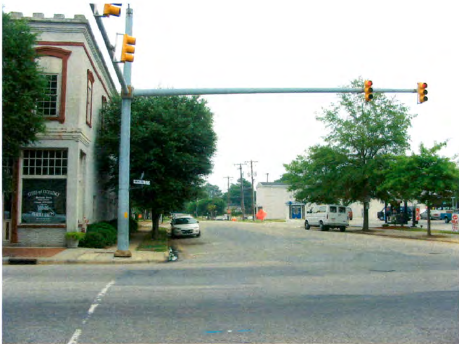
Plate 2. Tarboro Historic District, Looking East Along Granville Street from Main Street (201 Main Street on Left).
