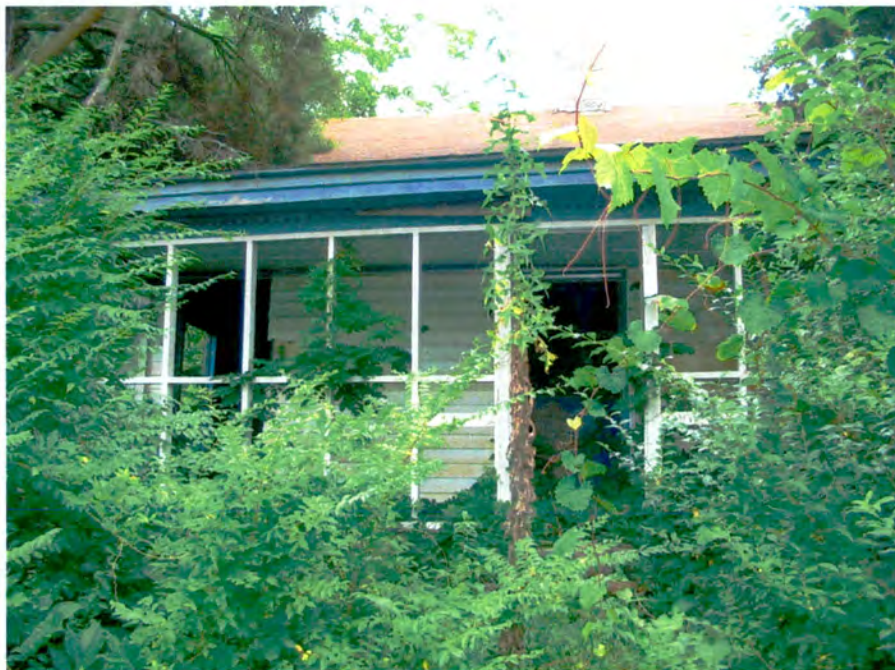
Plate 19. House, 101 Mutual Boulevard, Facade and Porch (Southwest Elevation), Looking Northwest.
