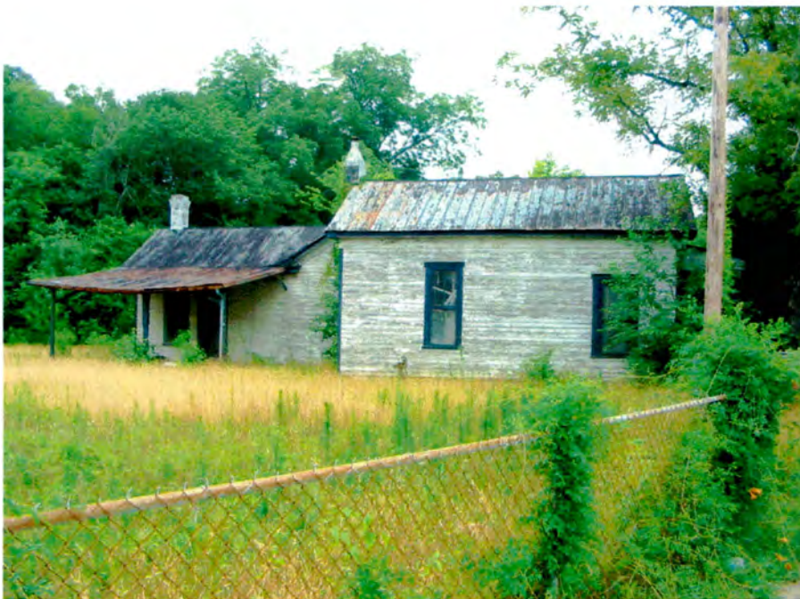
Plate 13. Abraham Wooten House, Side (West) Elevation, Looking Northeast from Mutual Boulevard.
