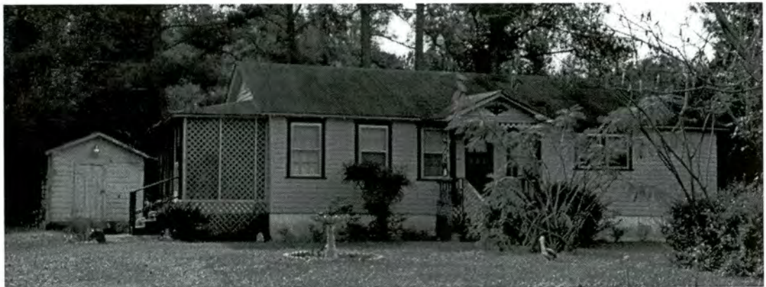
Property 38. House, circa 1930, 128 Peterson Hill Road
