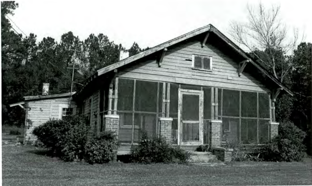
Property 36. House, Circa 1925, 131 Peterson Hill Road
