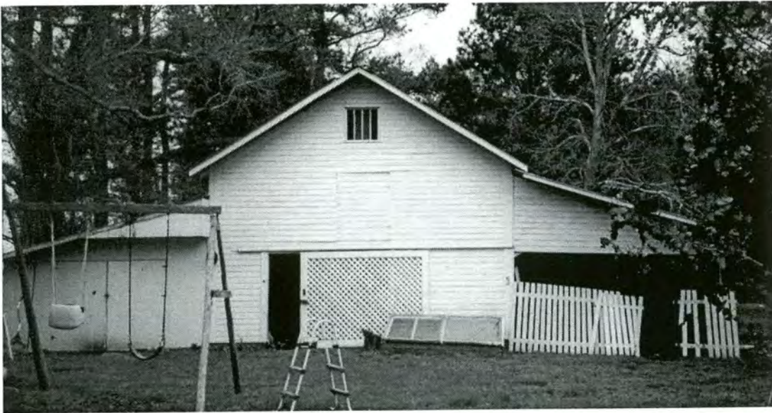
Barn north of Tate E. Bowen House (Property 85) South Elevation
