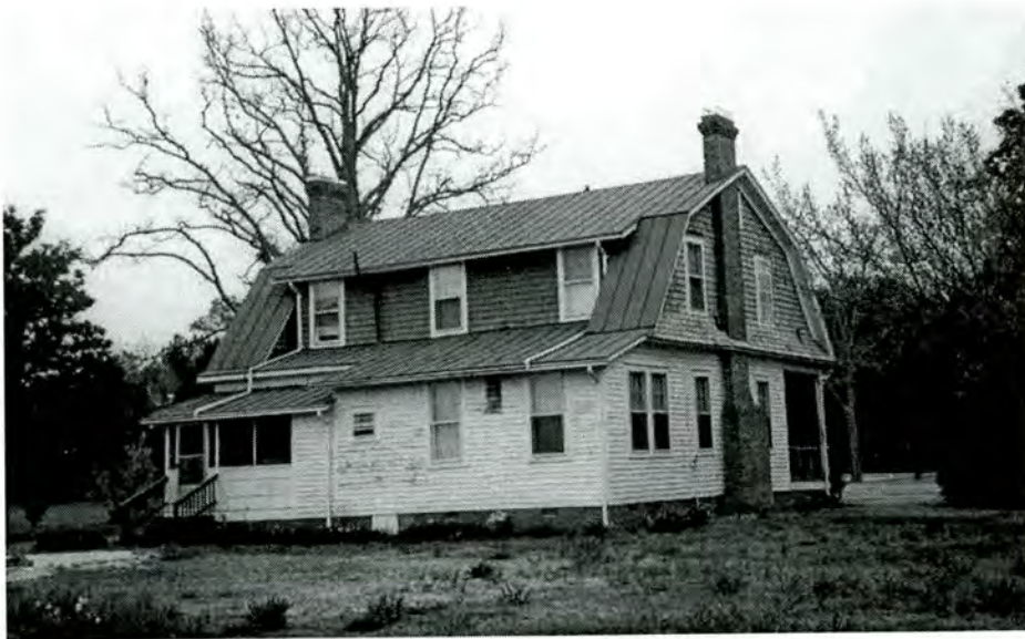
Stuart Vann Bowen House (Property 80) North and West Elevations
