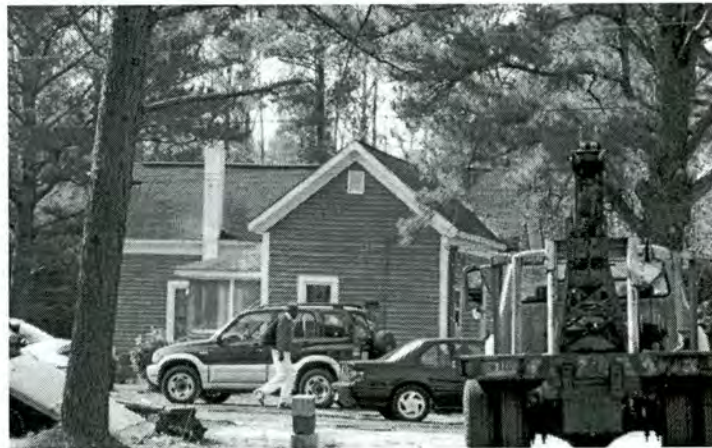
Property 54. House, circa 1900, 705 SR 1345 (facing RR tracks)
