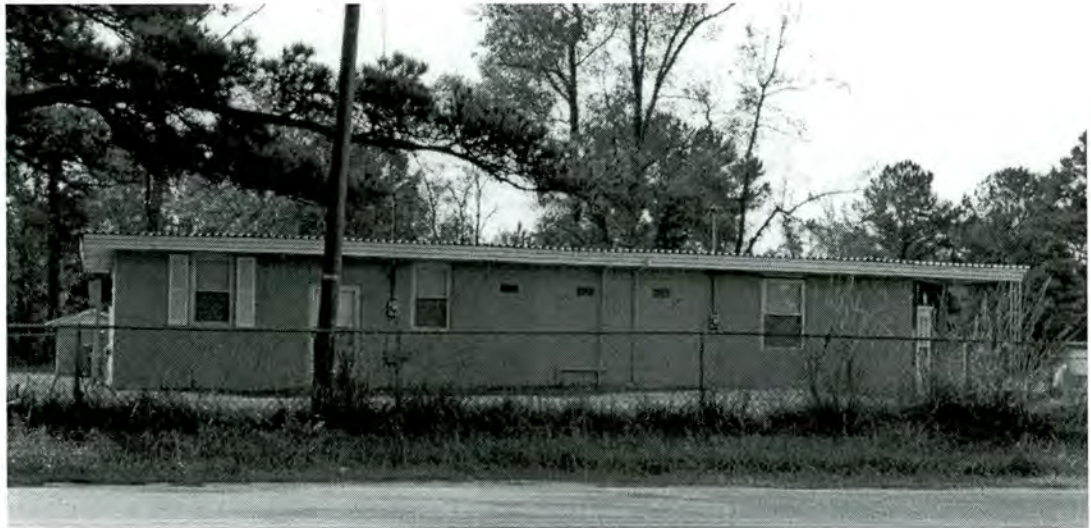
Property 1. Motel Complex, circa 1950, SE corner SR 1509 and NC 53
