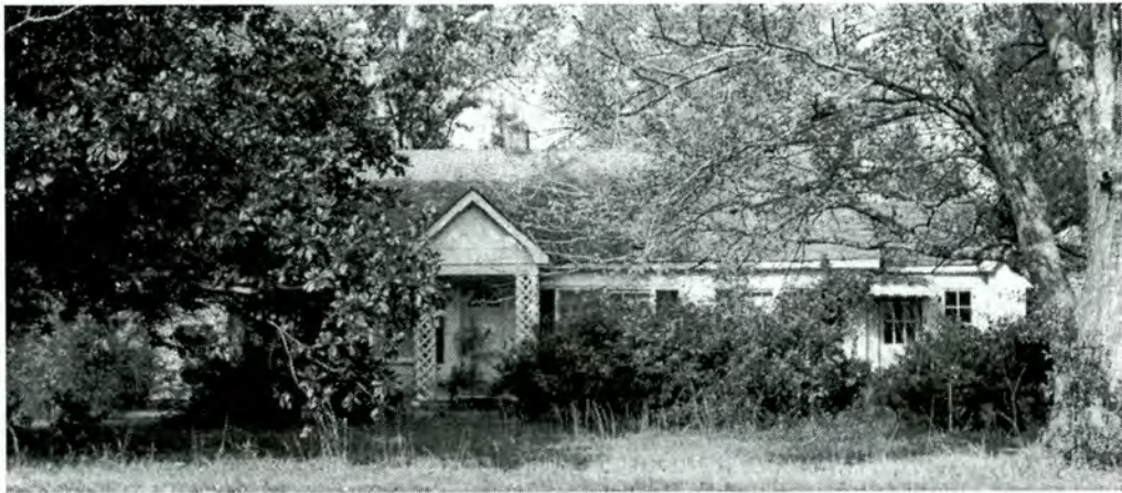
Property 2. House, circa 1940, W side NC 53, opposite SR 1509
