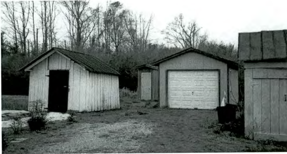
Smokehouse and Sheds north of Stuart Vann Bowen House (Property 80)
