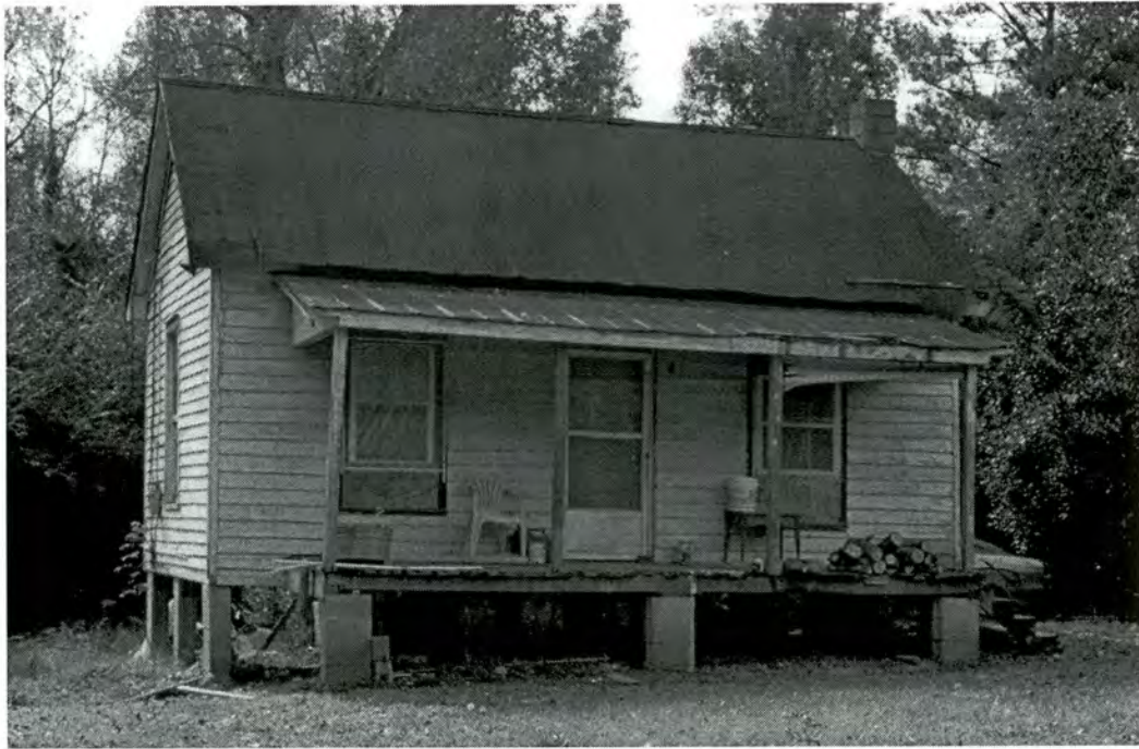
Property 37. House, circa 1920, Peterson Hill Road
