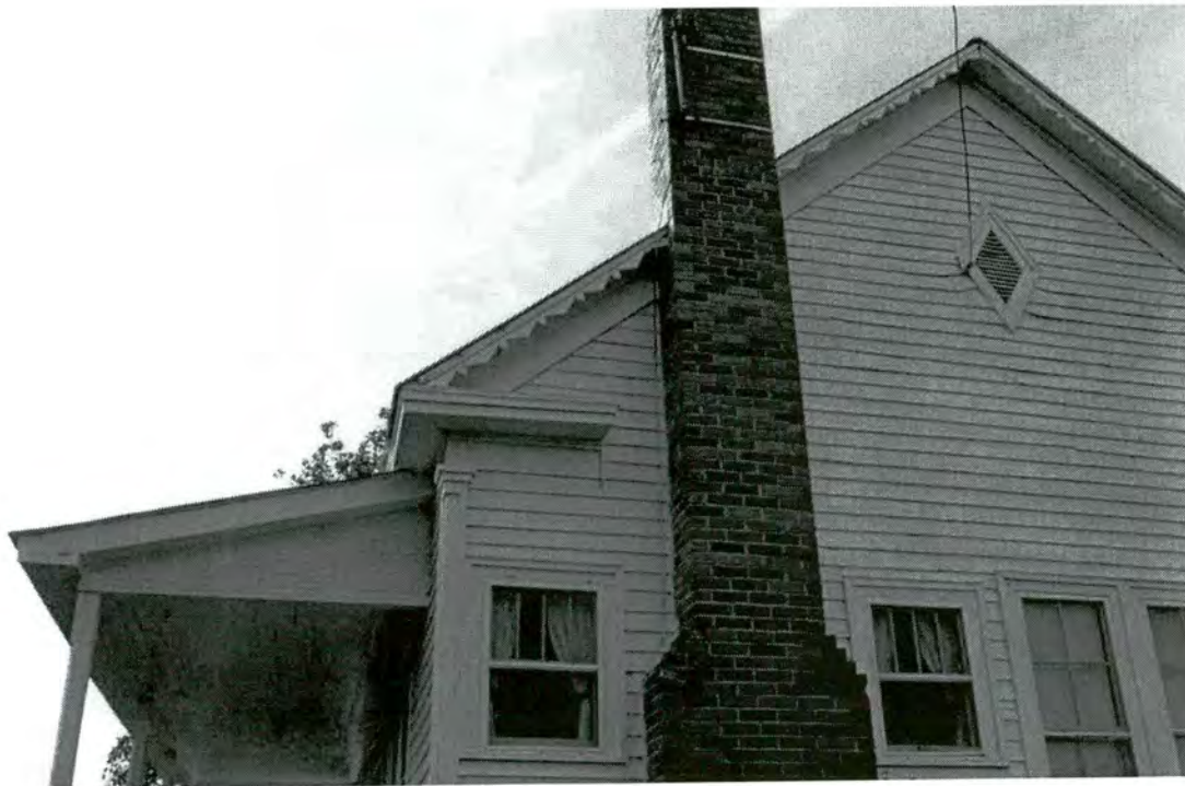
Douglas Towles Bowden House (Property 71) Detail of Bargeboard and Greek Revival Corner Pilaster
