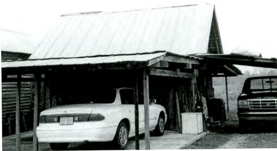
Corn Crib west of John Wright Bowen House (Property 79) South and East Elevations
