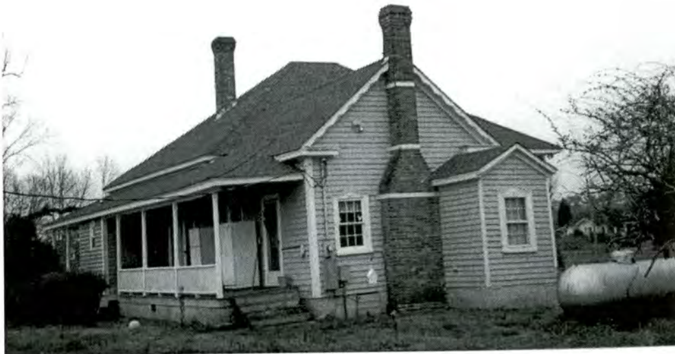
John Wright Bowen House (Property 79) North and East Elevations
