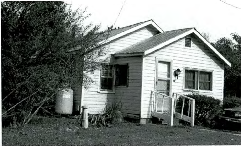
Property 35. House, circa 1930, 65 Peterson Hill Road
