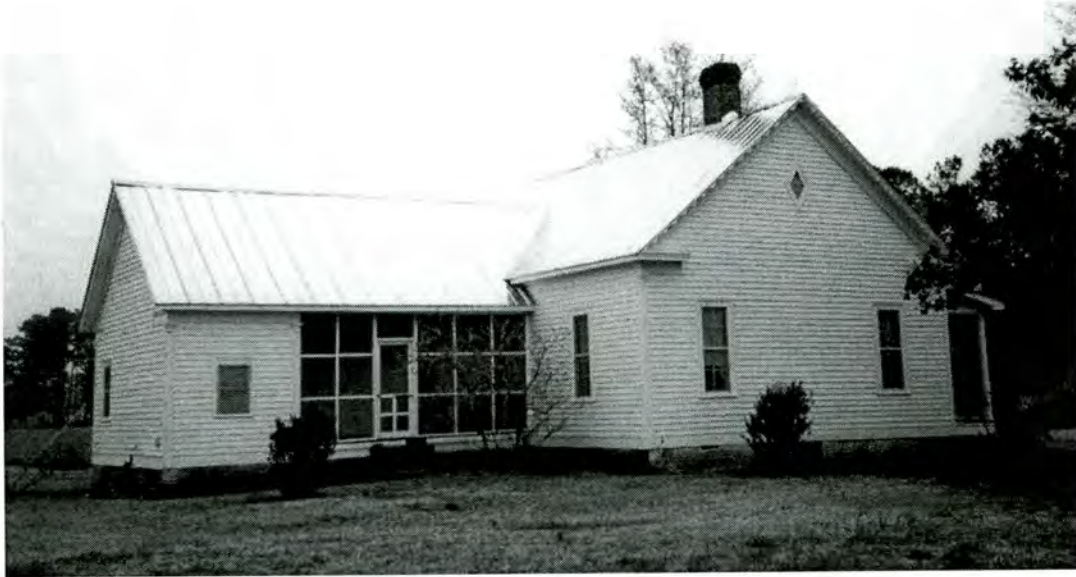
Douglas Towles Bowden House (Property 71) North and West Elevations
