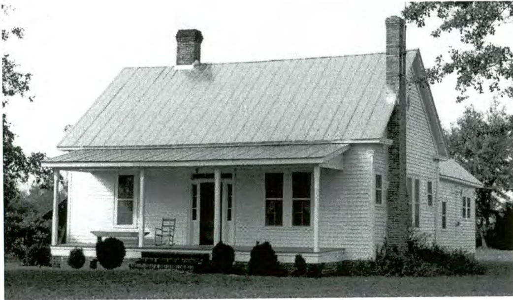
Douglas Towles Bowden House (Property 71) South and East Elevations
