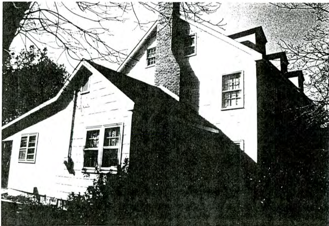
Plate 21: Ralph Potter House (#28)—east front and south side elevations
