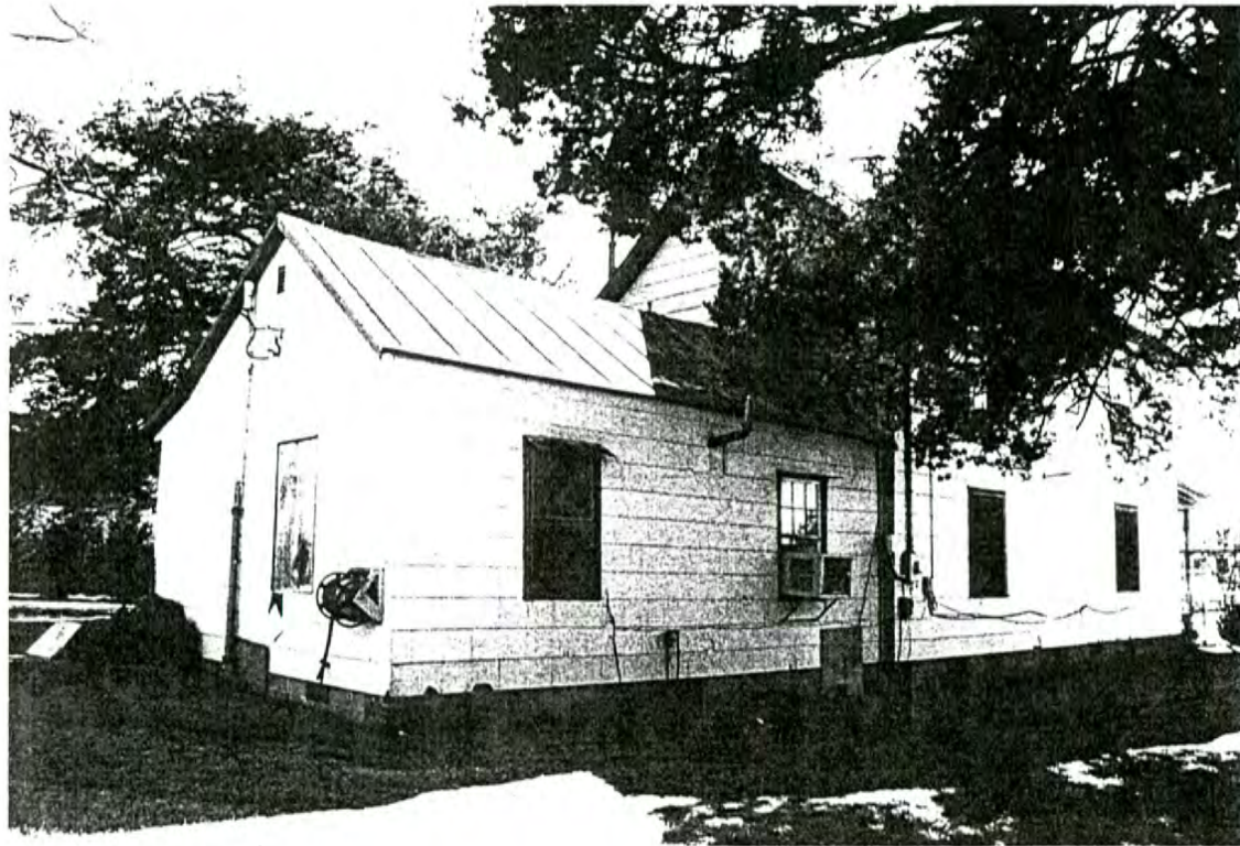
Plate 2: House (#39)— north side and east rear elevations
