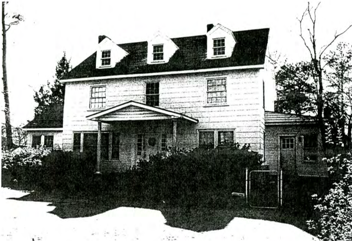
Plate 20: Ralph Potter House (#28)—east front and north side elevations
