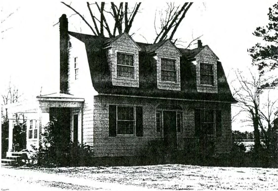
Plate 16: Charles Keener House (#20)—east front and south side elevations
