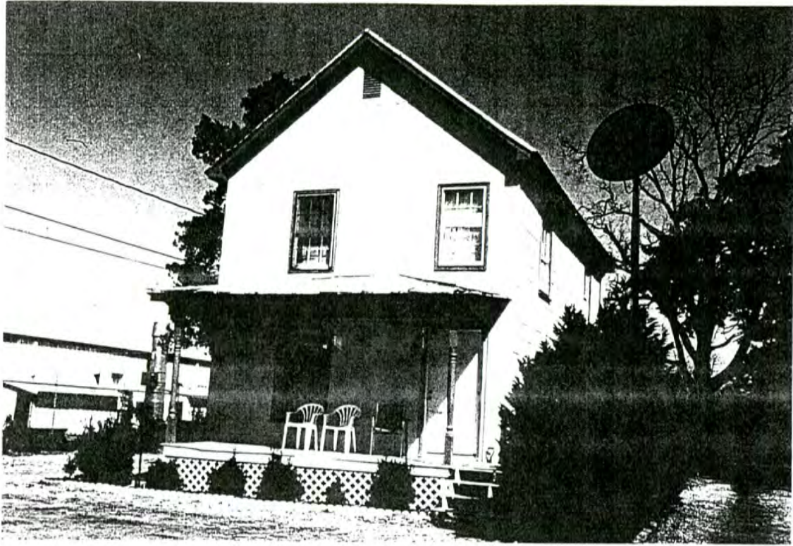
Plate 1: House (#39)— west front and south side elevations
