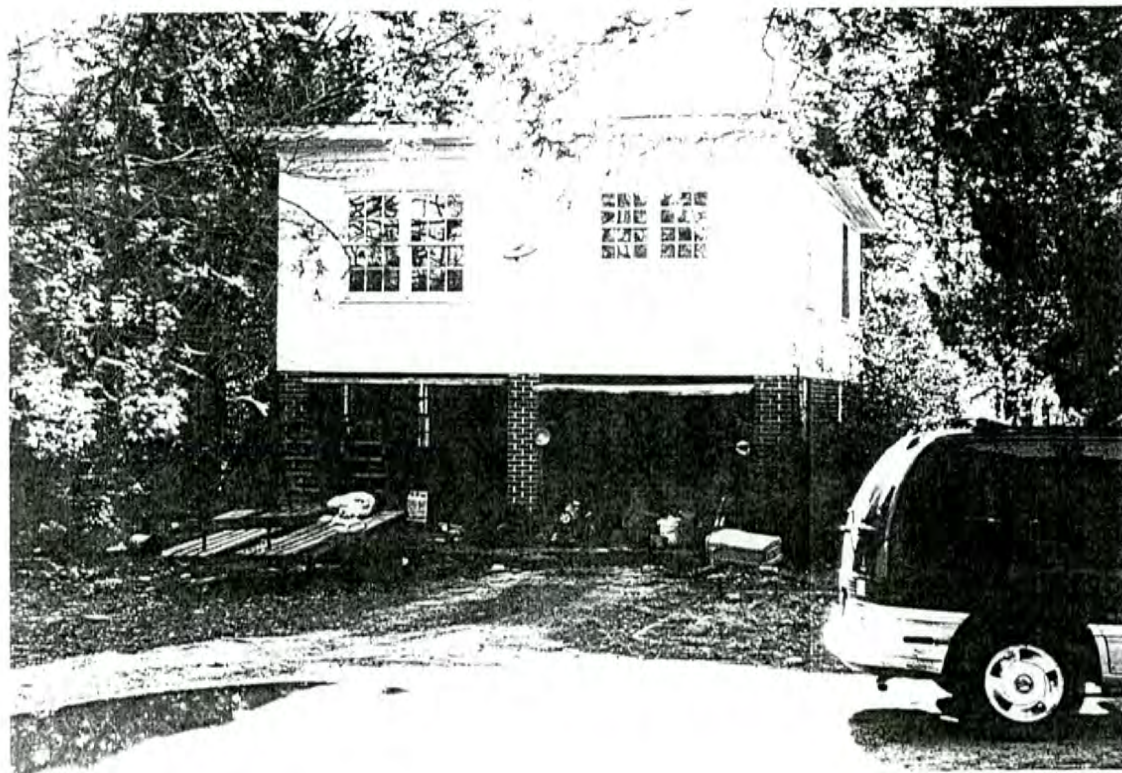
Plate 15: Ferebee House (#6)—east and north elevations of garage/ apartment
