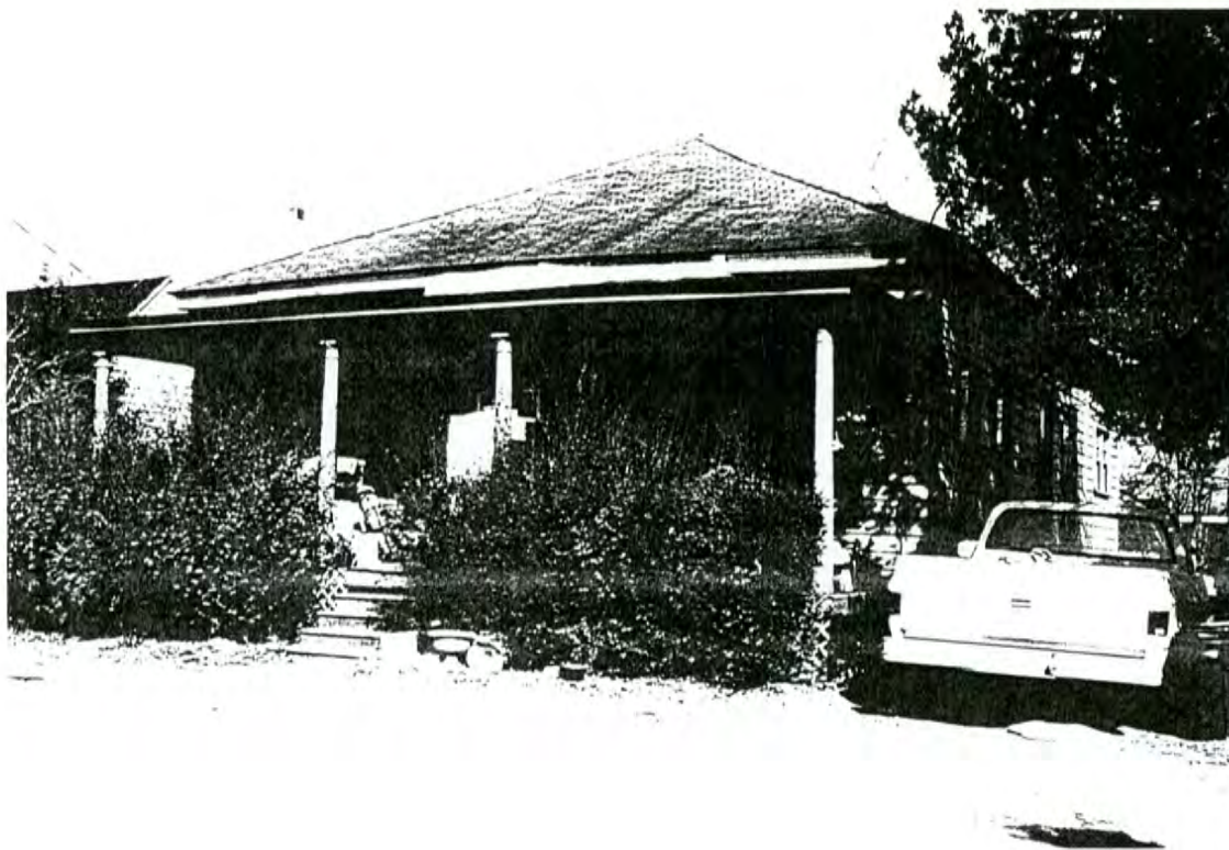
Plate 3: House (#41)— west front and south side elevations
