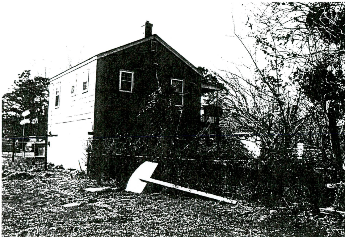
Plate 11: House (#43)— south and east elevations
