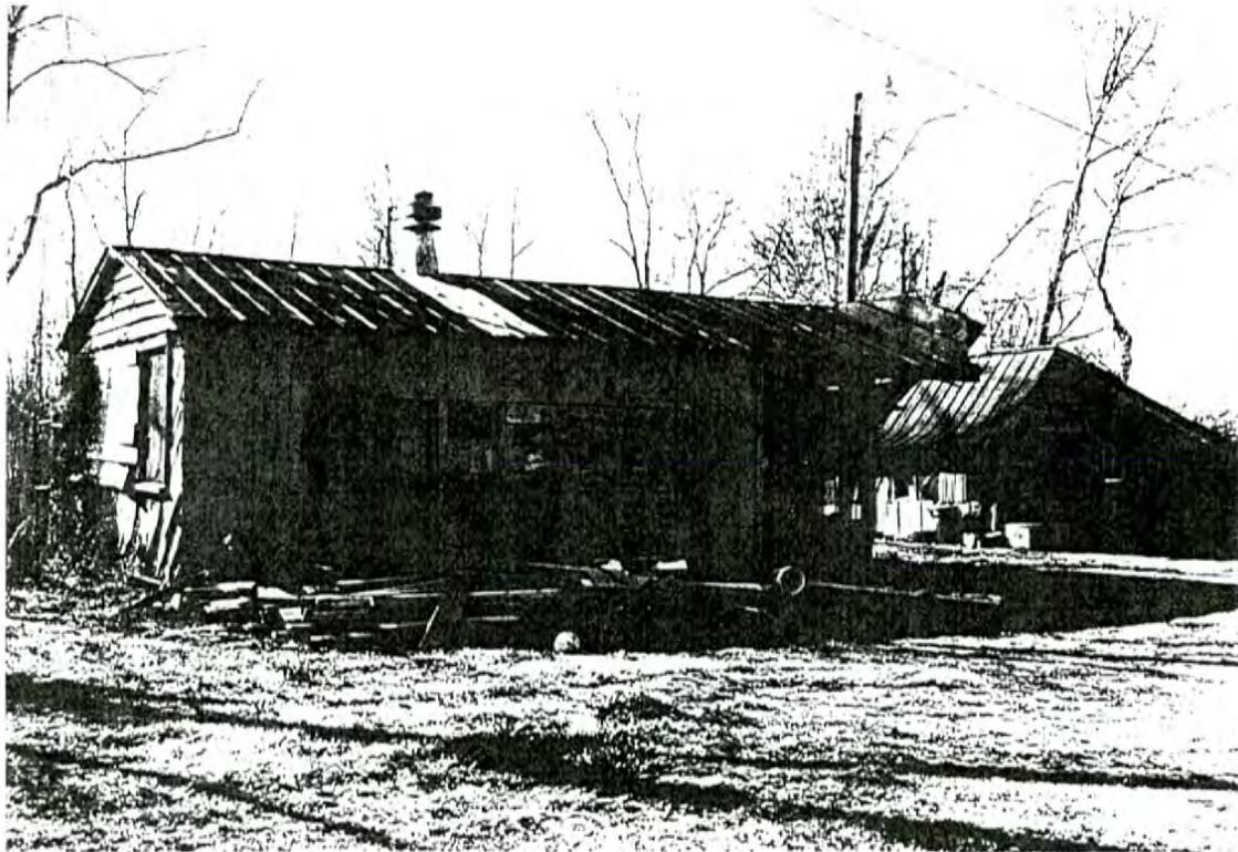
Plate 19: Charles Keener House (#20)—east and north side elevations of outbuildings
