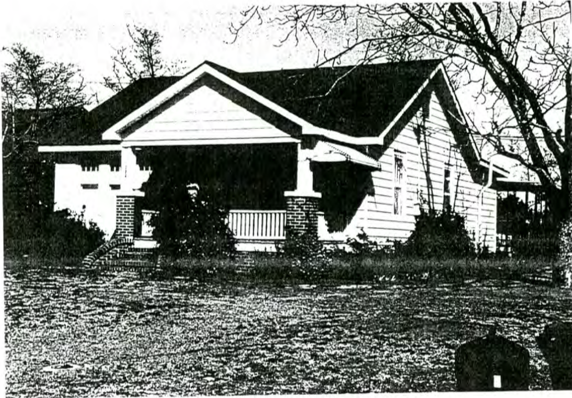
Plate 5: House (#44)— west front and south side elevations
