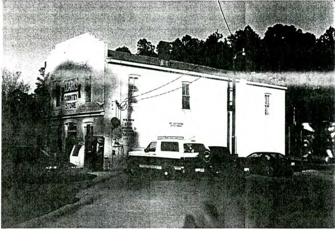
Plate 28: Abner Wetherington Store, SR 1225, Clarks
