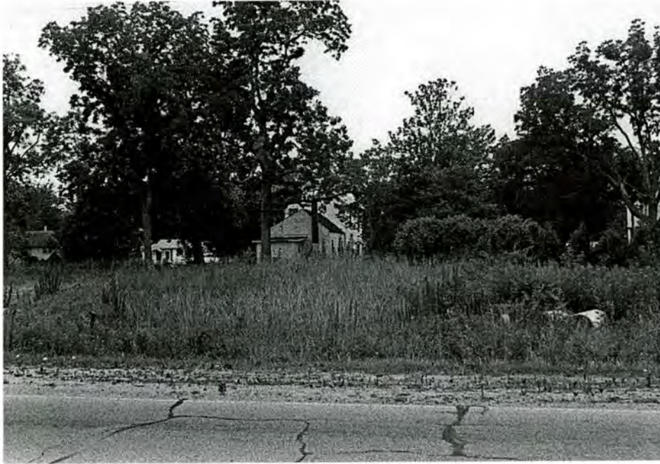
40. House, 912 C Street, Bridgeton Historic District. View W from US 17 to rear of house.
