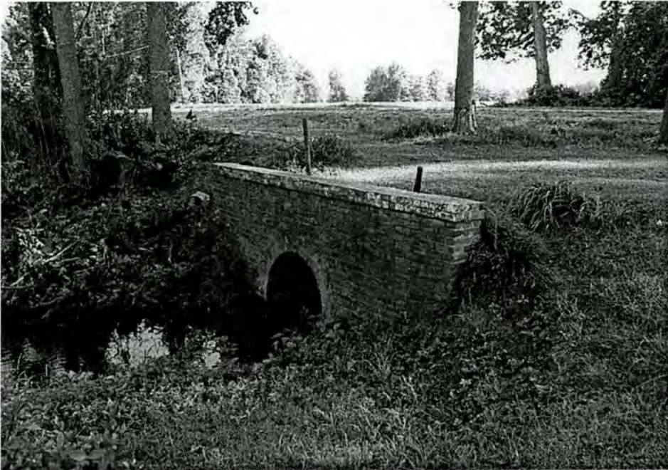
10. Brick Road (New Bern-Washington Brick Road Historic District). Original brick culvert.
