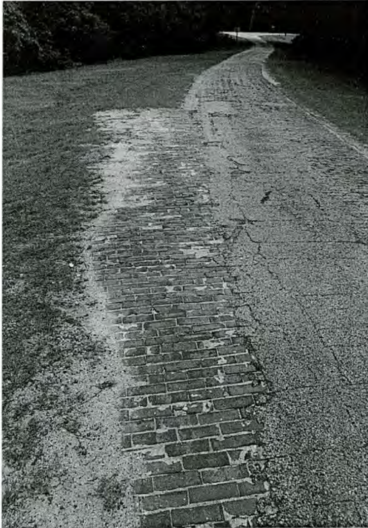
5. Ernul Brick Road (New Bern-Washington Brick Road Historic District). View S at US 17 terminus. Original brick pavers in foreground.
