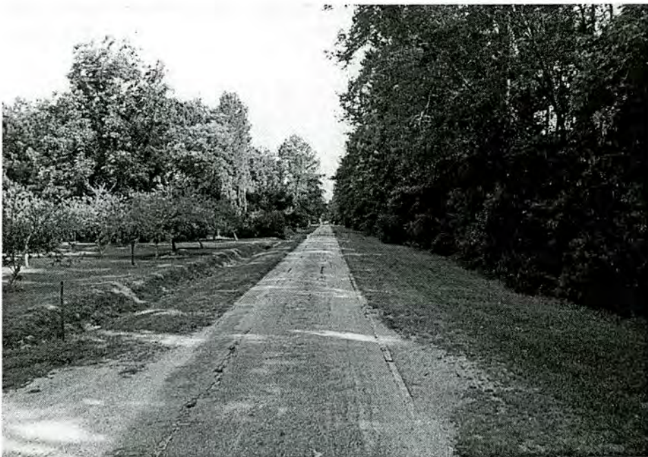
5. Ernul Brick Road (New Bern-Washington Brick Road Historic District). View S showing typical rural character.
