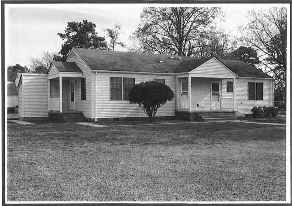
Figure 11. Above: Photograph of Building 312, Officers Single Family Residence. Below: Photograph of a typical Lanham Housing duplex unit (Building 597).
