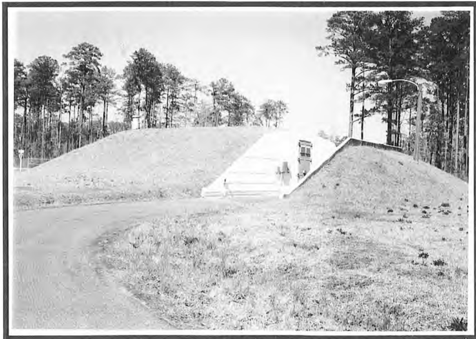
Figure 12. Above: Photograph of a typical above-ground magazine (Building 1231). Below: Photograph of a typical earth-covered magazine (Building 1203).
