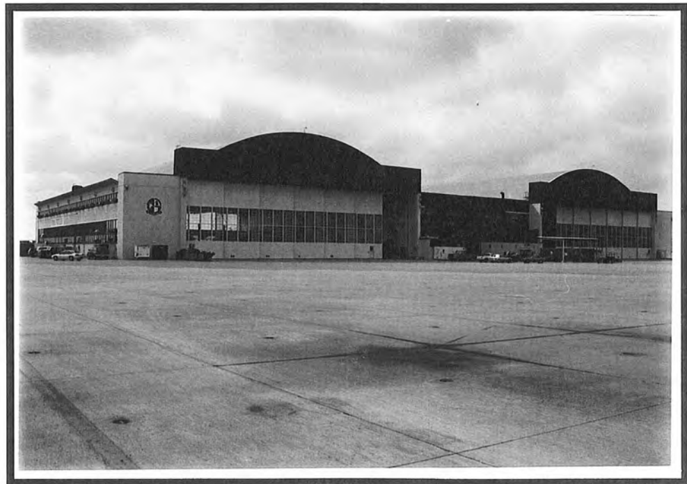
Figure 14. Above: Photograph of Hangar 188. Below: Photograph of Hangar 250.
