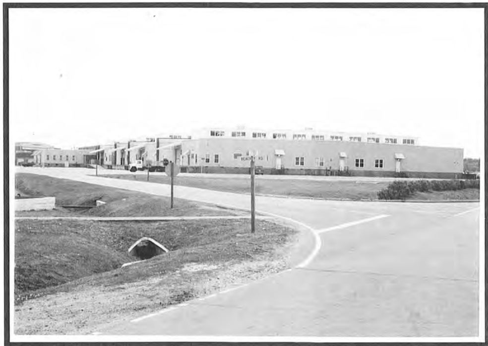
Figure 9. Above: Photograph of aircraft storehouse (Building 145). Below: Photograph of general storage warehouse (Building 150).
