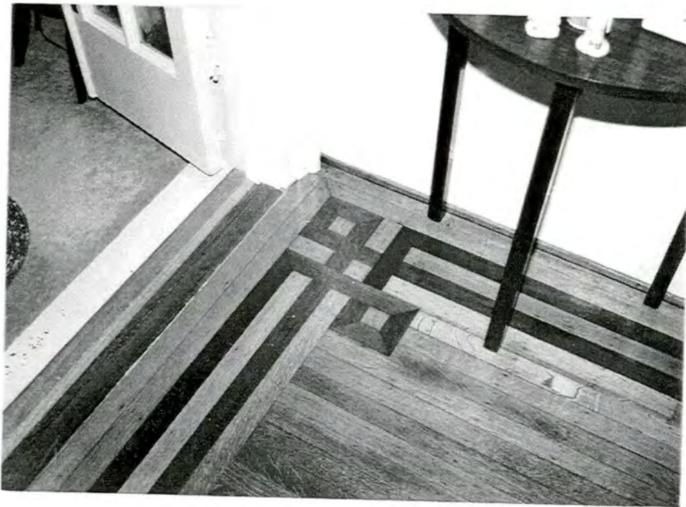
Spruill-Easley House. Floor detail in parlor.
