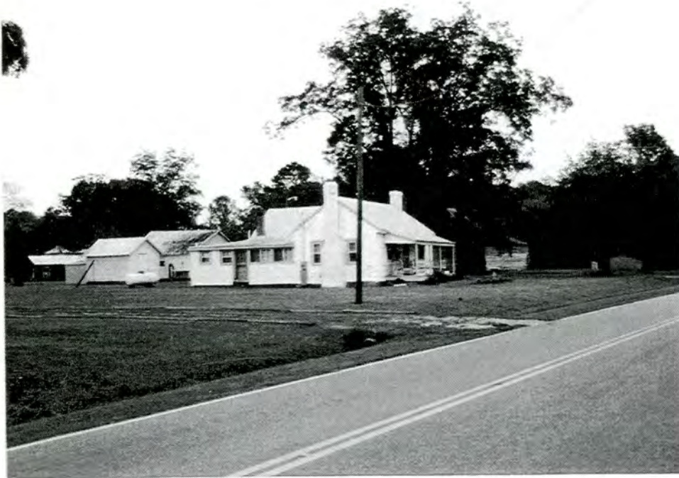
187. House and Outbuildings
