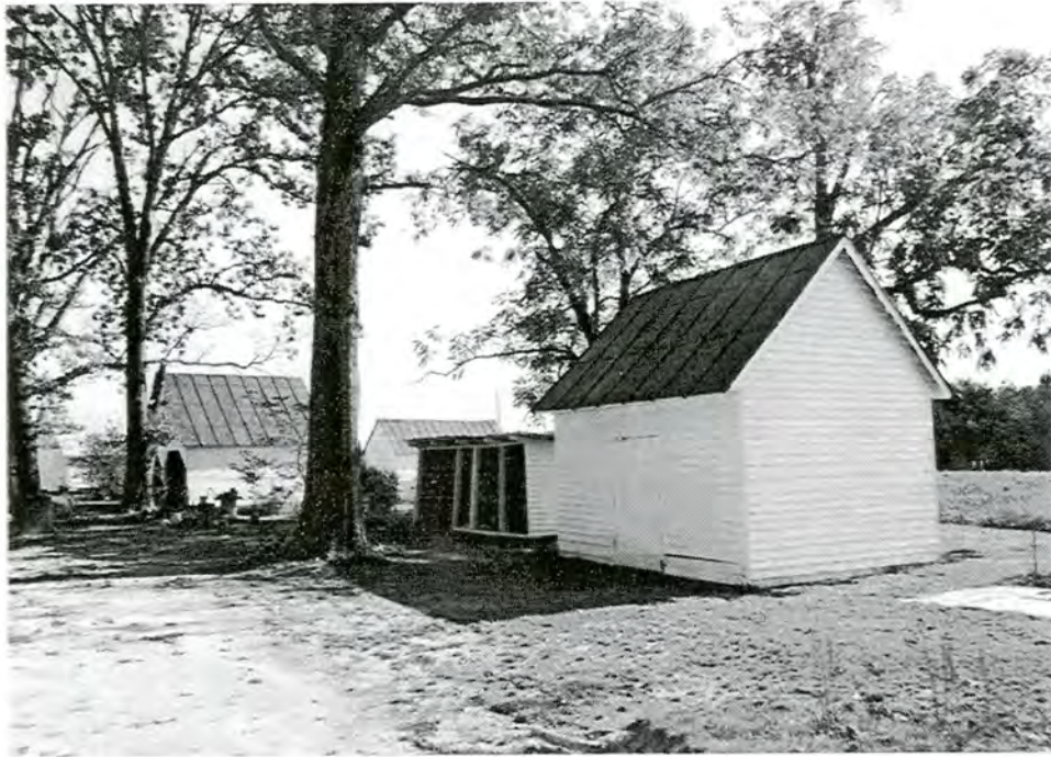
Daughtridge Farm. Commissary at left (B), equipment shed in middle (C), garage at left (D).
