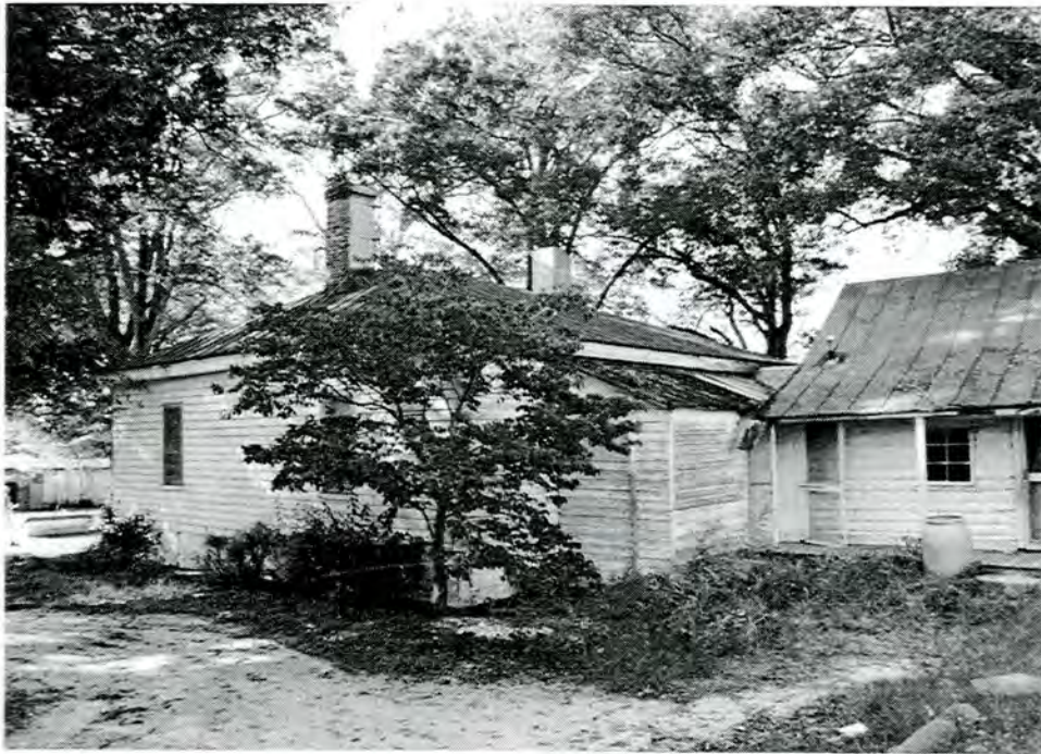
Worsley Overseer's House (R).
