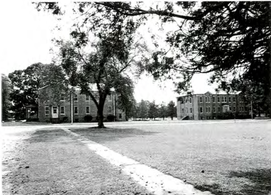
East Carolina Industrial Training School. Home Building (left) and McCain Building.
