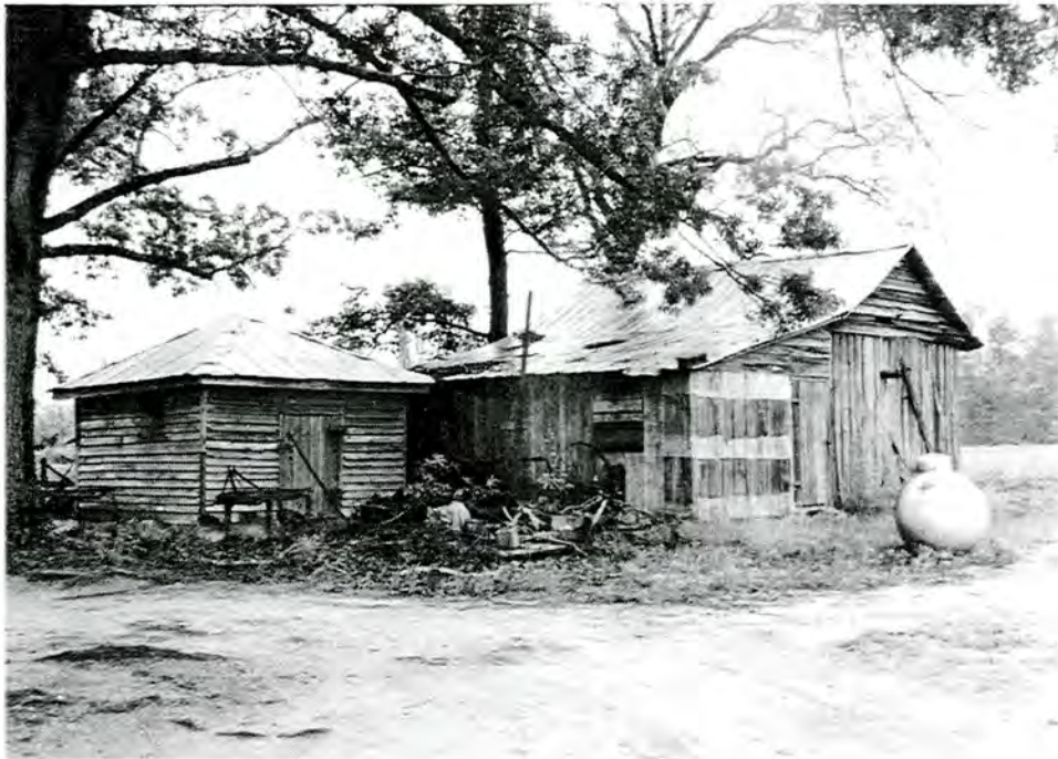
Brown Farm. Hipped-roof shed (O) and barn (P).
