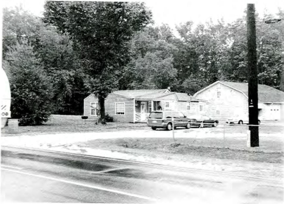
34. House and Outbuildings
