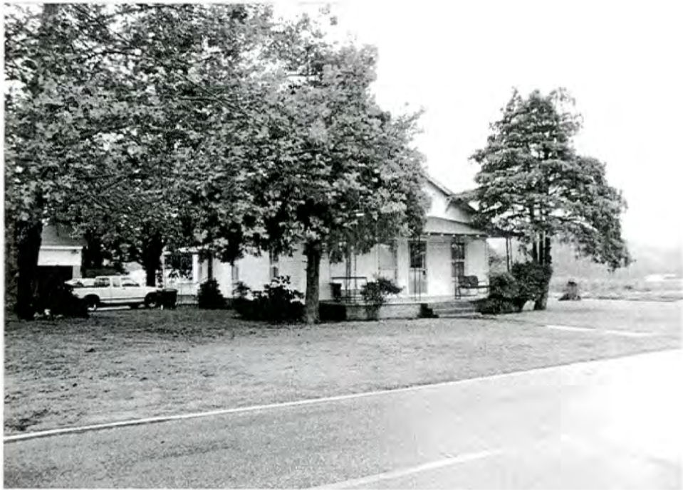
32. House and Outbuildings
