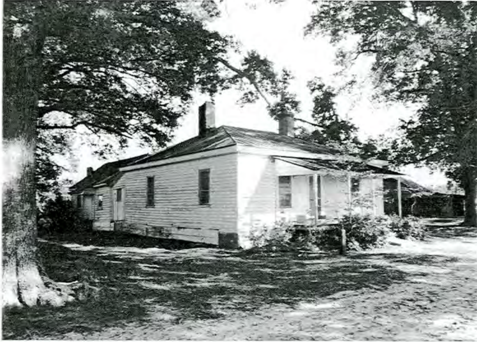
Worsley Overseer's House (R).
