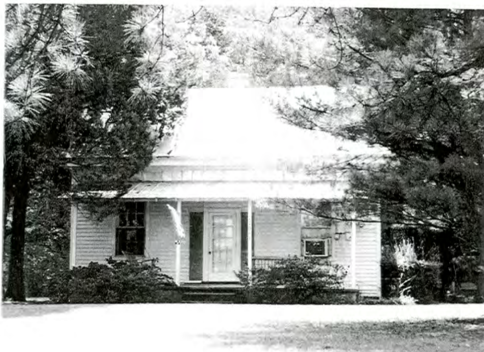
74. House and Outbuildings
