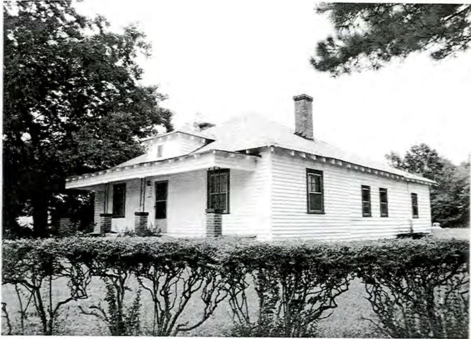
101. House and Outbuildings
