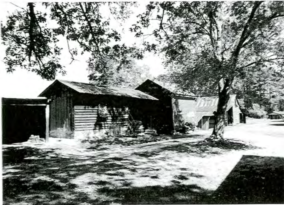
Bulluck Farm. Office-packhouse (G); hay loft in background (K).
