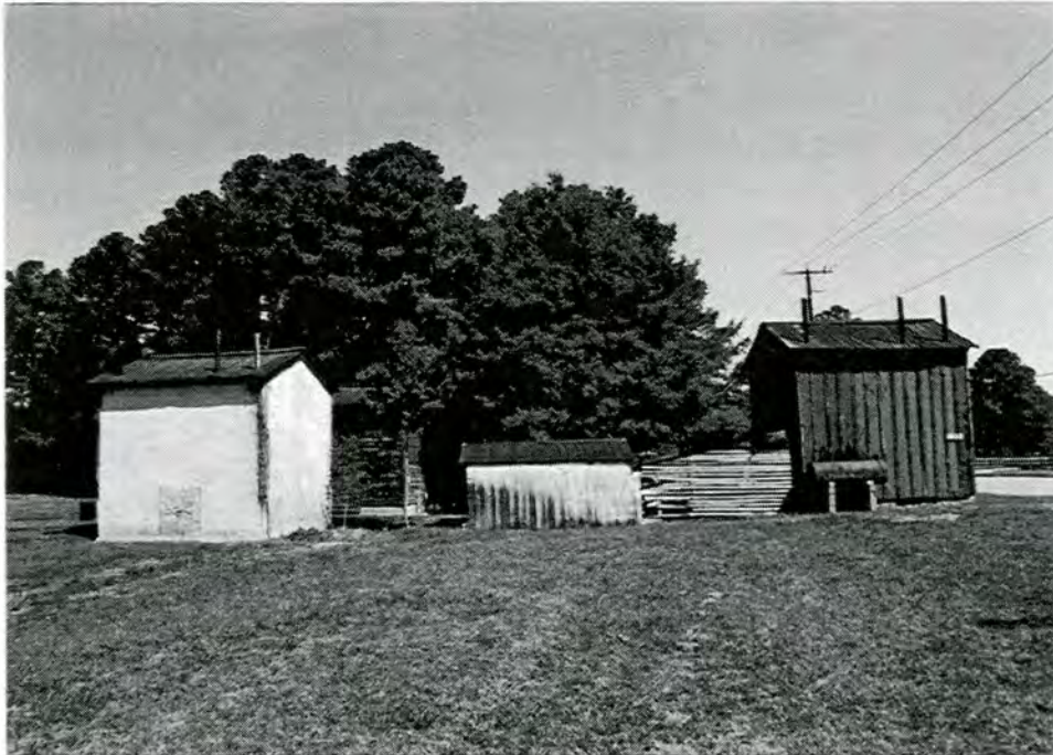
Bulluck Farm. Left to right: tobacco barns (N, O), tractor shed (P), and tobacco barn (Q).
