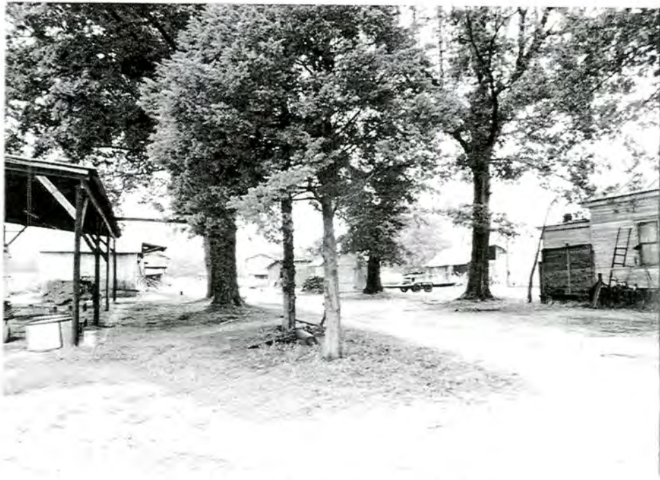
Brown Farm. View N of farm complex lane.
