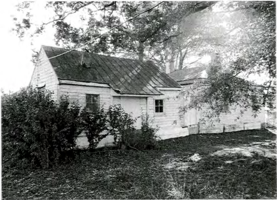
Worsley Overseer's House (R).
