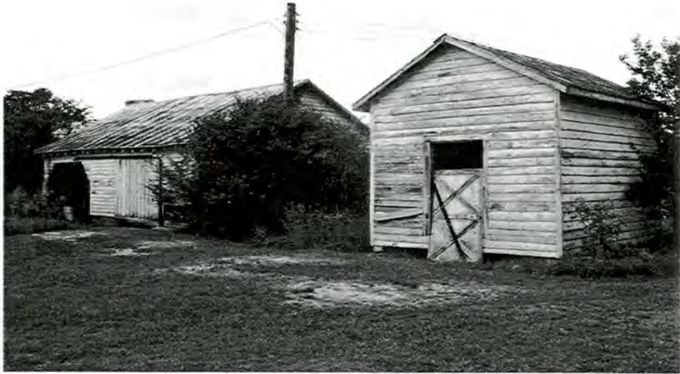
Ricks-Boseman Farm. Garage and shed.
