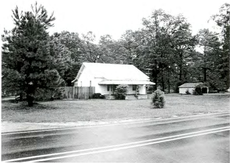
36. House and Outbuildings
