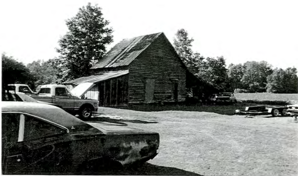
Worsley Tenant House. Packhouse (B).
