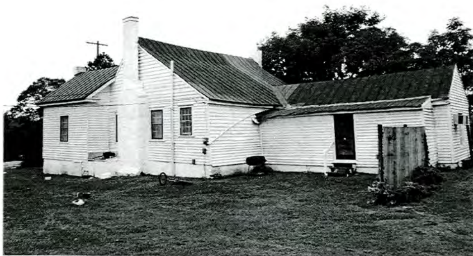
Haverson Griffin House. View from NE.
