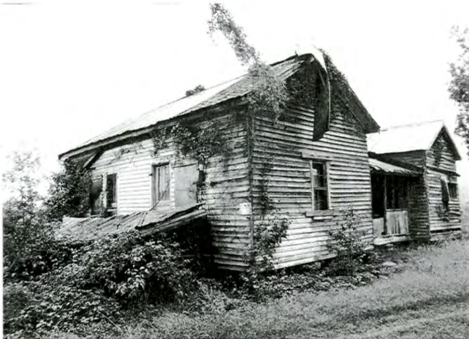
14. House and Outbuildings
