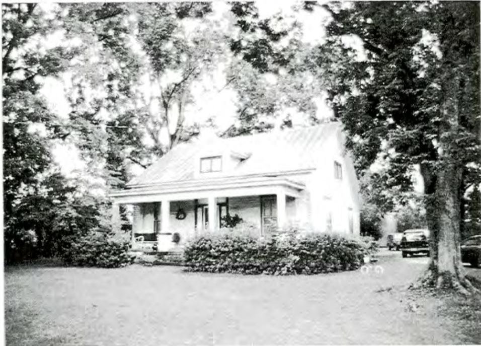
173. House and Outbuildings
