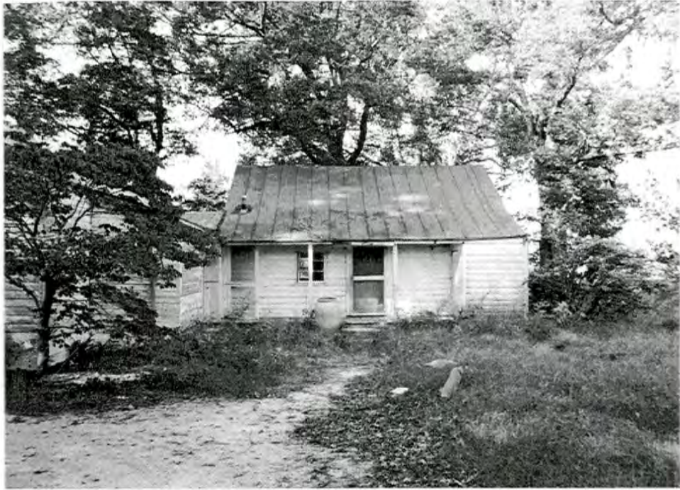
Worsley Overseer's House (R).
