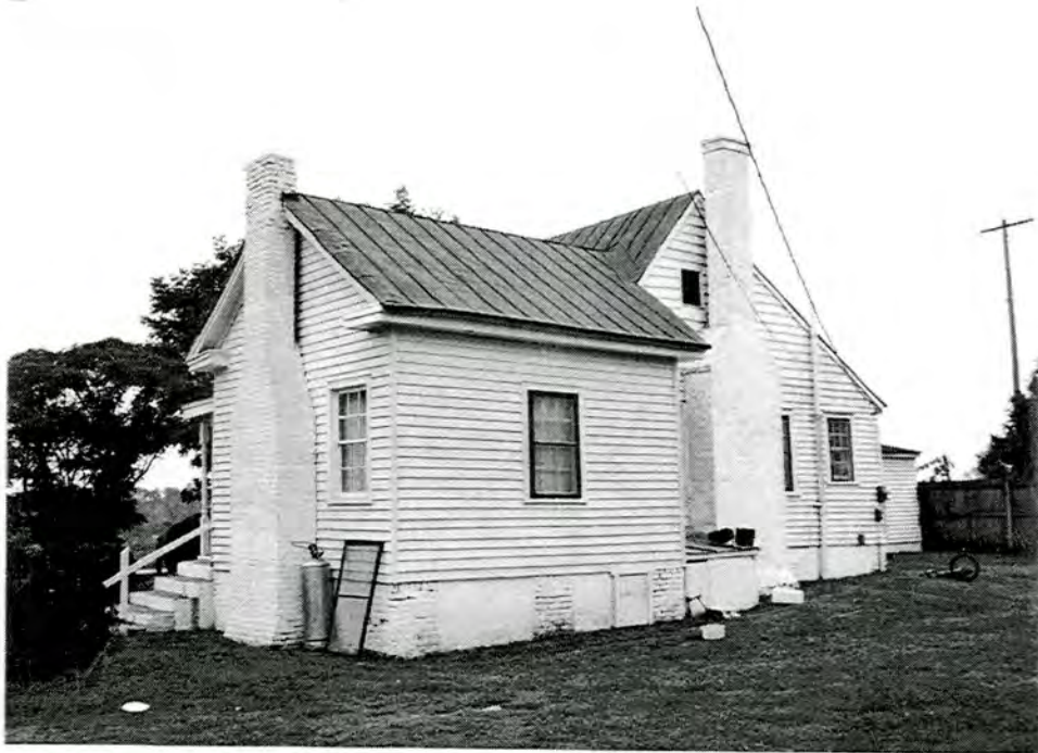
Haverson Griffin House. View from SE.
