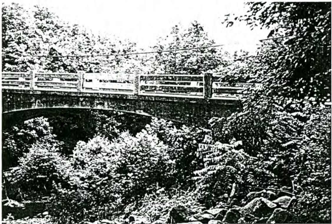
Figure 4 – View of Bridge No. 42
