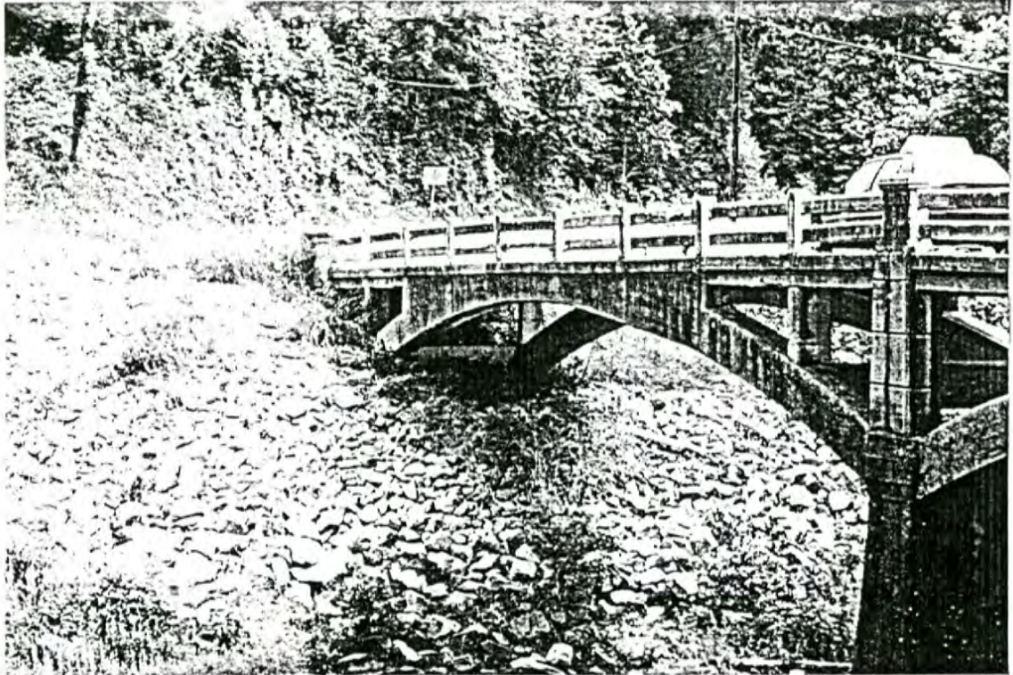
Figure 3 – View of Bridge No. 42
