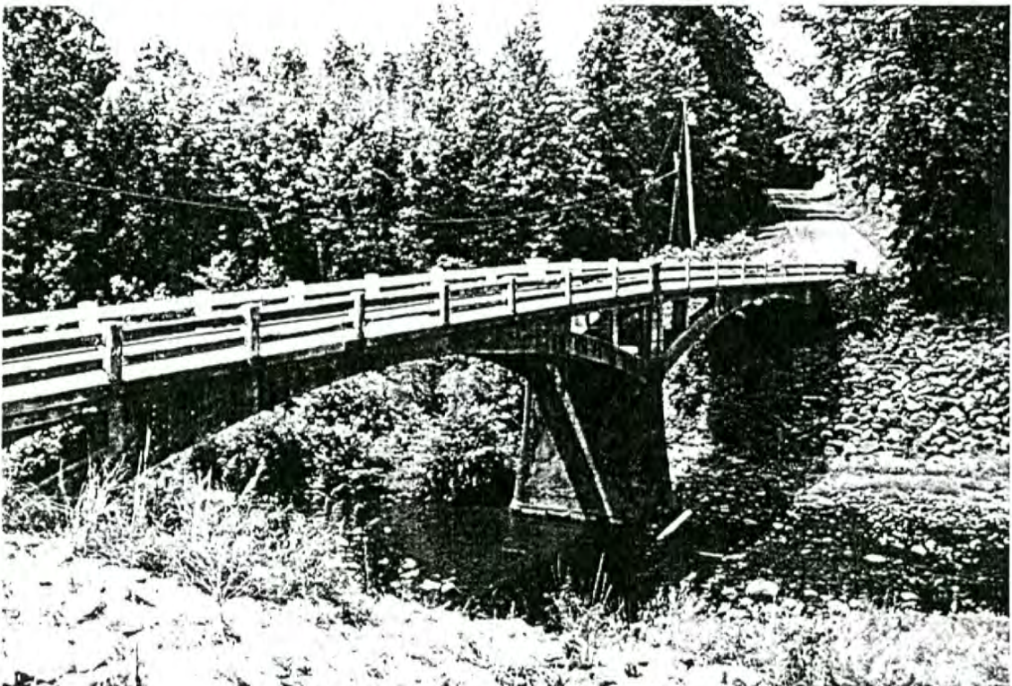
Figure 2 – View of Bridge No. 42
