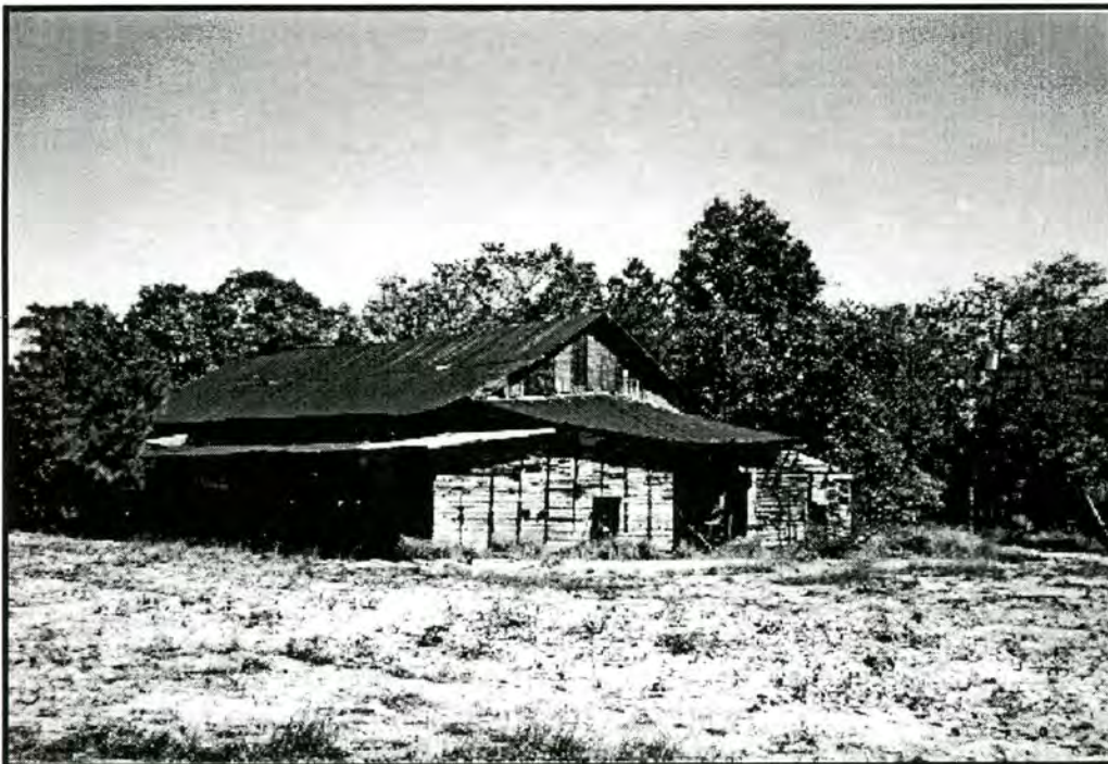
Fig. 13 Property #5 - Barn View Southeast
