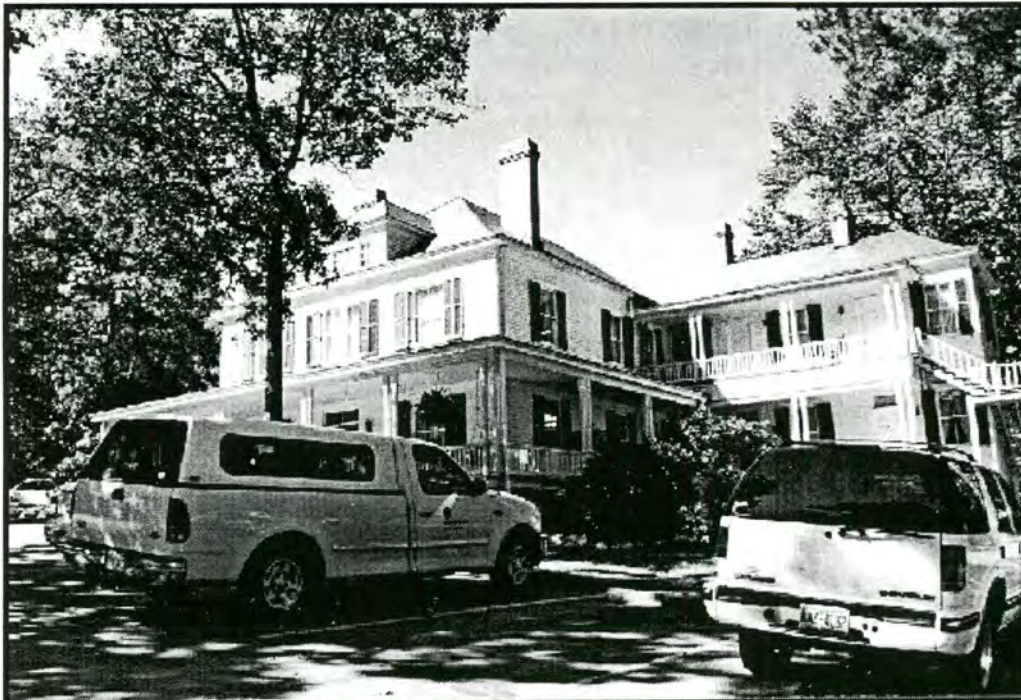
Fig. 4 Property #1 - Ellerbe Springs Hotel View Southwest
