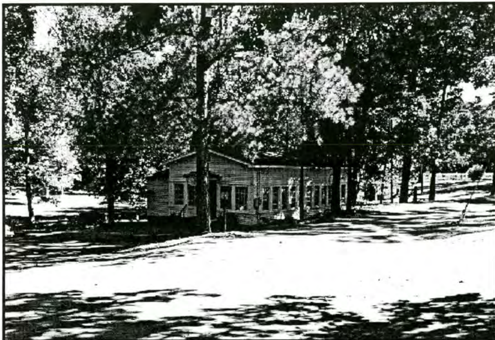
Fig. 7 Property #1 - Dance Pavilion or "Springhouse" View Northeast
