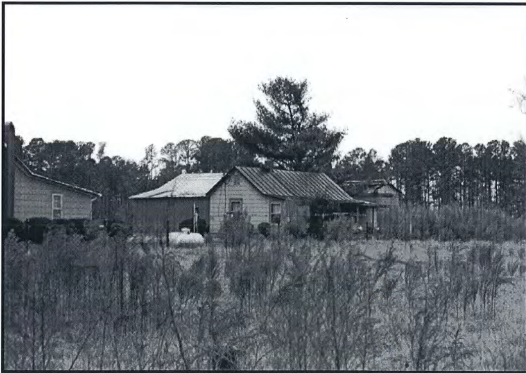
Fig. 8 Property #5 - Outbuilding/Dwelling View Northwest
