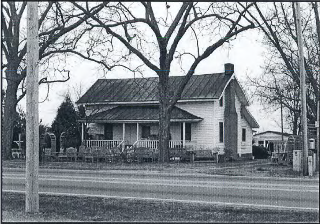
Fig. 14 Property #9 - House West (Street) Facade
