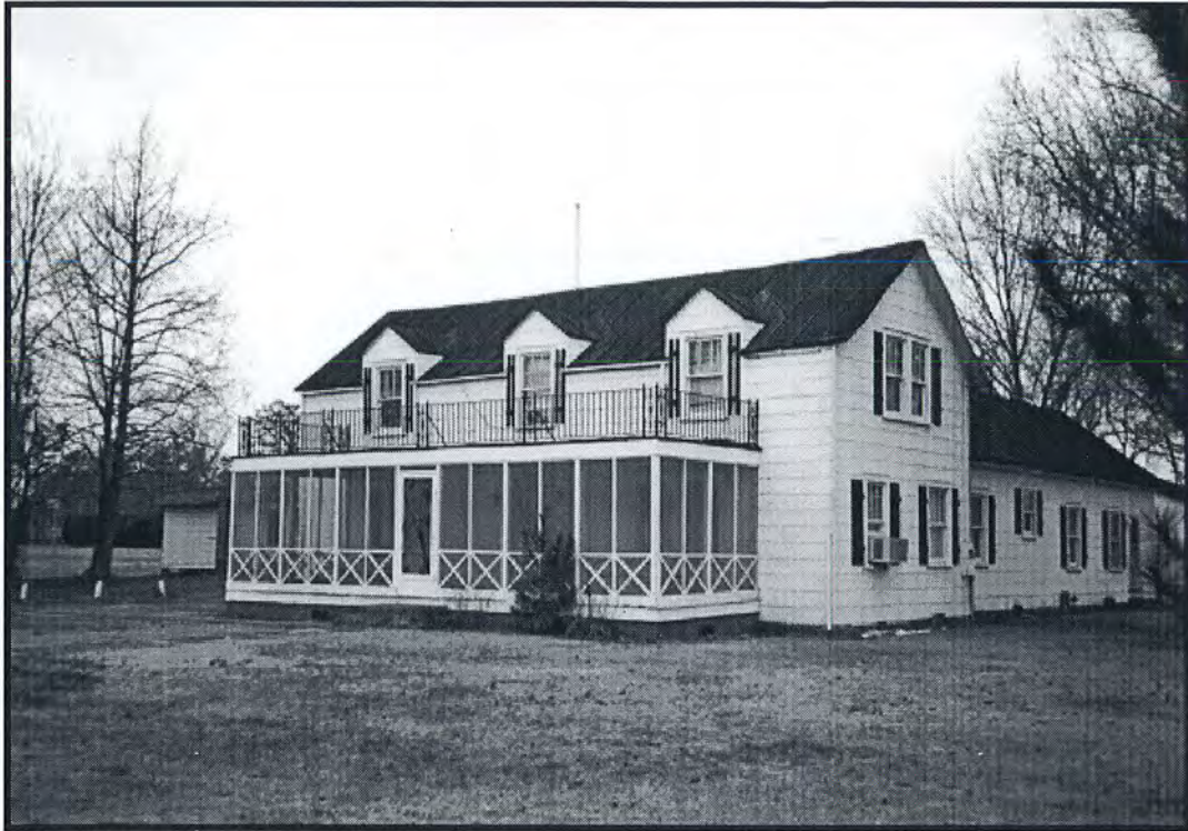
Fig. 12 Property #8 - House South (Street) Facade
