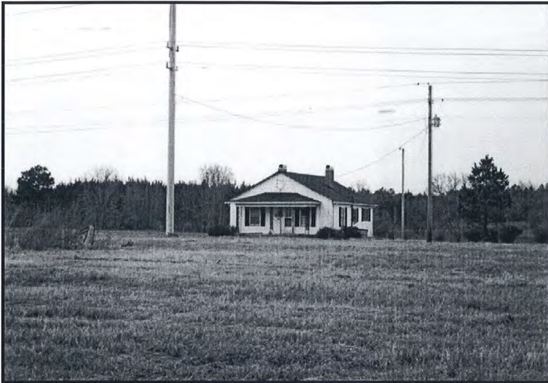
Fig. 15 Property #10 - House South (Street) Facade
