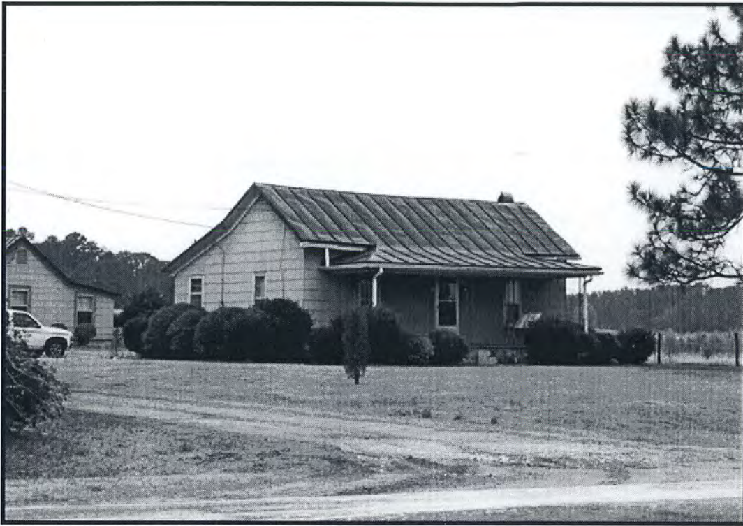
Fig. 7 Property #5 - House South (Street) Facade
