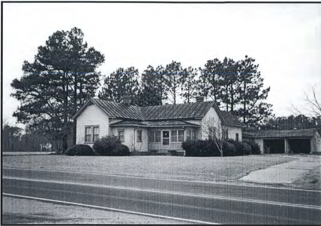
Fig. 6 Property #4 - House South (Street) Facade
