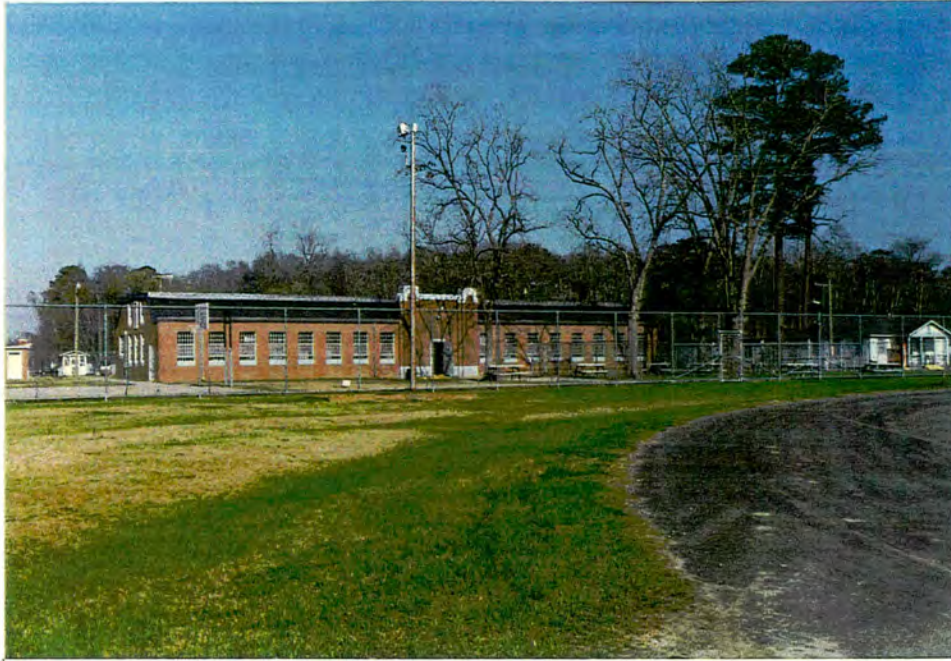
Washington Correctional Center. View of original dormitory from S. (Warden's house/office at extreme R).
