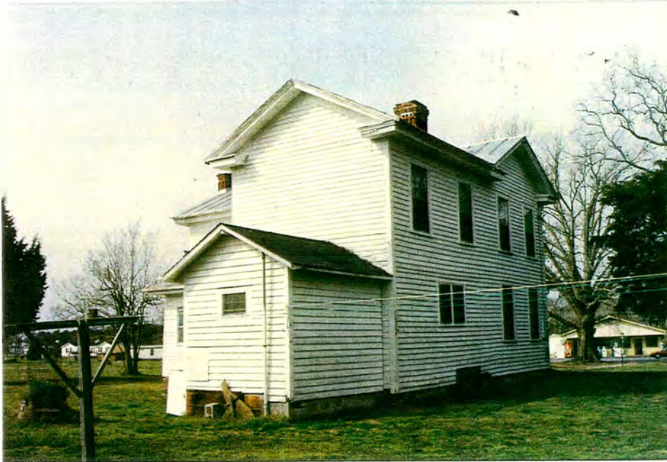
Farm (#133). View of farmhouse from SE.
