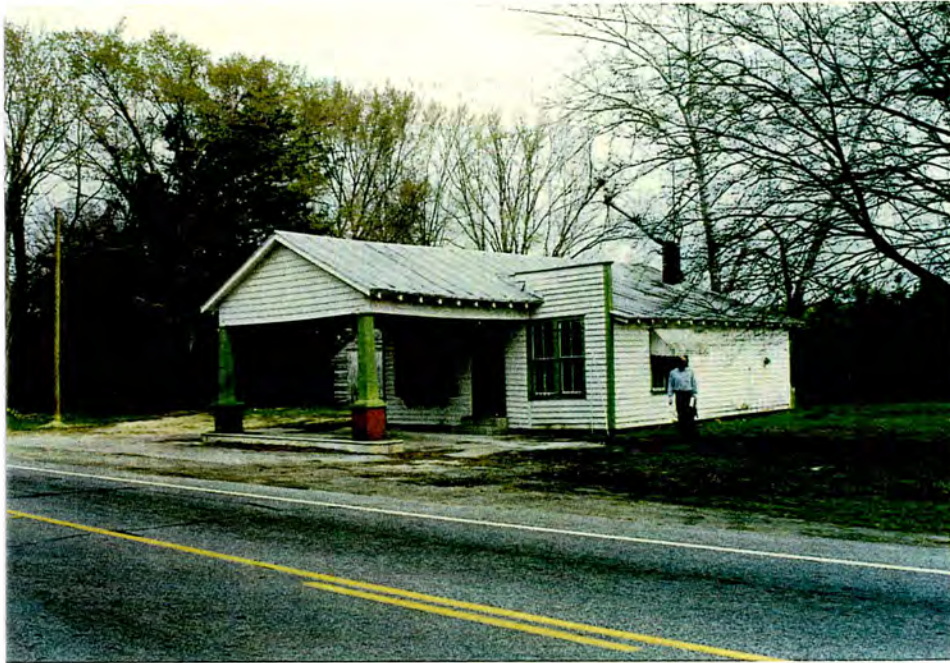
Pleasant Grove Store. View from NW. ED standing at edge of ROW.
