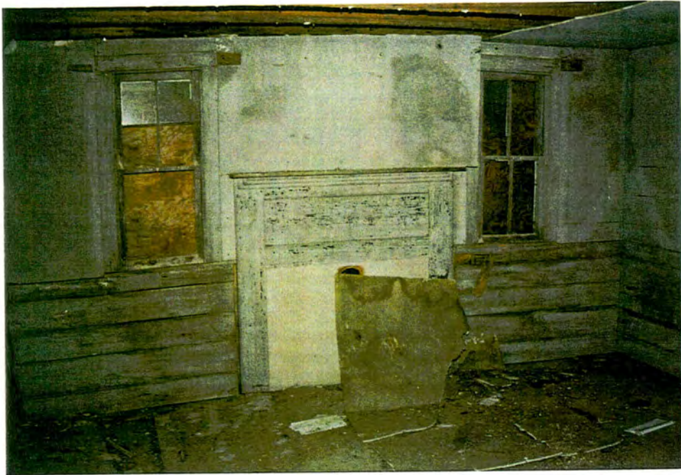
Homestead Farm. Mantel in Thompson House.
