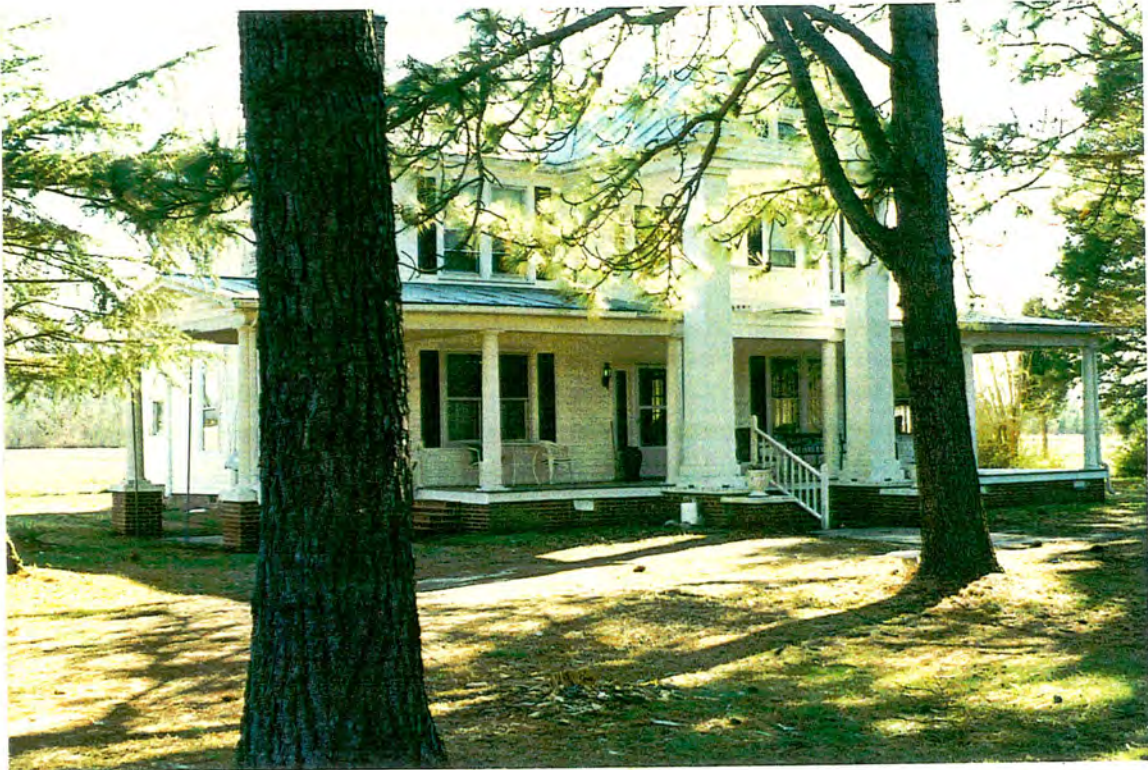
Tarkenten House. View from NE.
