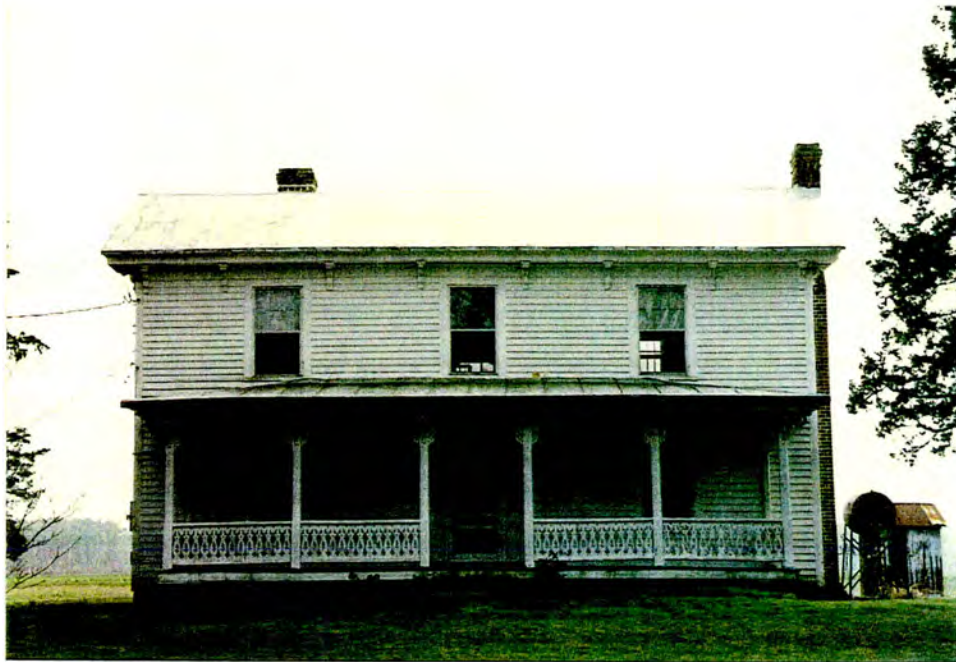
Farm (#133). North elevation of farmhouse.
