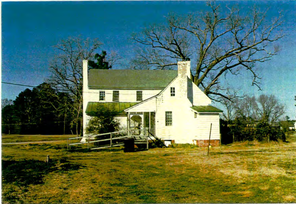
Hassell House. South elevation.
