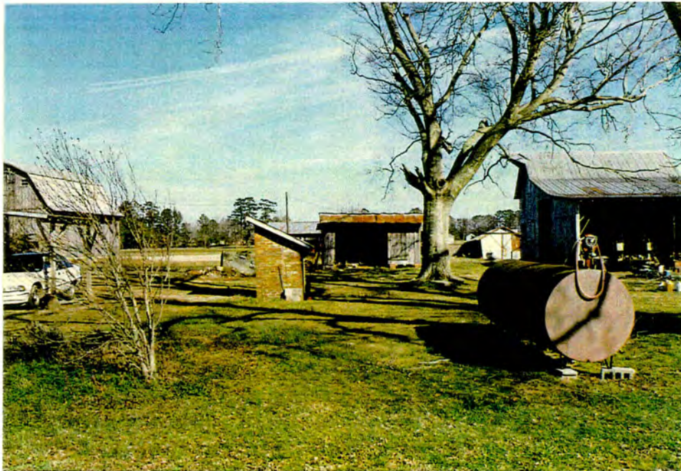
W. W. Mizell Farm. Outbuildings behind farmhouse.
