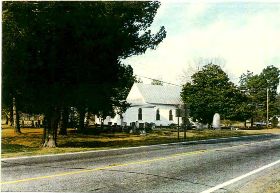
Pleasant Grove Methodist Church. View NE.
