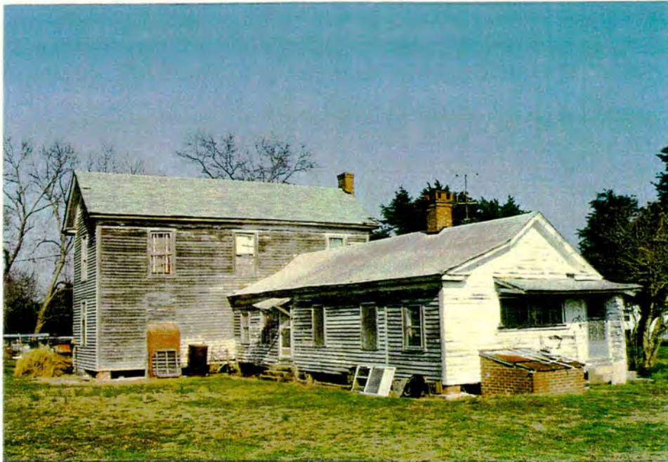
Pritchard Farm. View of farmhouse from SW.
