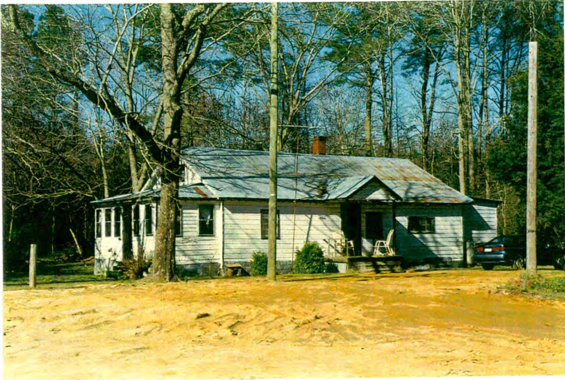
146. House (#2 in June 1, 1996 report)
