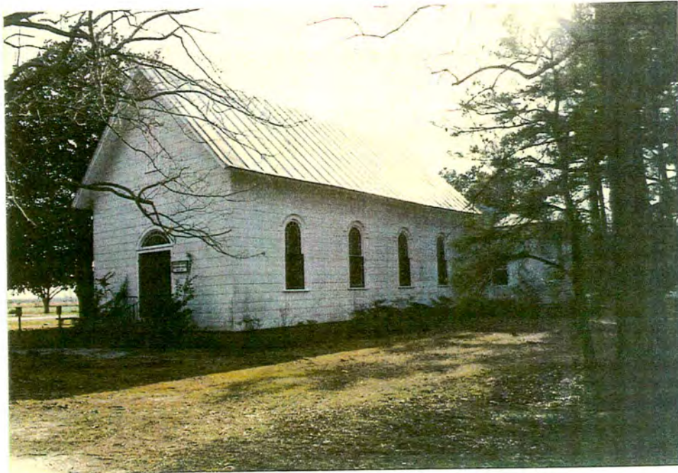
Pleasant Grove Methodist Church. View SW.
