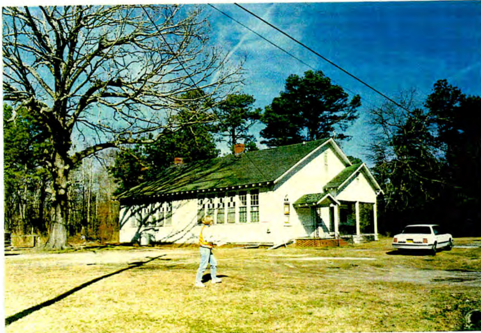
Former Rosenwald School. View from SW.
