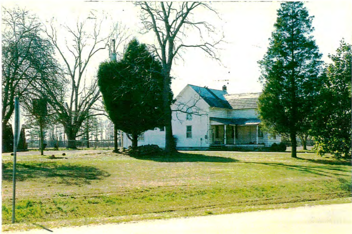
145. House (#3 in June 1, 1996 report)
