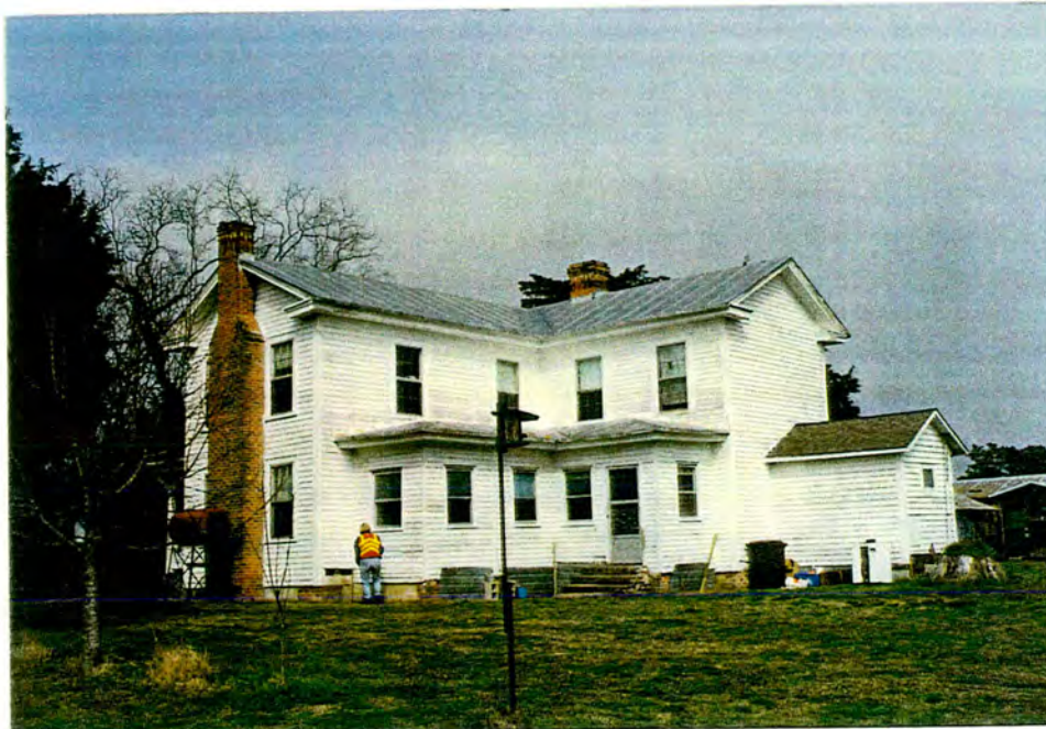
Farm (#133). View of farmhouse from SW.
