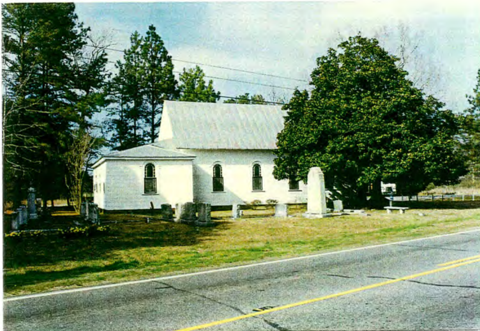
Pleasant Grove Methodist Church. South elevation (facing US 64).
