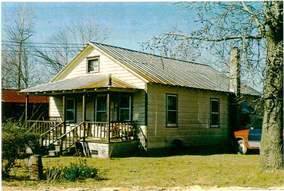
144. House (#4 in June 1, 1996 report)
