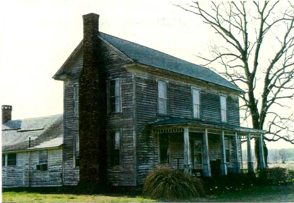
Pritchard Farm. View of farmhouse from NE.
