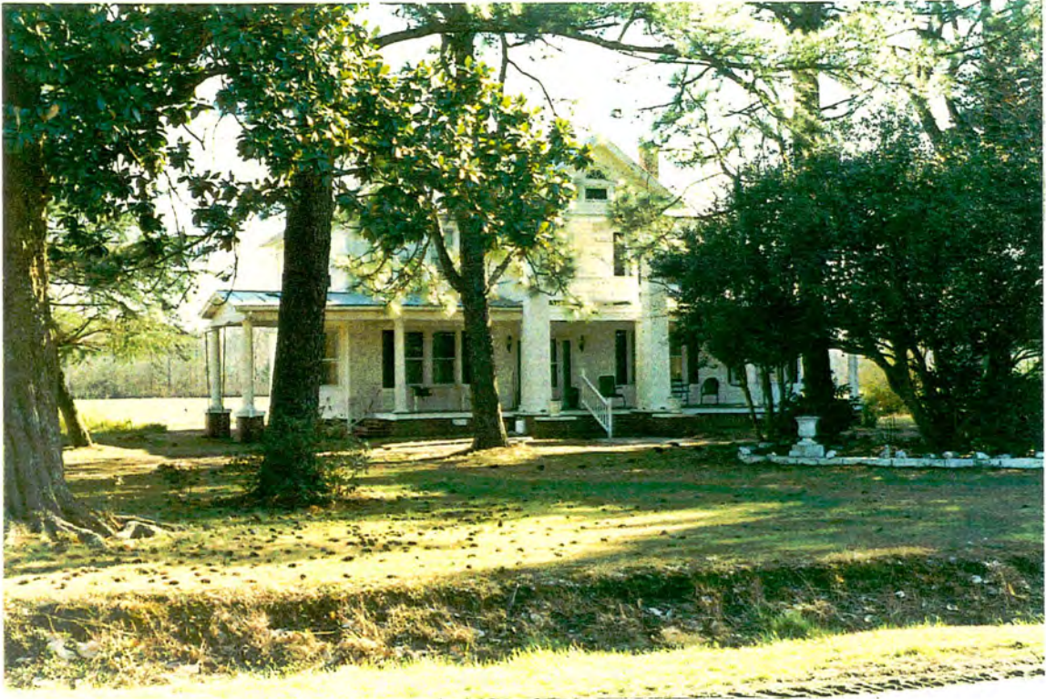
Tarkenten House. View from NE.
