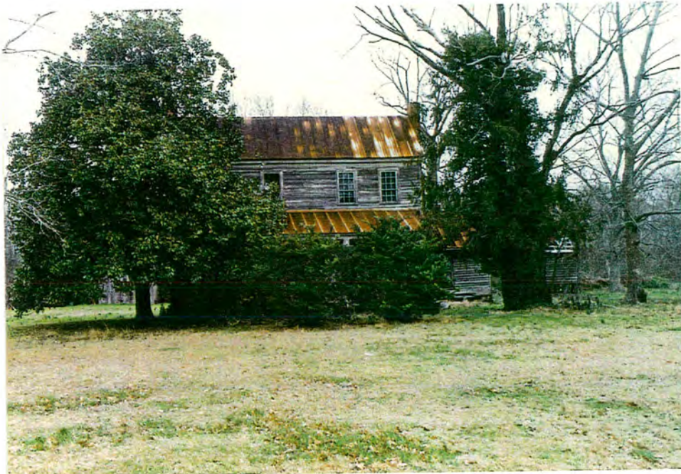
William R. Chesson House. South elevation.
