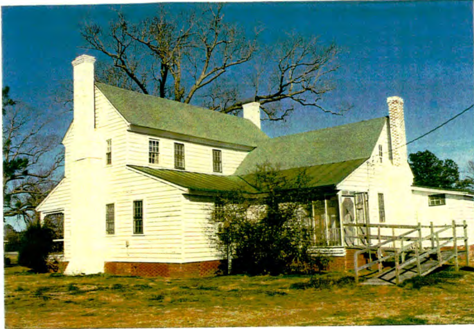
Hassell House. View from SW.
