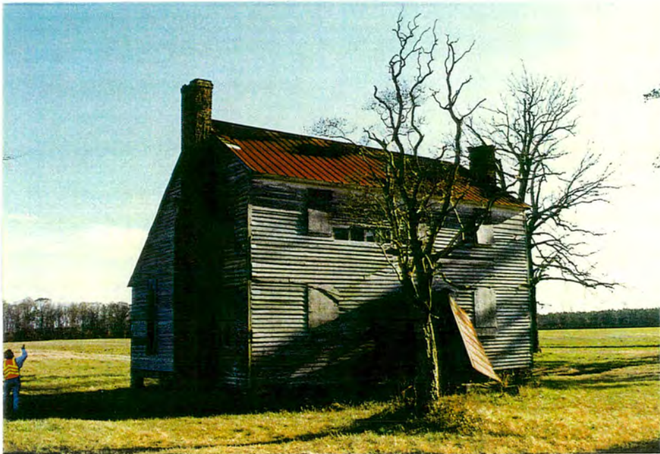
Homestead Farm. View of Thompson House from NE.
