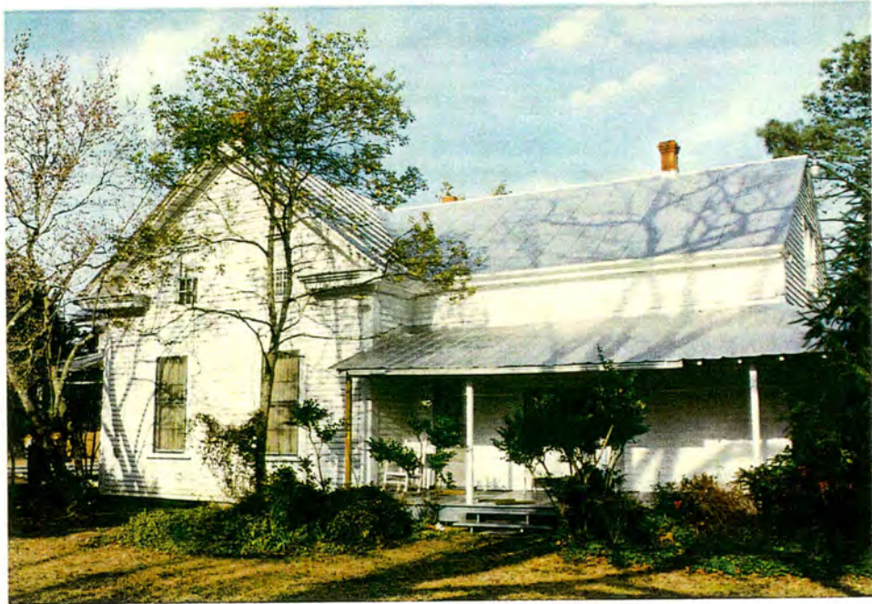
Former Schoolhouse. West elevation.
