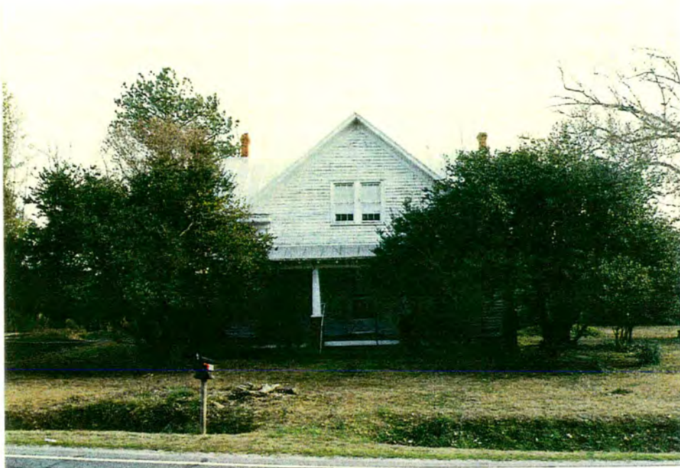
Former Schoolhouse. North elevation.
