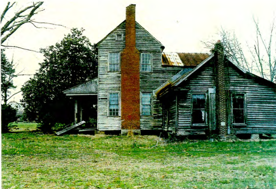
William R. Chesson House. East elevation.
