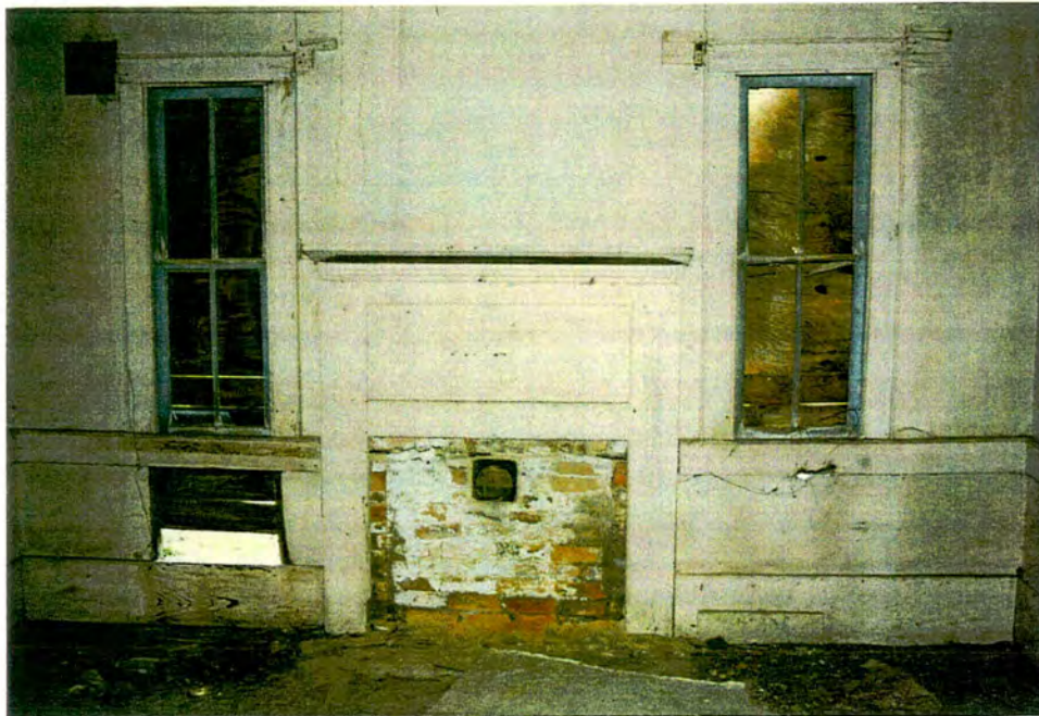
Homestead Farm. Mantel in Thompson House.
