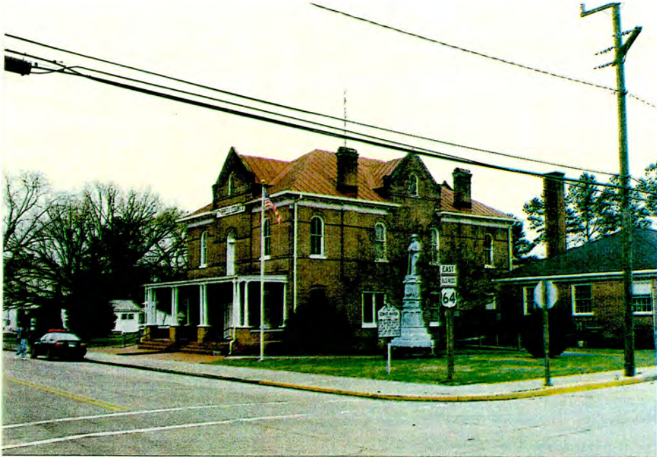
Columbia H.D. Tyrrell County Courthouse (NR). Not in APE.
