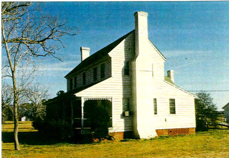
Hassell House. View from NW.
