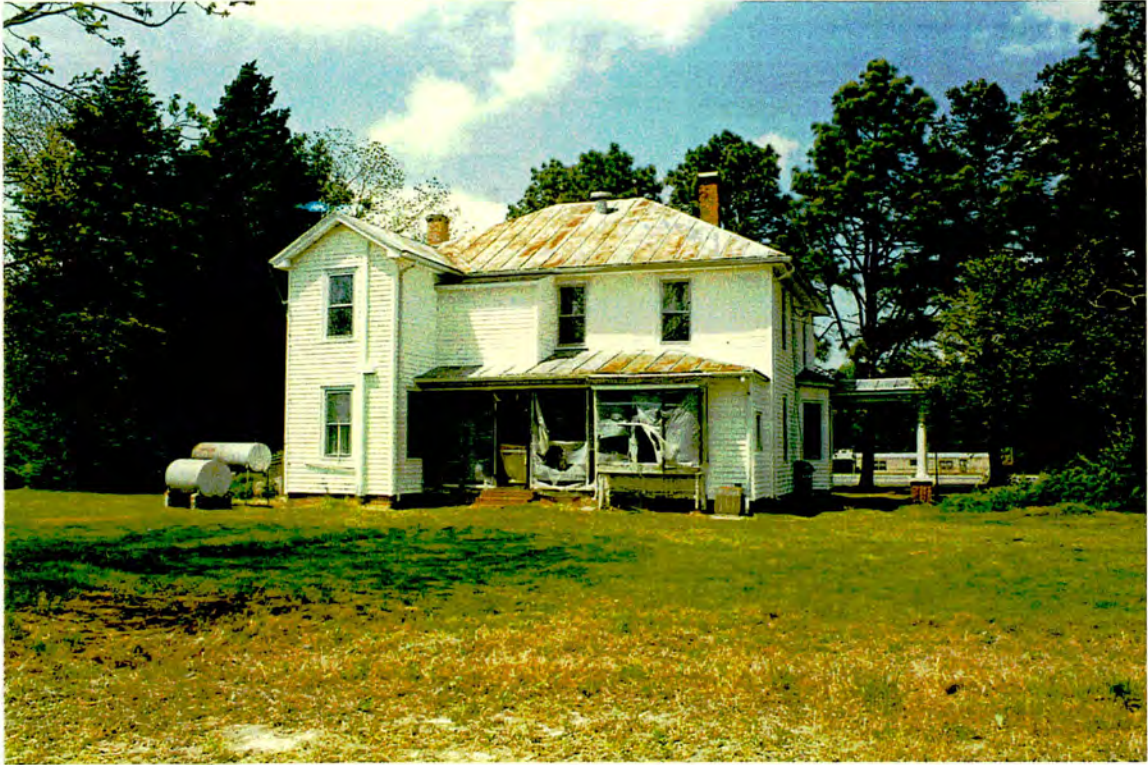
Tarkenten House. South elevation.
