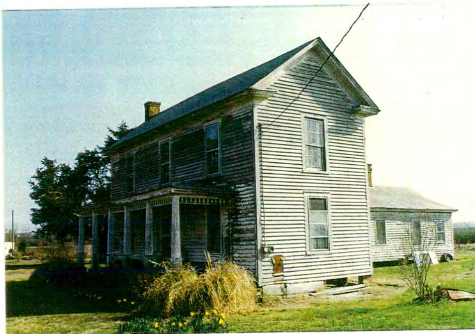
Pritchard Farm. View of farmhouse from NW.
