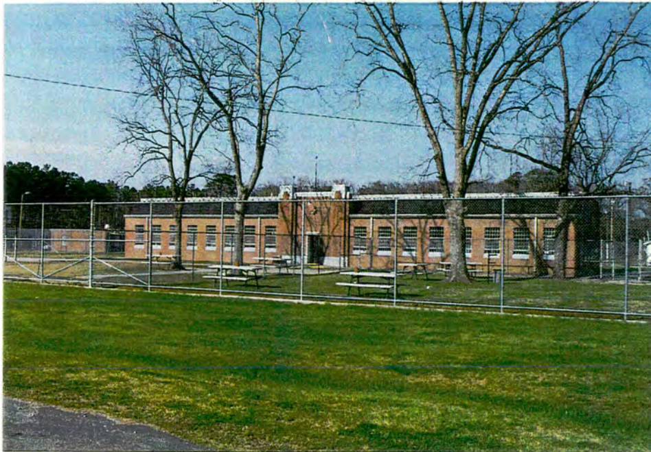
Washington Correctional Center. View of original dormitory from SE.
