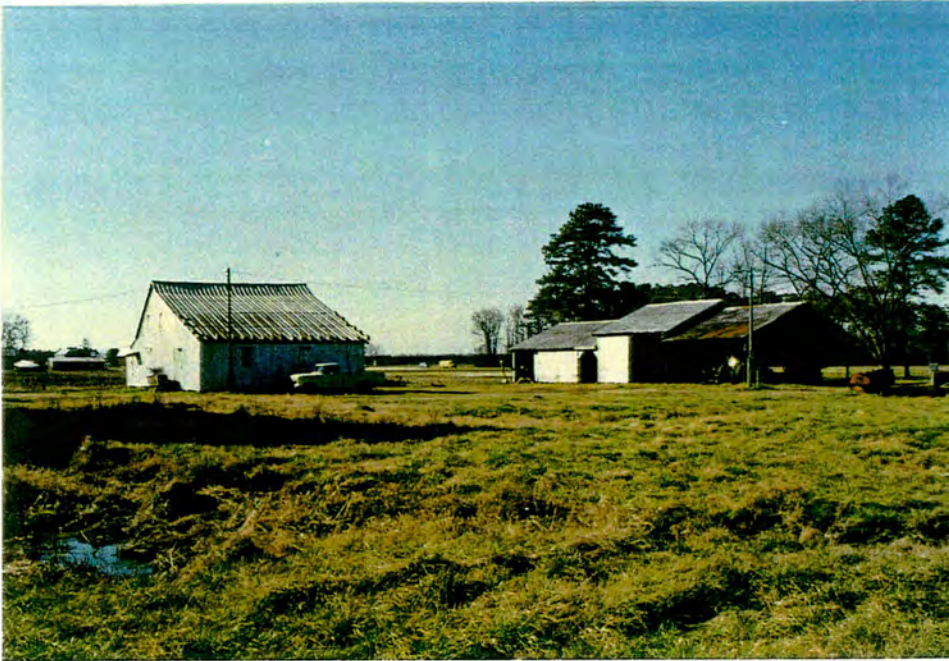
Homestead Farm. Metal-sided building and equipment sheds SW of Hassell House.
