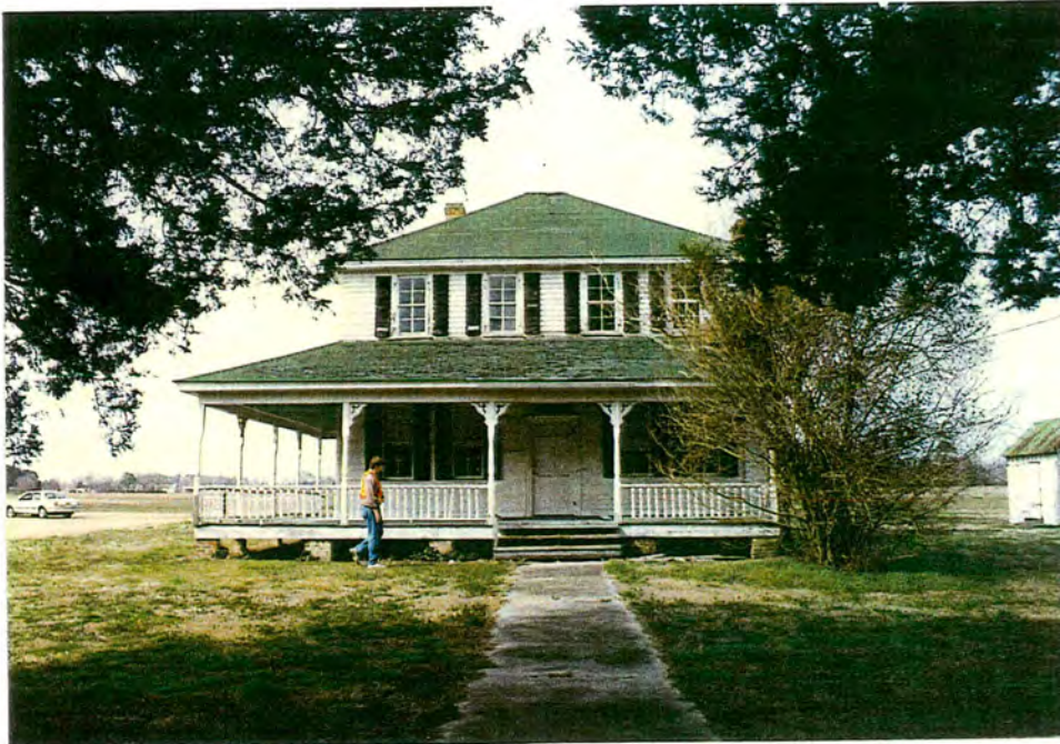
Downing-Spruill House. South elevation.
