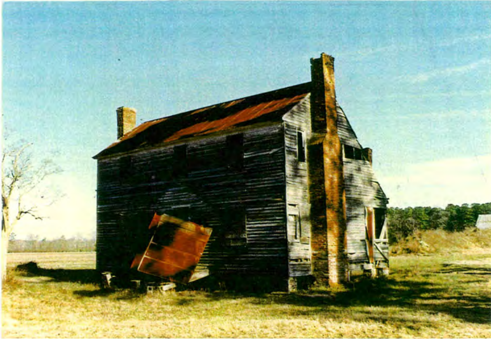
Homestead Farm. View of Thompson House from NW.
