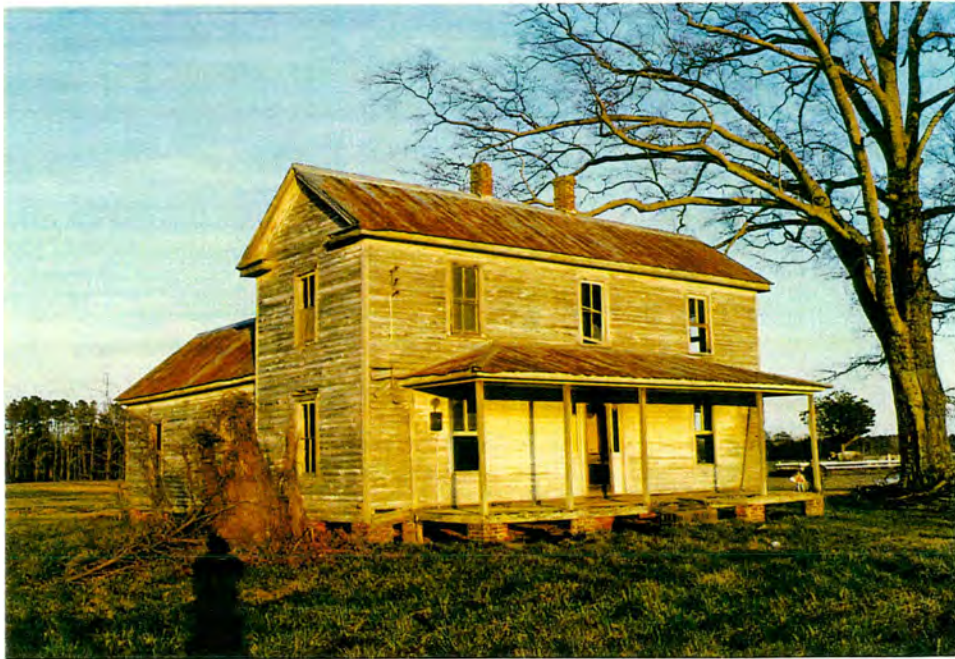
Turner Farms. View of two-story farmhouse from NW (#42).
