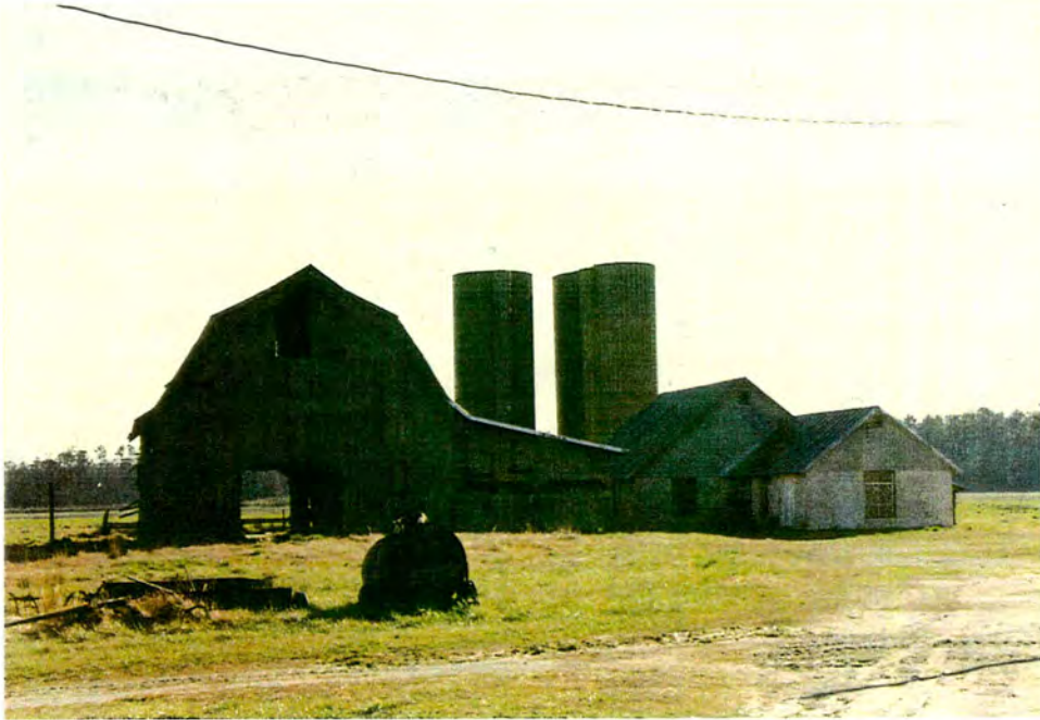
Homestead Farm. Barn, concrete block buildings, and silos.
