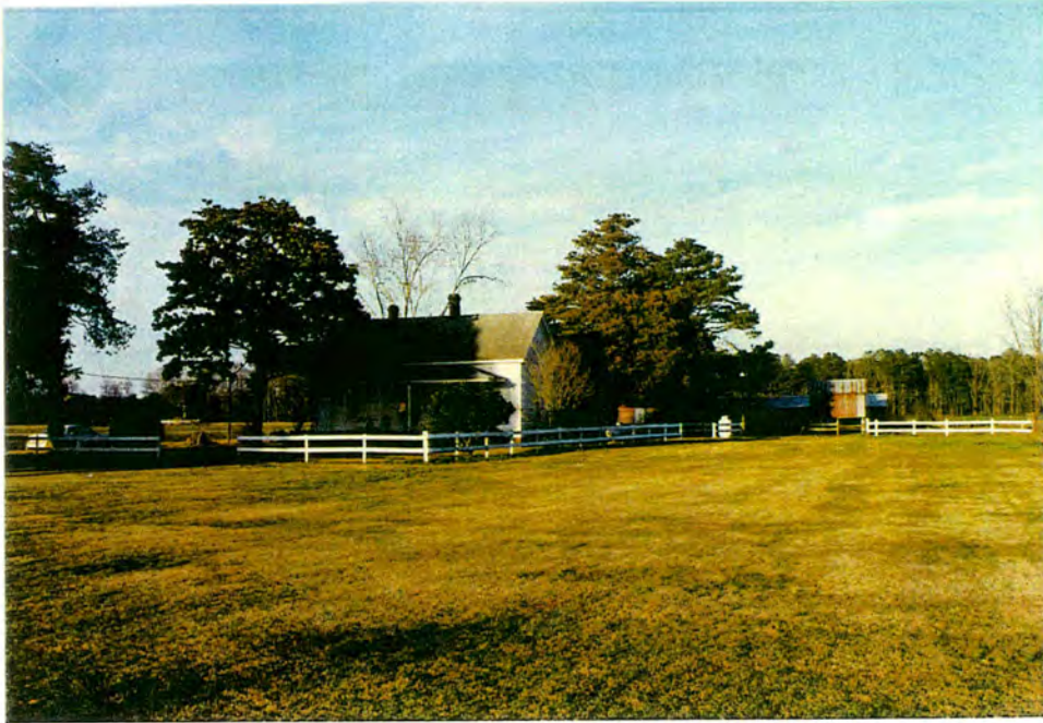
Turner Farms. View of one-story farmhouse from SW (#41).
