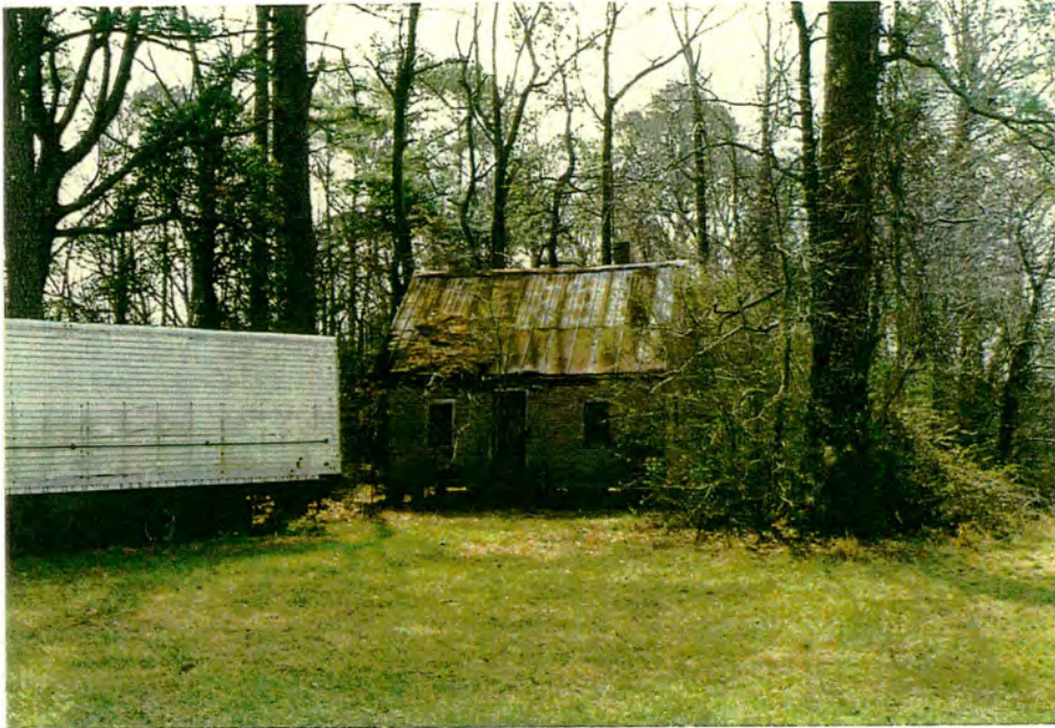
Homestead Farm. Tenant house #1 (on south side of US 64, east of SR 1120).
