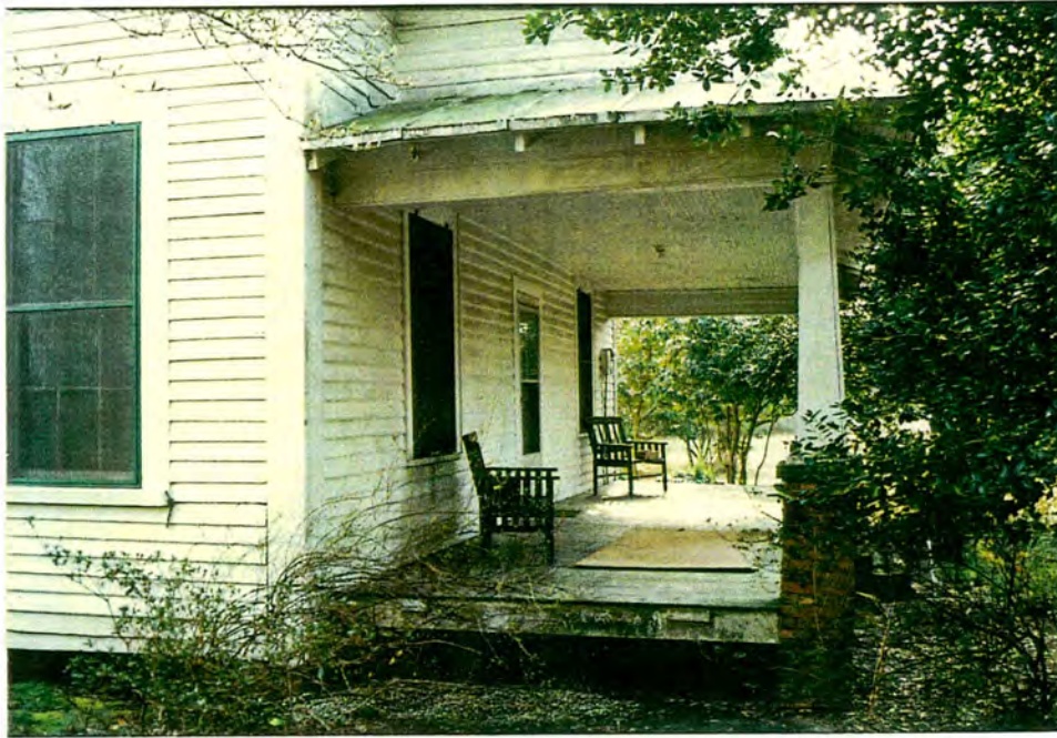
Former Schoolhouse. Front porch.
