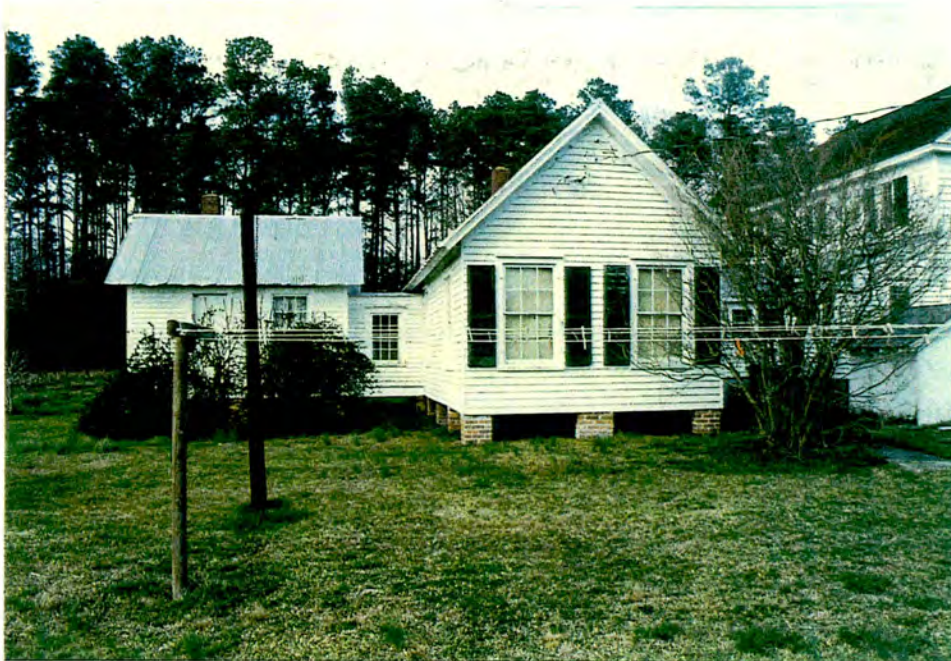
Smithson House. View N of rear additions.
