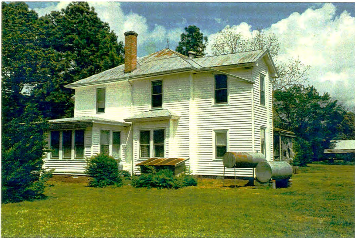
Tarkenten House. West elevation.
