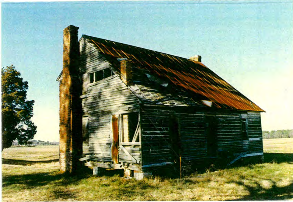
Homestead Farm. View of Thompson House from SW.
