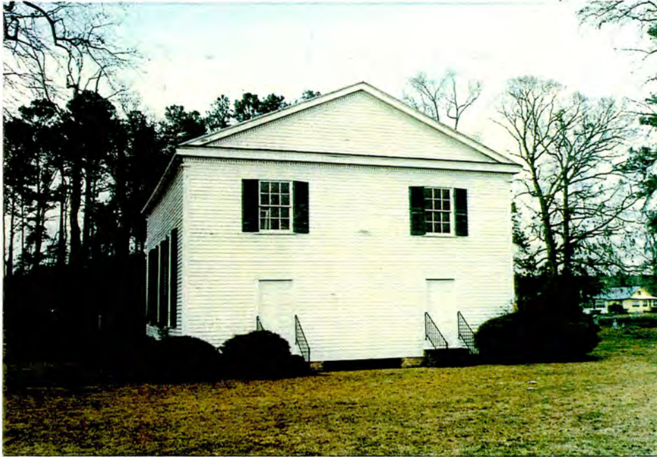
Rehoboth Methodist Church. South elevation.
