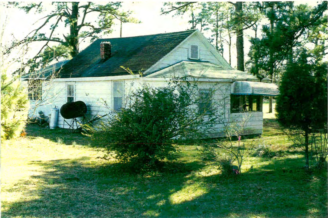
192. House (#1 in June 1, 1996 report)
