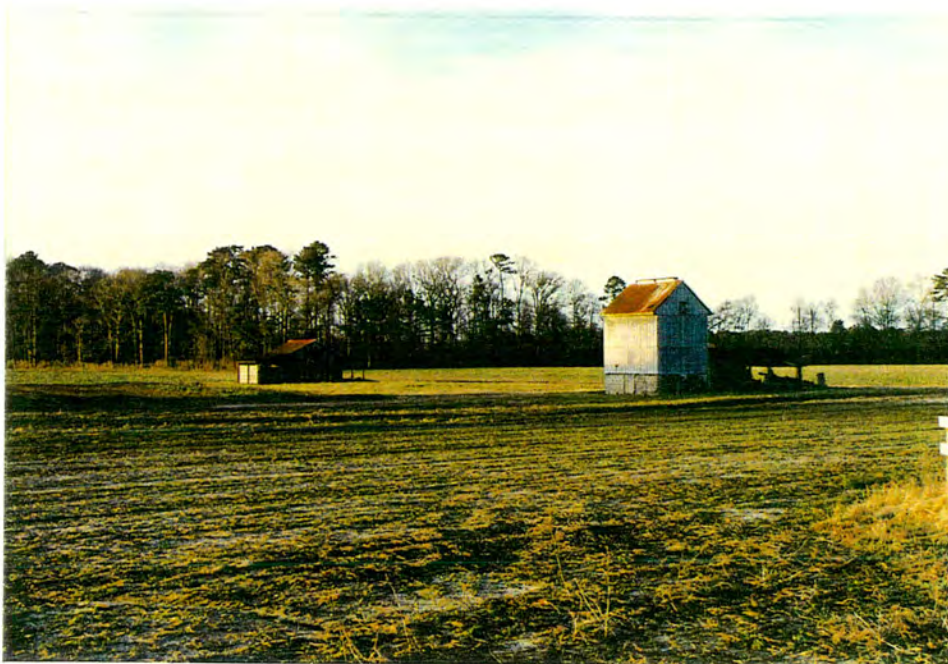
Turner Farms. Outbuildings of northern farm complex (#42).
