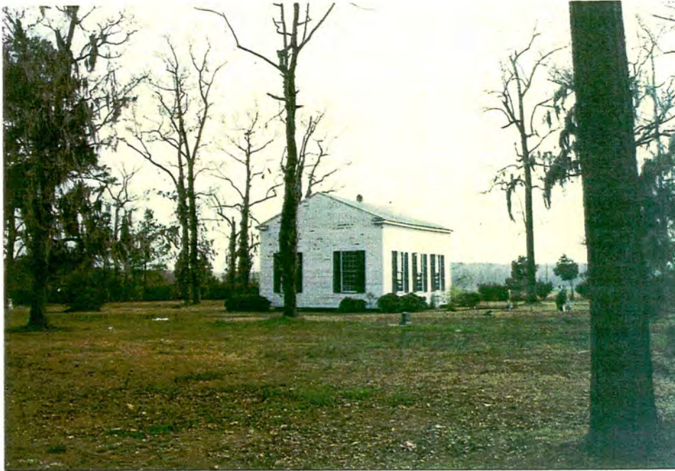
Rehoboth Methodist Church. View from US 64.
