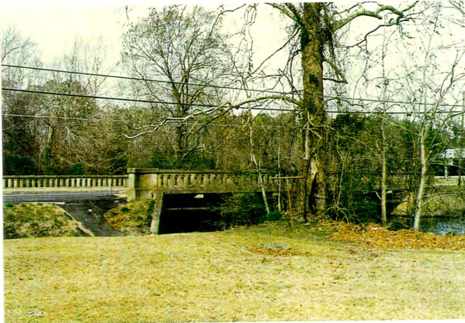
Roper H.D. Kendrick's Creek Bridge (#51). Built 1935.
