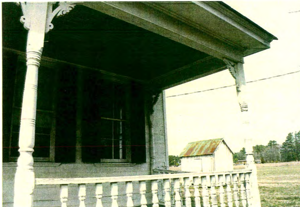
Downing-Spruill House. First-floor windows on SE corner.
