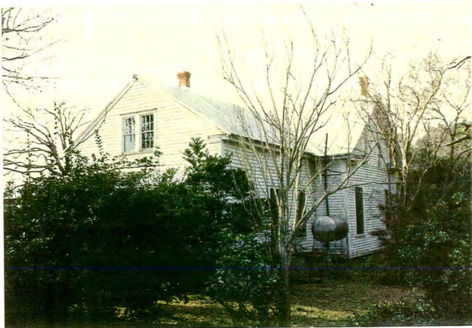
Former Schoolhouse. View from SE.
