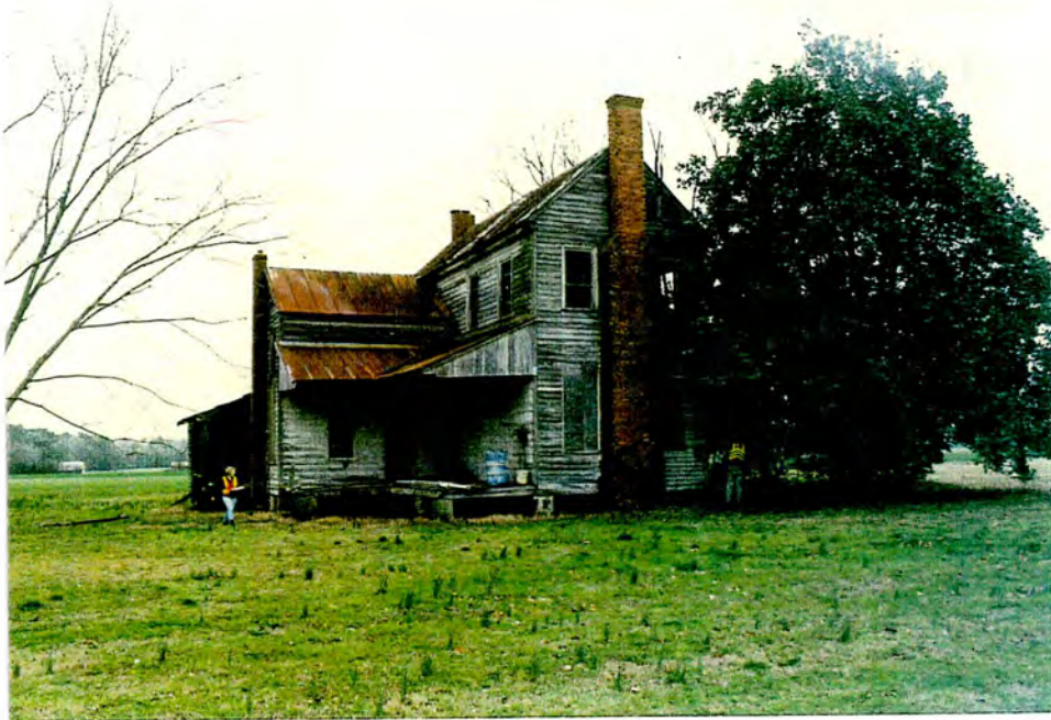
William R. Chesson House. View from NE.
