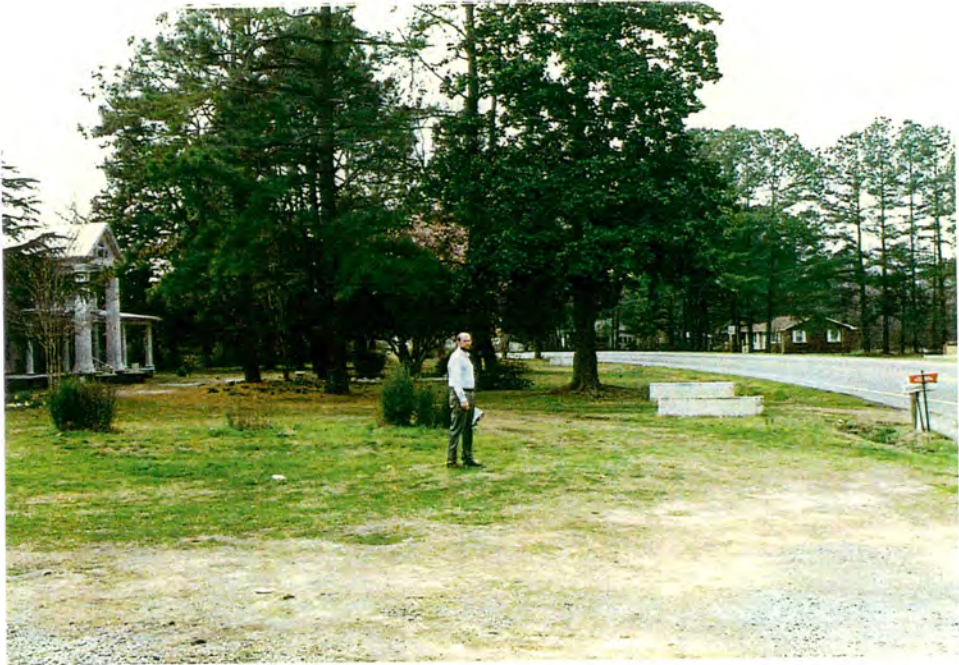
Tarkenten House. View W along US 64. ED standing at edge of ROW.
