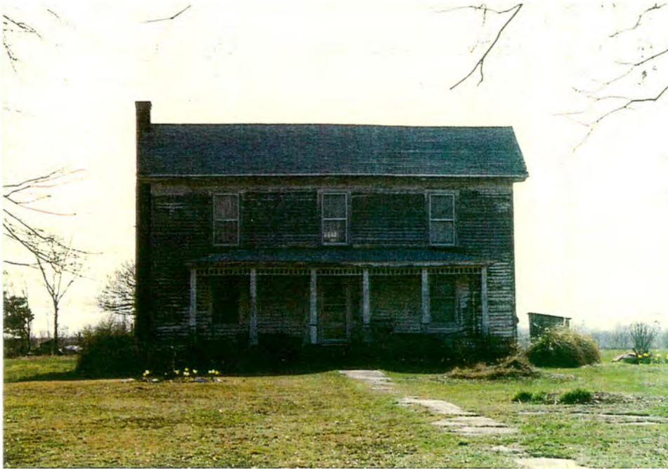
Pritchard Farm. North elevation of farmhouse.
