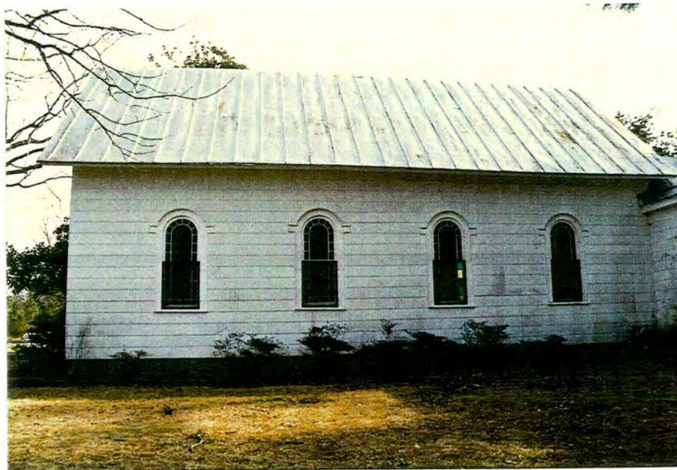
Pleasant Grove Methodist Church. North elevation (facing SR 1300).
