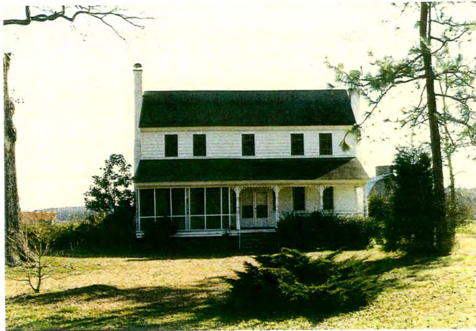
Hassell House. North elevation.
