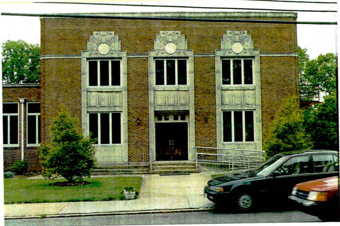
#11, Entrance Facade, former Ardmore Elementary School.
