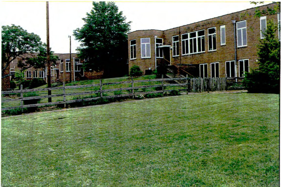
#12. Rear Elevation, former Ardmore Elementary School.
