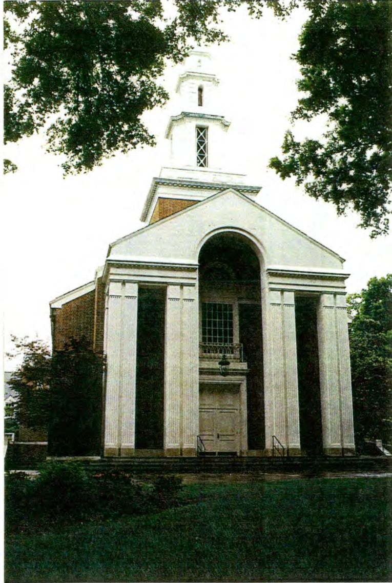
#22. Highland Presbyterian Church. Southwest corner of Cloverdale Avenue and Magnolia Street.
