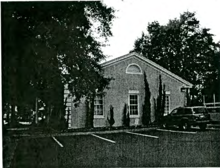
59. Durham Life Insurance Company Building, 331 High Street
