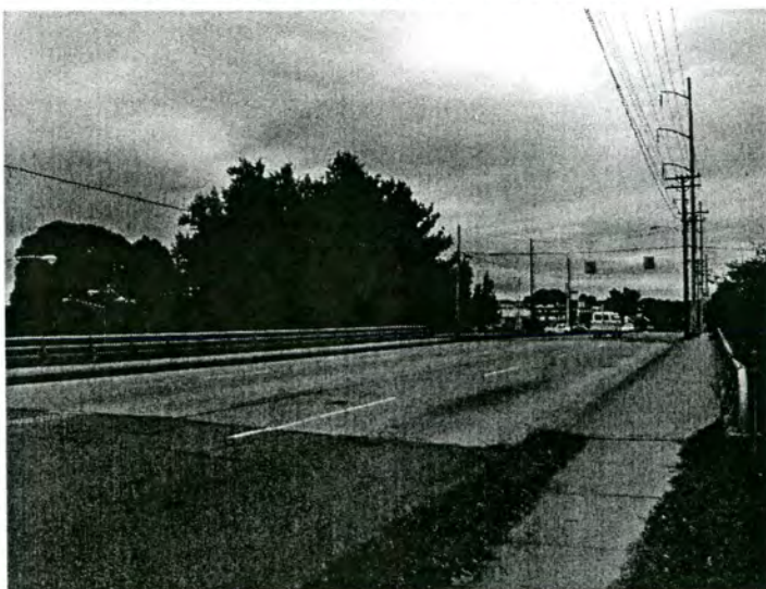
49. Broad Street Bridge over I-40 Business
