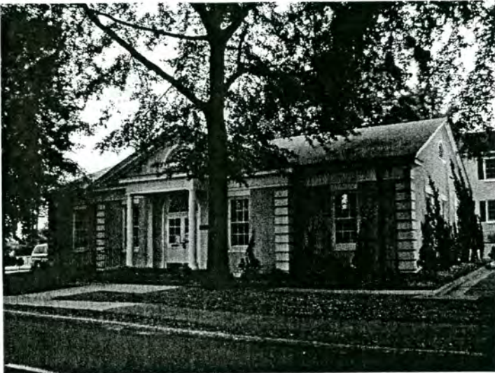
59. Durham Life Insurance Company Building, 331 High Street
