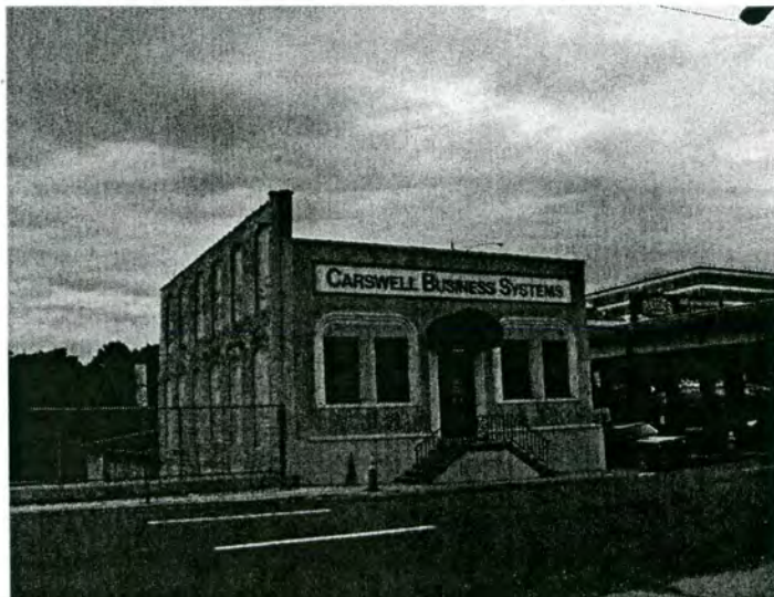
69. Carswell Building Systems, 210 S. Liberty Street
