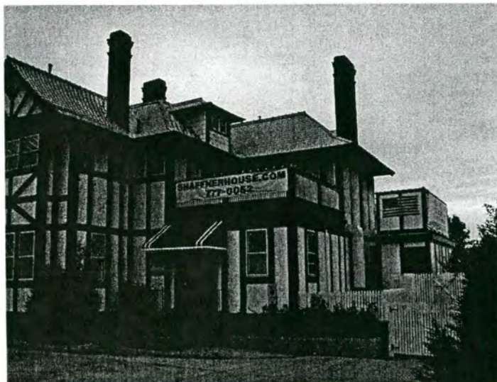
55. Henry F. Shaffner House (SL) 403 High Street
