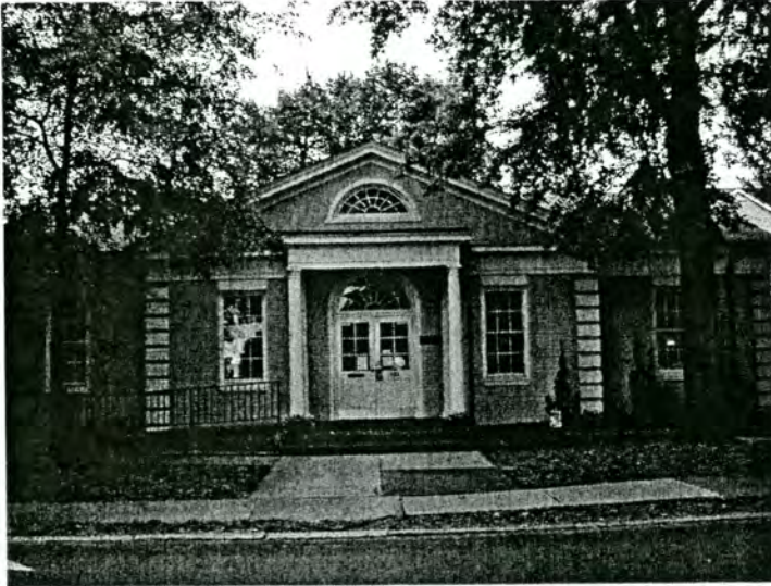
59. Durham Life Insurance Company Building, 331 High Street
