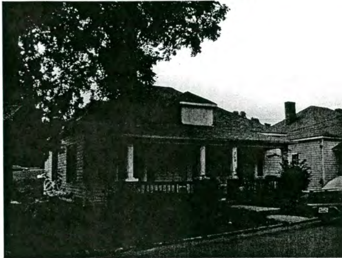
15. House, 308 Gregory Street
