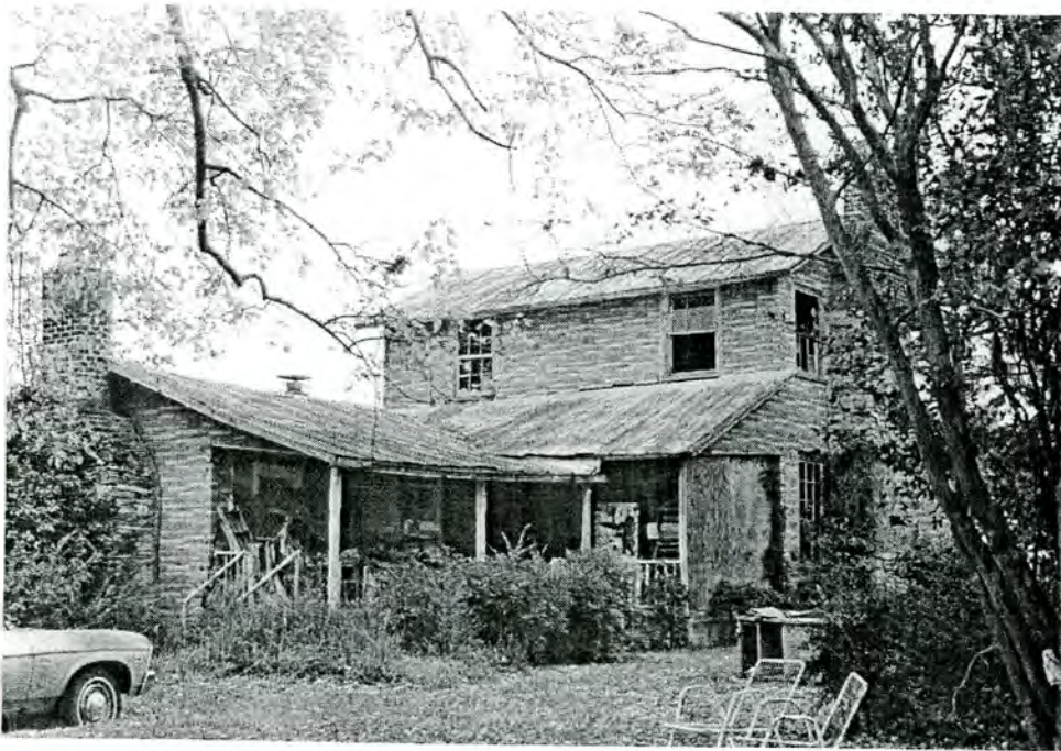
Plate 31. Varner Place, Rear (South) Elevation and Rear Ell, Looking Northwest.
