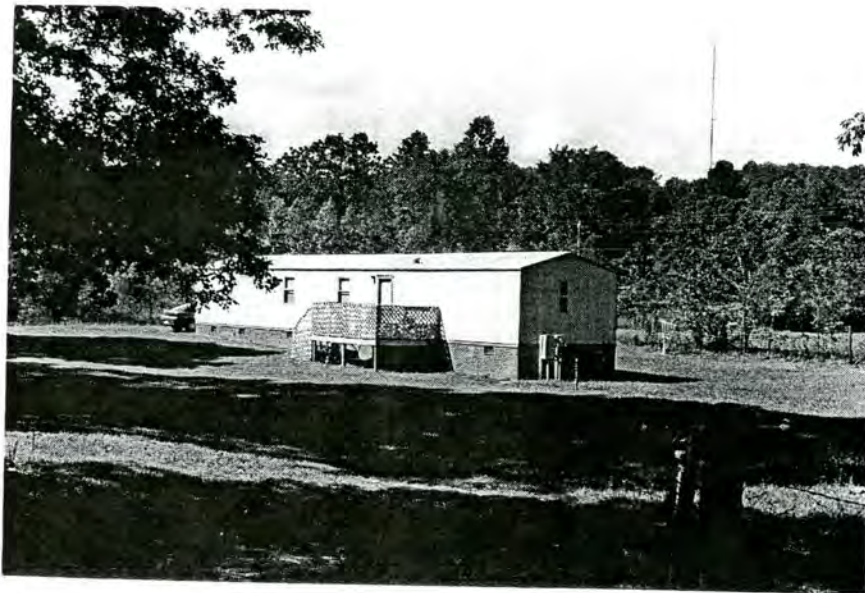
Plate 18. Cox-Brown Farm--Mobile Home, Looking West.
