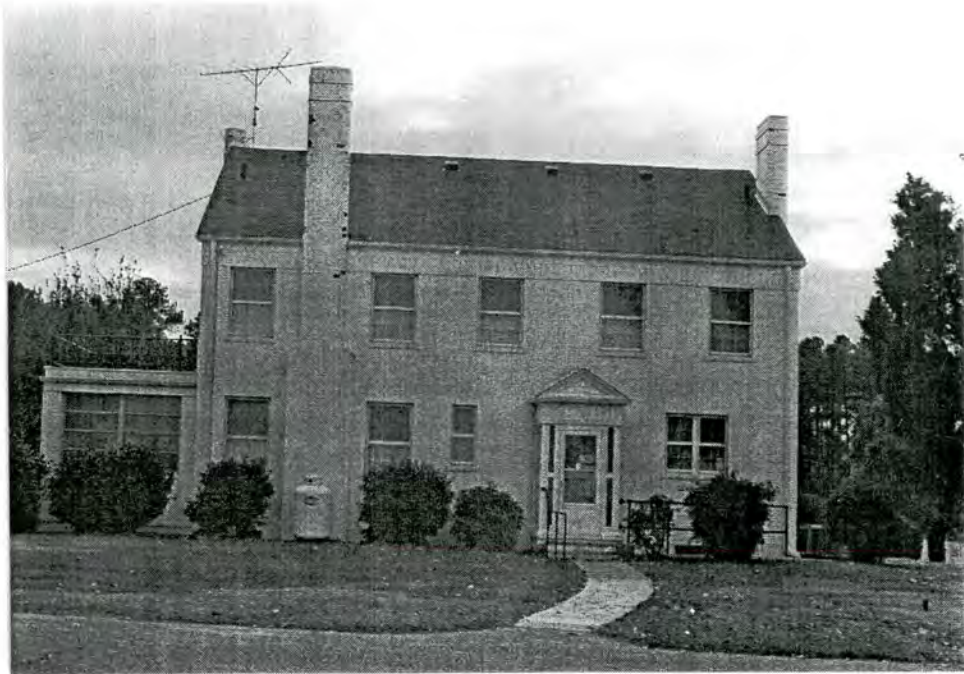
Plate 22. Wrape Farm--Rear Elevation of House, Looking South.
