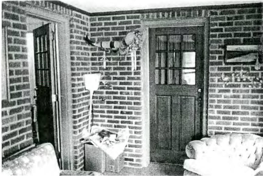
Plate 3. Cox-Brown Farm--House, Entry Doors on Porch, Looking North.
