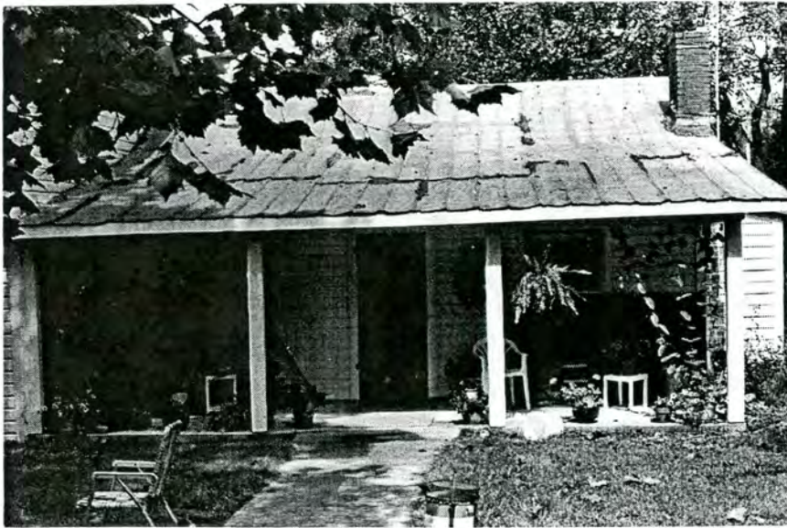
Plate 41. Spoon House, Rear Ell, Looking North.
