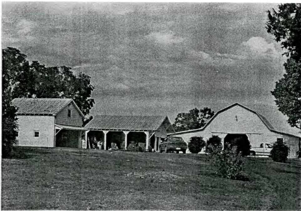
Plate 23. Wrape Farm--Barn, Equipment Shed, and Garage, Looking Northwest.
