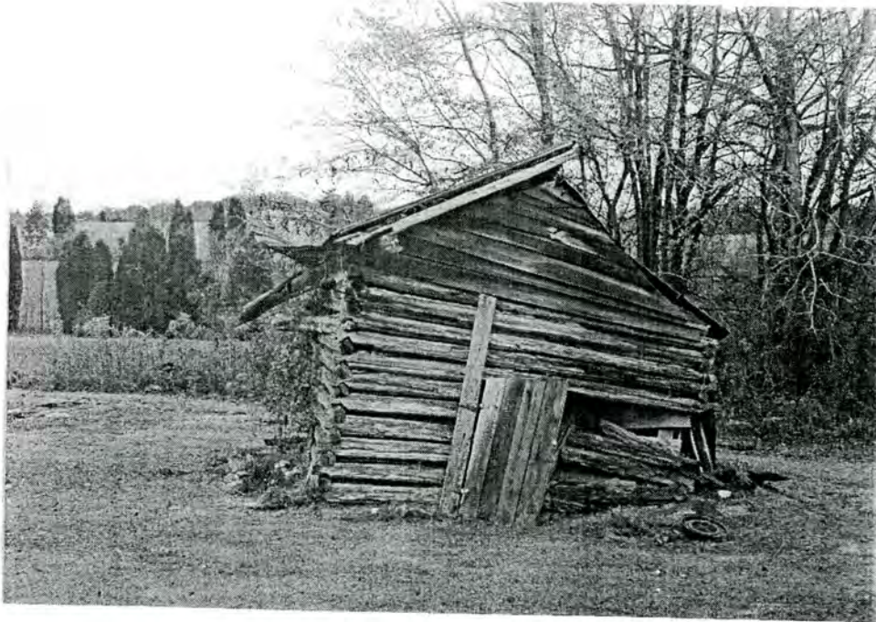
Plate 36. Varner Place, Ruinous Smokehouse, Looking West.
