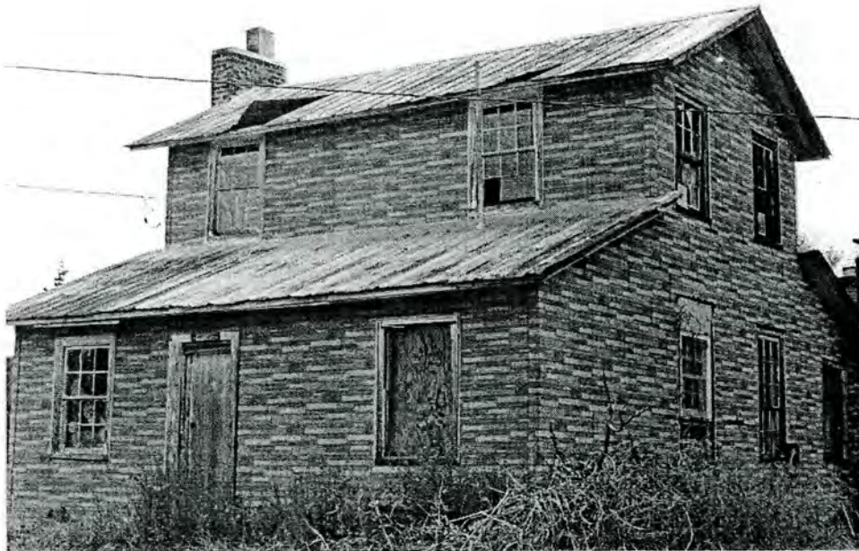
Plate 29. Varner Place, Facade (North) and West Elevation, Looking Southeast.
