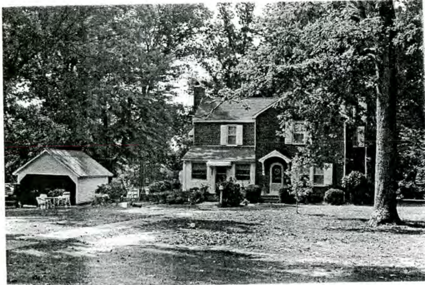
Plate 1. Cox-Brown Farm, House and Setting, Looking Southwest.
