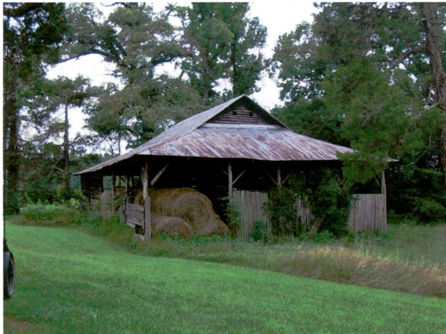
Plate 17. Helper Log Barn (No. 3), Overall View, Looking South.
