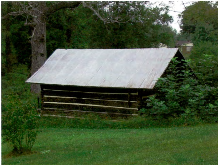
Plate 19. Helper Log Barn (No. 3), Log Smokehouse, Looking Northwest.
