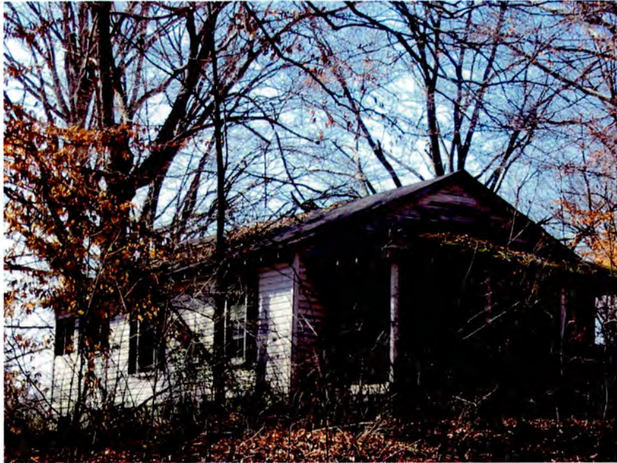
House (No. 27), Looking South.
