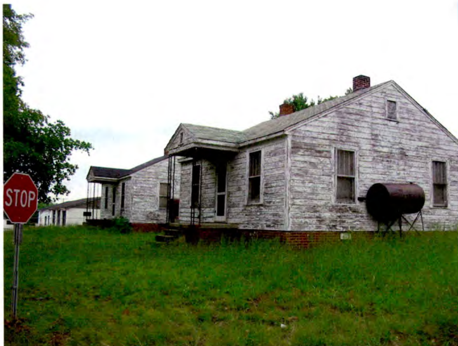
Houses (No. 11), Looking Northeast.
