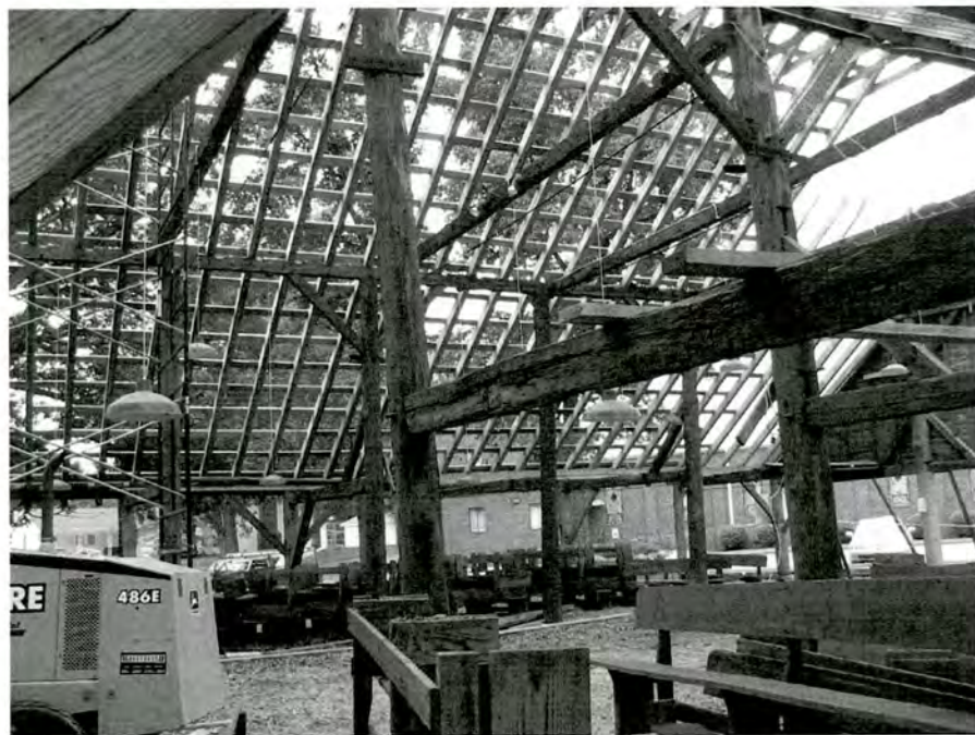
Plate 4. Center Arbor (No. 1), Interior Showing Roof Renovations.
