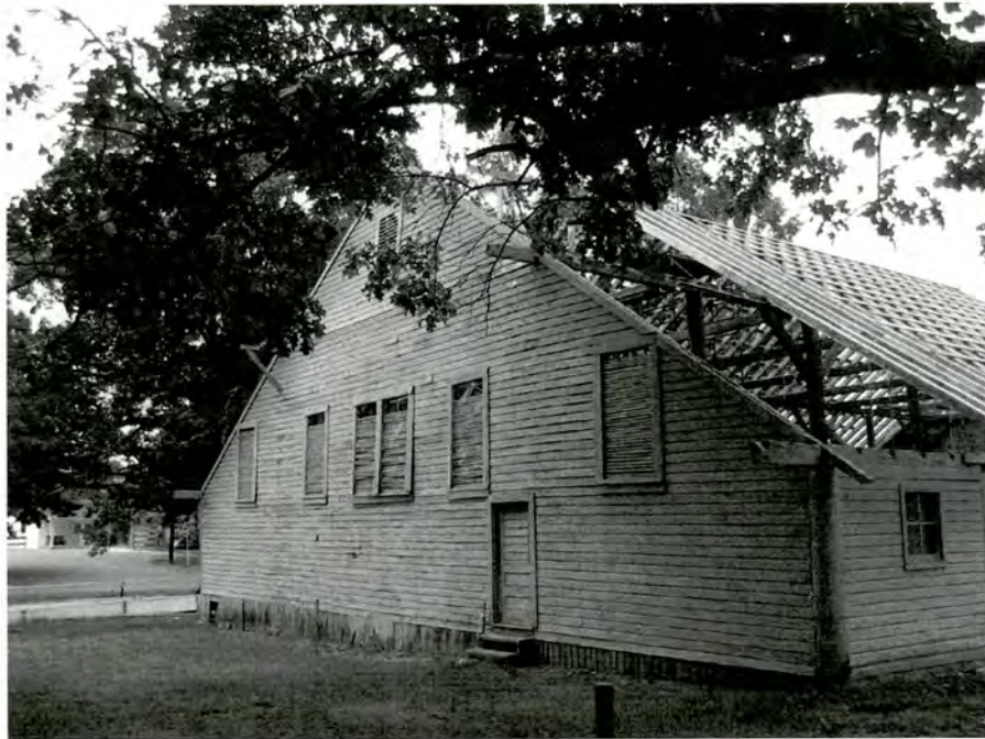
Plate 3. Center Arbor (No. 1), Enclosed Gable End, Looking West.
