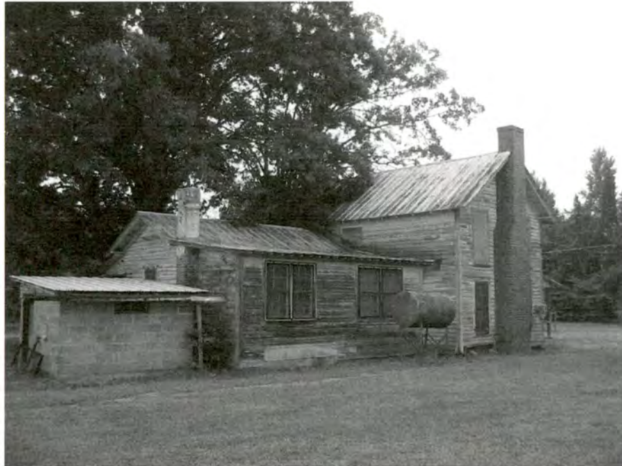
Plate 14 Tutterow House (No. 2), Rear Ell and Side (West) Elevation, Looking South.
