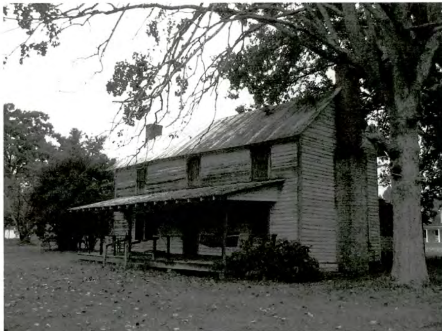
Plate 13. Tutterow House (No. 2), House Façade and Side (East) Elevation, Looking Northwest.
