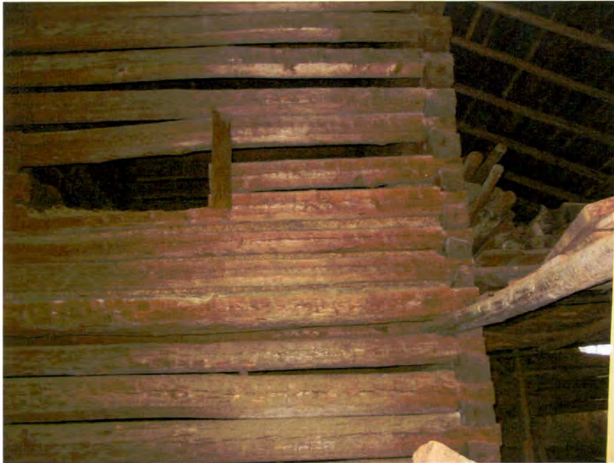
Plate 18. Helper Log Barn (No. 3), Detail of Log Notching.
