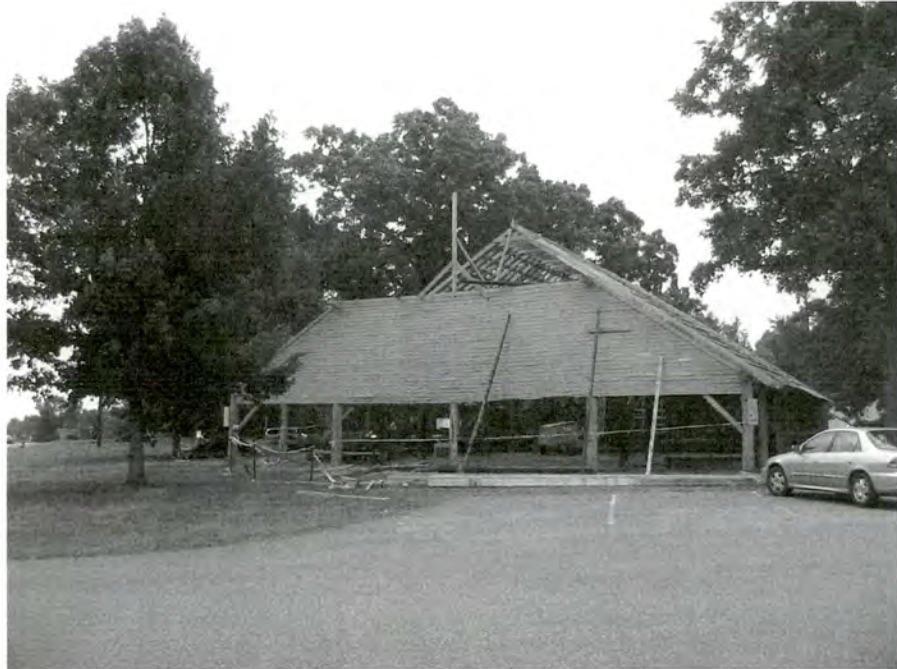
Plate 1. Center Arbor (No. 1), Looking Southeast From Church Parking Lot.
