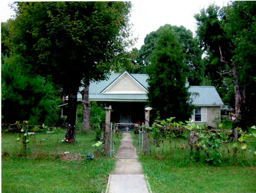
House (No. 8), Looking South.
