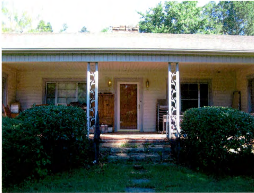
House (No. 16), Looking North.
