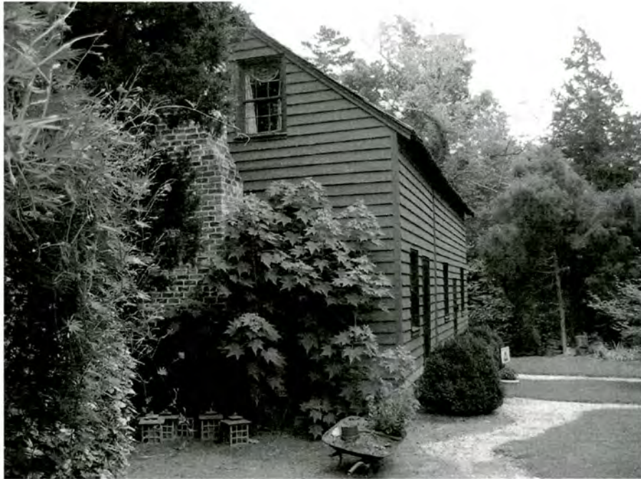
Plate 5. McGuire-Setzer House (No. 10), Looking East.
