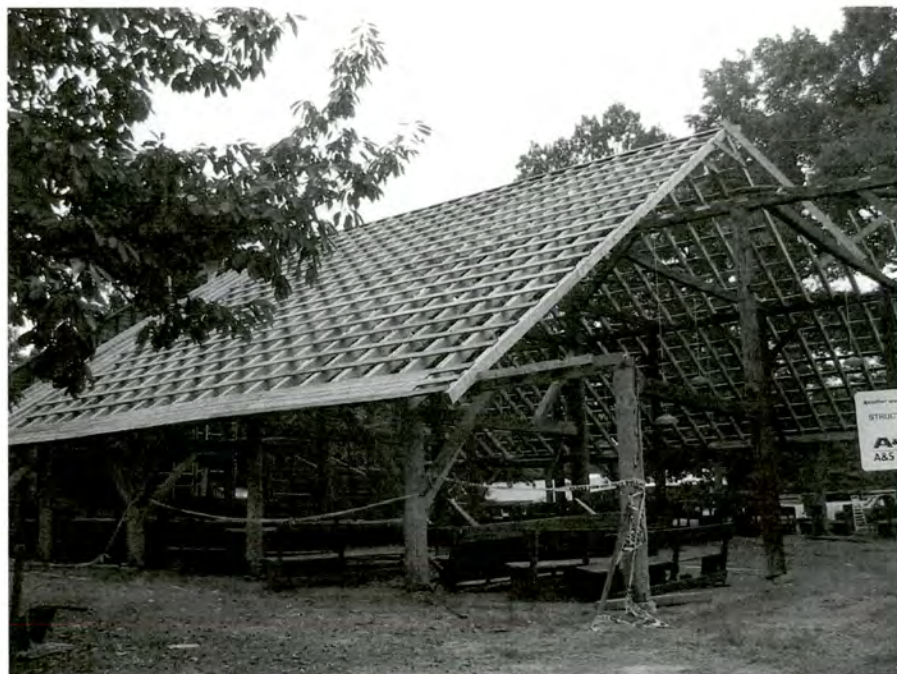
Plate 2. Center Arbor (No. 1), Roof Renovations.
