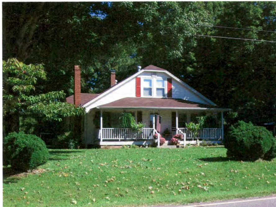
House (No. 17), Looking North.
