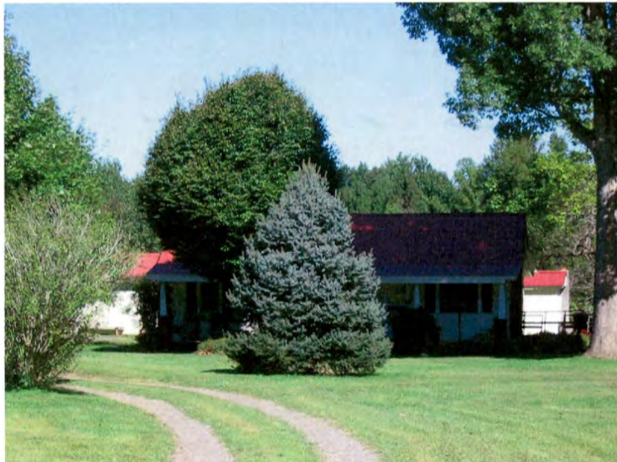
House (No. 18), Looking North.
