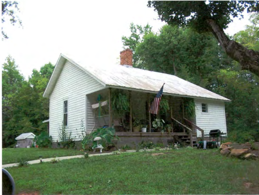
House (No. 12), Looking North.
