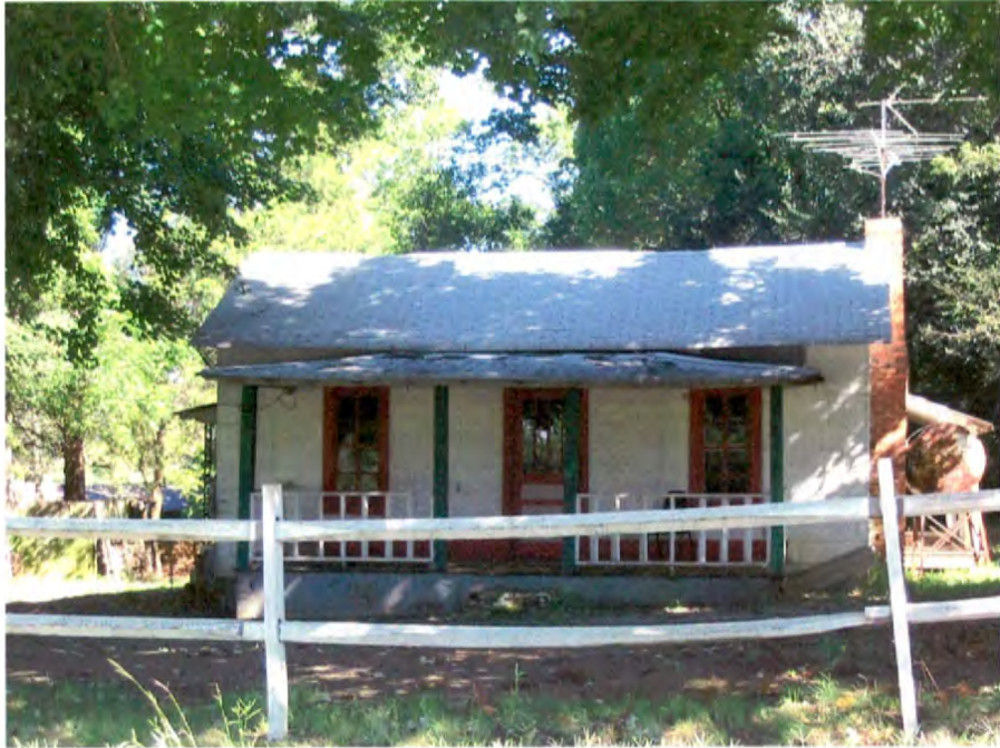
House (No. 19), Looking North.
