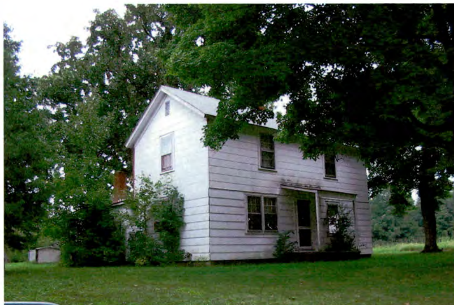
House (No. 5), Looking North.
