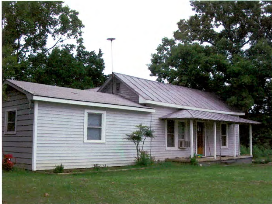
House (No. 4), Looking North.
