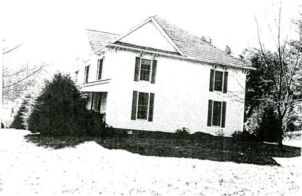
Plate 29: Hoke A. Wagoner House—west side and north front elevations
