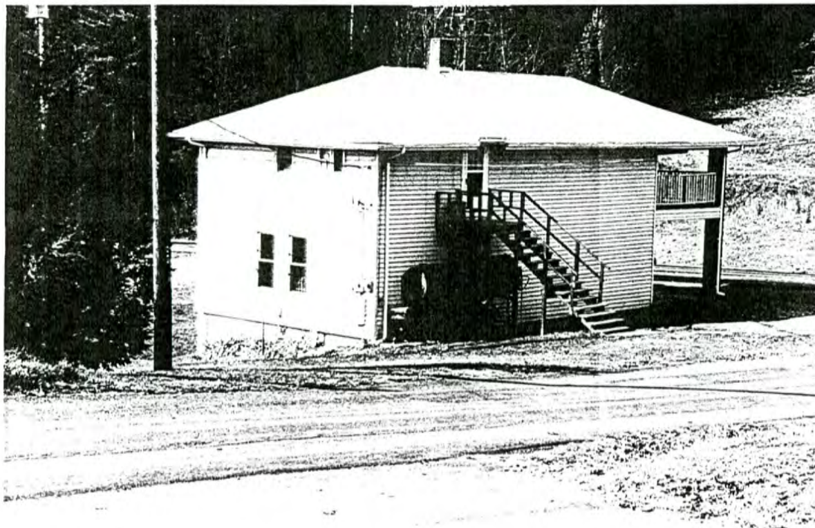
Plate 12: Former Dancy-Maines Store and Post Office—south rear and east side elevations
