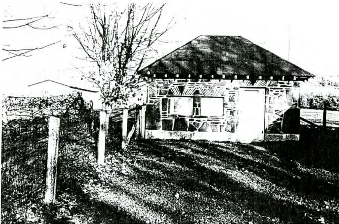
Plate 41: James Edward Witherspoon House—south front elevation of cold cellar
