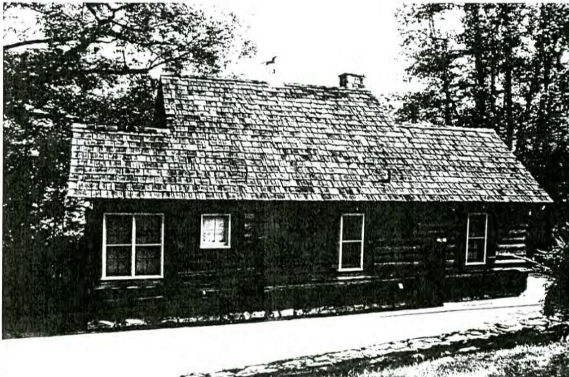
Plate 24: Blevins- Stump House—south rear elevation
