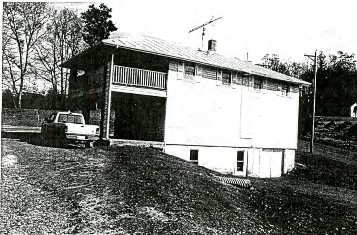
Plate 10: Former Dancy-Maines Store and Post Office—west side and north front elevations
