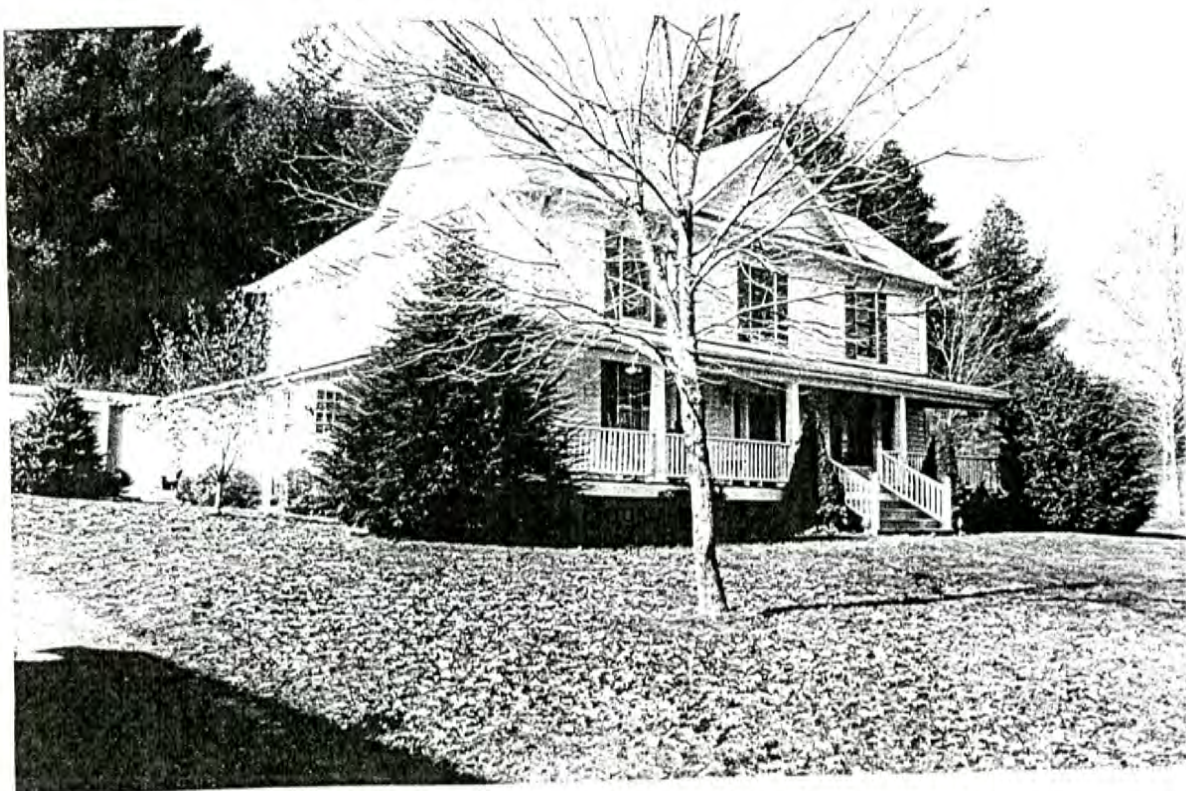
Plate 27: Hoke A. Wagoner House—north front and east side elevations
