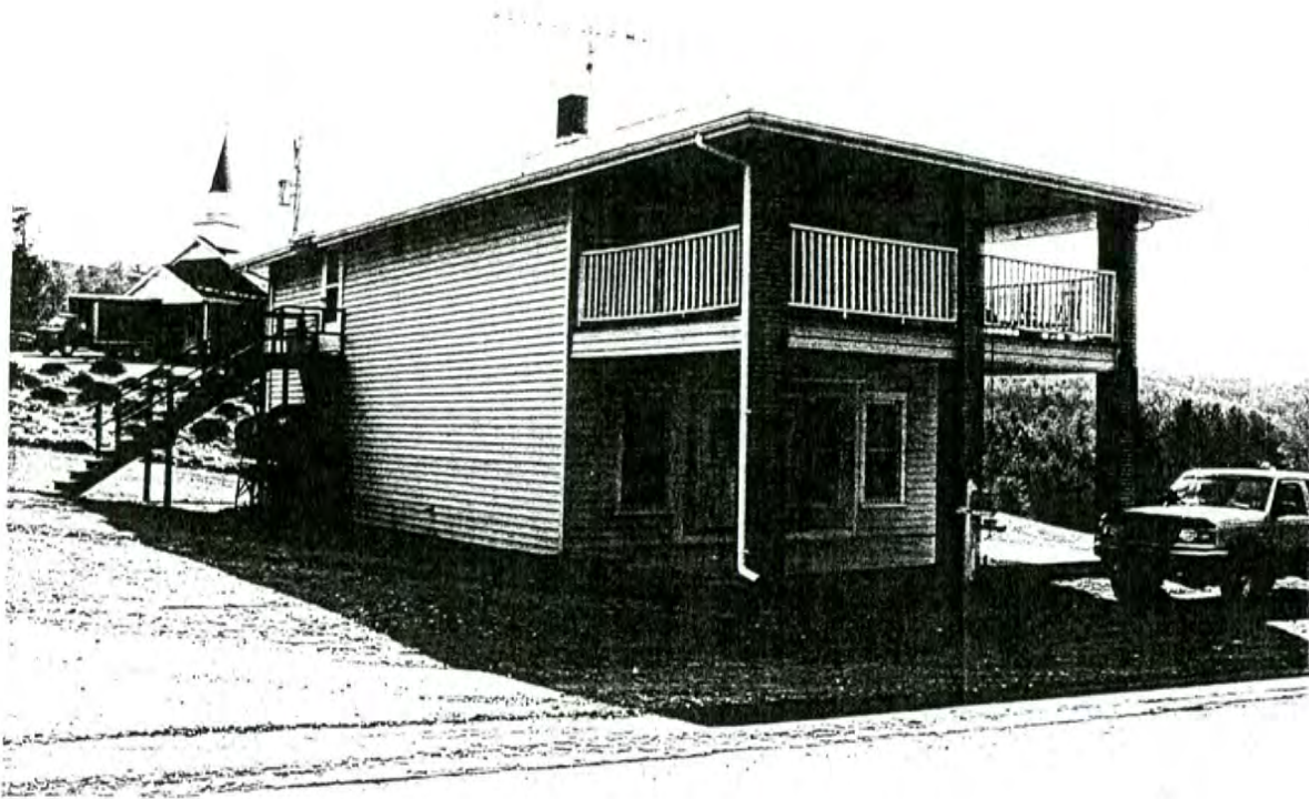
Plate 11: Former Dancy-Maines Store and Post Office—east side and north front elevations
