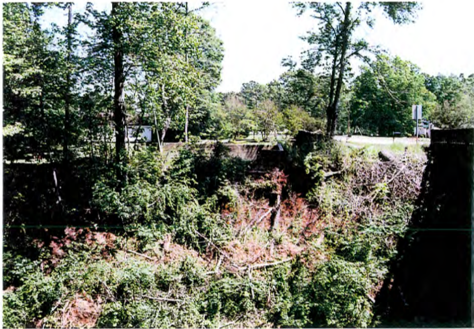
Figure 14: Dry kiln foundations
