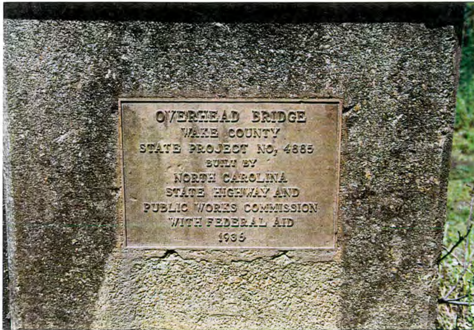
Figure 5: Bridge No. 462, detail, bridge plate
