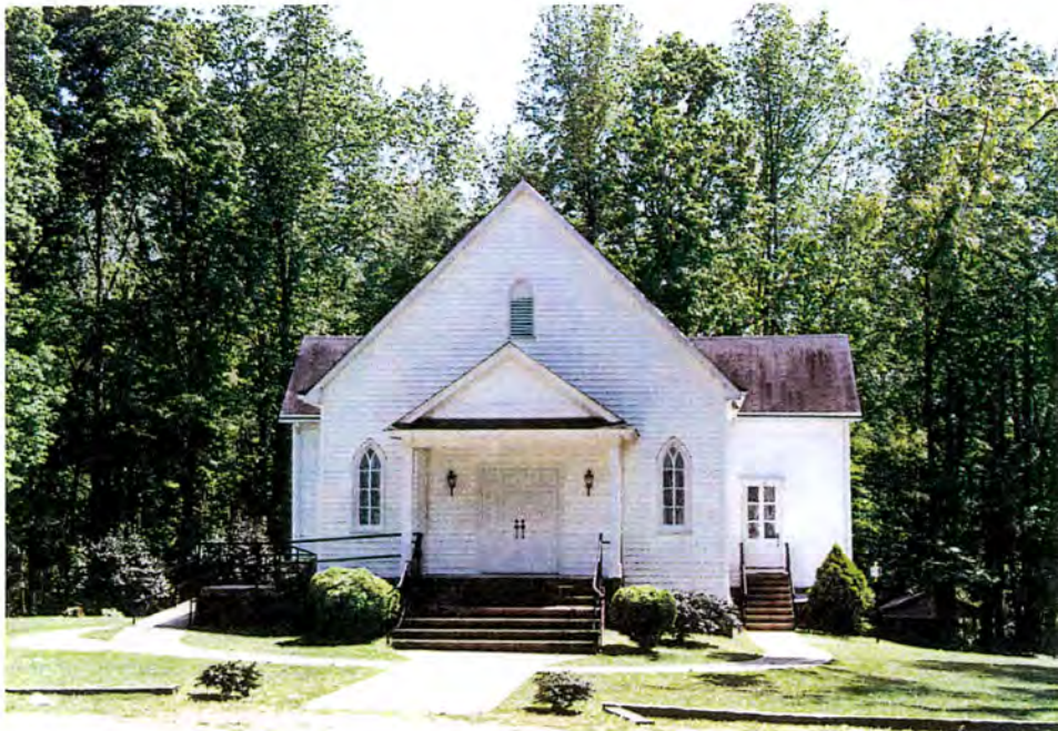
Figure 6: Wentworth Christian Church (WA 1220), facade
