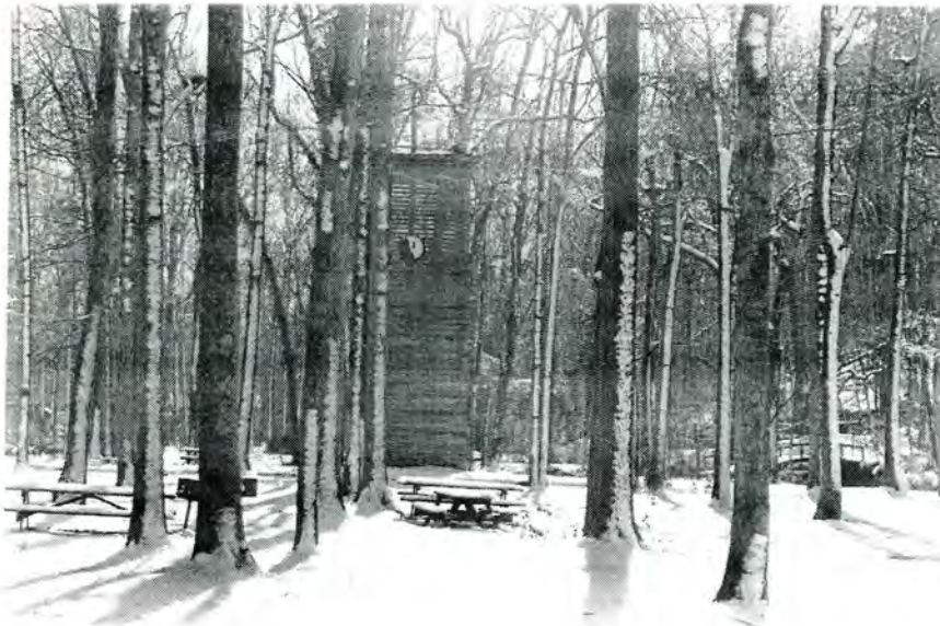
Plate 6. Rock Creek Park, Rappelling Tower, Looking South.
