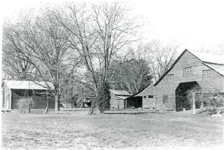
Plate 11. Hatley Farm, Farm Complex, Looking West From ca. 1910 Barn.
