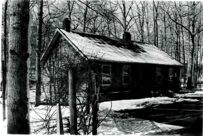
Plate 5. Rock Creek Park, Park Administration Building, Looking Northwest.
