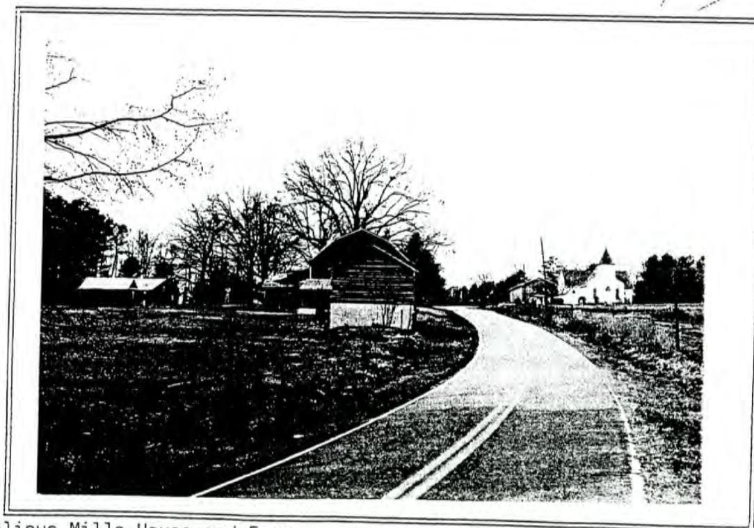
Alious Mills House and Farm View from SR 1615
