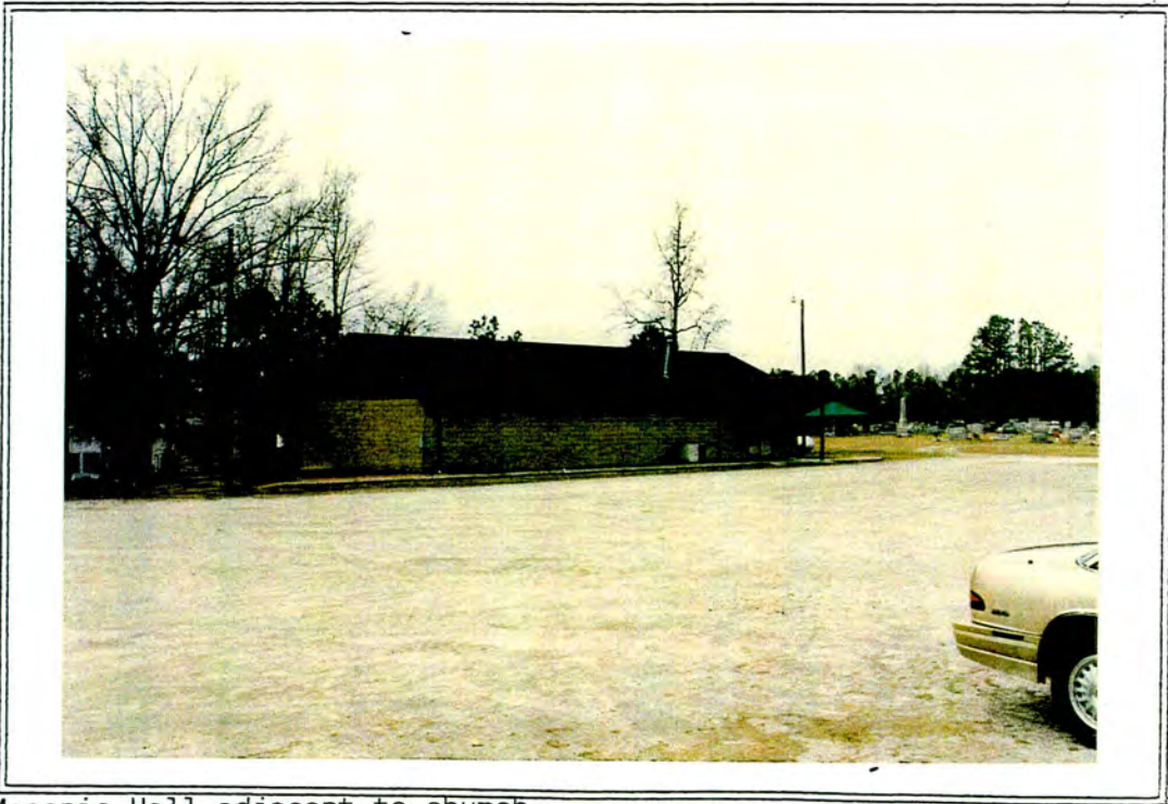
Masonic Hall adjacent to church (Noncontributing structure)
