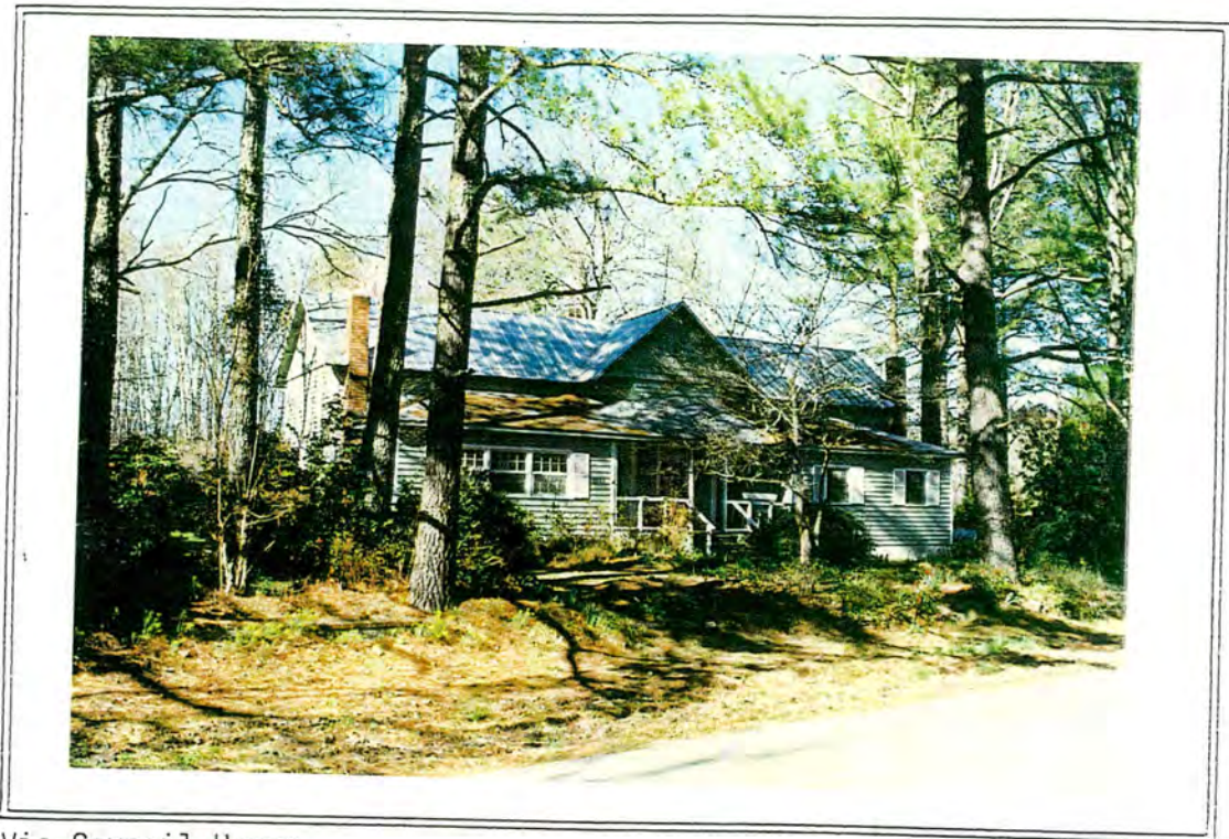
Vic Council House
