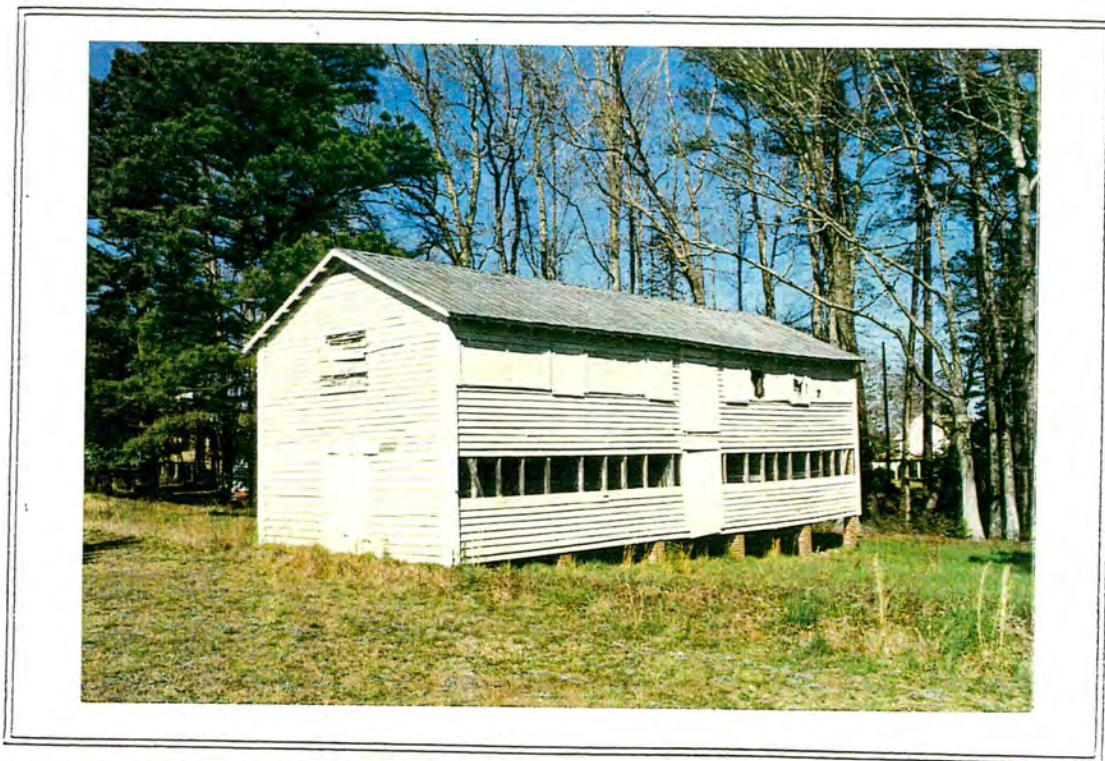
Stable located behind 1930's House
