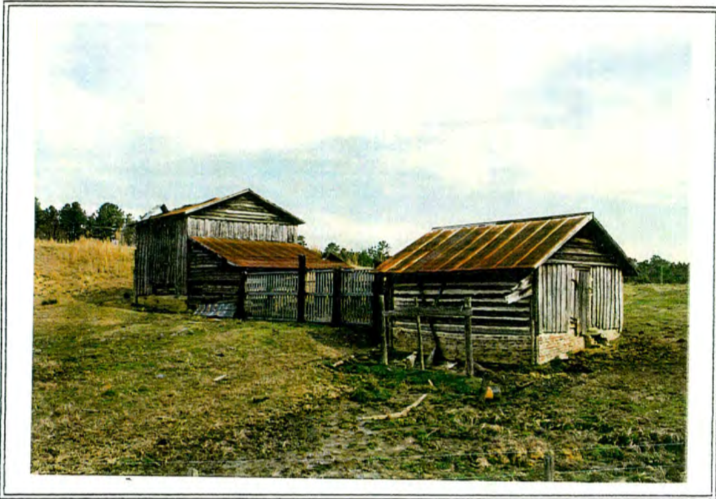
Alious Mills Farm Outbuildings located on East side of SR 1615
